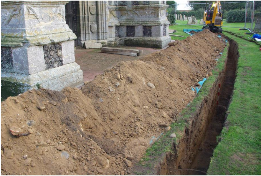
Plate 1: Trench 1, W of tower, looking S, 0.5m scale
