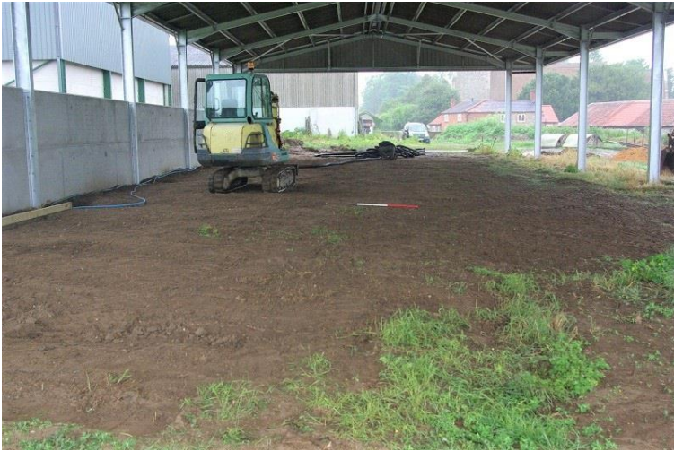
Plate 9: Area 17 within new cattle shed, looking NNW, 1m scale
