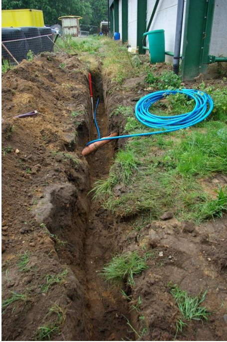
Plate12: Trench 16, looking W, 1m scale
