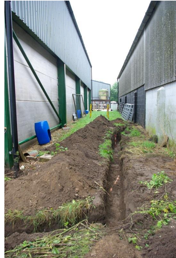
Plate 11: Trench 15 between existing buildings, looking W, 0.5m scale
