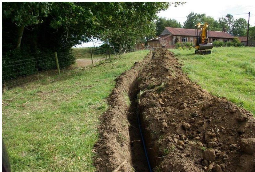
Plate 2: Trench 6, looking ENE, showing connection point at Church Lane
