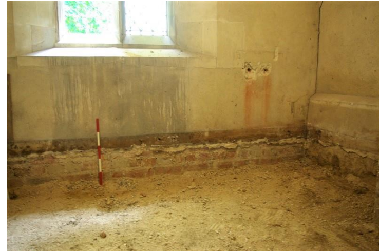
Plate 15: Vestry; floor level lowered, deposit [20], looking WNW, 0.5m scale
