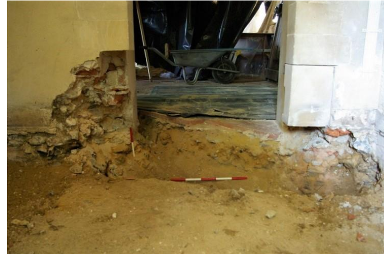
Plate 17: Vestry; floor level lowered and threshold removed, looking E, 0.5m scale
