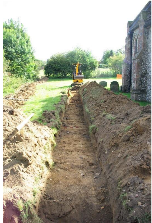
Plate 11: Trenches 10 and 3 (to left); looking E, 0.5m scale
