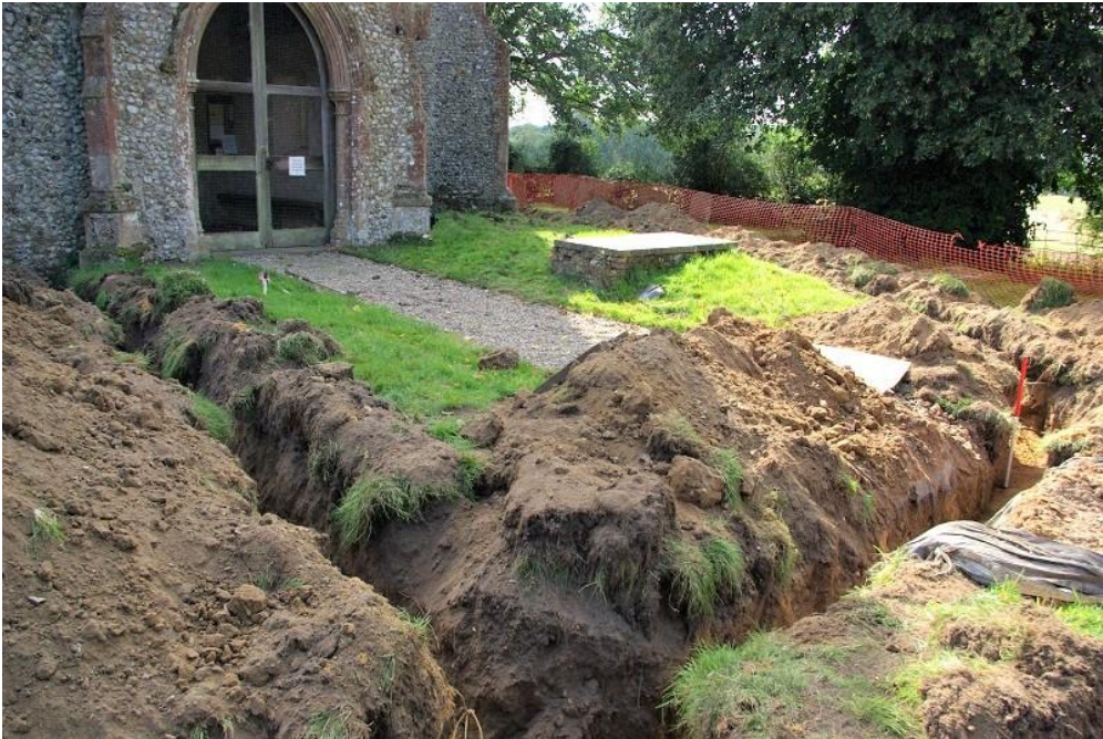
Plate 5: Trenches 1 and 3, looking NW, 1m scale
