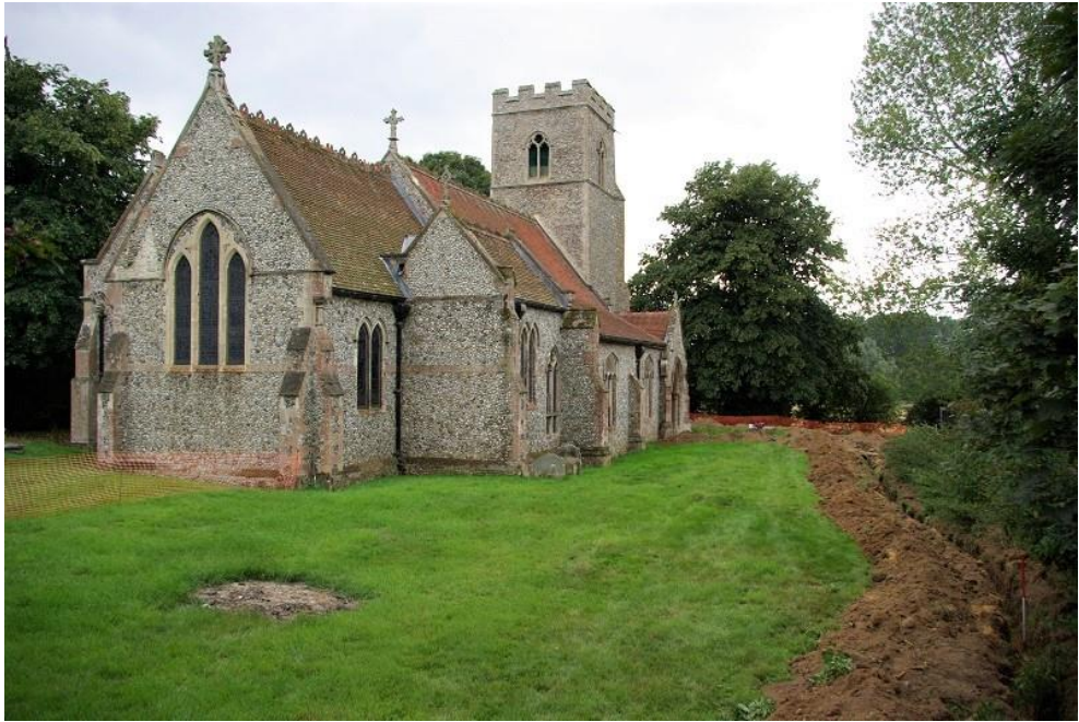
Plate 4: Trench 3, looking E, 1m scale
