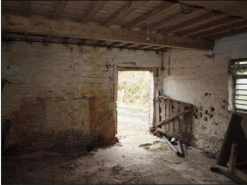
Plate 28: Interior of west stable room
