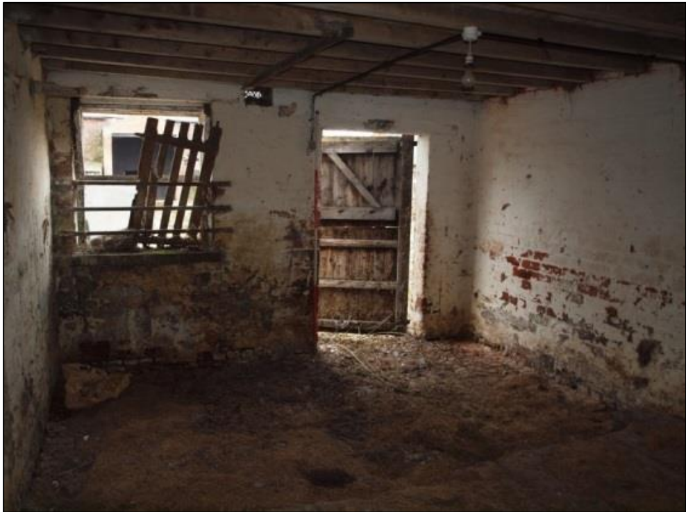
Plate 58: Interior of northern stable room
