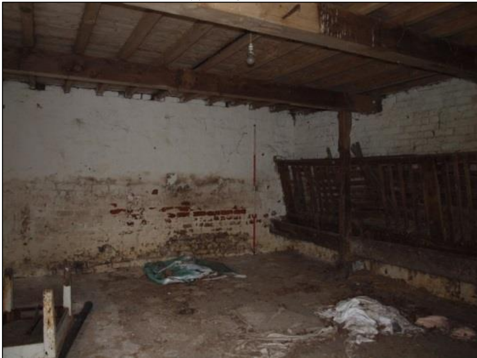
Plate 27: Interior of west stable room
