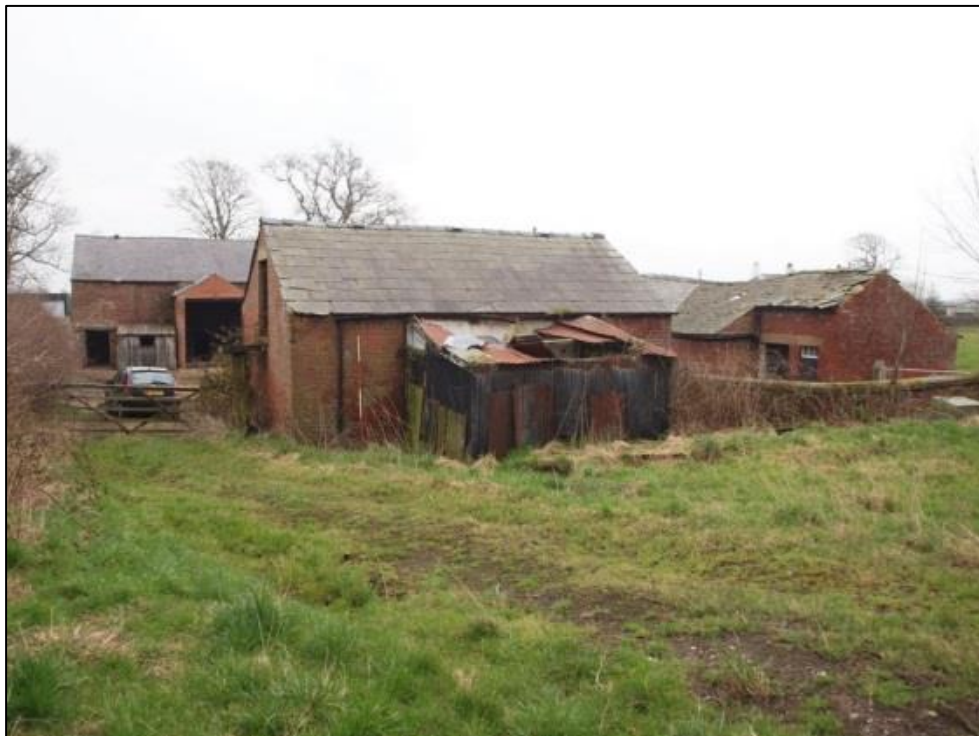
Plate 7: Rear of two bay stable with barn (left) and shippon (right) beyond
