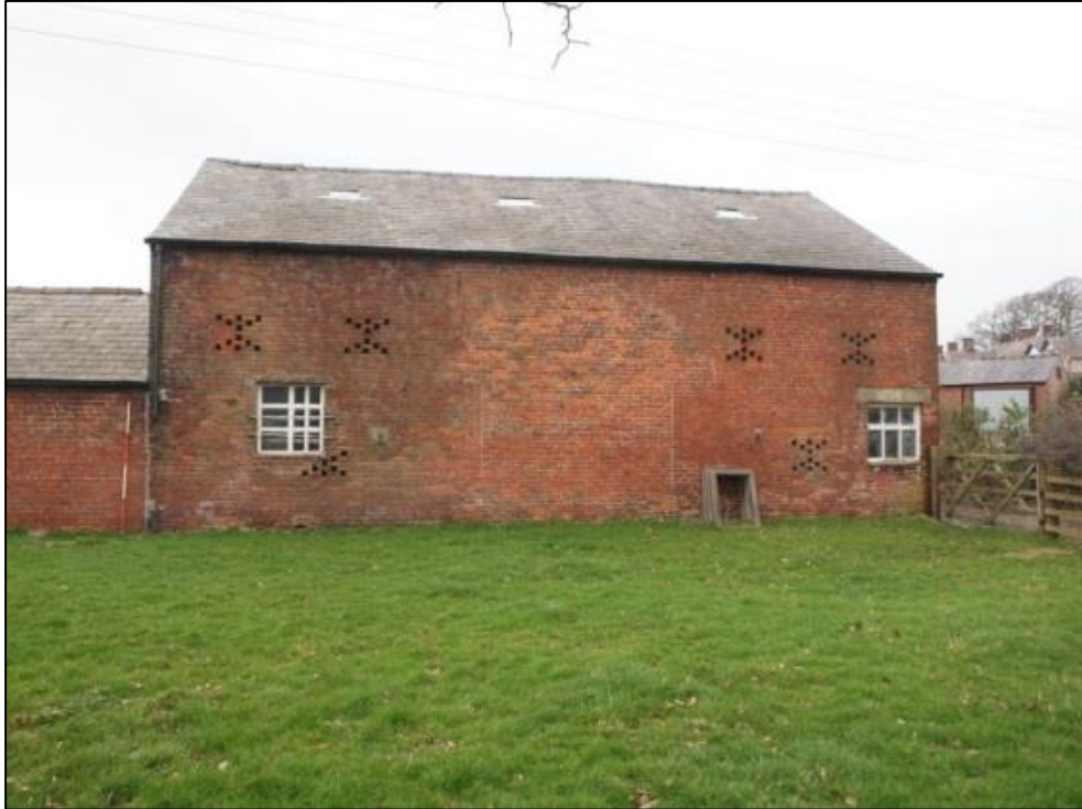
Plate 14: East elevation showing blocked doorway and inserted windows
