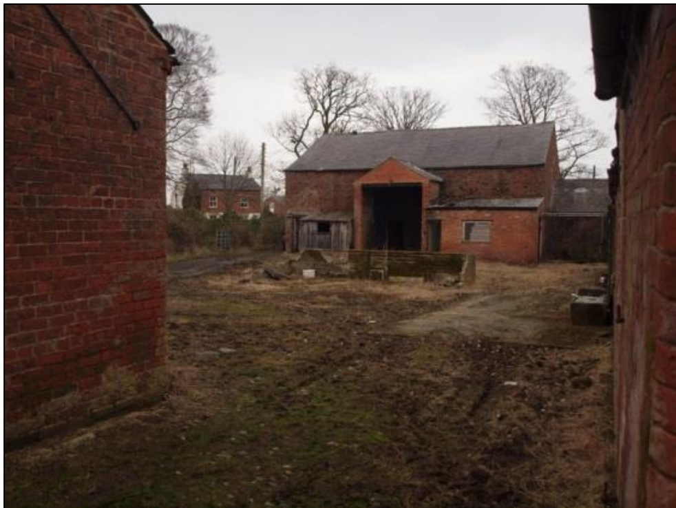
Plate 3: Yard as viewed from the east, with the gable of the two bay stable (left) and barn (centre).
