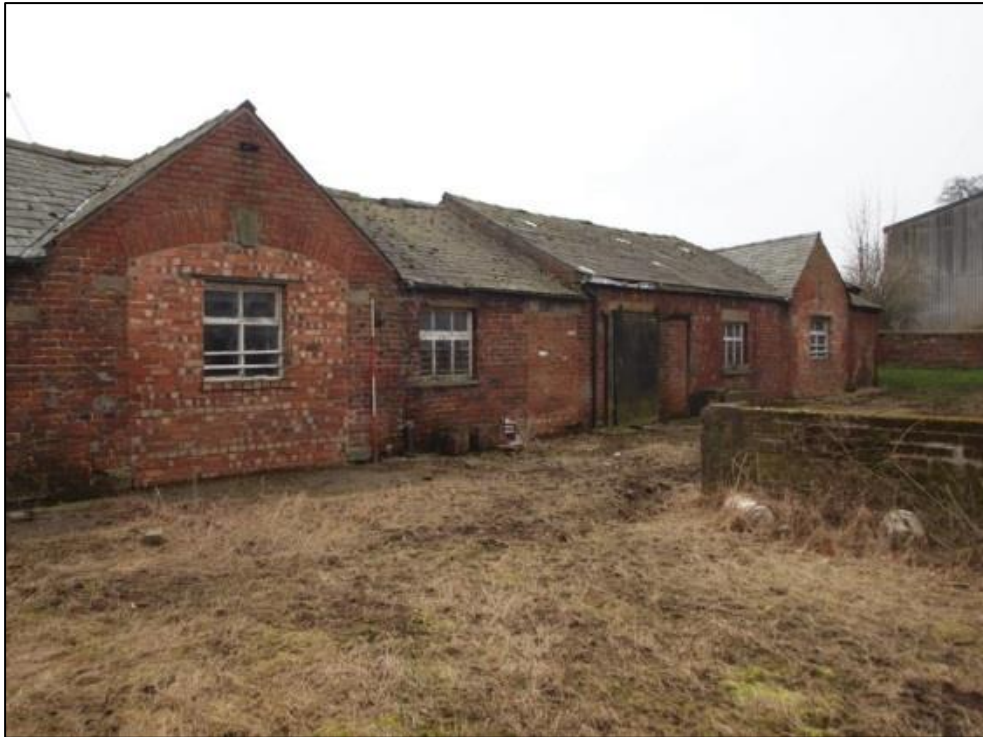
Plate 33: West end of North elevation showing both gables and blocked doorway
