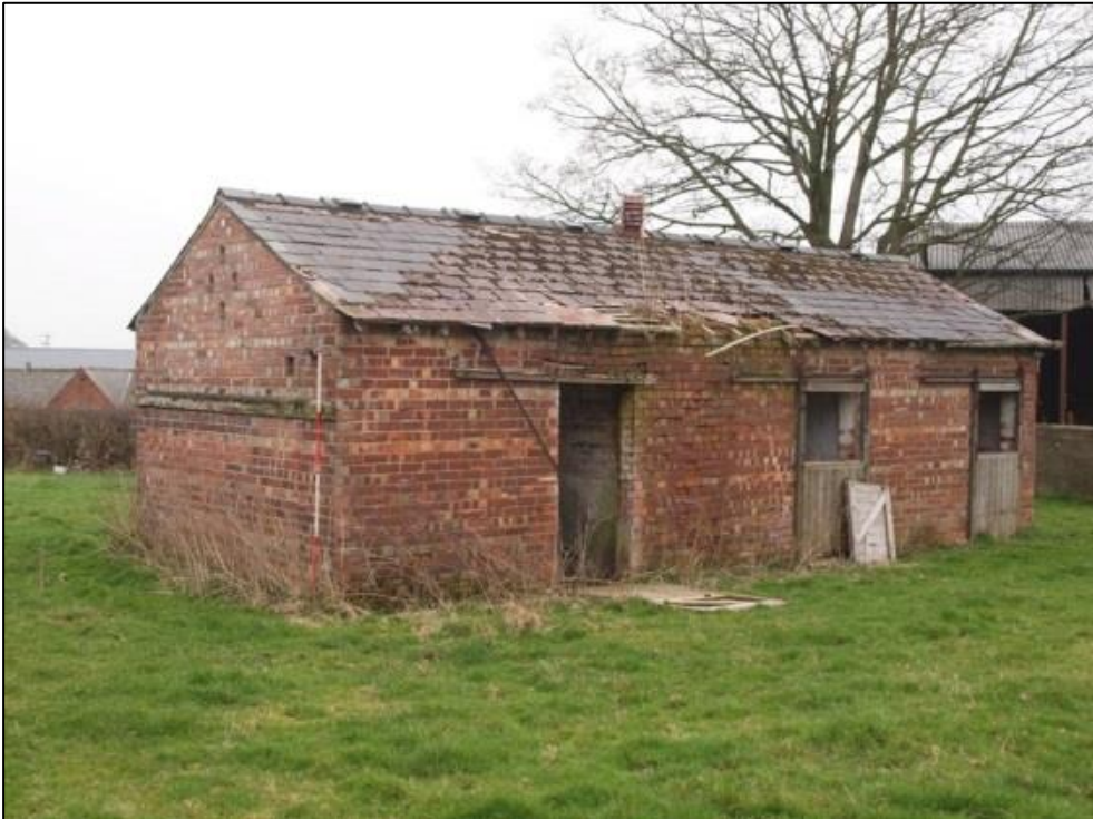
Plate 61: West (front) elevation and north gable
