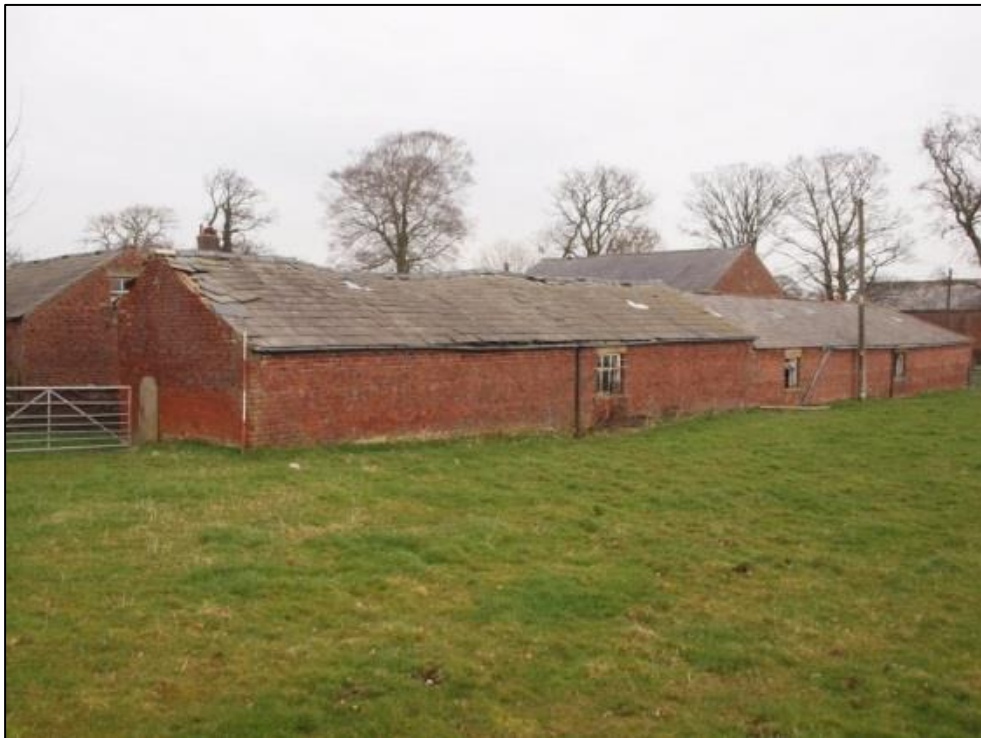
Plate 37: West gable and wet end of south elevation
