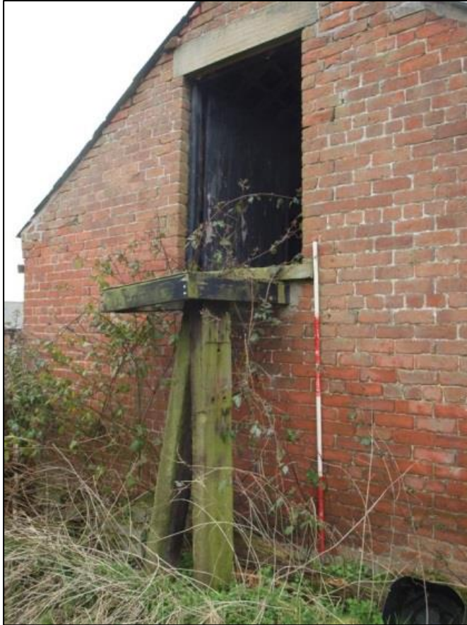
Plate 55: Detail of doorway and remains of timber stairs
