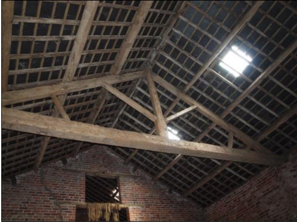
Plate 24: Detail of king post truss
