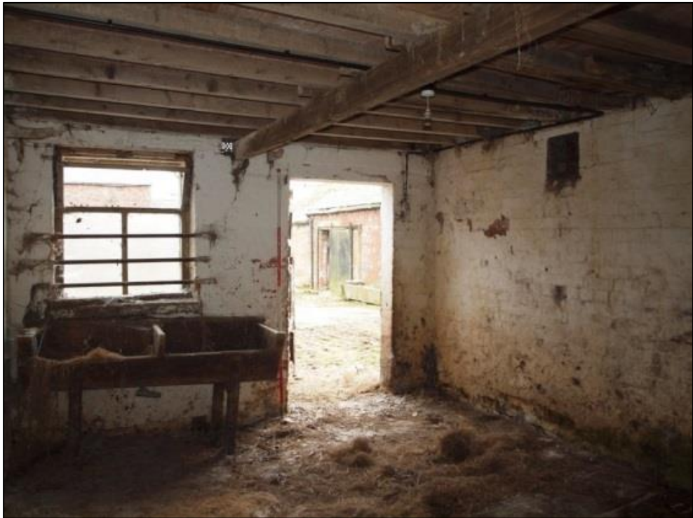
Plate 57: Interior of southern stable room
