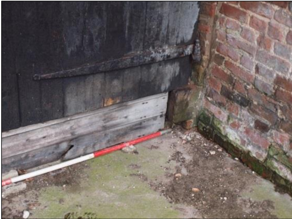
Plate 25: Detail of timber board at base of barn door
