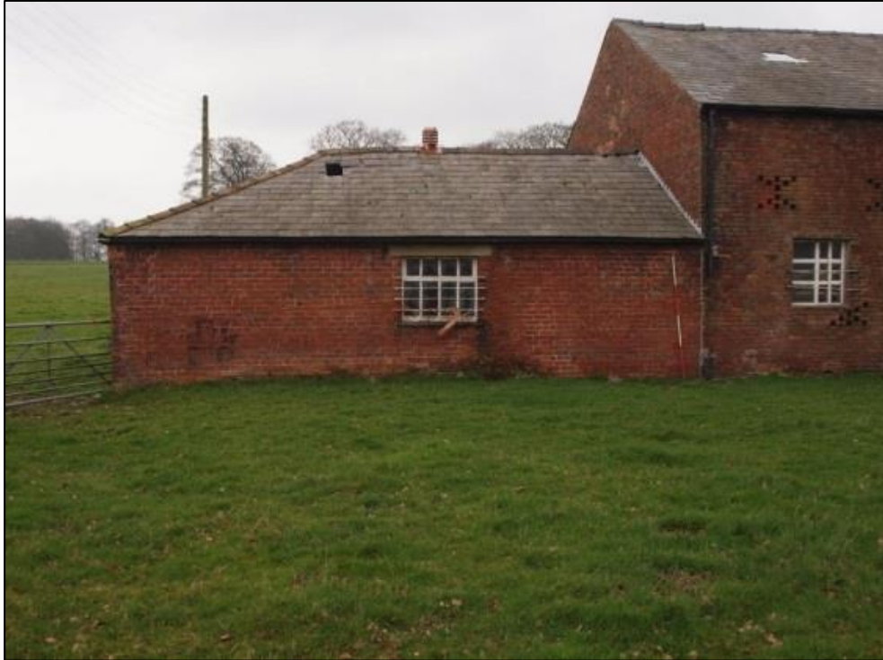
Plate 40: East elevation with faint rough joint to the left
