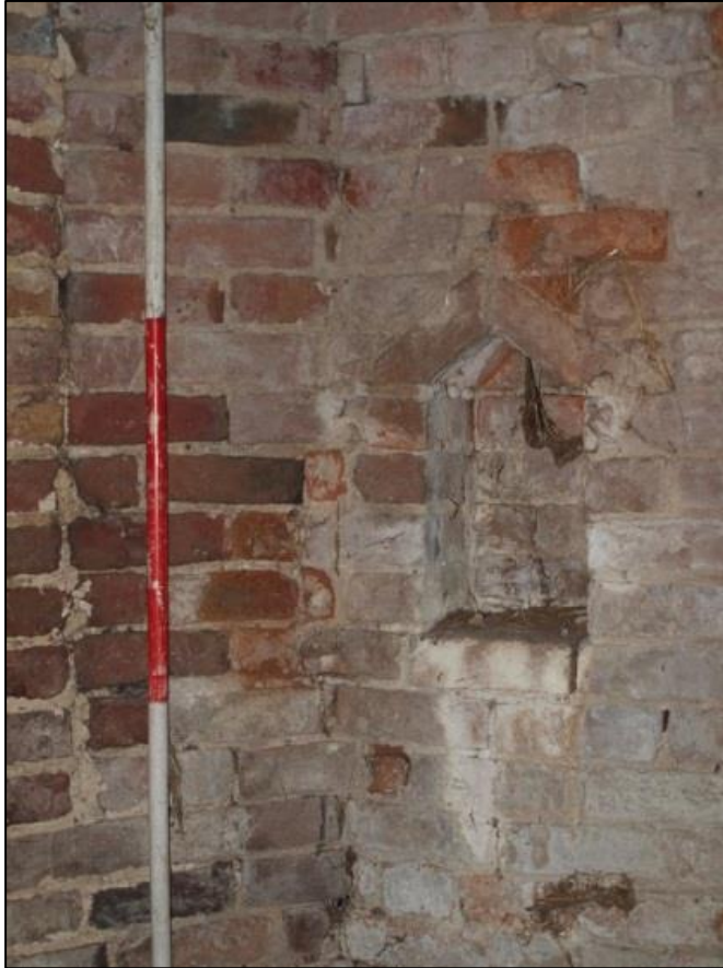
Plate 26: Detail of niche in in supporting column.
