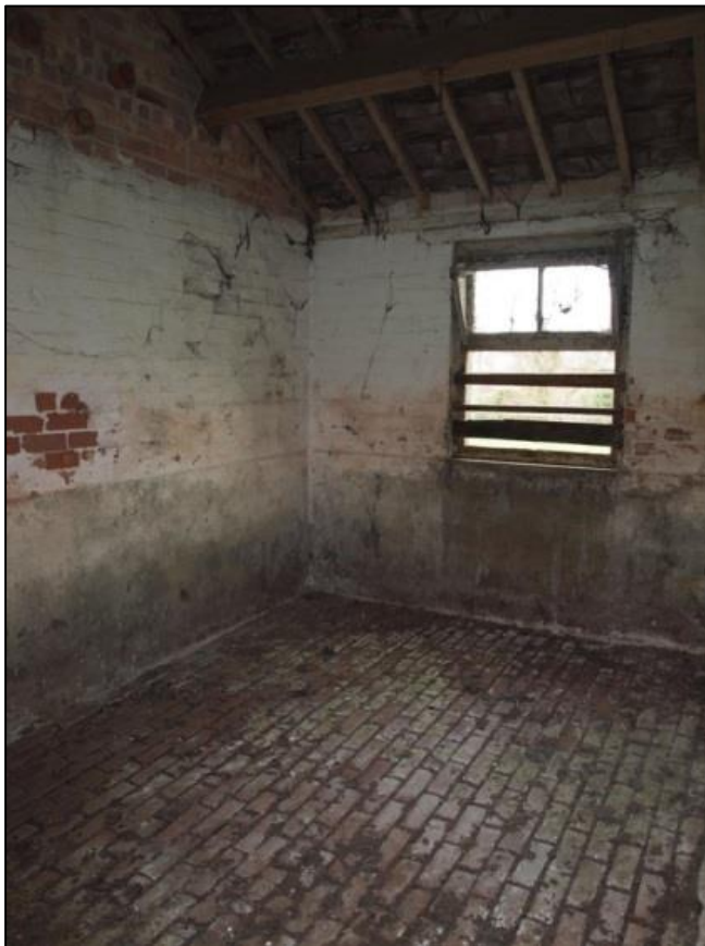
Plate 65: Interior of southern stable room
