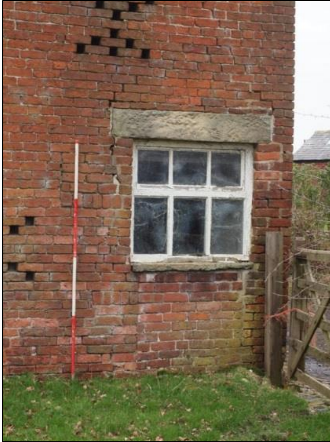
Plate 16: Blocked doorway with inserted window
