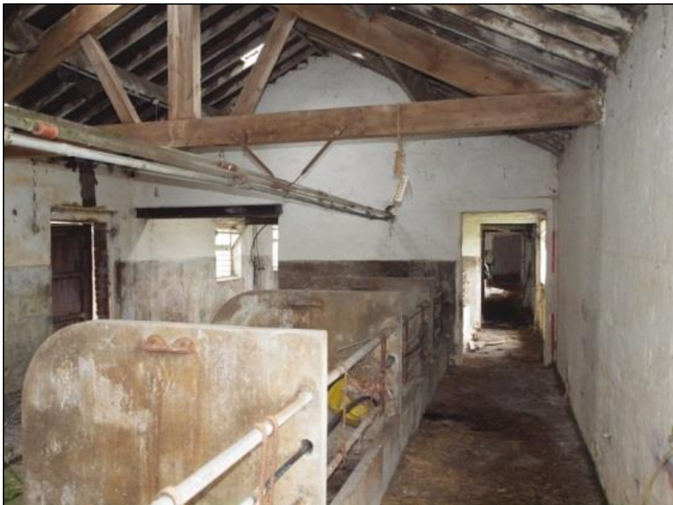
Plate 47: General view of shippon showing truss, boskins, feeding passage and cattle doorway
