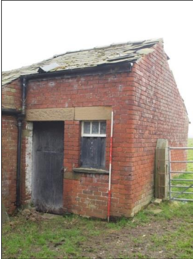
Plate 36: Recessed western end of north elevation and western gable
