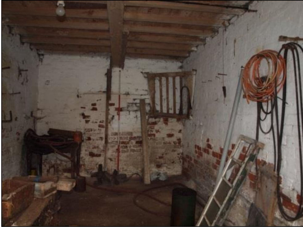
Plate 30: East store room showing blocked doorway
