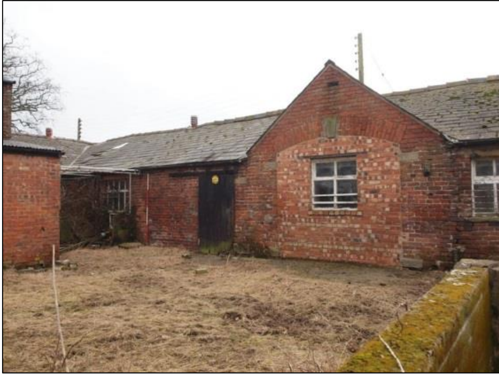
Plate 32: East end of north elevation showing gable with blocked cart doorway
