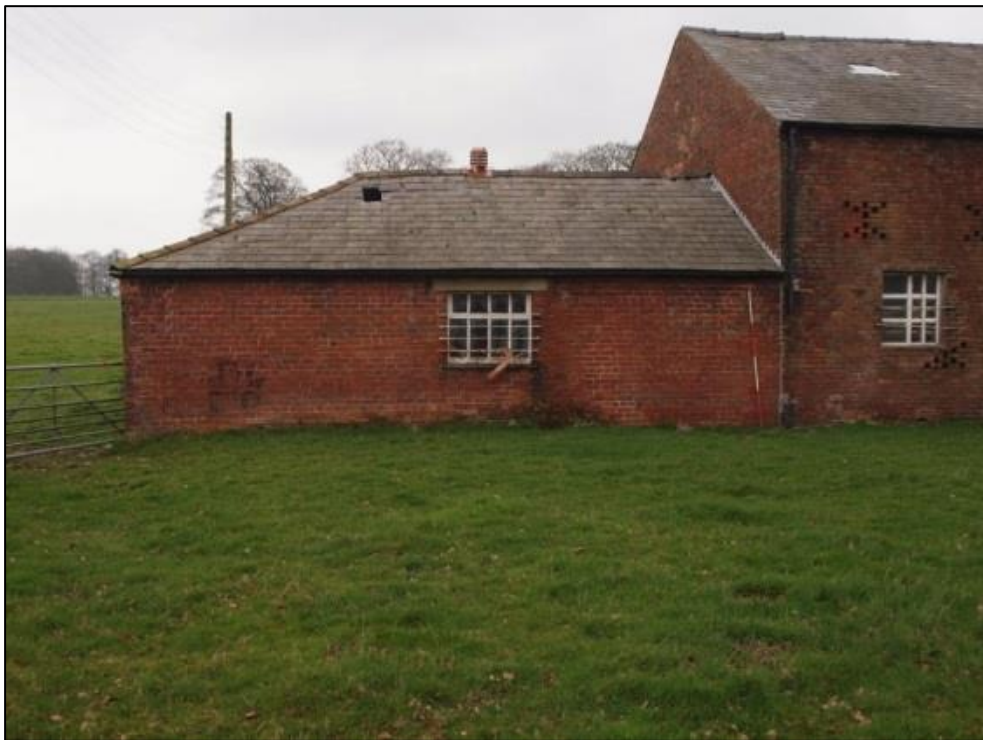
Plate 13: Southern gable with east face of shippon
