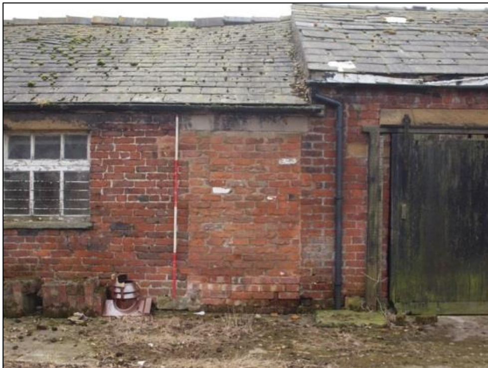
Plate 34: Detail of blocked doorway and change in roof levels
