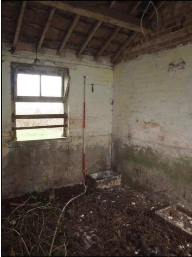
Plate 64: Interior of northern stable room
