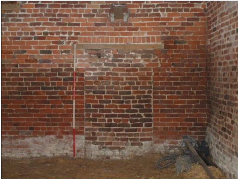
Plate 23: Detail of blocked doorway
