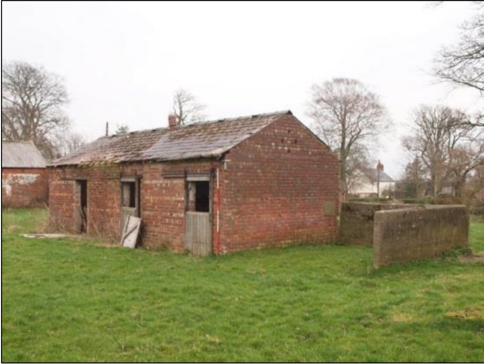
Plate 60: West (front) elevation and south gable
