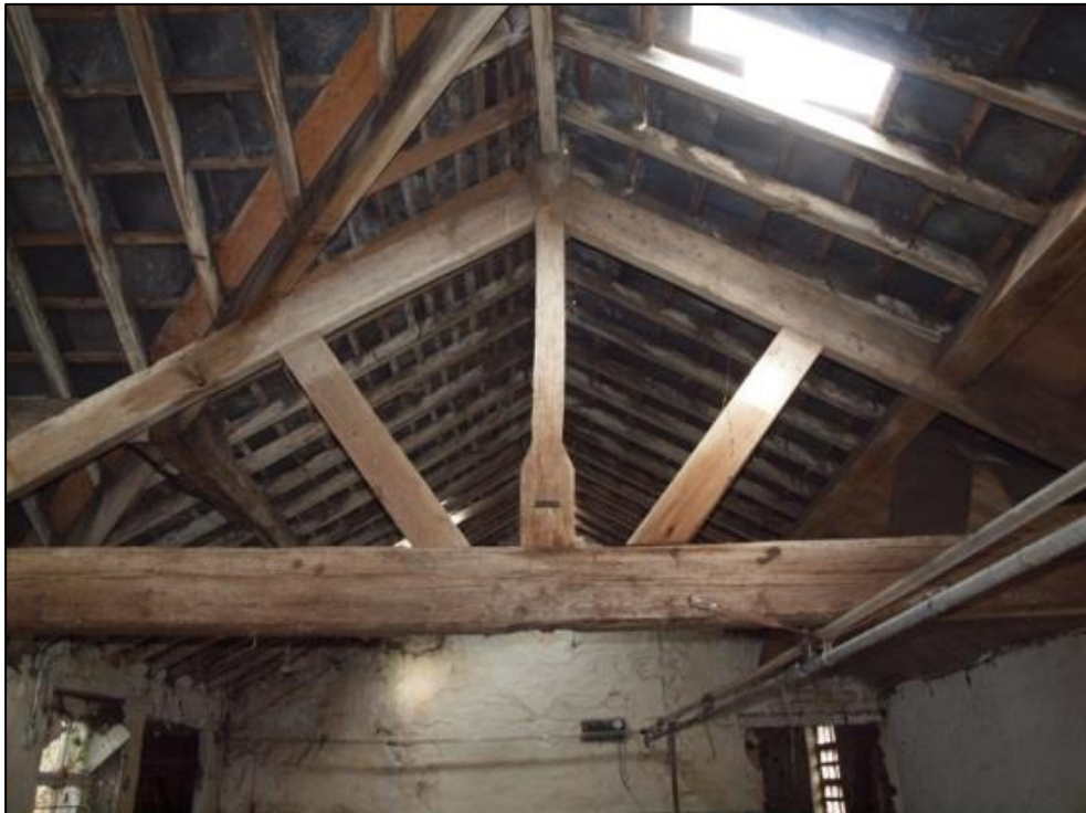
Plate 43: Detail of truss
