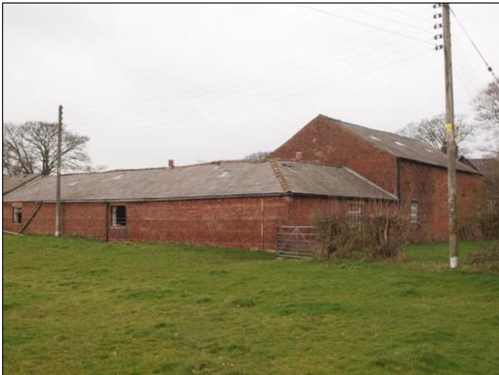
Plate 39: East end of south elevation
