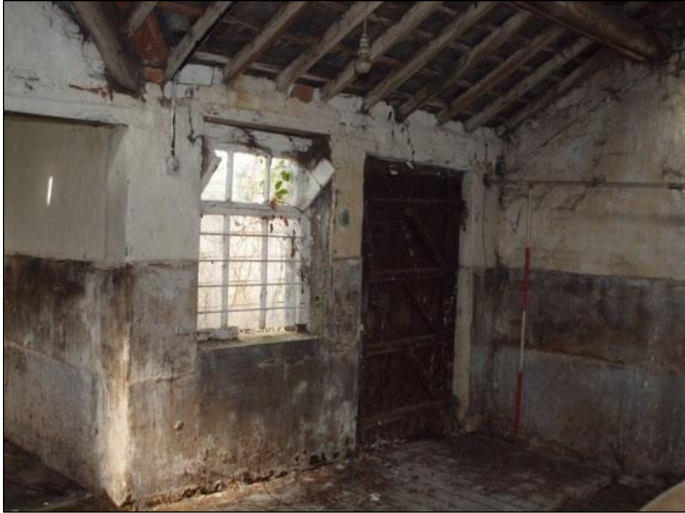
Plate 44: Detail of external doorway and window, blocked from view externally.
