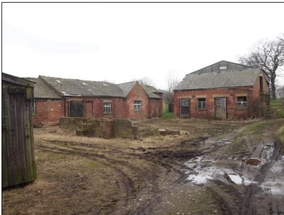
Plate 1: General shot of the farm yard looking west towards the two bay stable (right).
