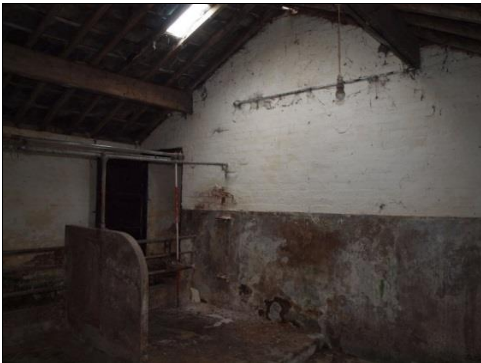
Plate 49: Bay 7 of shippon showing doorway to bay 8.
