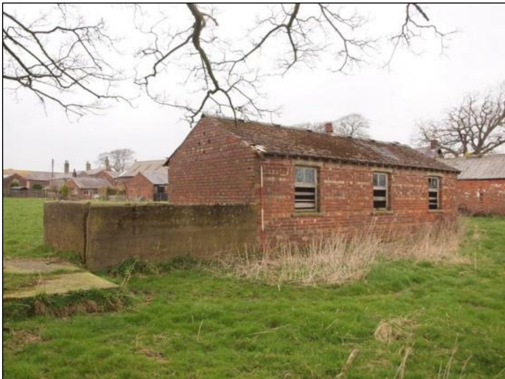
Plate 63: East (rear) elevation and south gable
