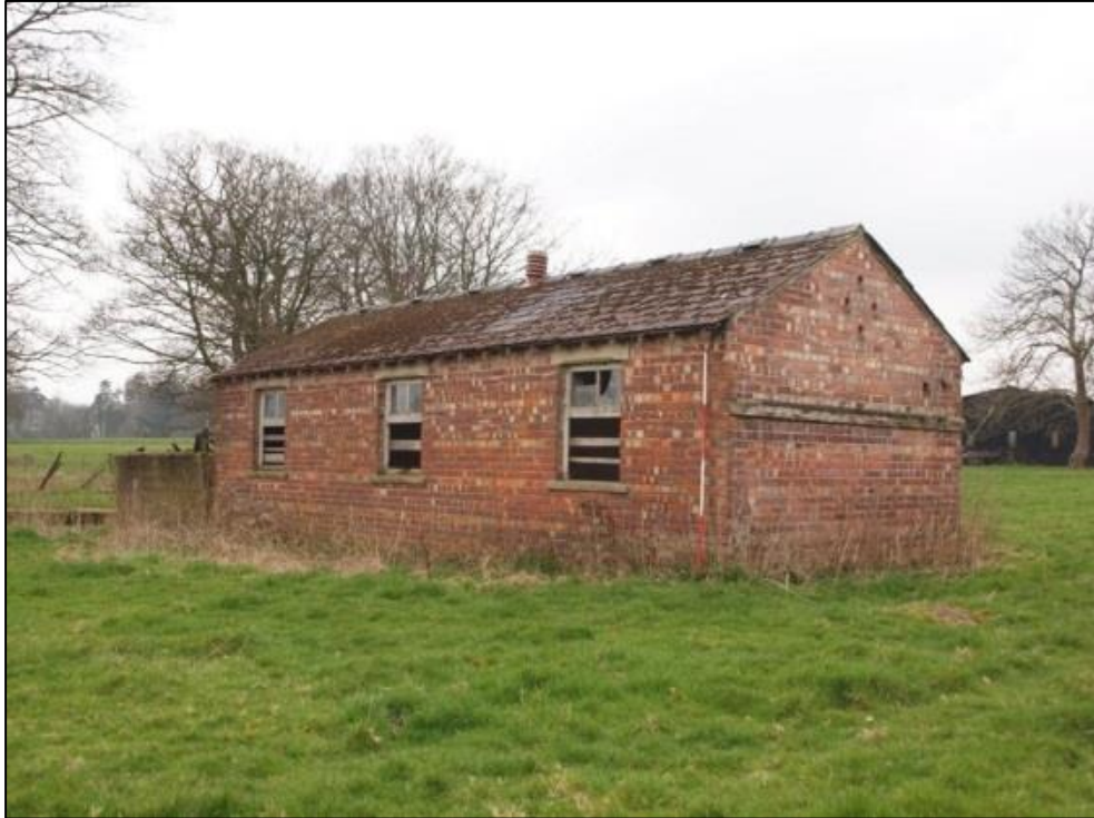
Plate 62: East (rear) elevation and north gable
