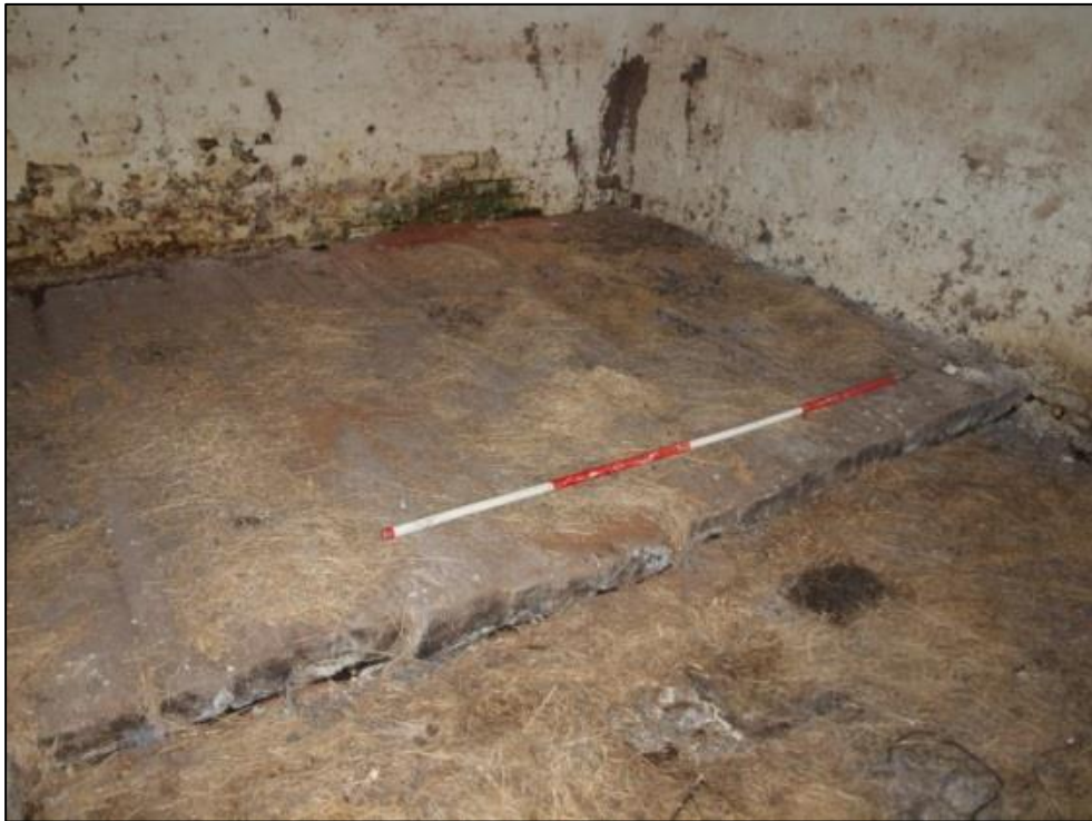
Plate 59: Floor of northern stable room showing raised floor of timber
