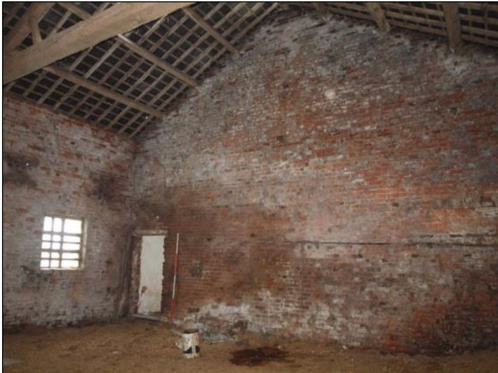
Plate 21: Interior of barn showing inserted doorway to shippon in south gable
