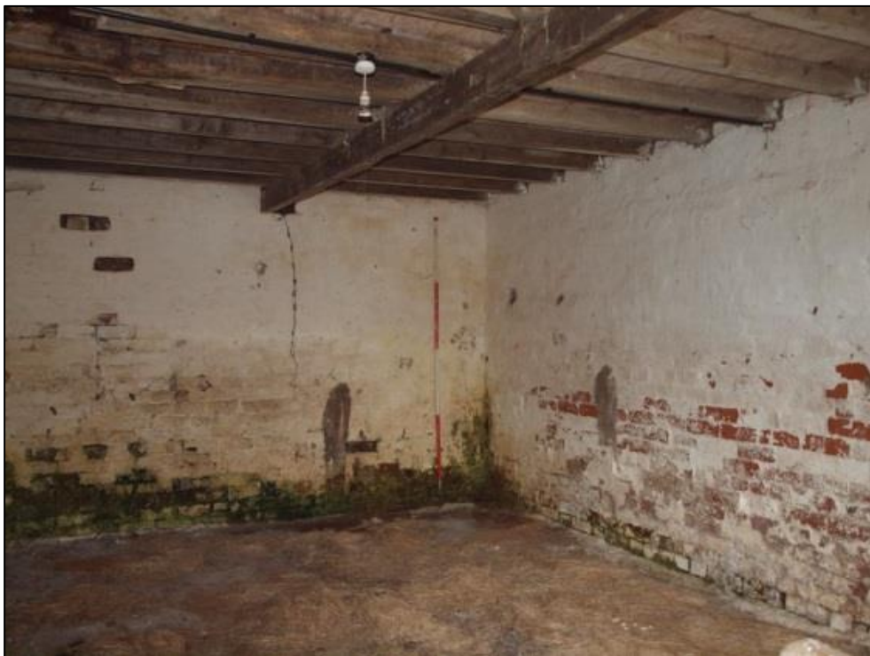
Plate 56: Interior of southern stable room
