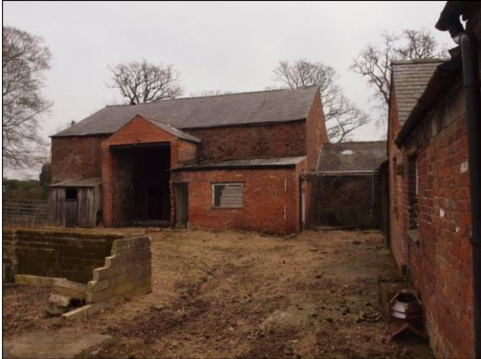
Plate 12: West elevation and southern gable
