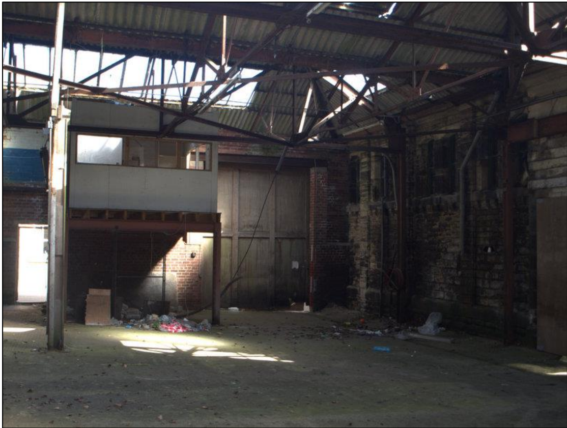
Plate 61: First floor office and loading door at northern end of extension
