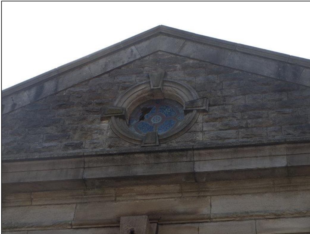
Plate 4: Detail of circular window in north elevation
