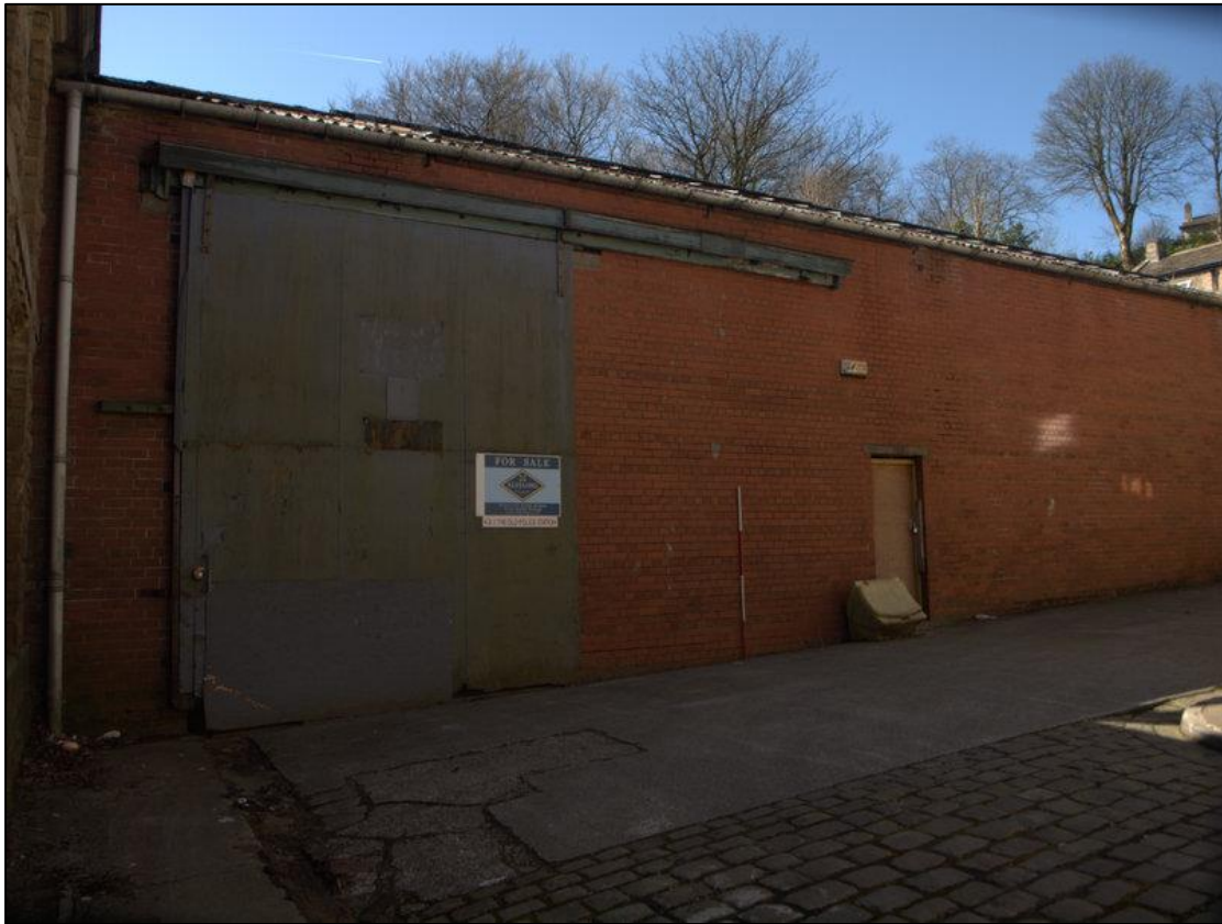
Plate 47: North elevation of extension
