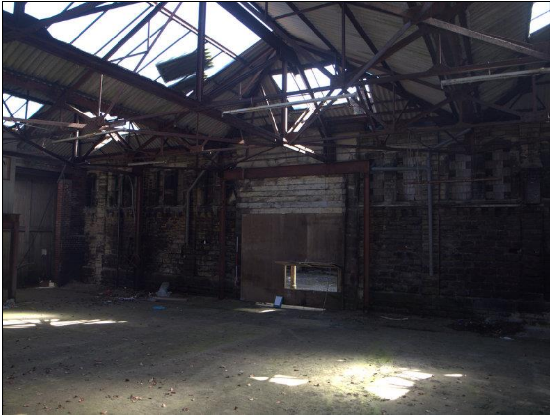
Plate 19: North elevation showing doorway, within later extension
