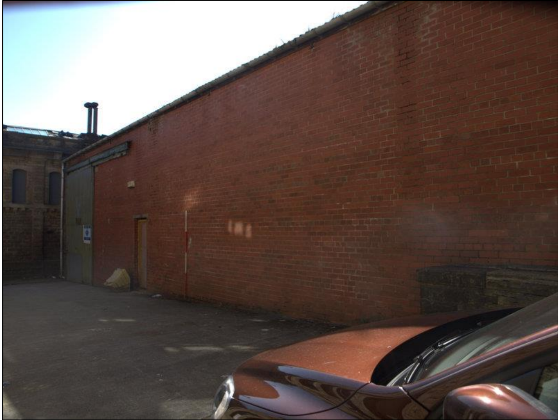
Plate 49: North elevation of extension
