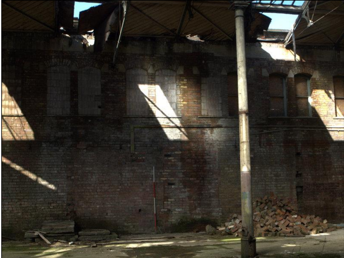
Plate 36: Section of western wall showing possible blocked doorway
