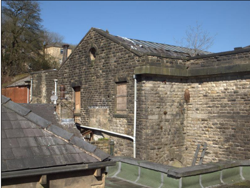
Plate 13: Detail of central bay in south elevation
