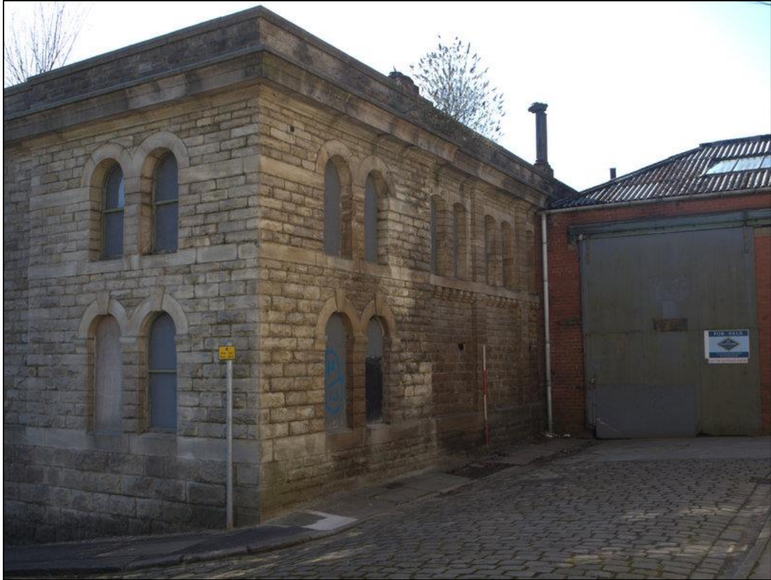
Plate 17: North end of west elevation
