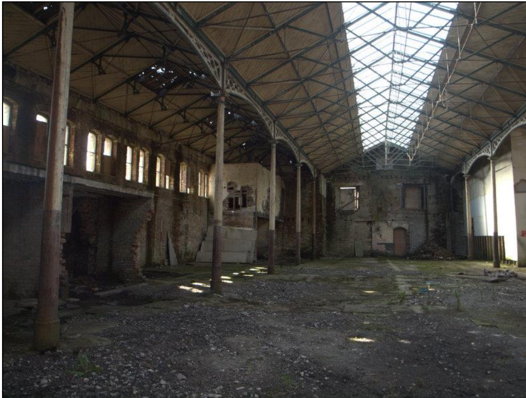
Plate 28: General shot of interior looking south
