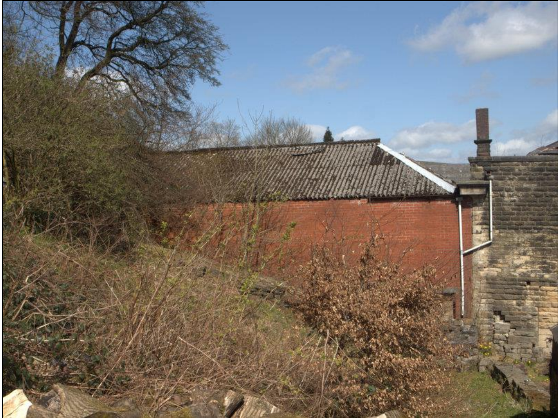
Plate 50: Southern elevation of extension
