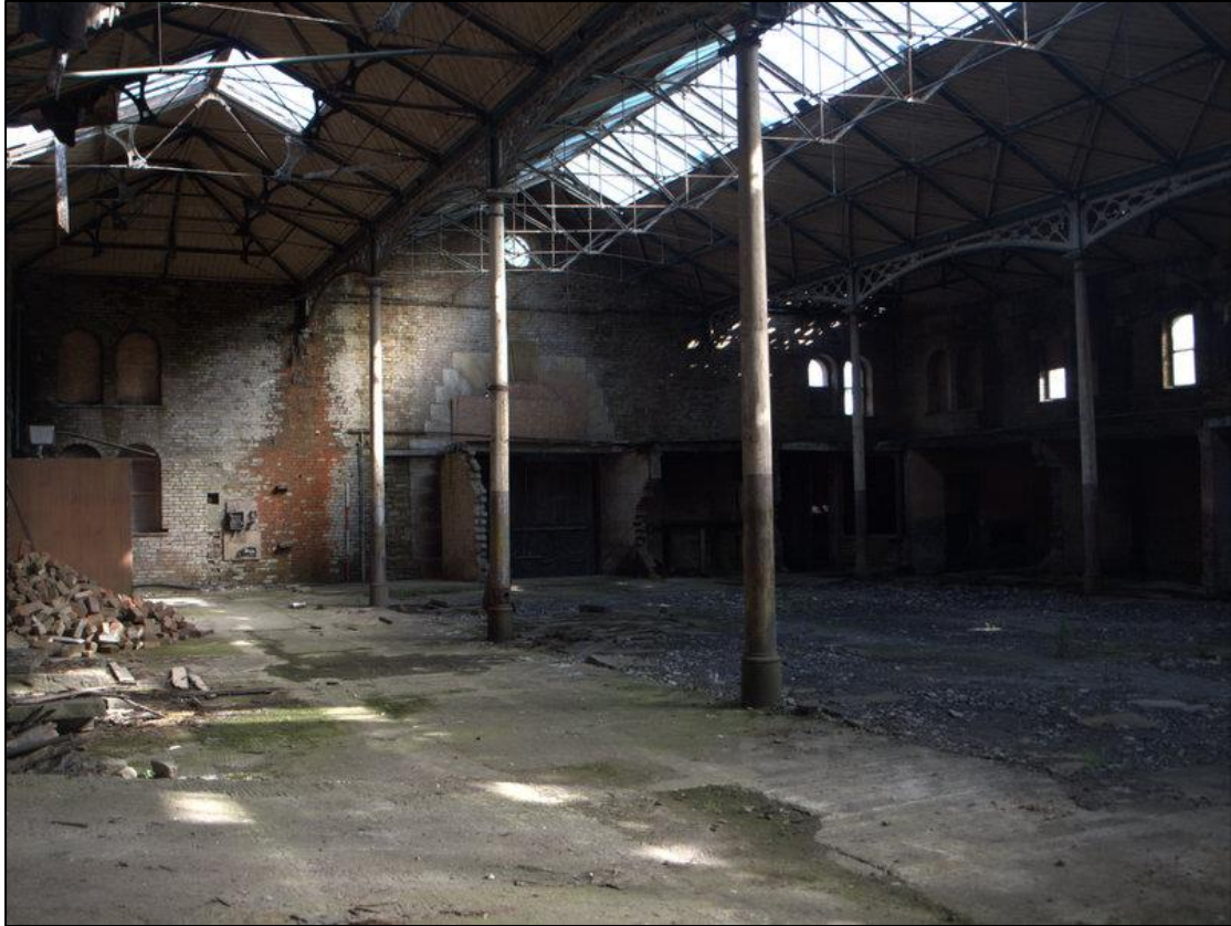
Plate 23: General shot of interior
