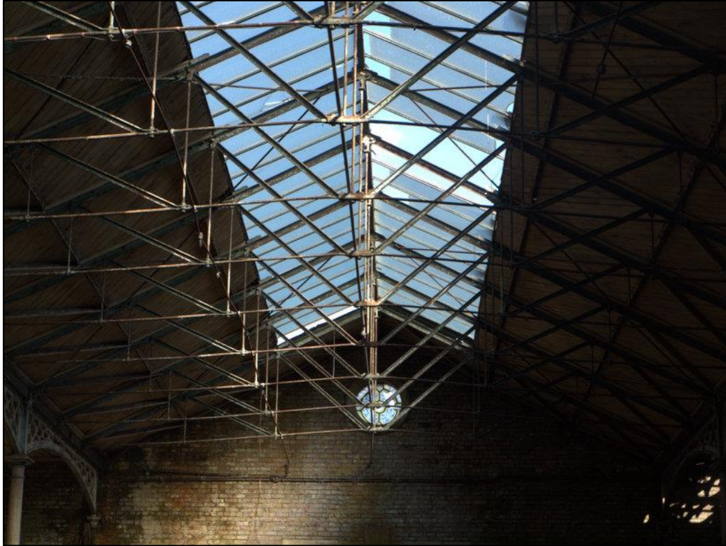
Plate 39: Detail of roof structure of central bay
