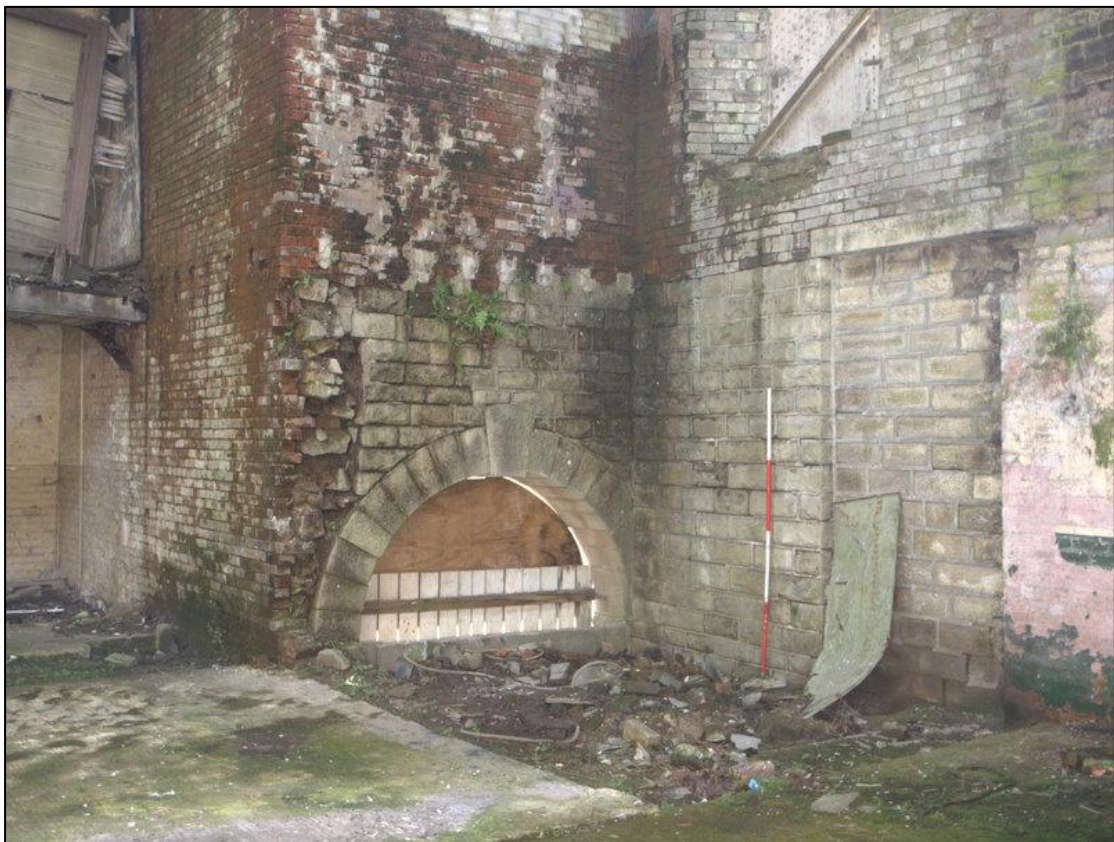
Plate 30: Blocked doorway and infilled staircase at southern end of east side.
