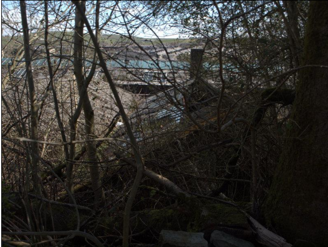
Plate 52: Extension viewed from the west showing roofs and market hall beyond
