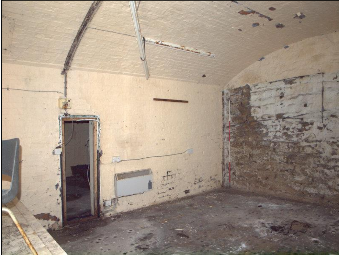
Plate 43: Southern wall of unit showing inserted doorway
