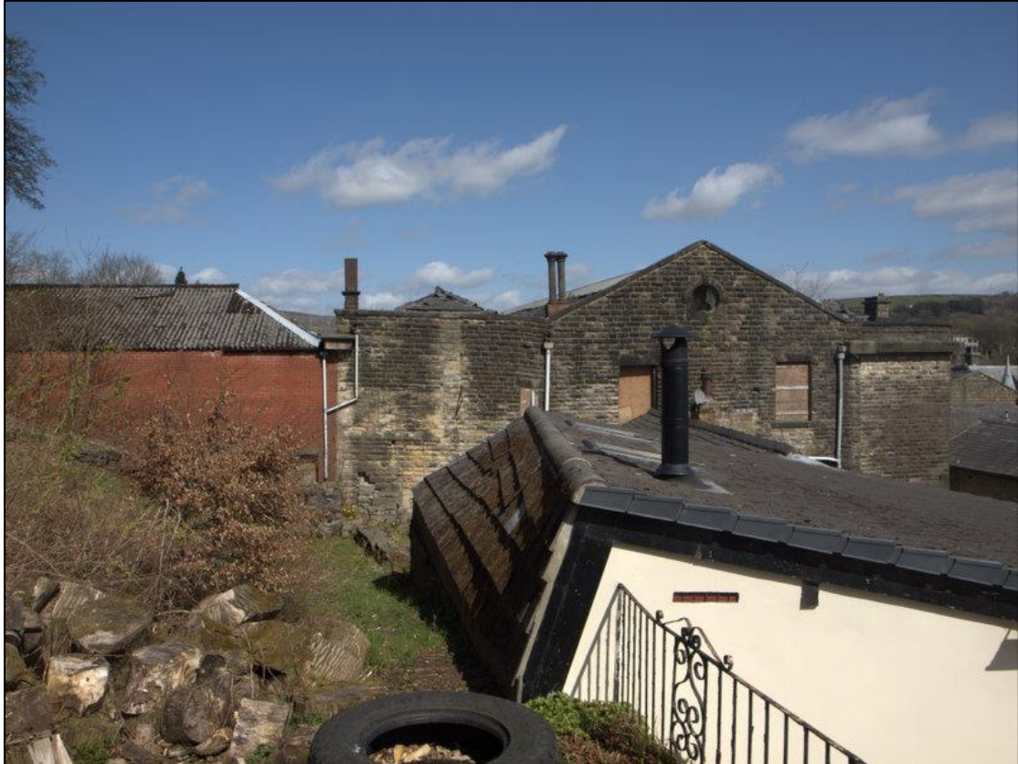
Plate 16: South elevation west side
