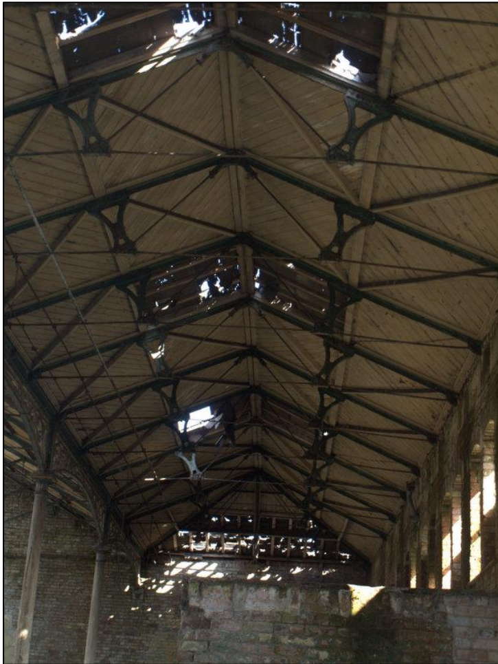
Plate 40: Detail of roof structure of eastern bay
