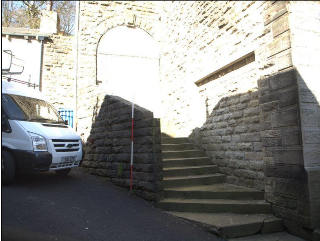
Plate 11: Stone steps leading up to blocked doorway in east elevation
