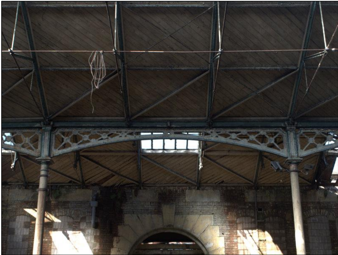
Plate 37: Detail of cast iron tie beams with western door beyond
