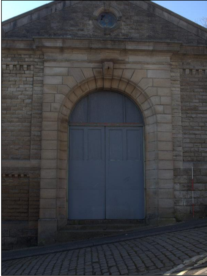
Plate 3: Detail of northern doorway
