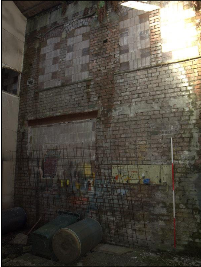
Plate 33: Blocked window and RSJ lintel in west elevation
