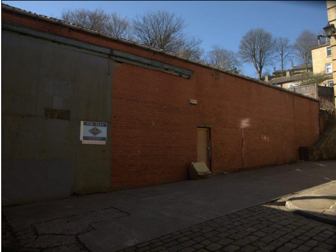
Plate 48: North elevation of extension
