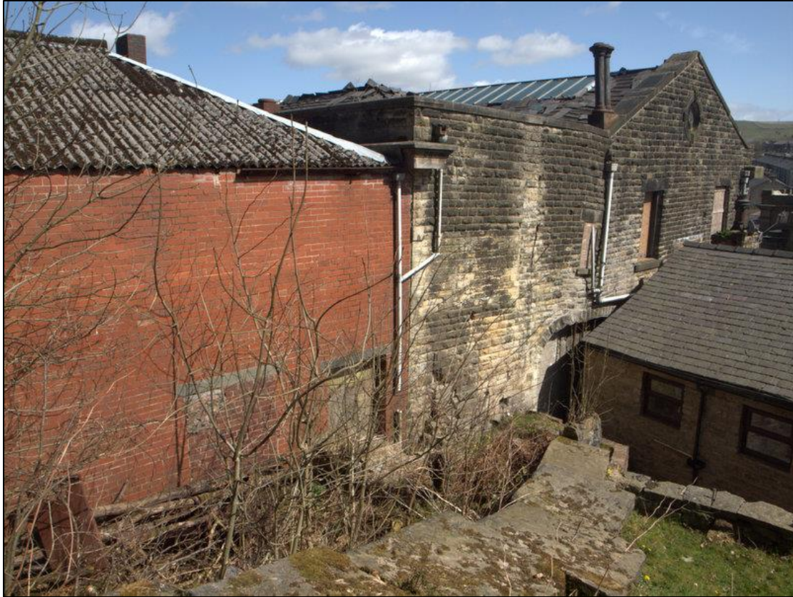
Plate 51: Southern elevation of extension
