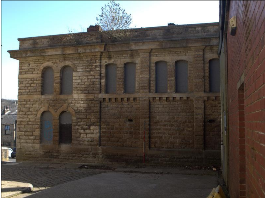
Plate 18: North end of west elevation
