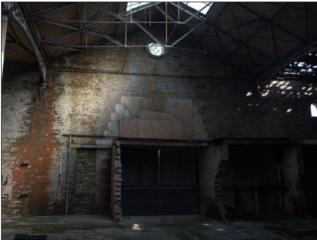
Plate 24: Detail of doorway in north elevation
