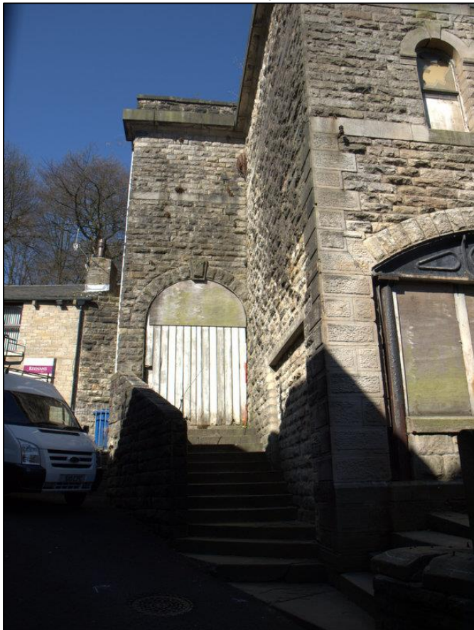
Plate 10: Blocked doorway at recessed southern end of east elevation
