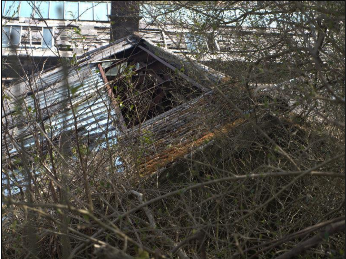
Plate 54: Detail of roof
