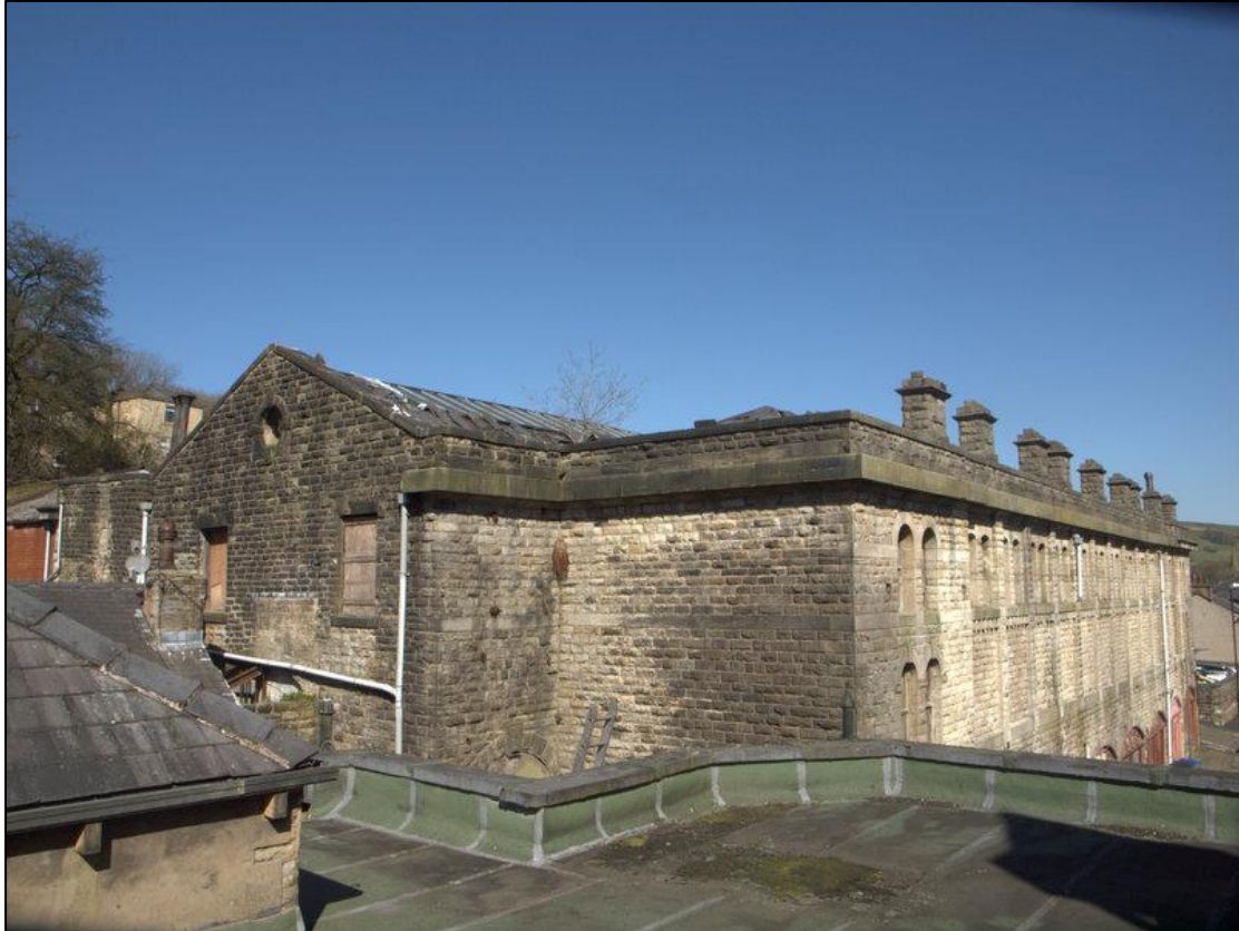
Plate 12: South elevation, east end
