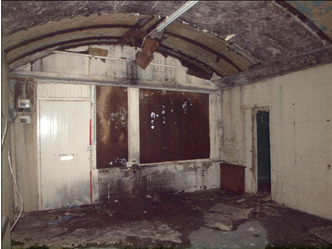
Plate 44: Second unit showing boarded frontage and further inserted doorway
