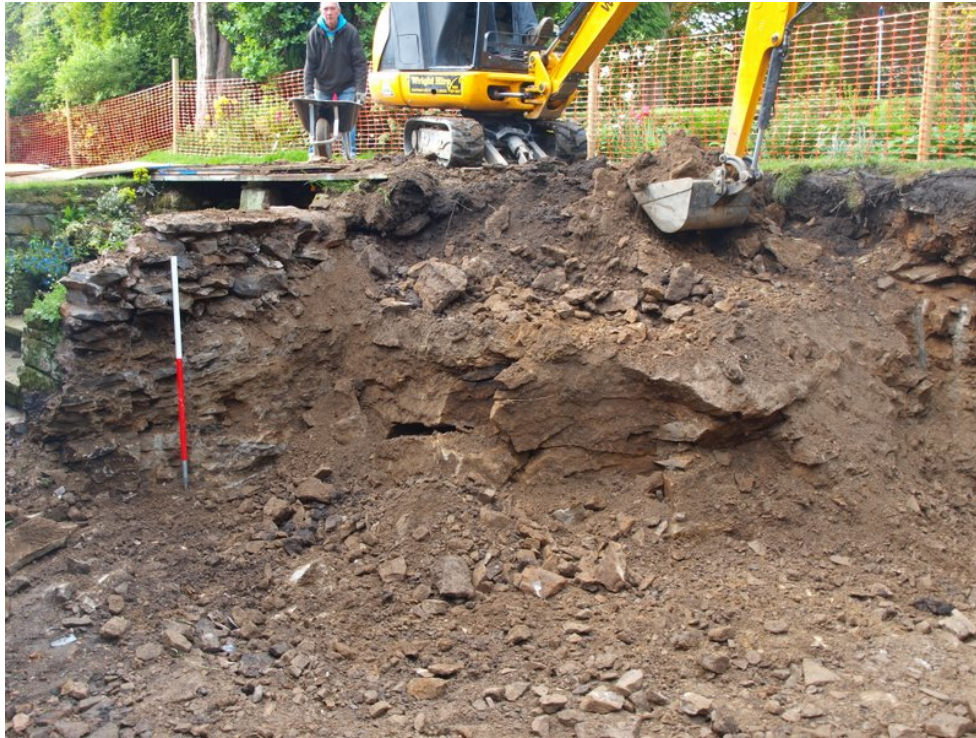
Plate 15: Removal of southwestern corner of excavation
