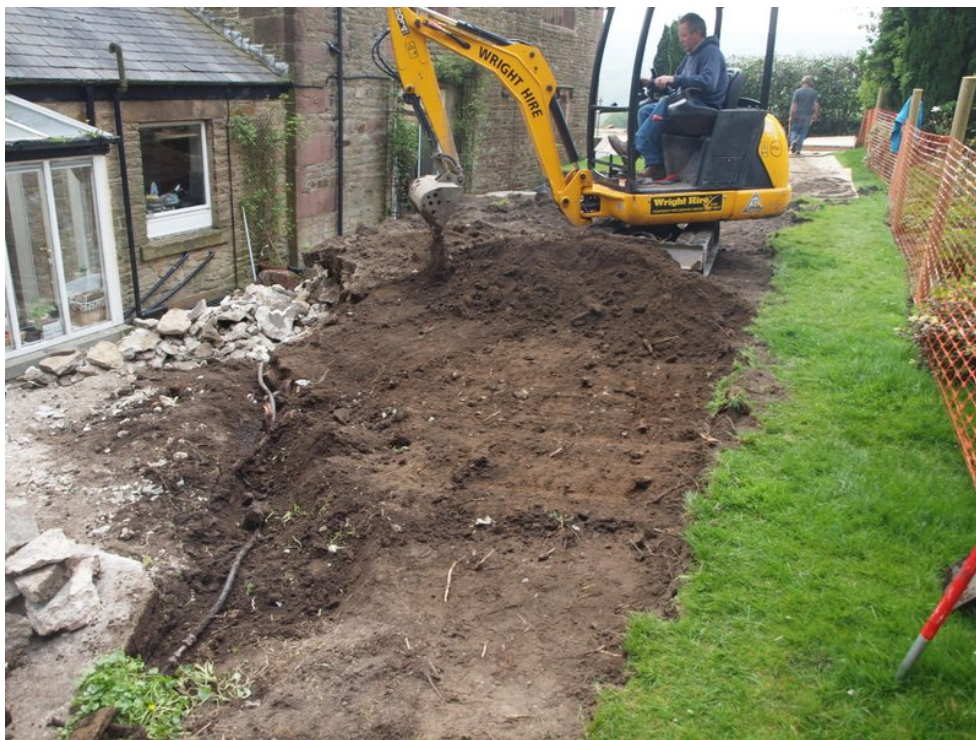
Plate 4: Removal of topsoil
