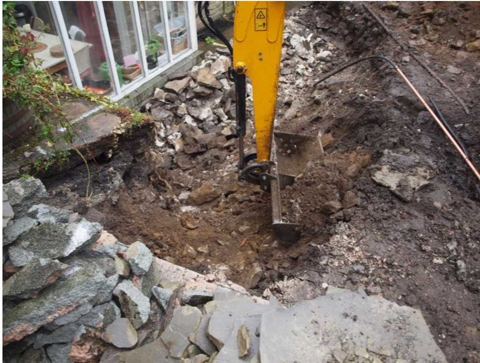
Plate 7: Excavation of garden wall and concrete
