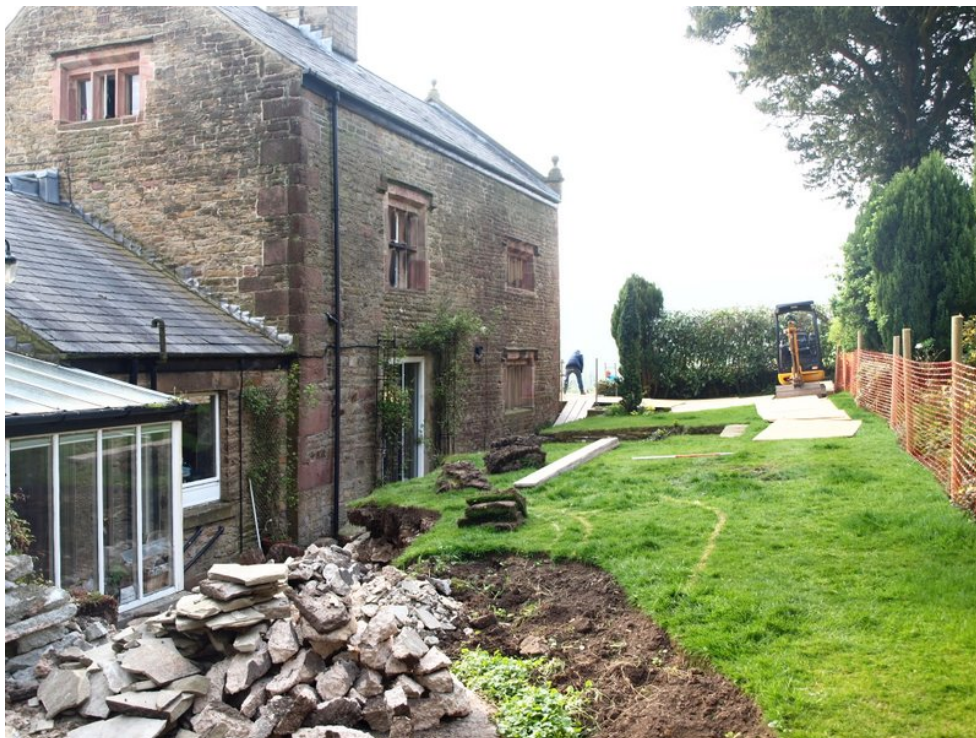
Plate 2: Site prior to excavation
