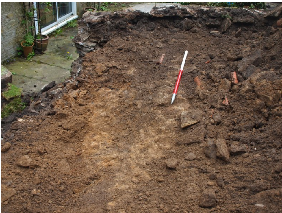
Plate 10: Southern end showing remains of land drain
