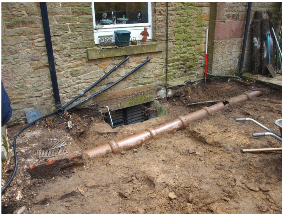
Plate 18: Modern drain and bedrock below flagstones
