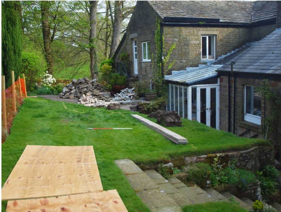
Plate 1: Site prior to excavation
