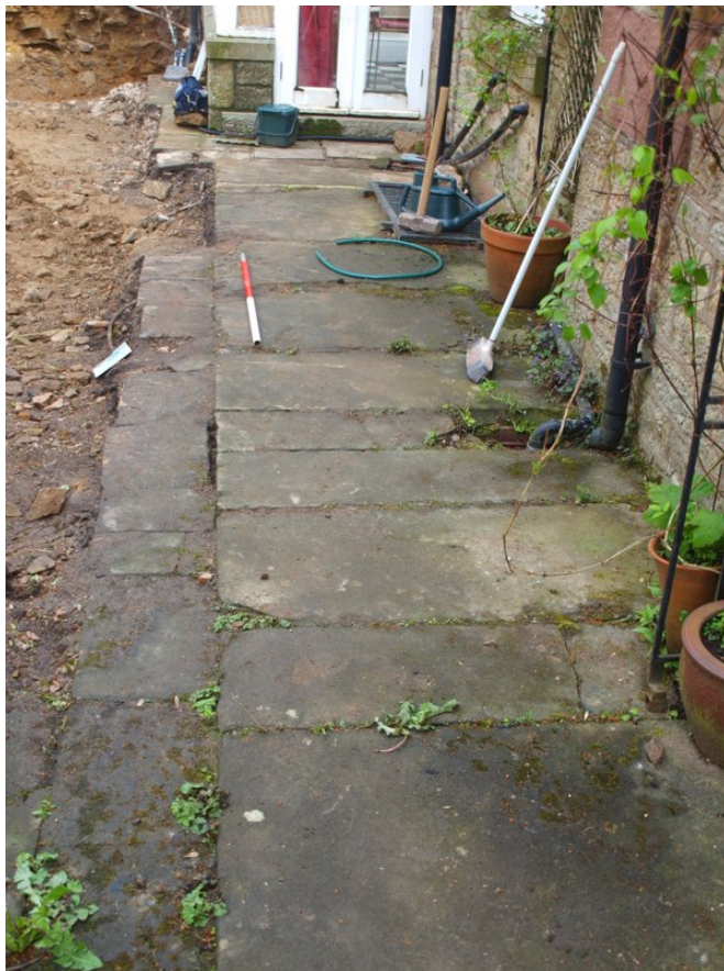
Plate 16: Flagstone surface prior to lifting
