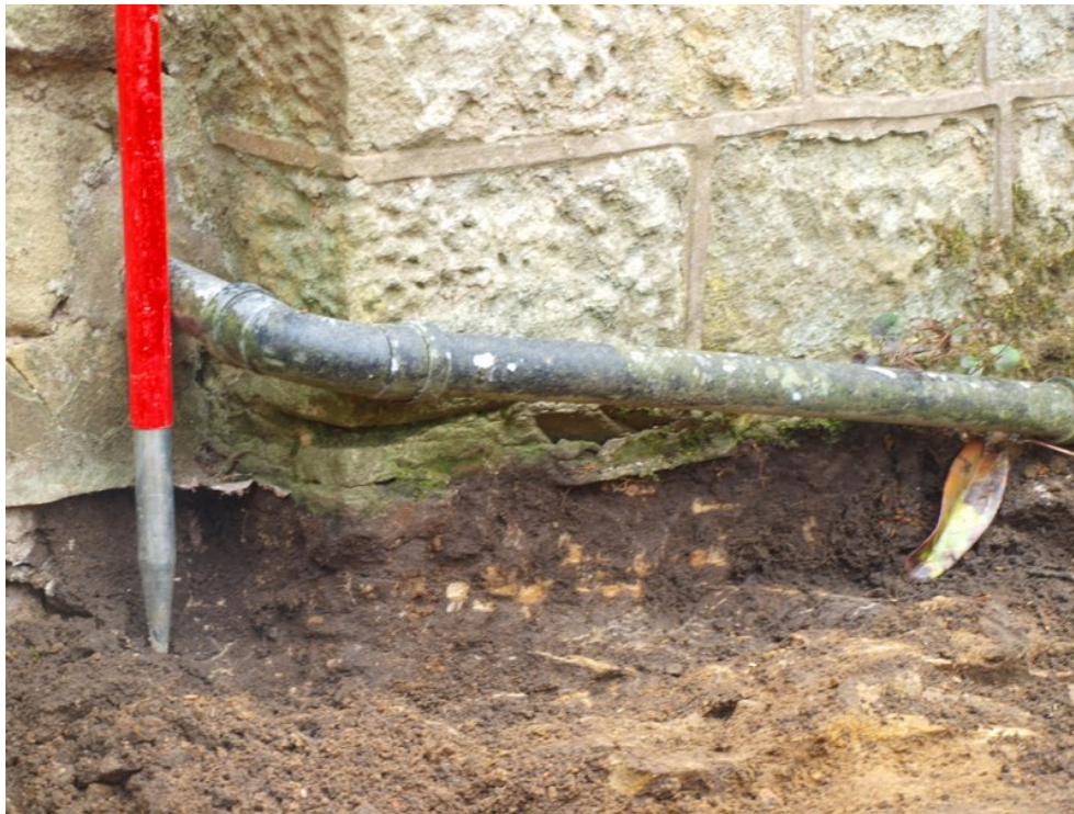
Plate 20: House foundations resting on bedrock
