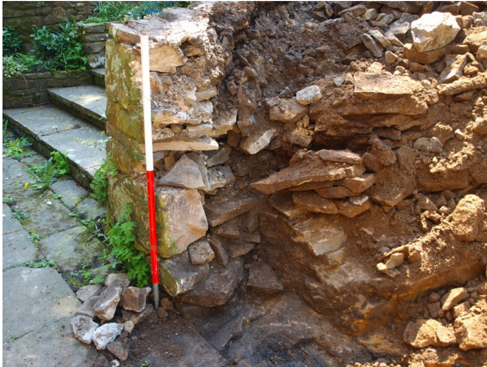
Plate 11: Bedrock cut for wall
