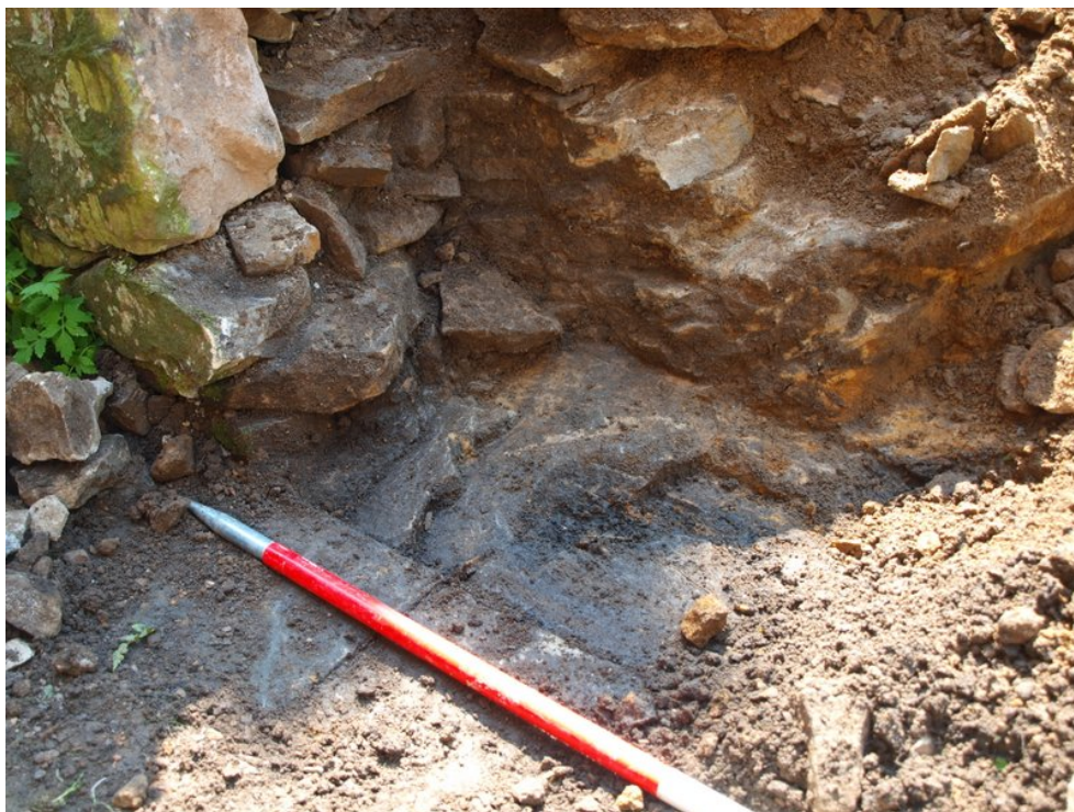
Plate 12: Shaped bedrock for wall construction
