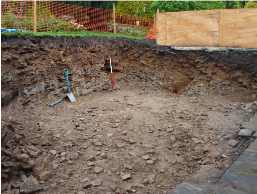
Plate 13: Final excavation through bedrock (03)
