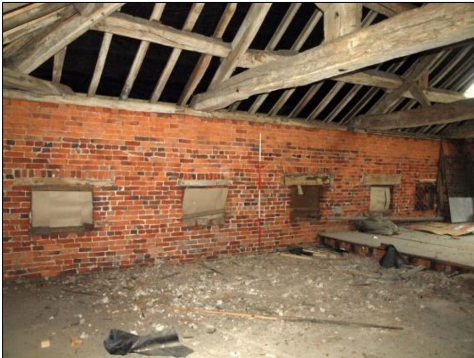
Plate 43: Blocked alcoves in room 14 east wall
