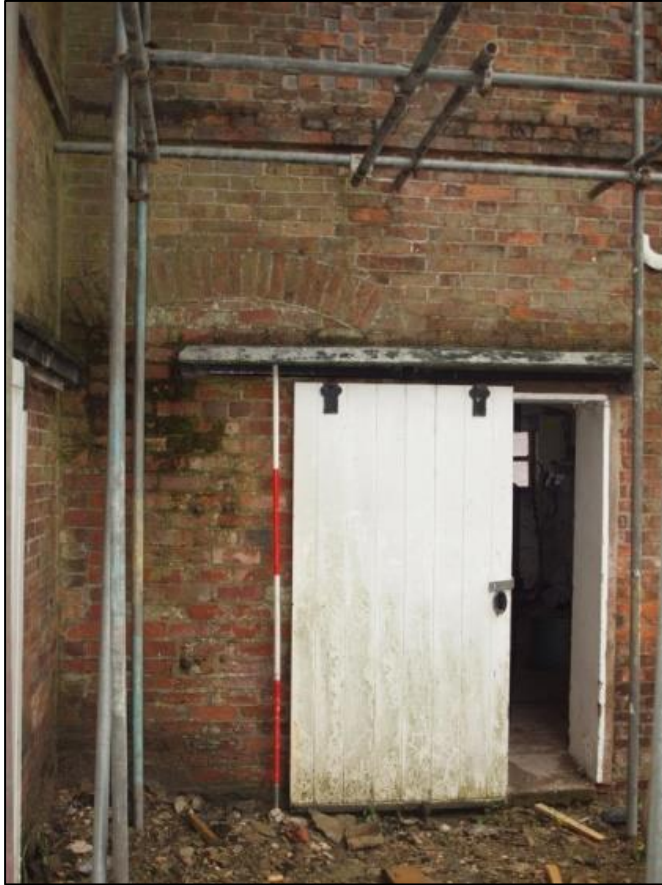
Plate 15: Detail of inserted doorway in blocked doorway in internal east elevation
