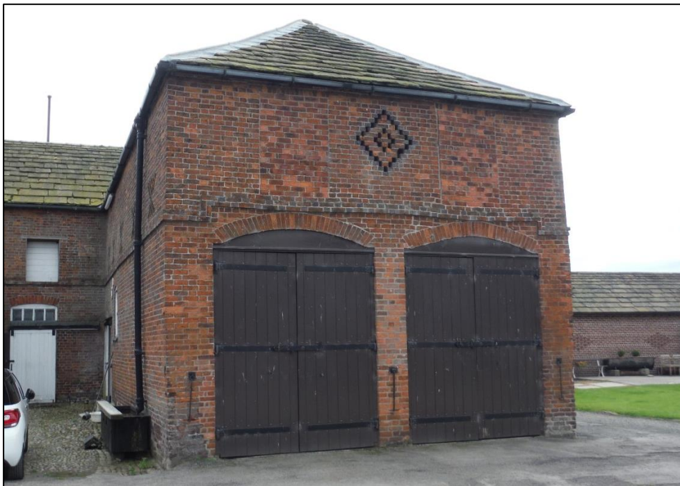
Plate 1a: As above before the scaffolding
