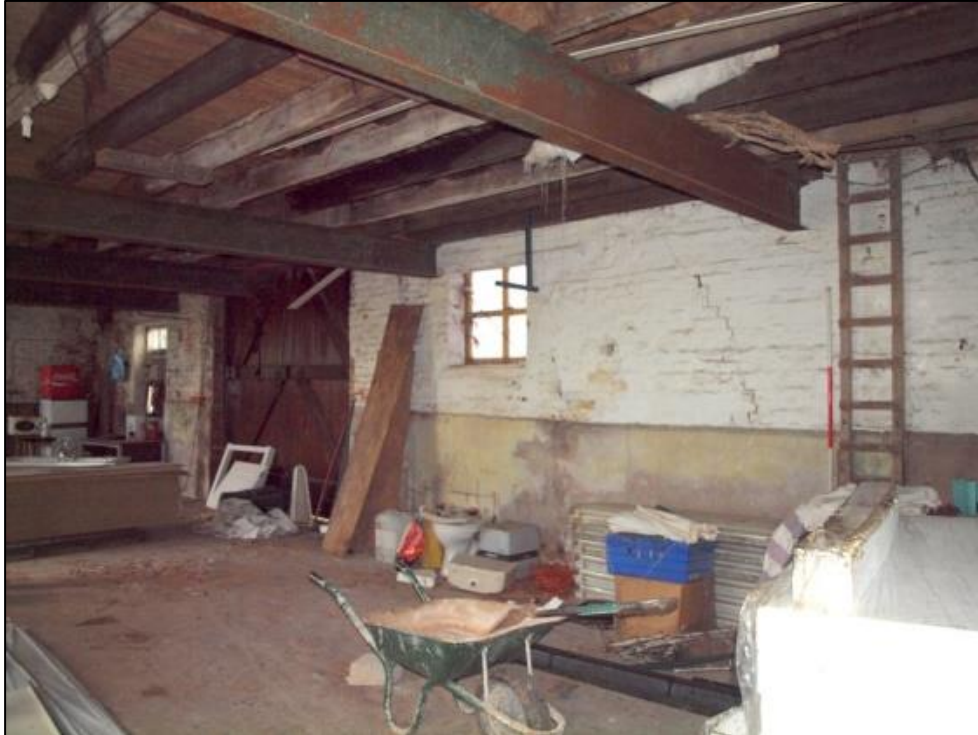
Plate 28: Room 4 looking northwest
