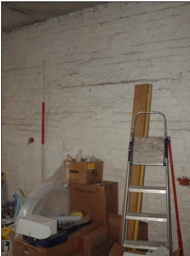
Plate 19: Detail of blocked doorway in above
