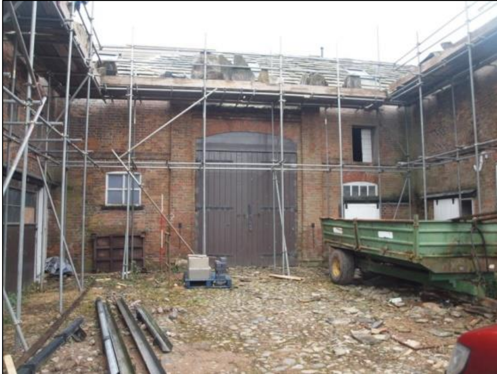
Plate 2: North elevation, centre
