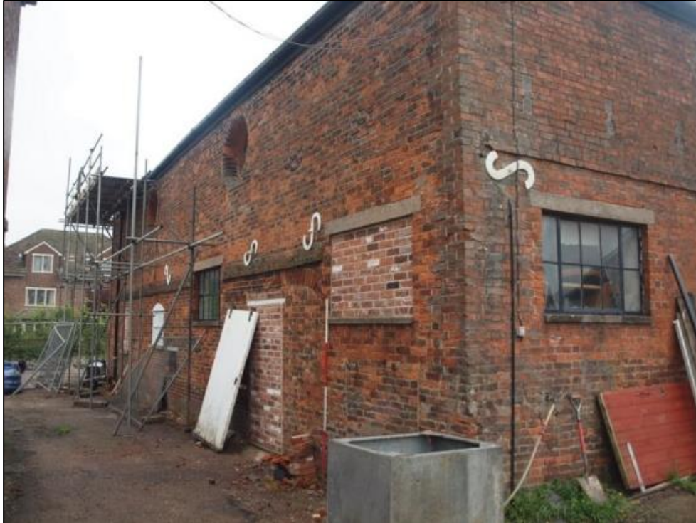
Plate 10: West elevation from south
