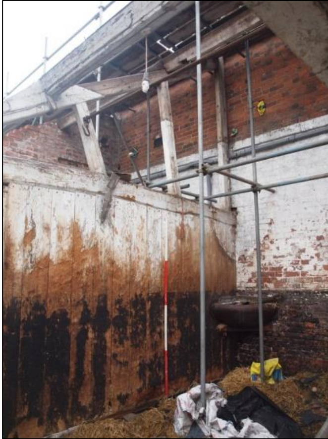
Plate 36: Room 8 showing timber dividing wall
