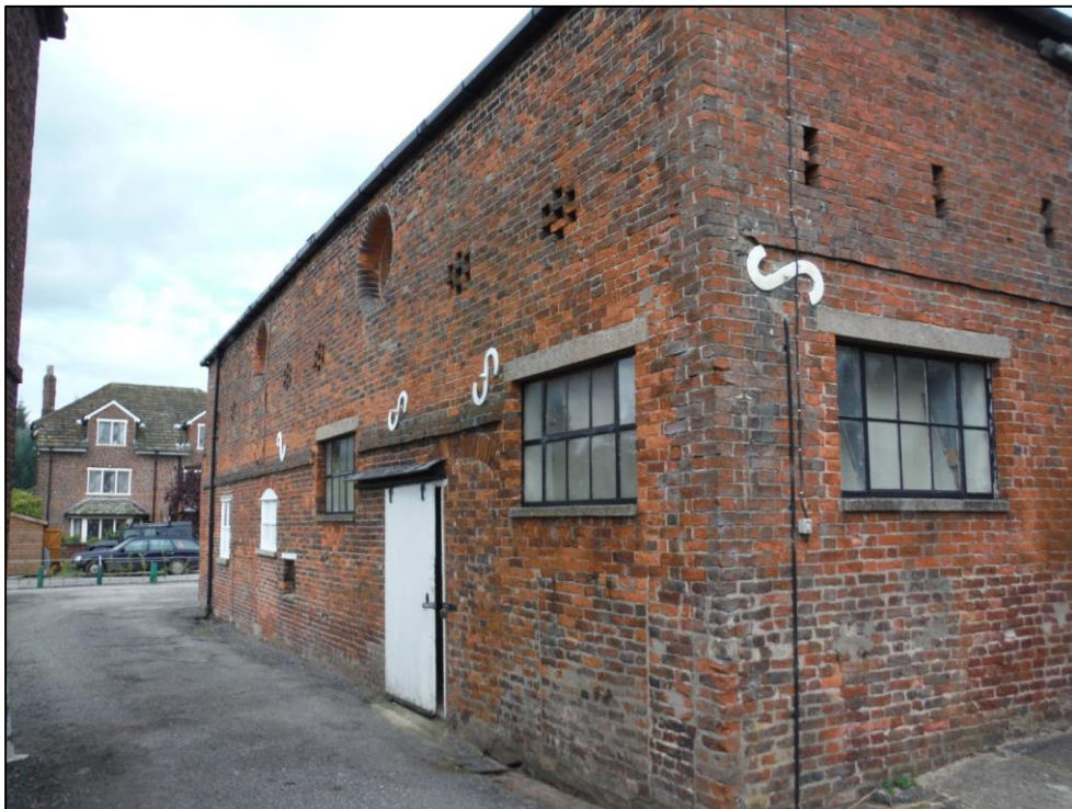
Plate 10a: As above before the scaffolding and blocking of door and window
