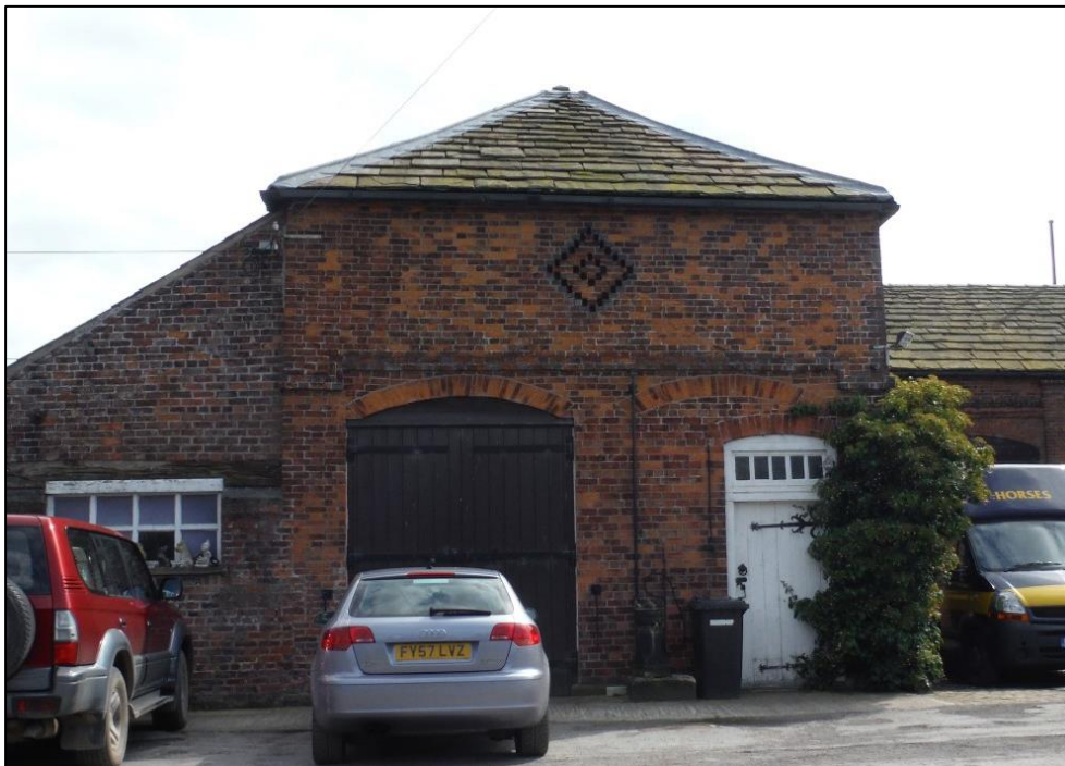
Plate 3a: As above before the scaffolding
