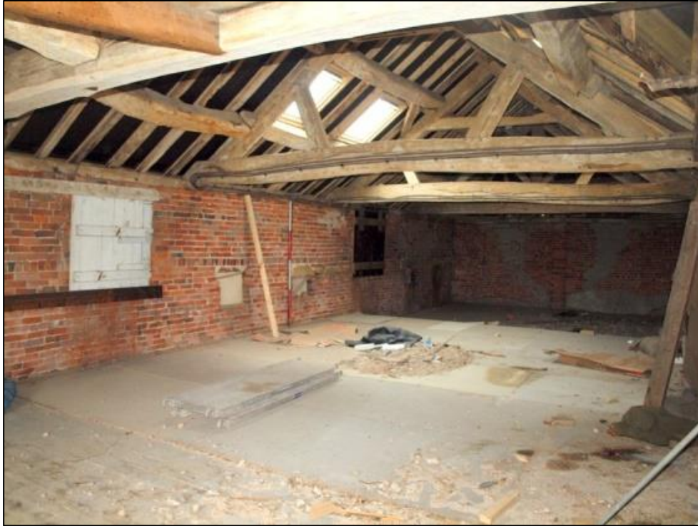
Plate 46: Room 14 looking north
