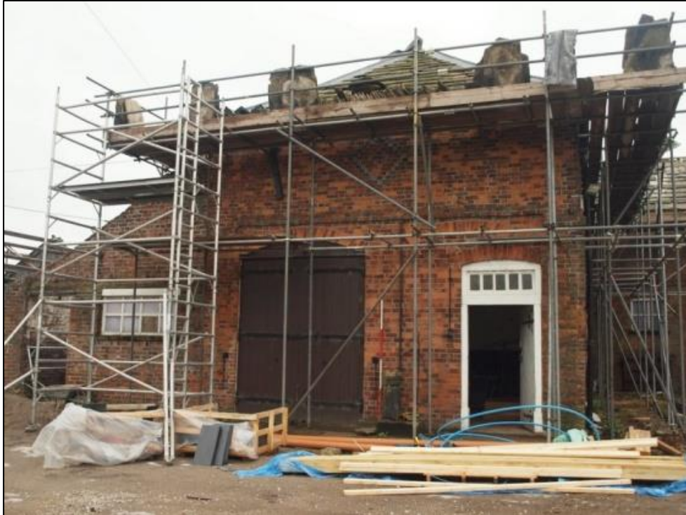
Plate 3: North elevation, East end
