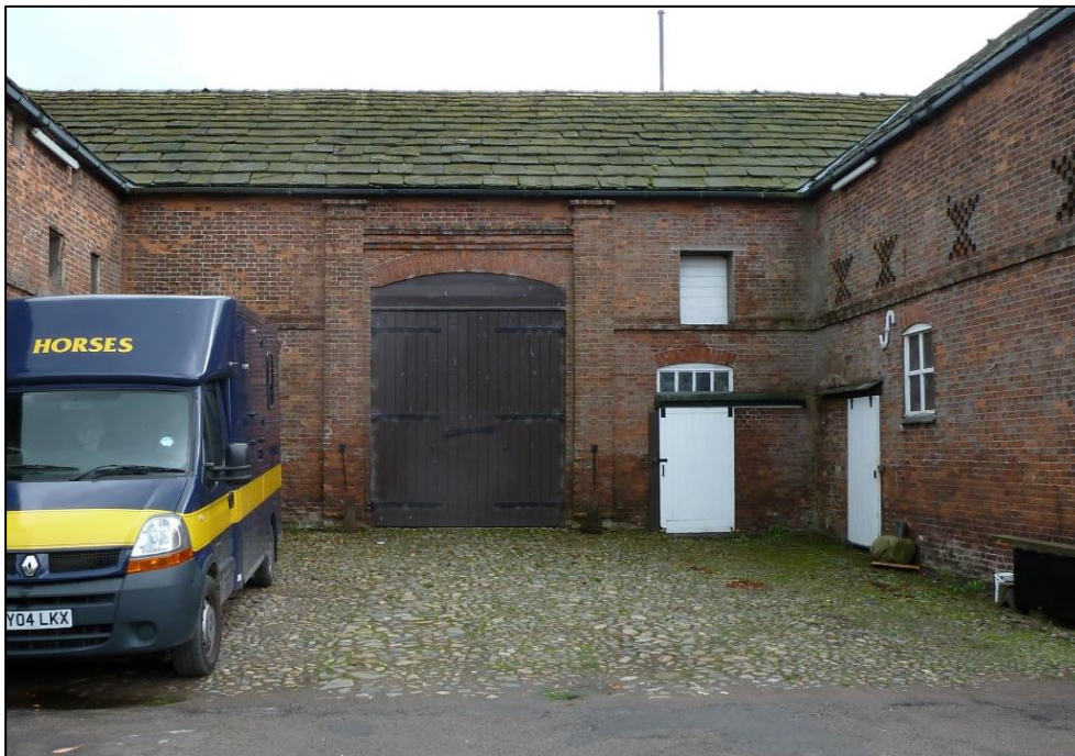
Plate 2a: As above before the scaffolding
