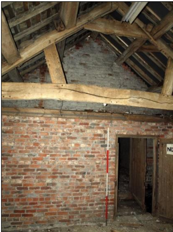
Plate 63: Room 16 looking north
