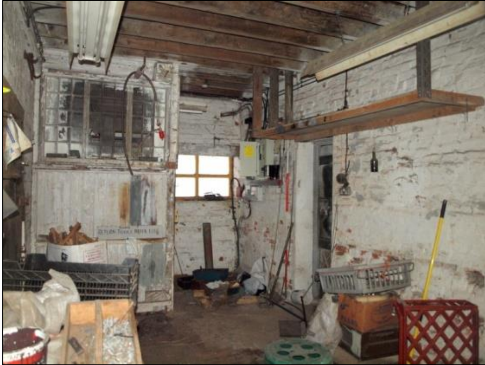
Plate 20: Room 2 looking west
