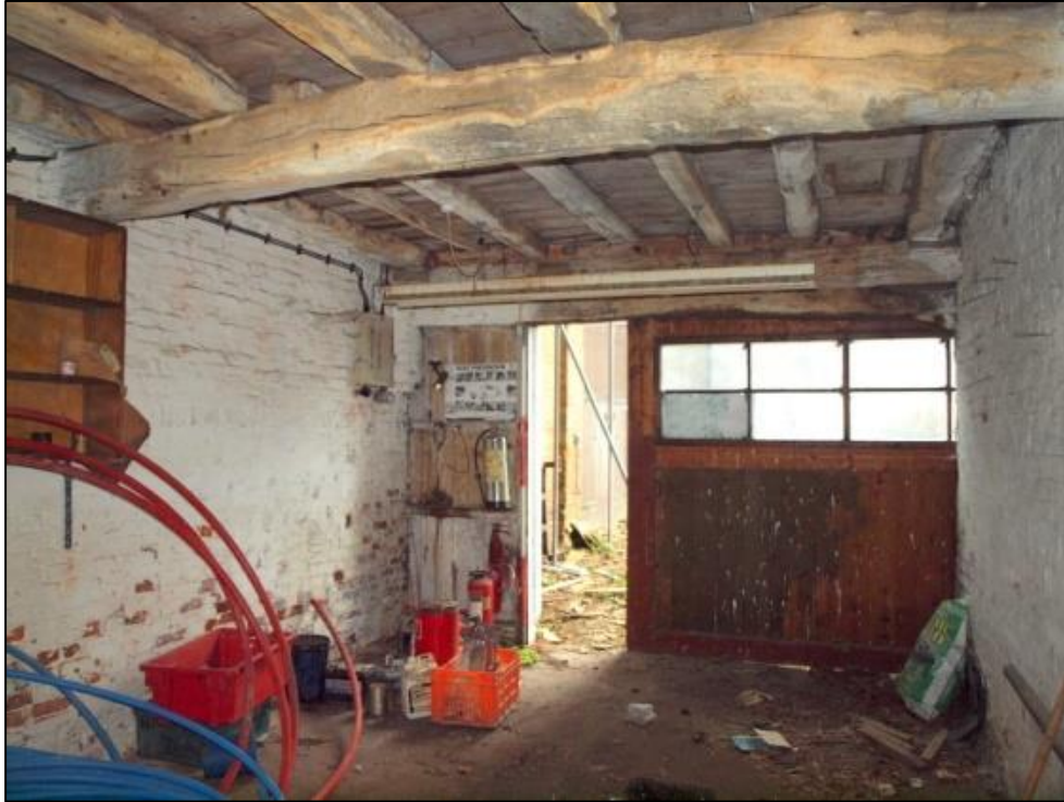
Plate 30: Room 5 looking west
