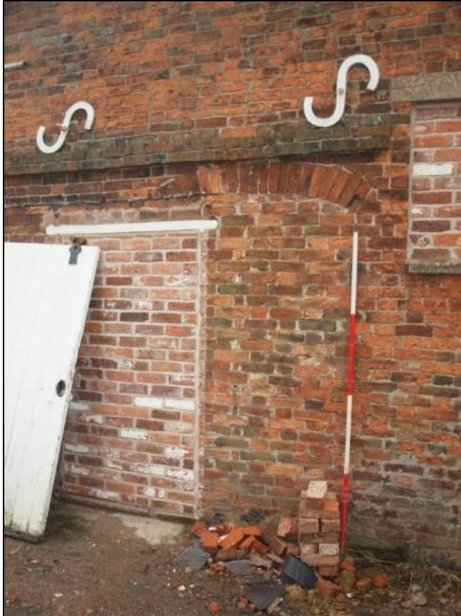
Plate 11: Detail of overlapping blocked doorways
