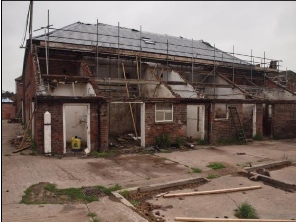
Plate 6: East elevation of lean-to from south
