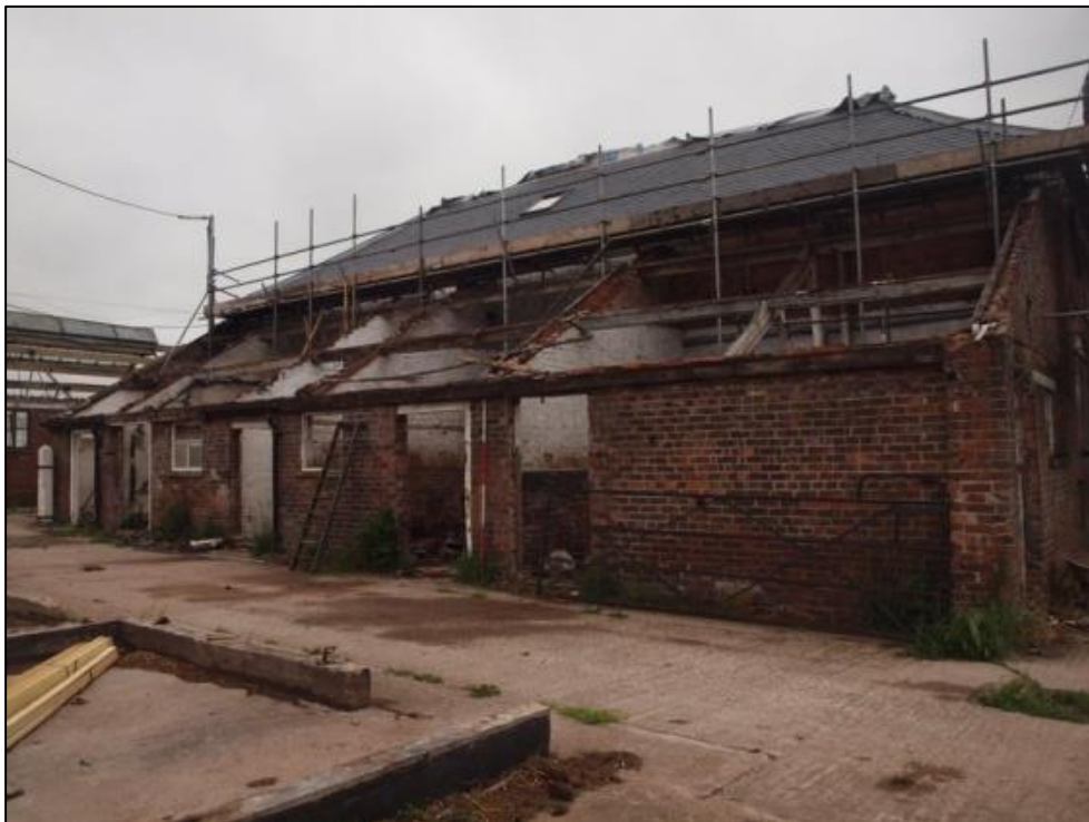
Plate 5: East elevation of lean-to from north
