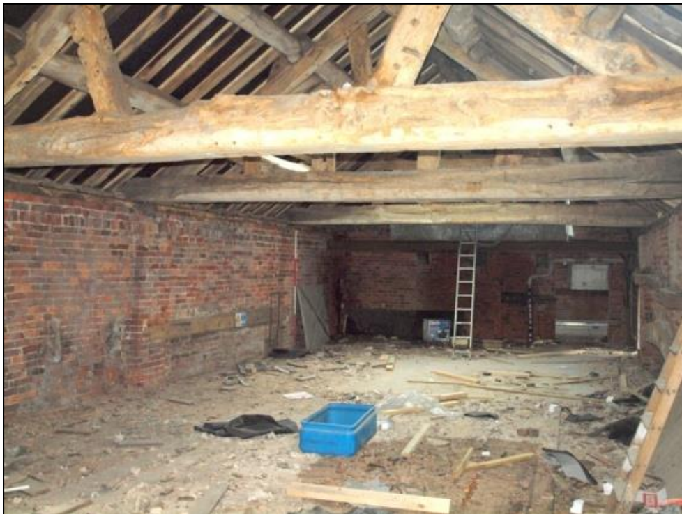
Plate 55: Room 15 looking west
