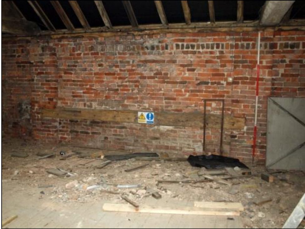
Plate 56: Detail of beam in centre of south wall
