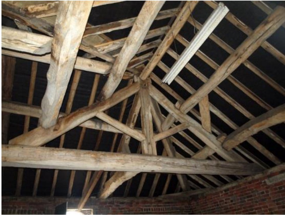
Plate 50: King post truss
