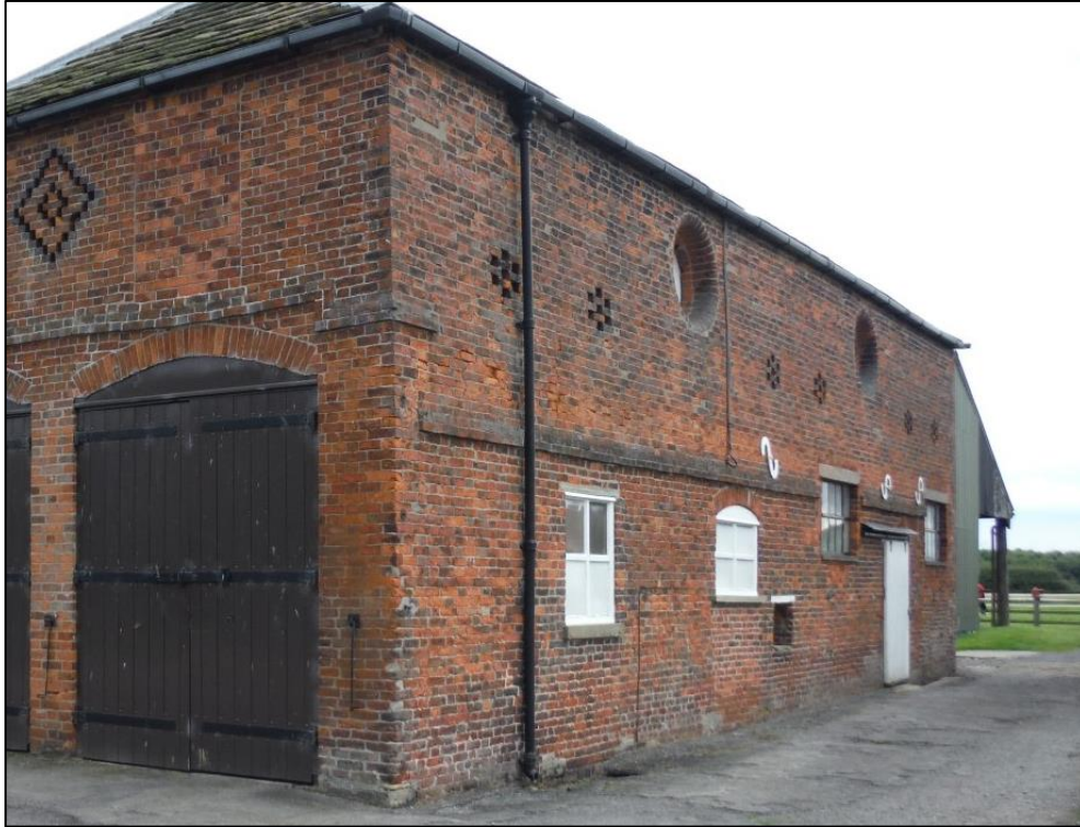
Plate 12a: As above before the scaffolding
