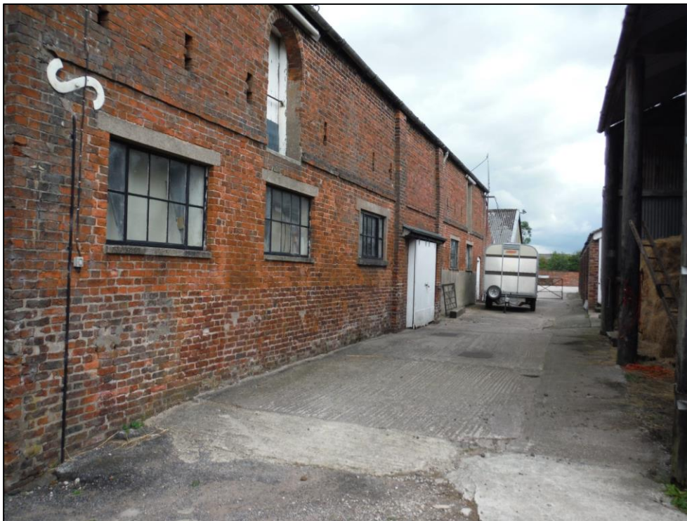
Plate 9a: As above before the scaffolding
