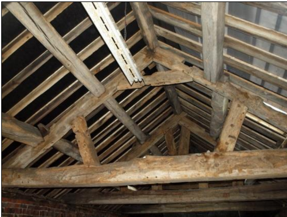
Plate: 59 Angled queen post in room 15
