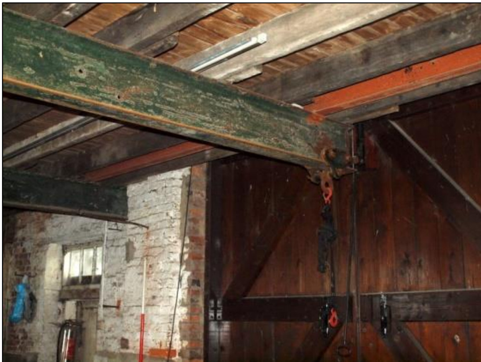
Plate 25: Room 4 showing barn door and RSJ beam
