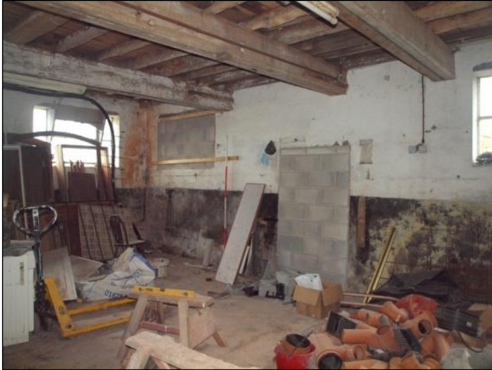
Plate 22: Room 3 looking west
