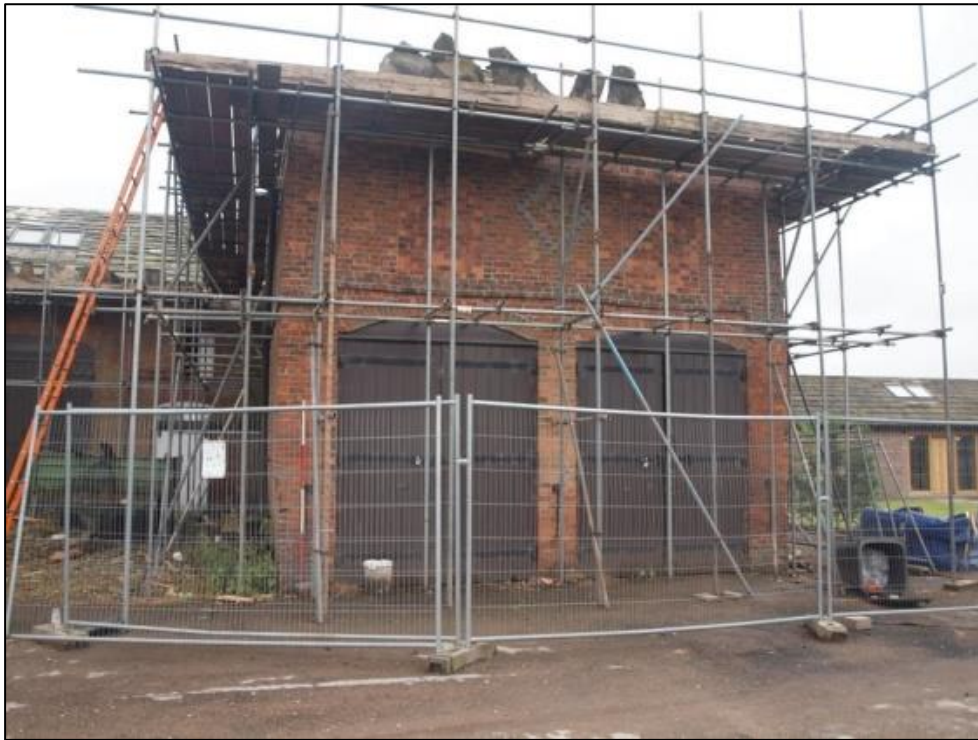
Plate 1: North elevation, west end
