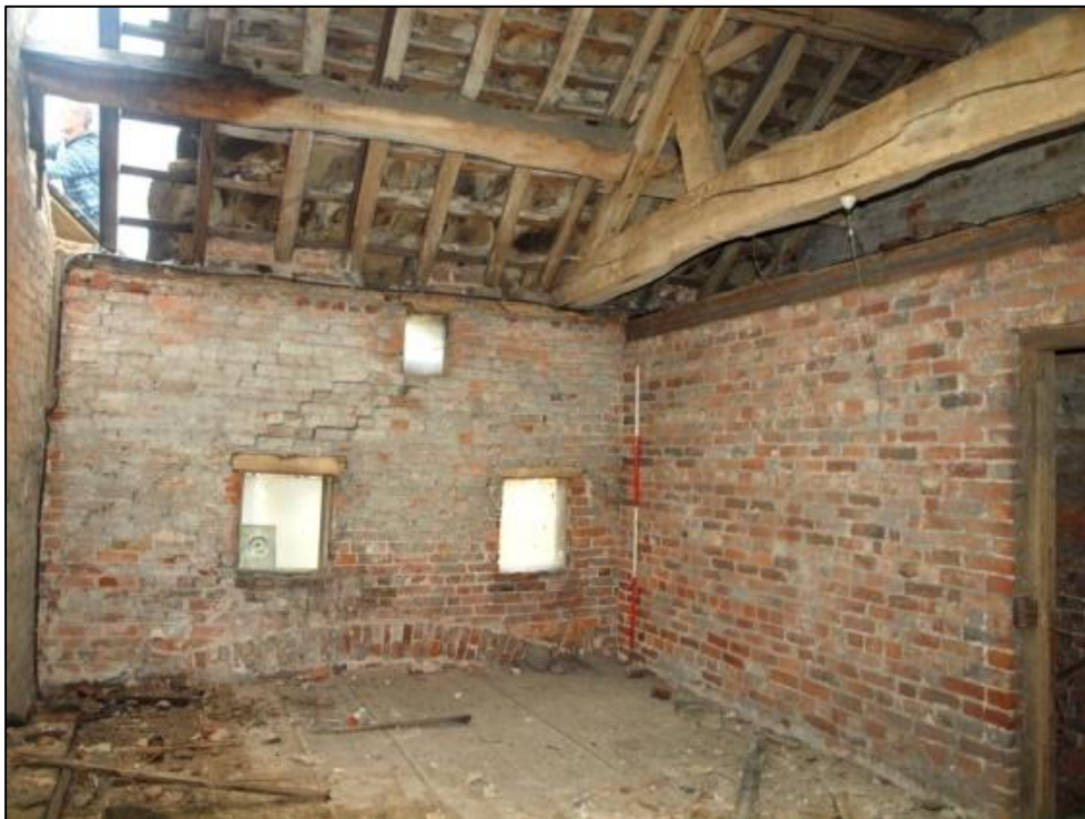
Plate 61: Room 16 looking west
