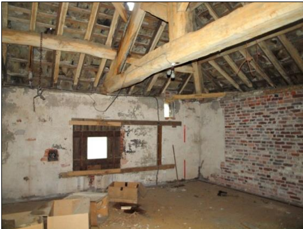
Plate 65: Room 17 looking west
