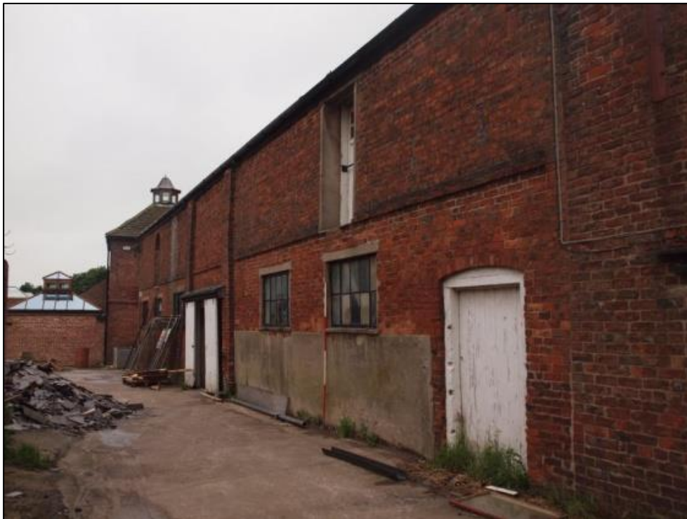
Plate 8: South elevation from east
