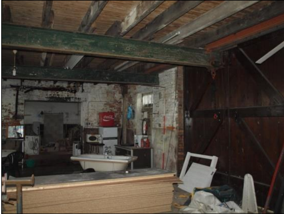
Plate 24: Room 4 looking west
