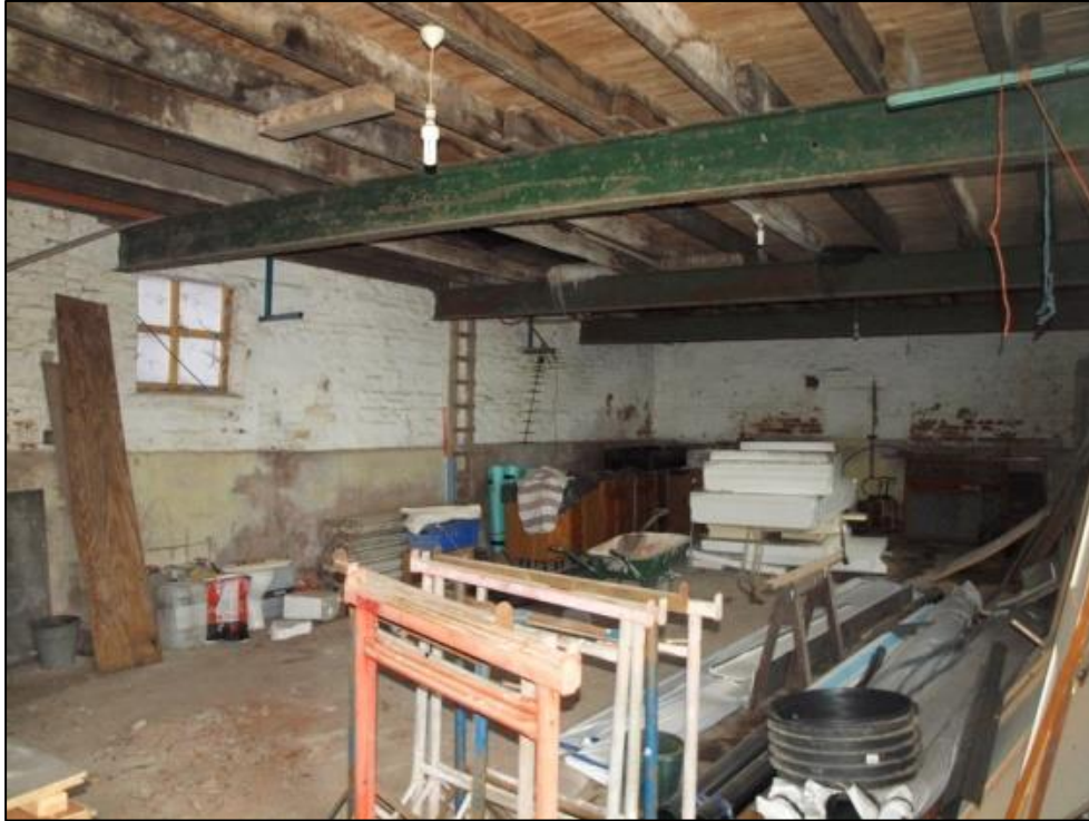
Plate 26: Room 4 looking northeast
