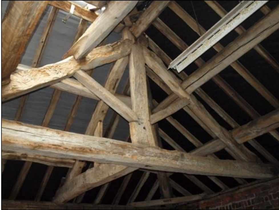
Plate 60: King post truss at east end of room 15
