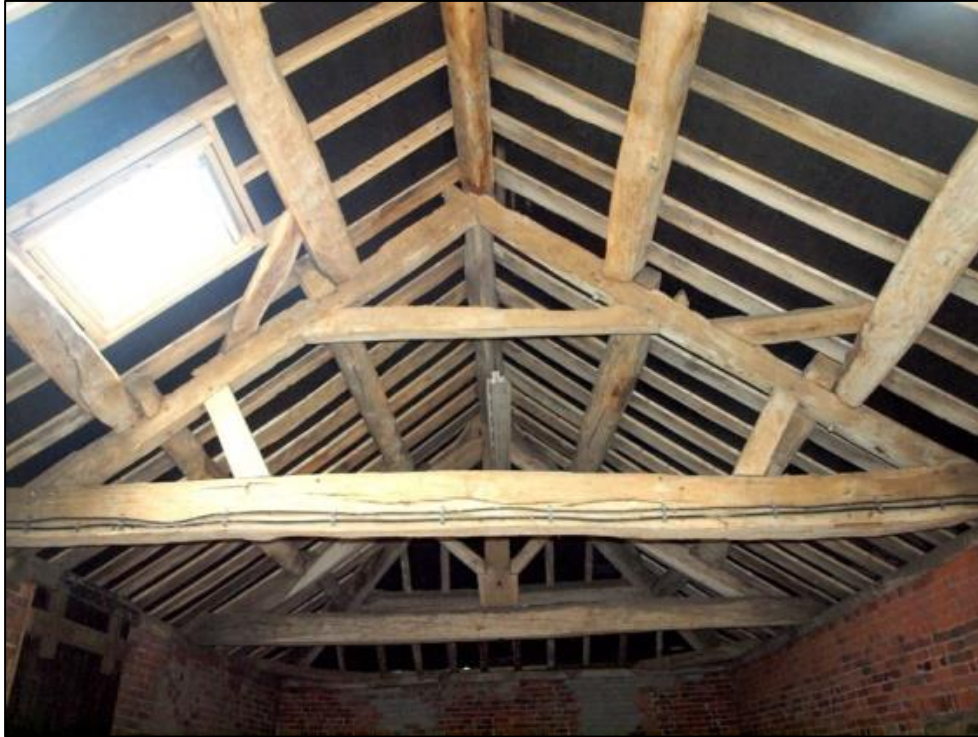
Plate 48: Angled queen post truss
