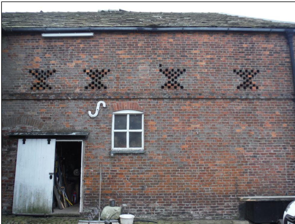
Plate 14a: As above before the scaffolding
