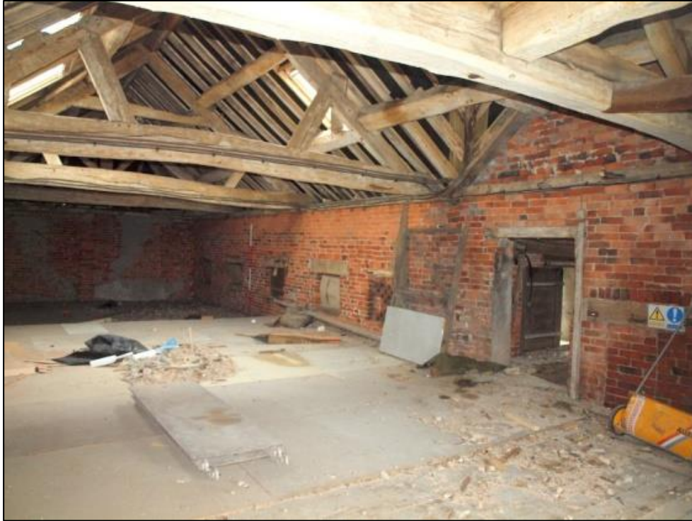
Plate 44: Room 14 blocked alcoves east wall
