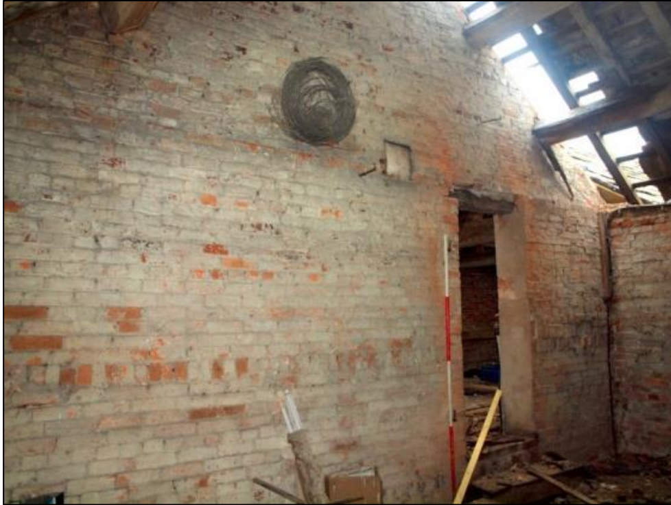
Plate 62: Room 16 looking south
