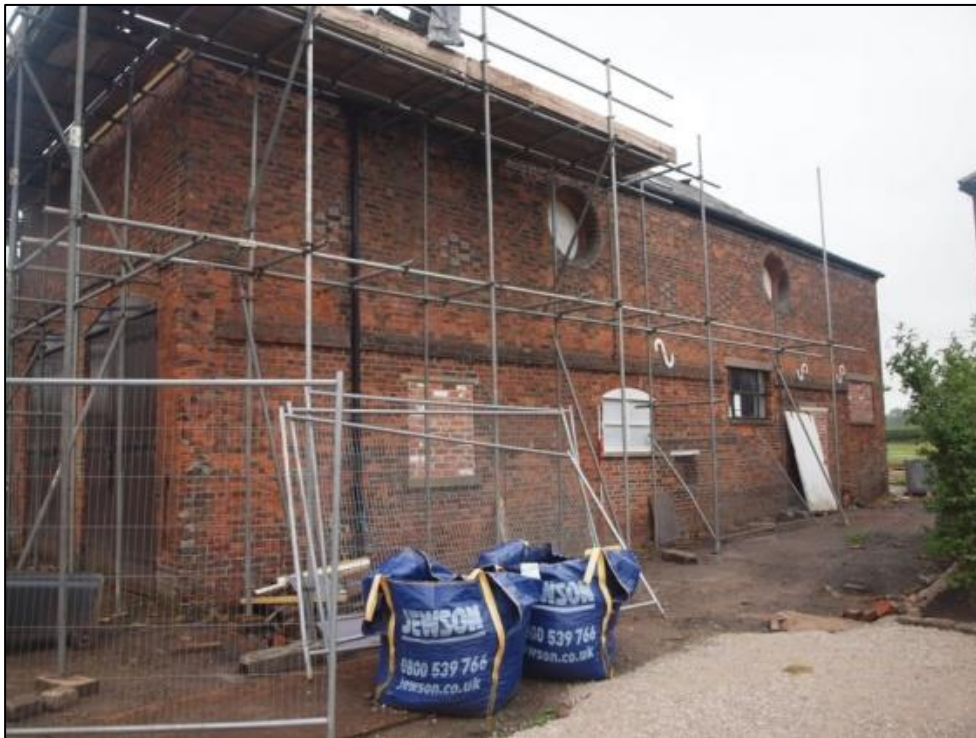
Plate 12: West elevation from north
