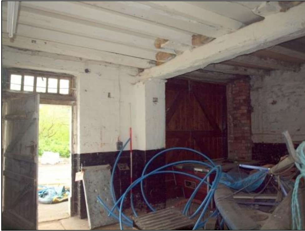
Plate 34: Room 7 looking north
