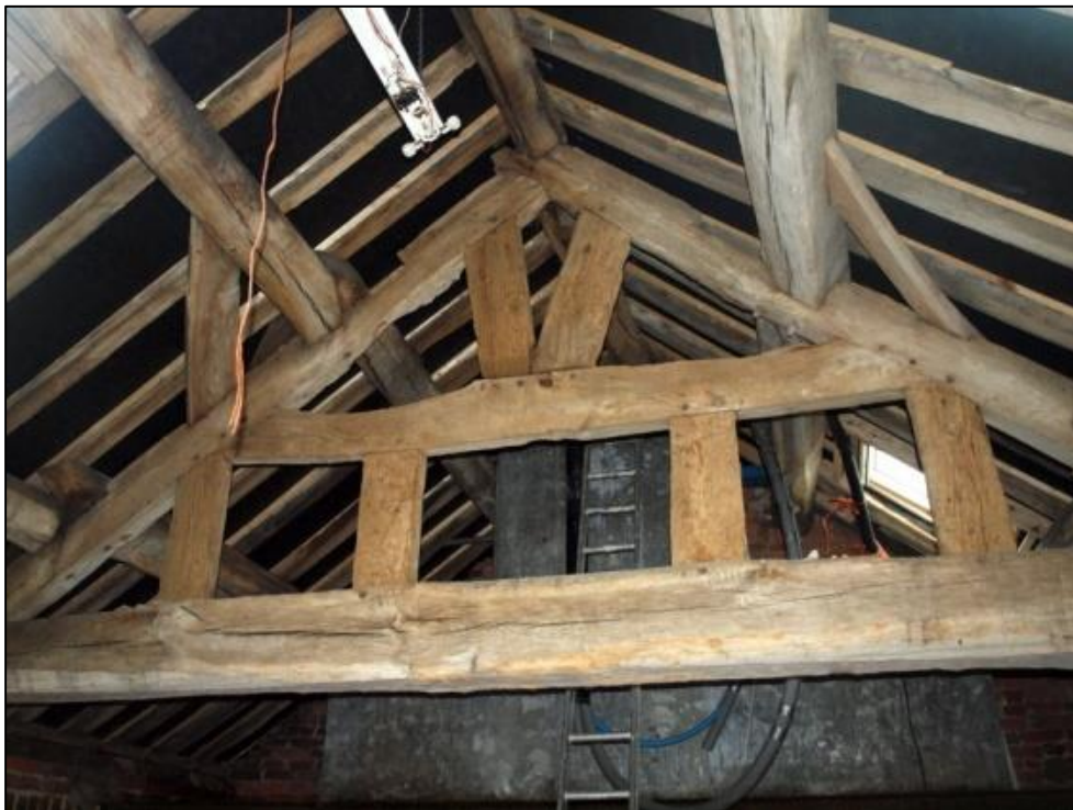
Plate 57: Modified queen post at west end of room 15
