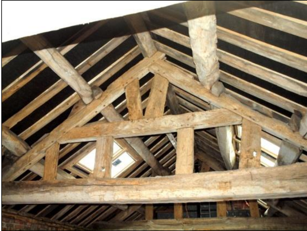
Plate 58: Modified queen post in room 15
