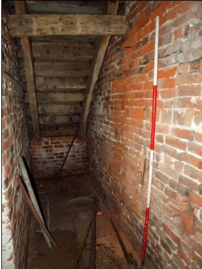
Plate 32: Space below stairs
