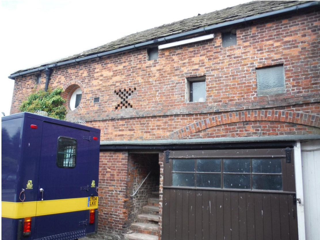
Plate 16a: As above before the scaffolding
