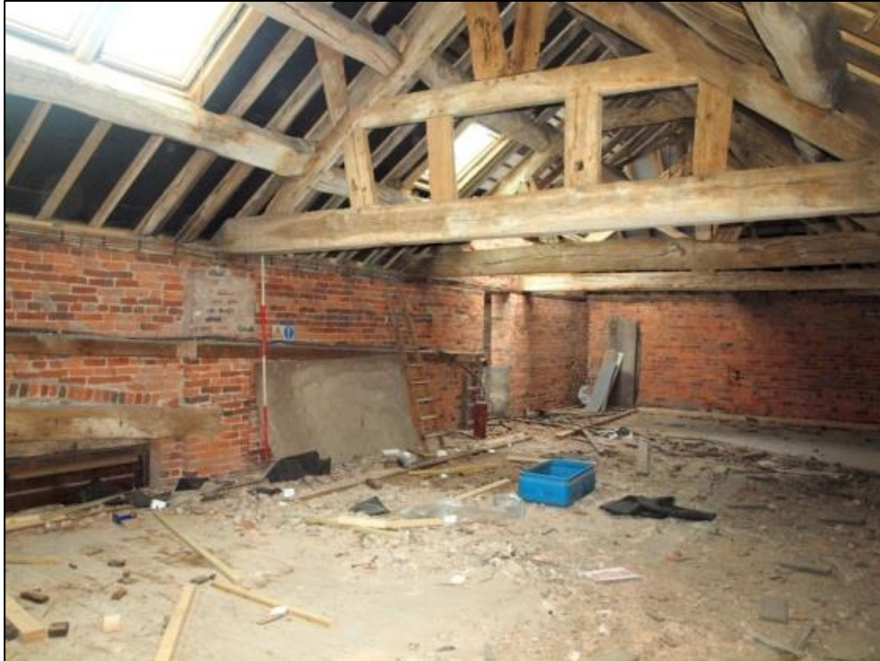
Plate 52: Room 15 looking northeast
