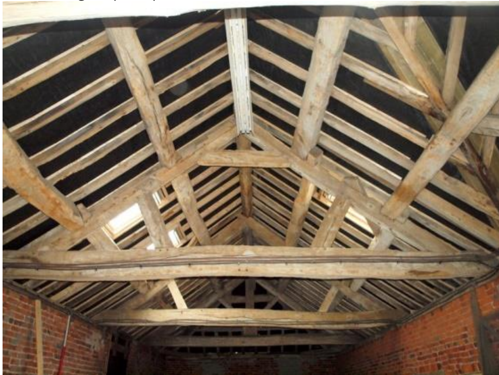
Plate 49: Angled queen post truss
