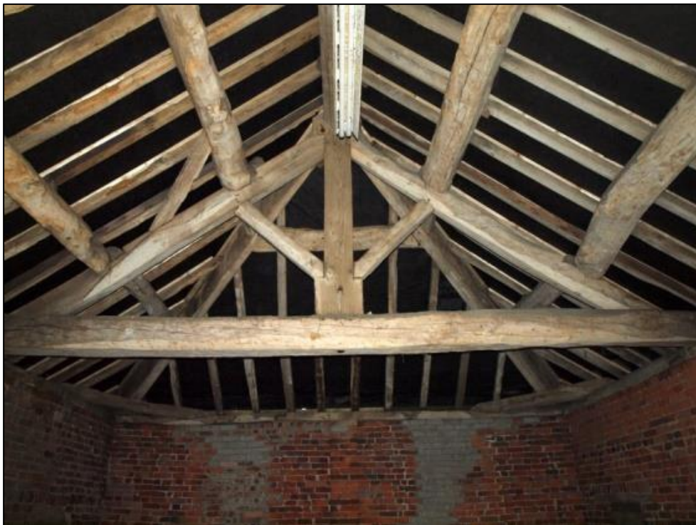
Plate 47: King post truss at north end
