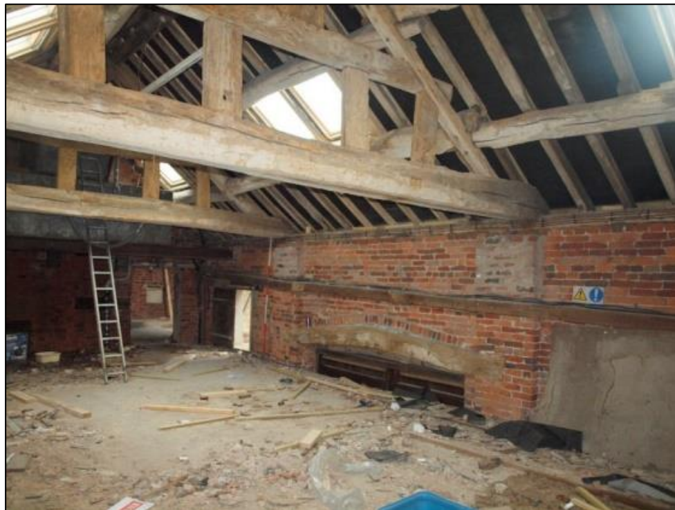
Plate 51: Room 15 looking northwest
