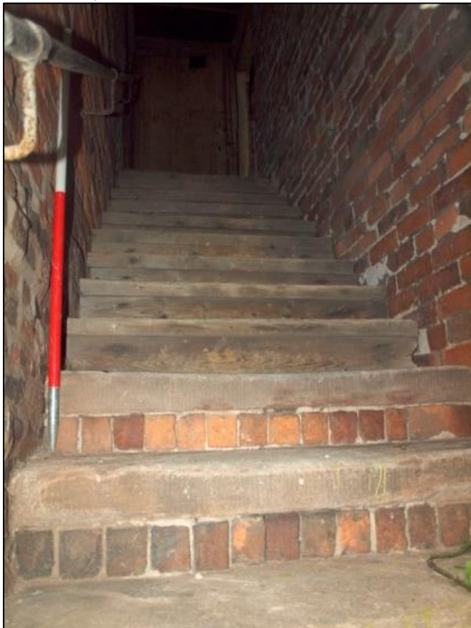
Plate 33: Stairs to first floor
