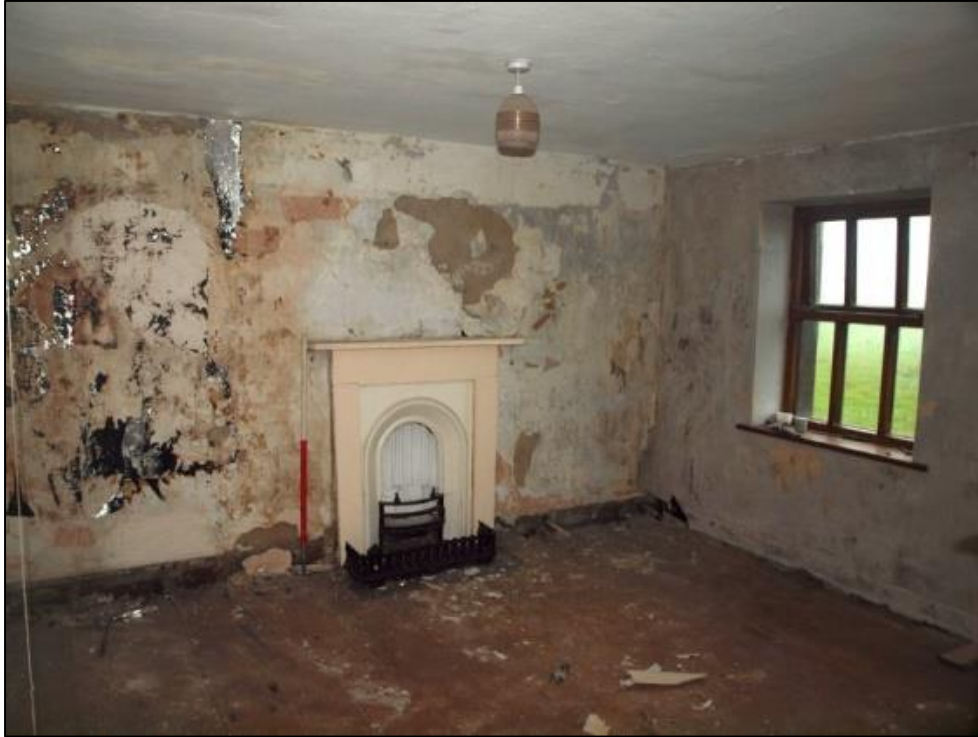
Plate 33: Fireplace in central bedroom on north side
