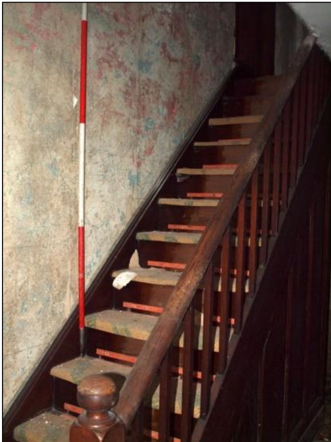
Plate 14: Staircase to first floor
