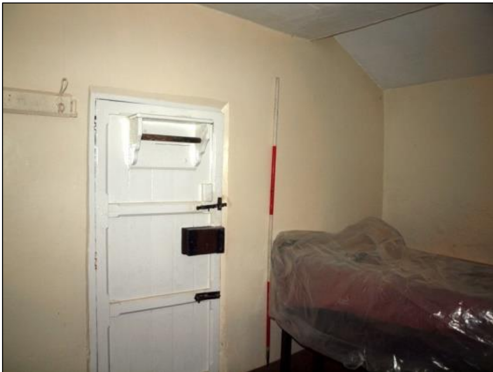
Plate 24: Utility extension doorway to porch
