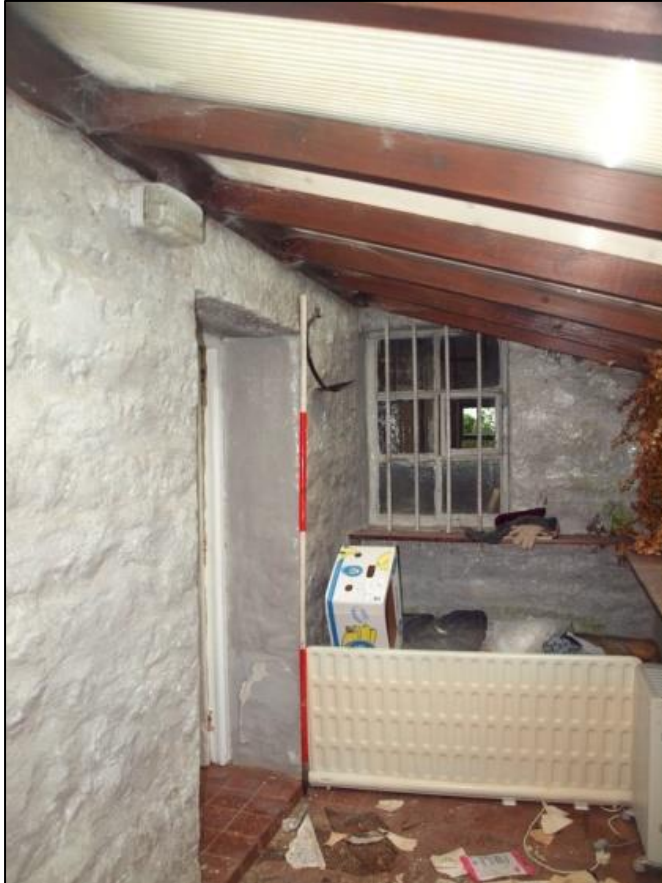
Plate 27: Window of in porch looking into pantry
