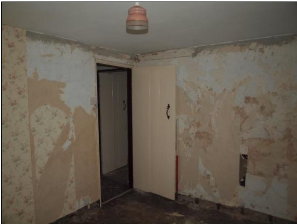
Plate 34: Bedroom in western corner
