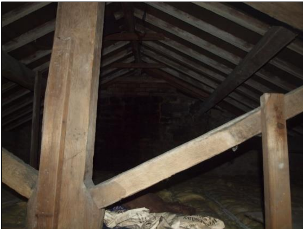
Plate 36: King post truss of machine cut timber
