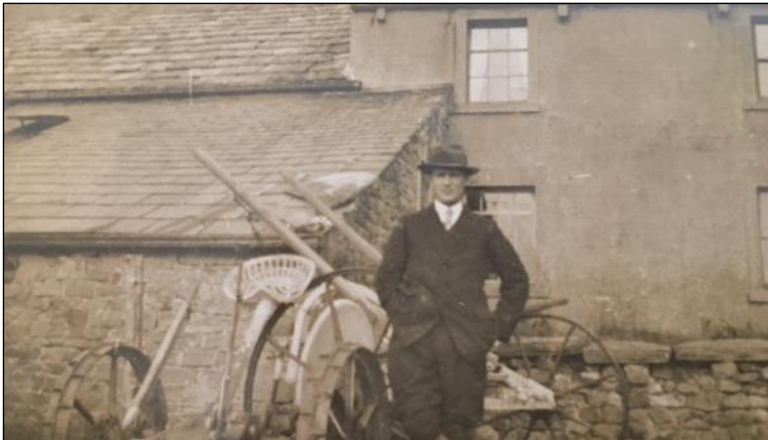
Figure 8: Photograph showing the southwest elevation of the house c. 1900. Note the nine paned window at first floor level which has since been replaced
