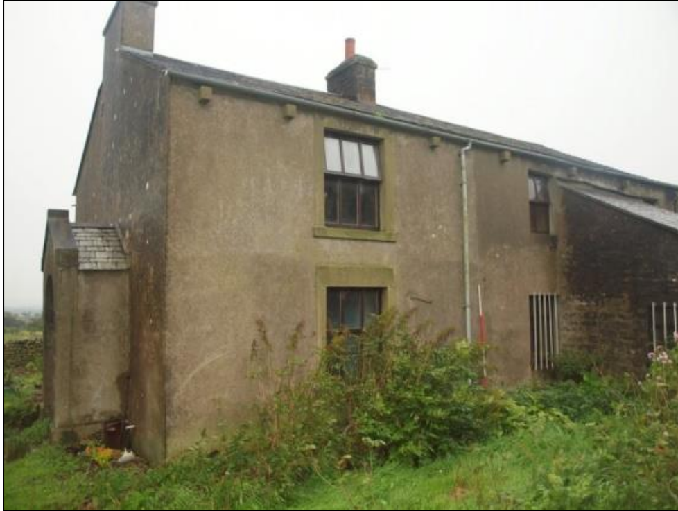
Plate 5: Detail of southern end of northeast elevation
