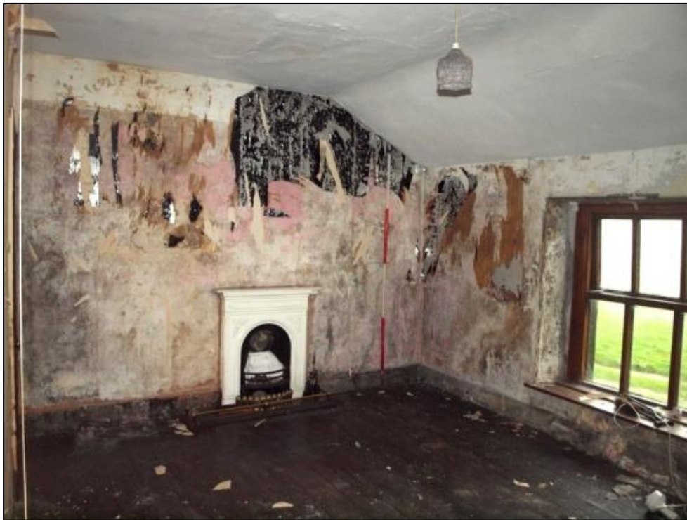
Plate 28: First floor bedroom in southern corner
