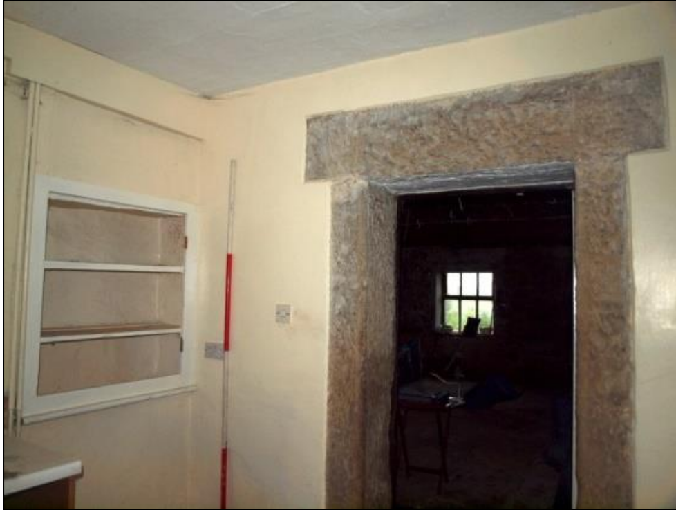
Plate 23: Utility extension doorway to dining room
