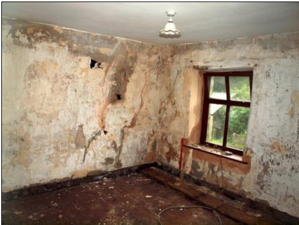
Plate 32: Bedroom in northern corner
