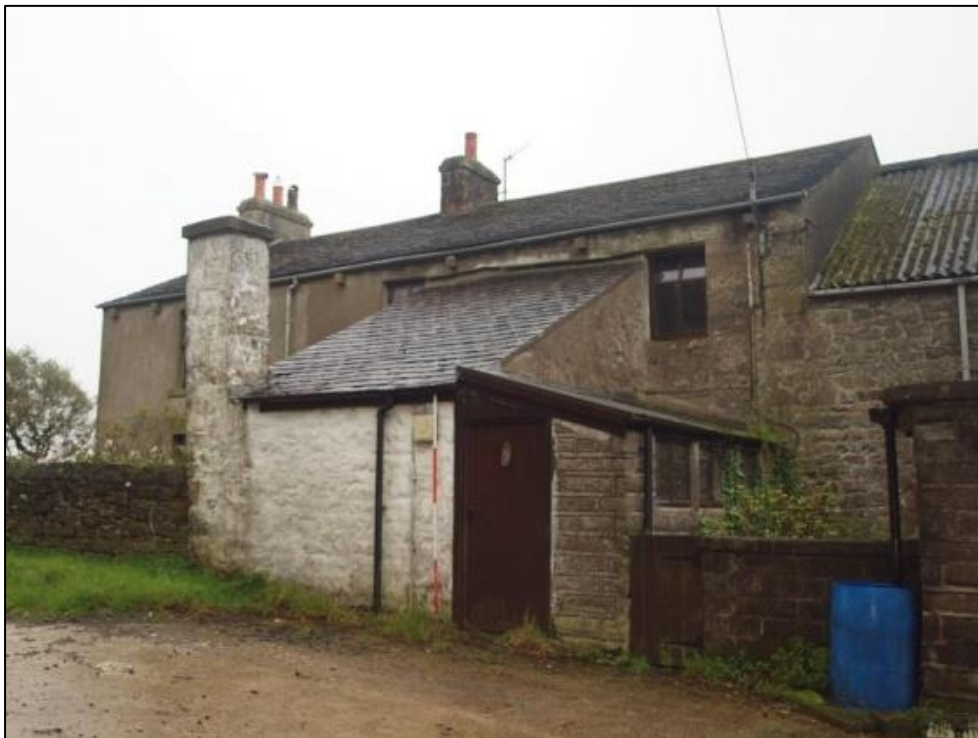
Plate 6: Detail of northern end of northeast elevation
