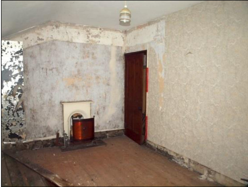
Plate 29: First floor bedroom in eastern corner
