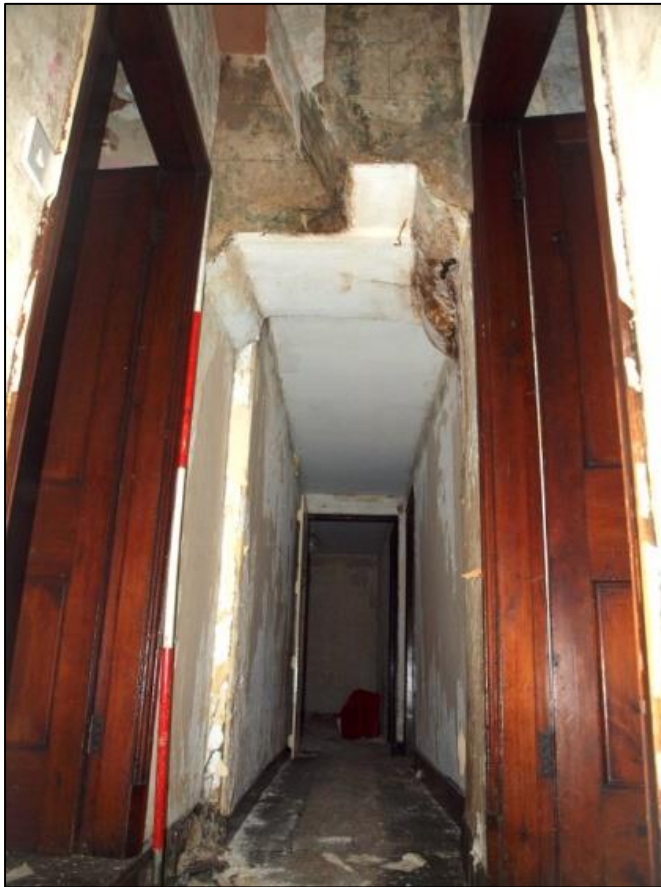
Plate 30: Central corridor of first floor showing cut through chimney stack above
