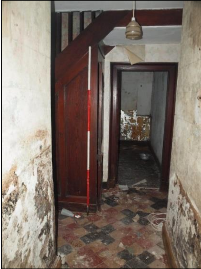
Plate 15: Northwest end of corridor looking towards living room
