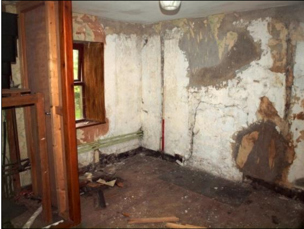
Plate 31: Blocked fireplace in central bedroom on north side
