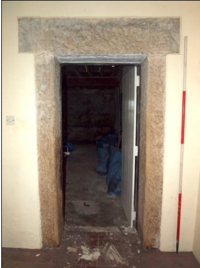
Plate 25: Detail of doorway to dining room
