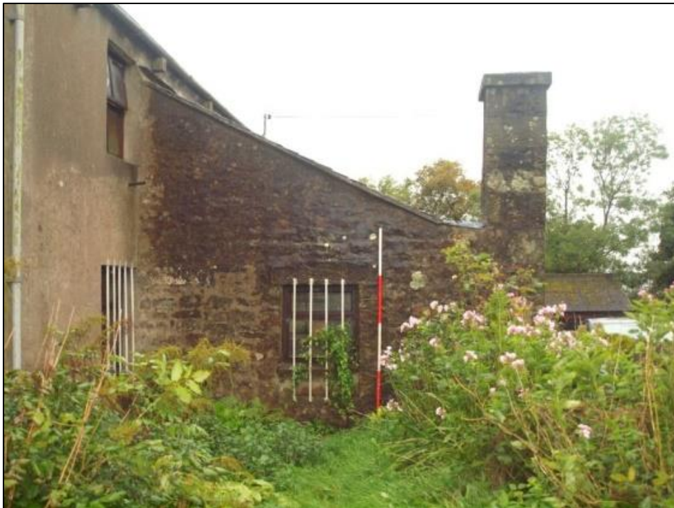
Plate 10: Southeast elevation of utility extension
