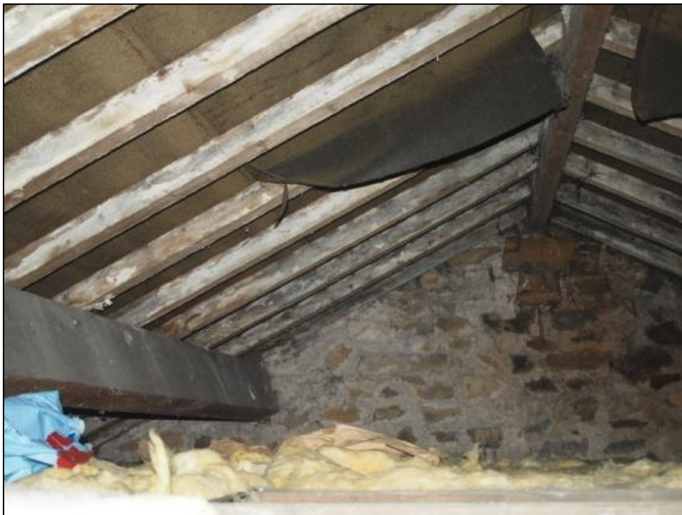
Plate 38: Attic space in southeastern extension
