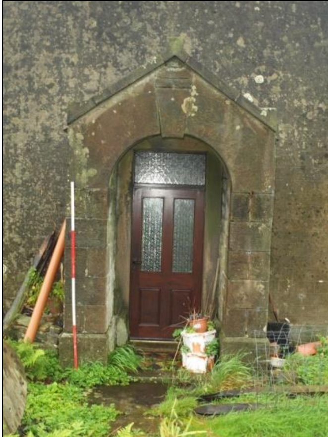
Plate 9: Detail of porch and doorway
