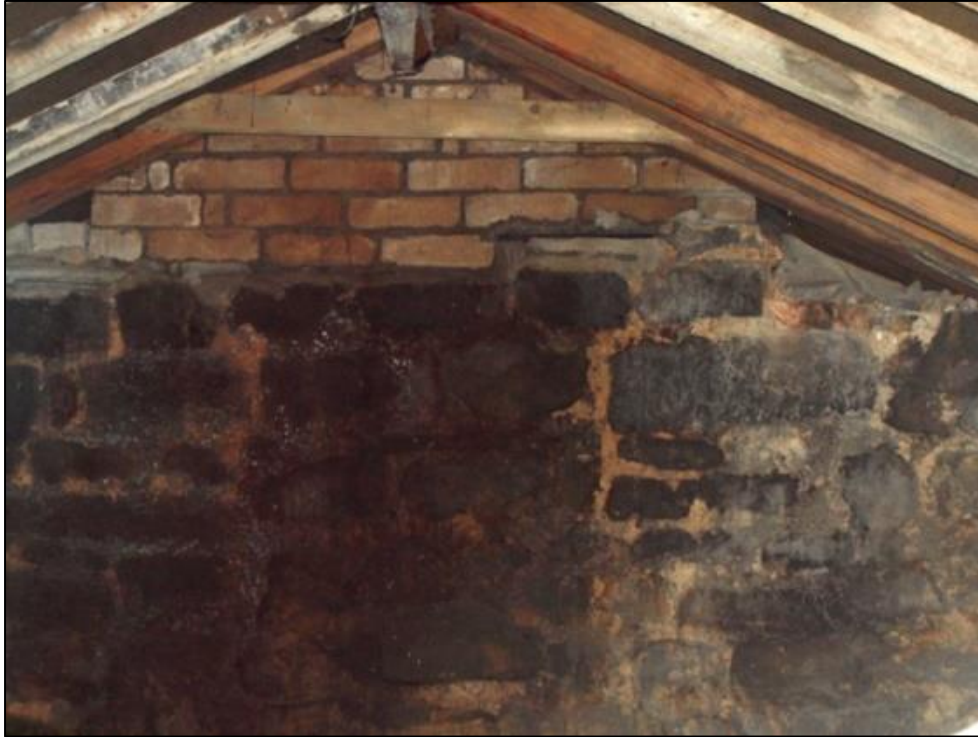
Plate 37: Possible blocked opening in stone cross wall
