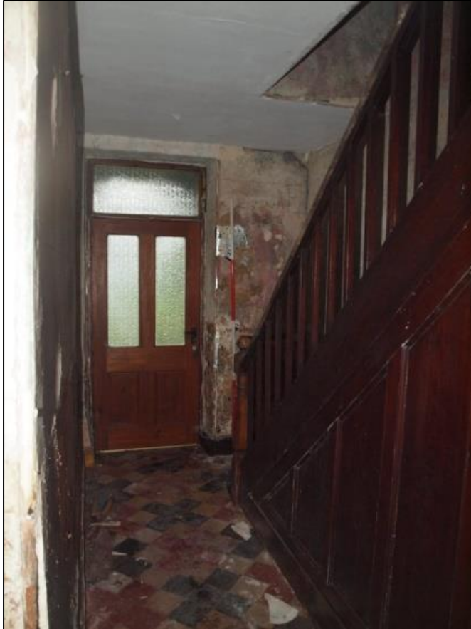
Plate 13: Ground floor tiled corridor
