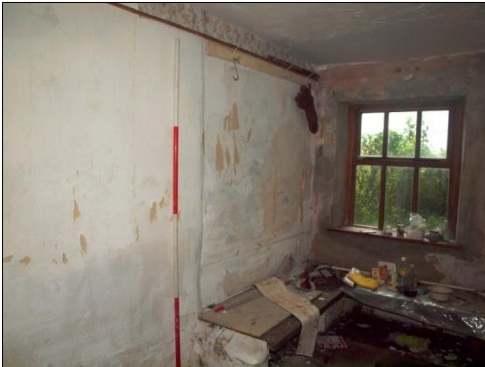
Plate 22: Southeast wall of pantry showing change in thickness
