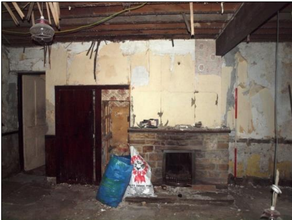
Plate 20: Southeast wall of dining room showing fireplace
