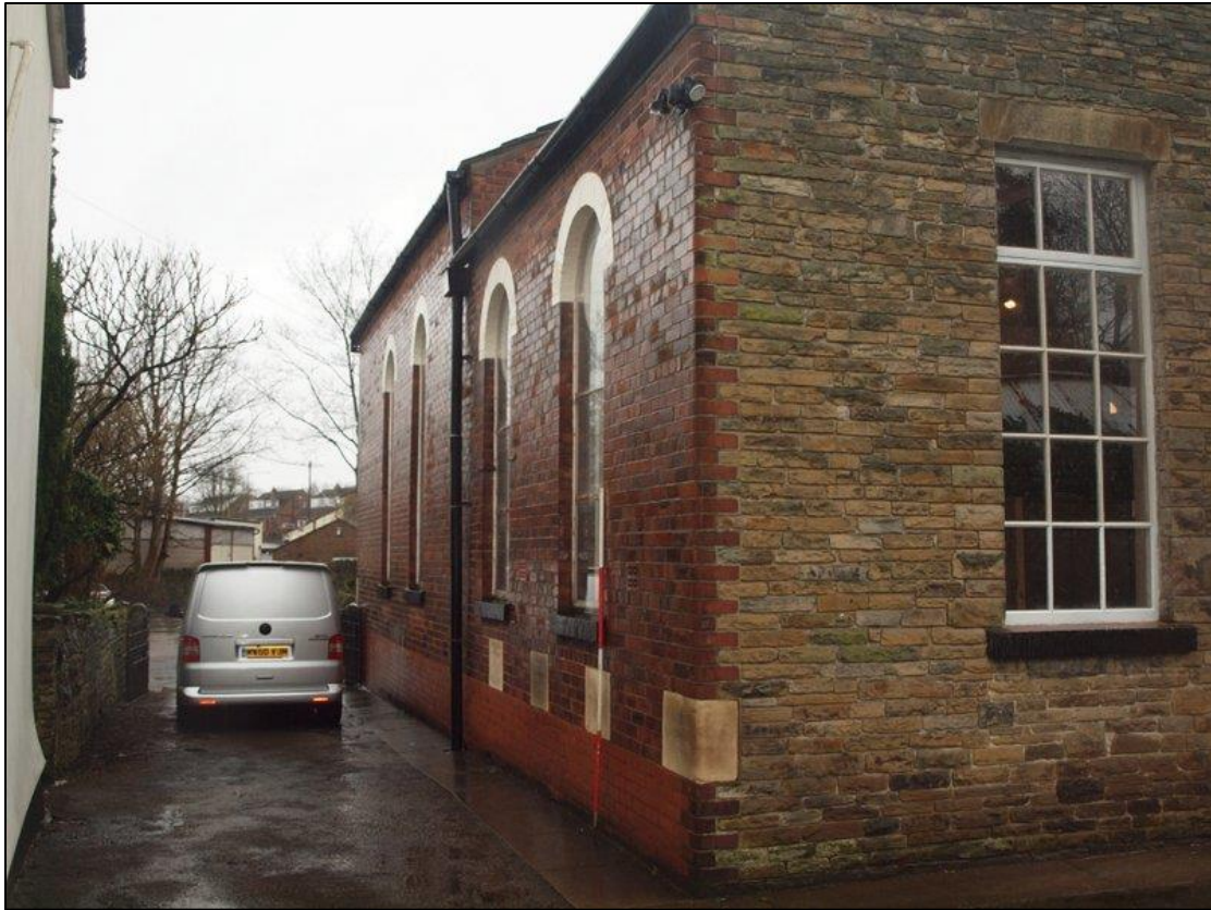
Plate 7: East elevation from north
