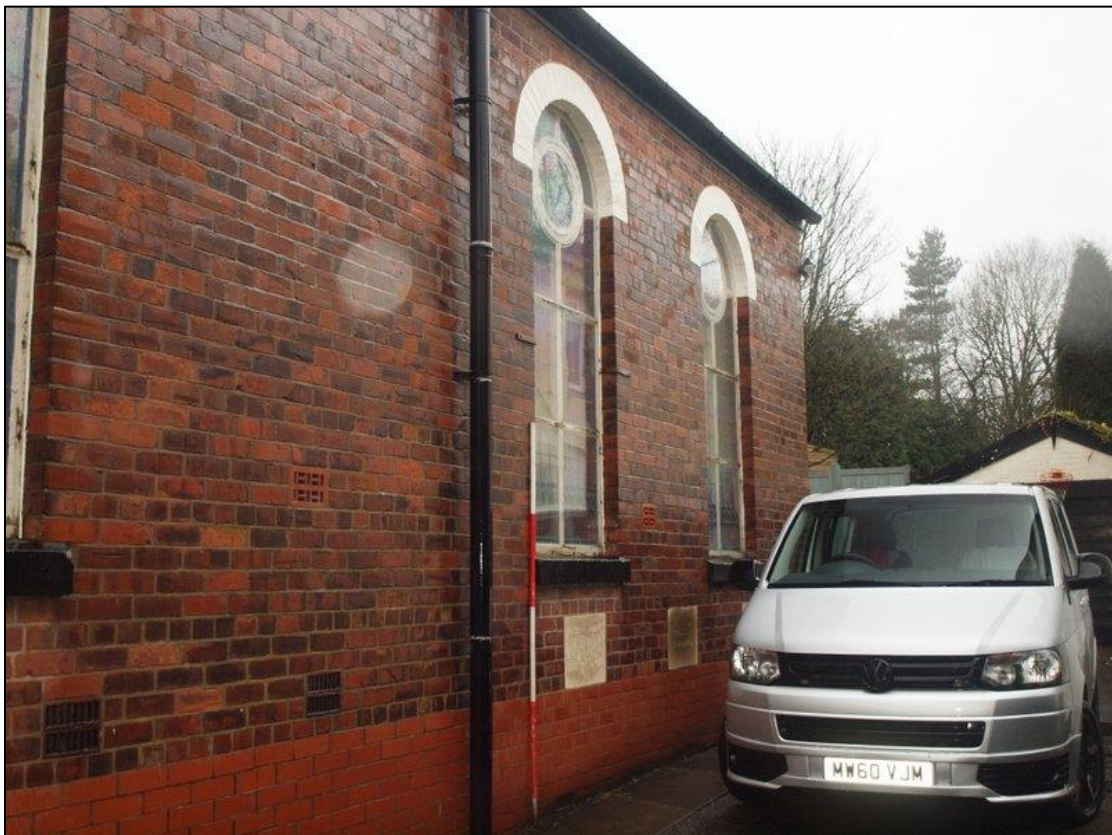
Plate 6: East elevation, north end
