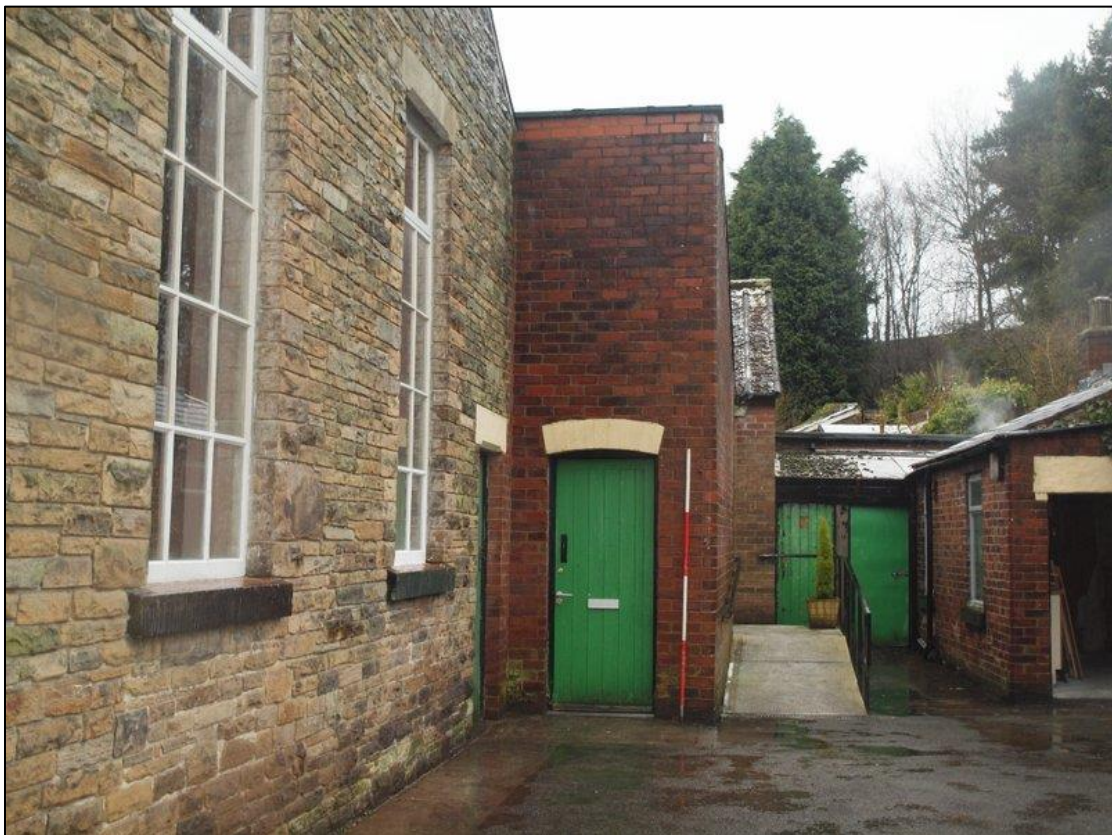
Plate 8: East elevation of extension
