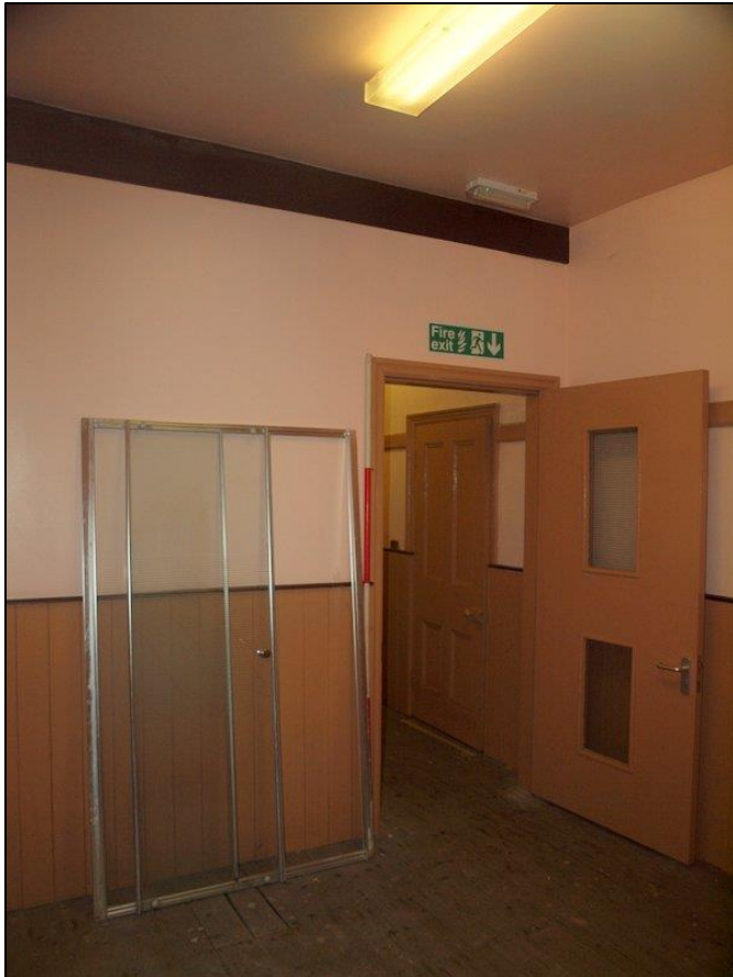
Plate 35: Central room of extension
