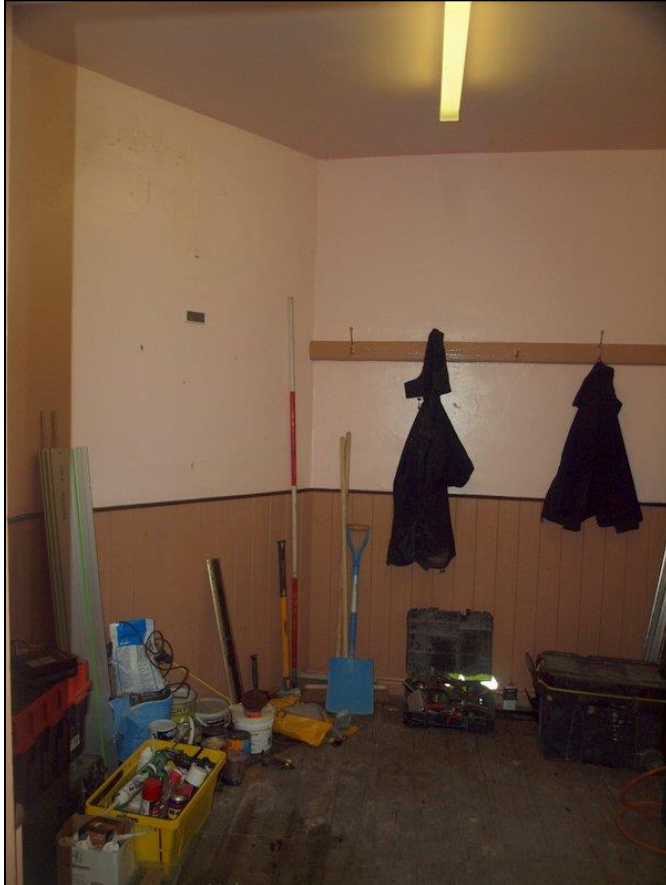
Plate 36: Southern room of extension
