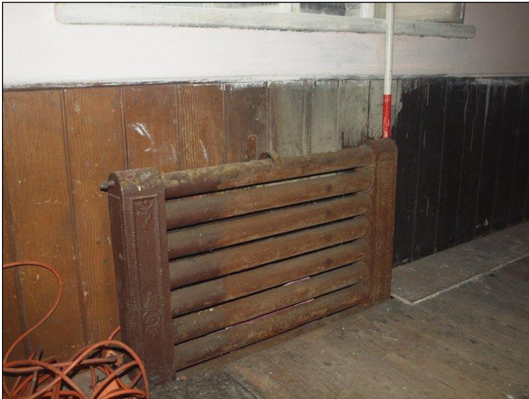
Plate 26: Detail of cast iron radiator
