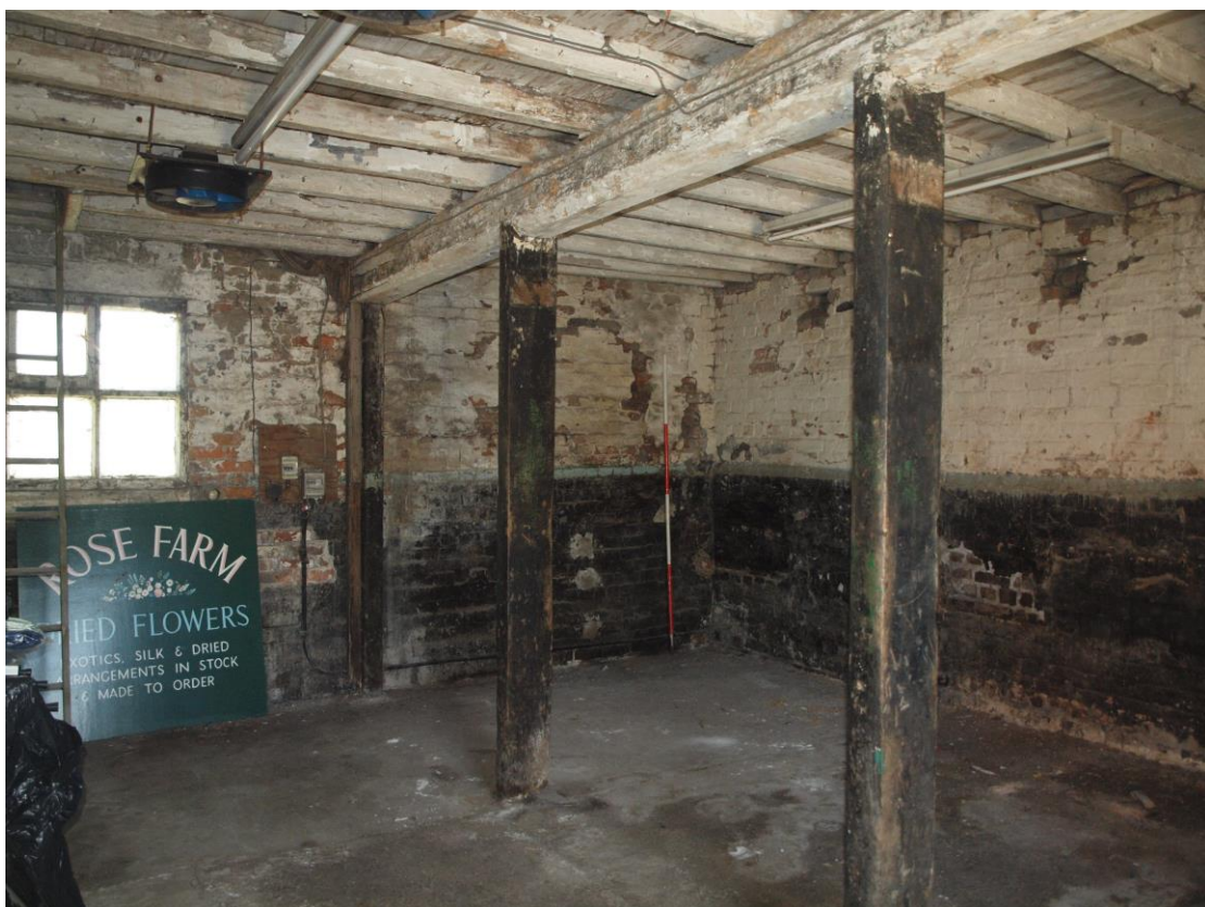
Plate 18: Room 3 showing timber uprights
