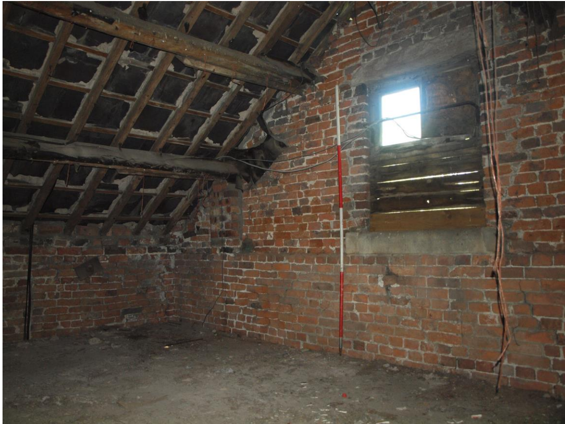
Plate 23: First floor room 1
