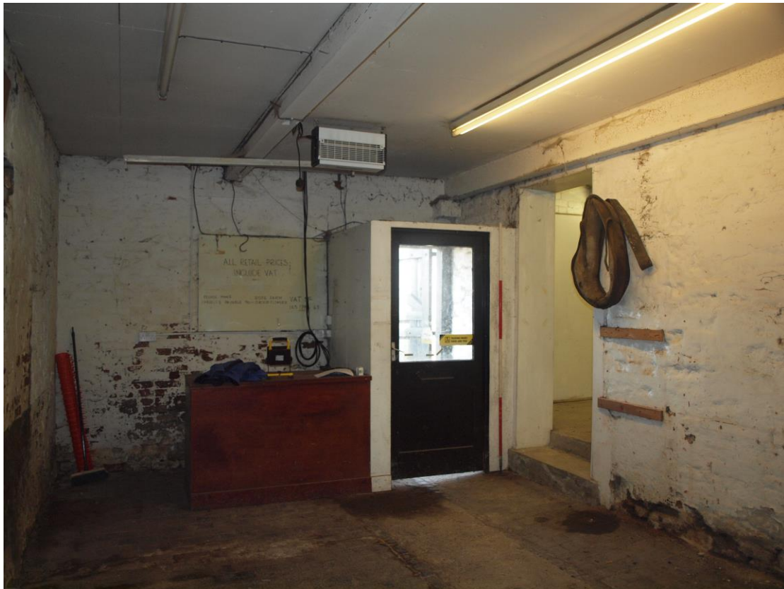
Plate 11: Room 1 showing timber 'porch'
