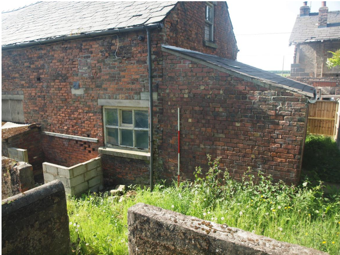
Plate 7: Detail of lean-to at north elevation
