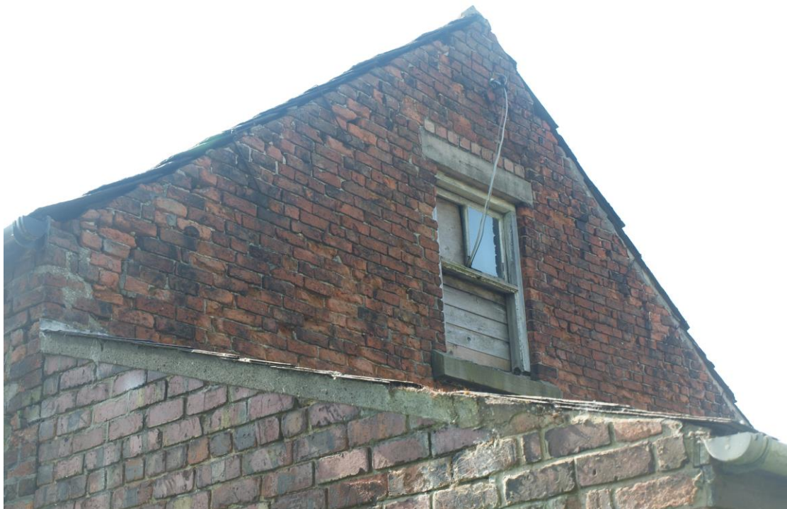
Plate 10: Detail of window in east gable
