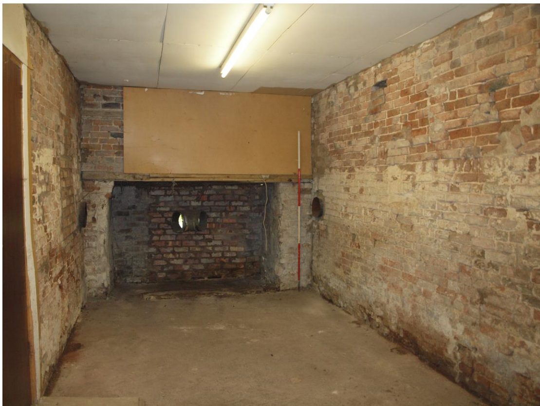
Plate 14: Room 2 showing inserted opening and low extension
