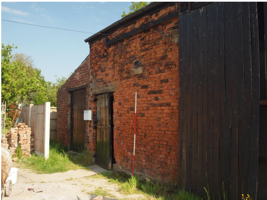
Plate 4: Detail of west end of south elevation
