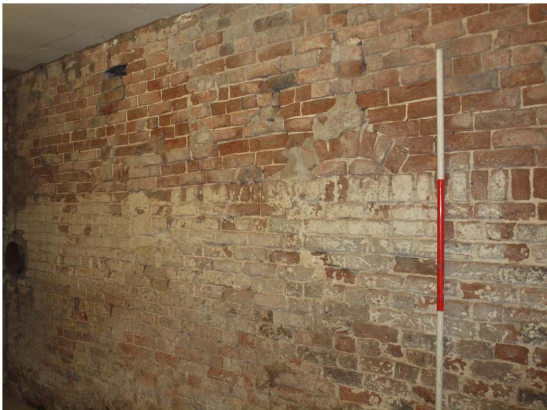
Plate 16: Blocked window detail in east wall
