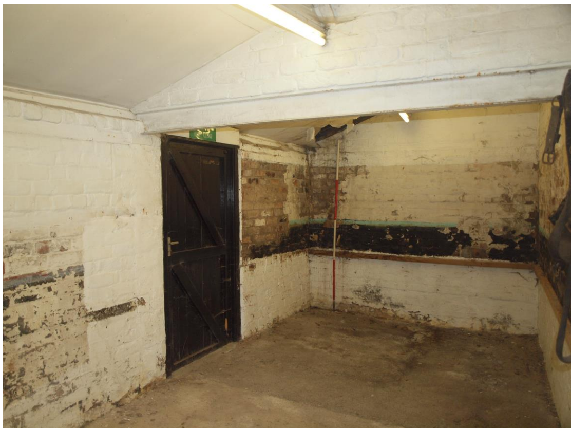
Plate 22: Lean-to interior looking north
