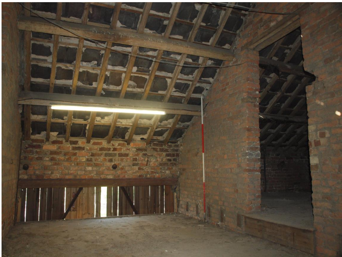
Plate 26: Room 2 showing top of barn door.
