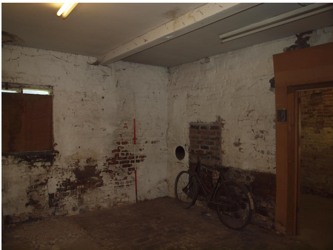
Plate 12: Room 1 showing blocked window and doorway to room 2
