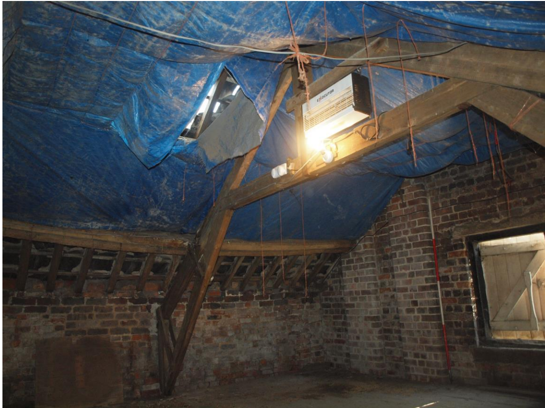
Plate 29: Truss detail in room 3
