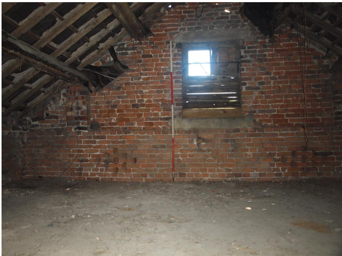
Plate 24: Window and flanking piers
