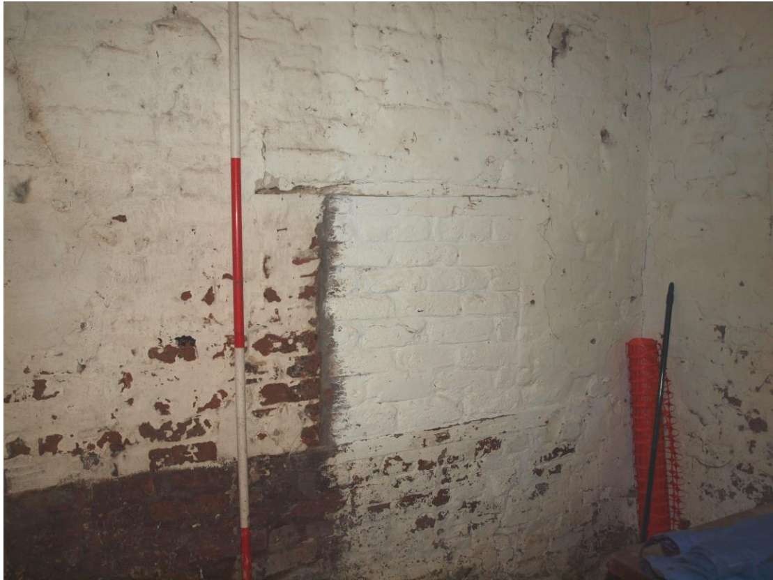
Plate 13: Detail of blocked window
