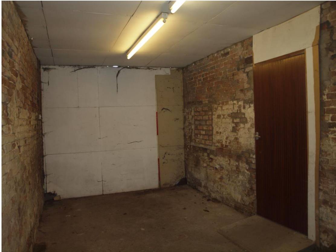
Plate 15: Southern wall blocking the barn door
