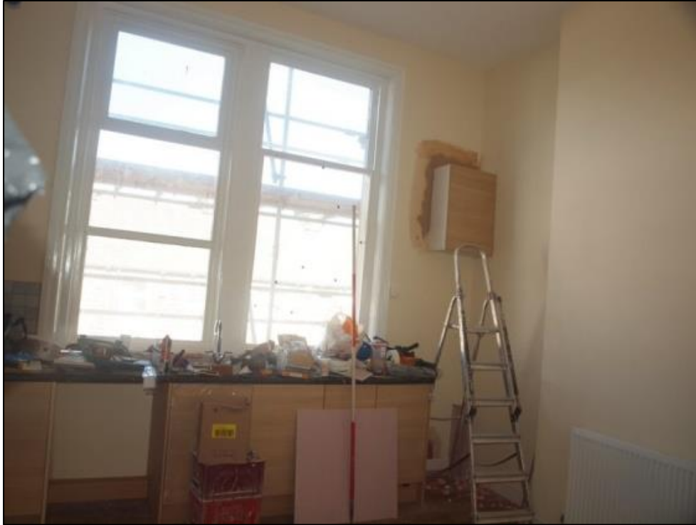
Plate 33: First floor room
