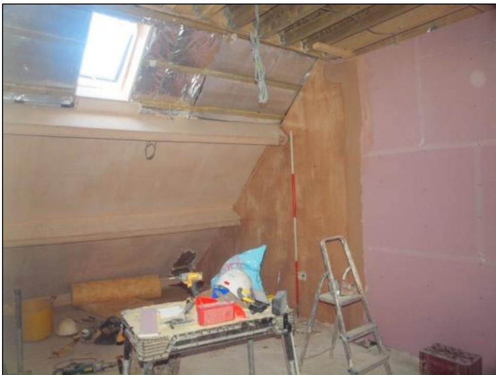
Plate 70: Converted attic space showing purlins
