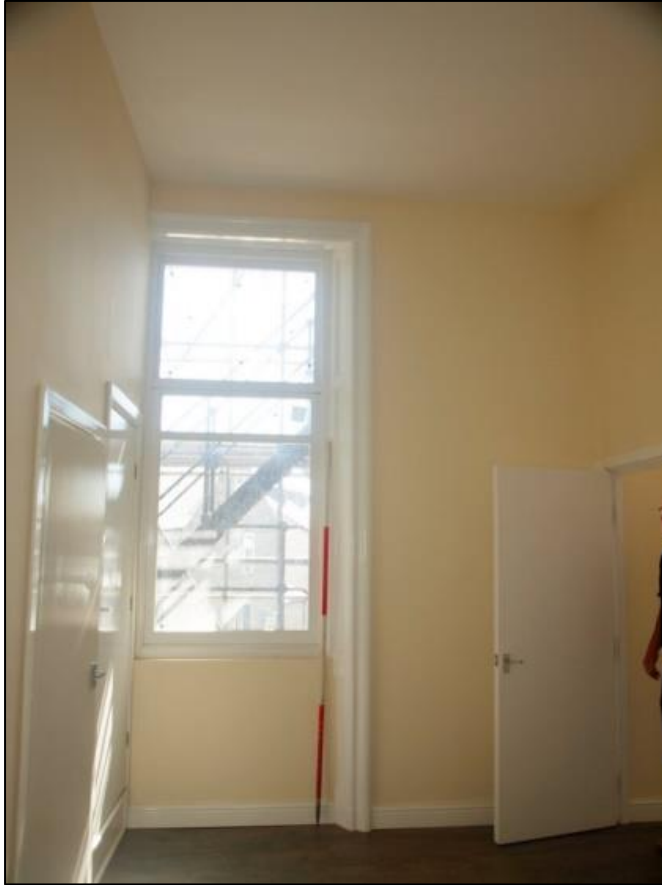
Plate 39: First floor window cut by inserted wall
