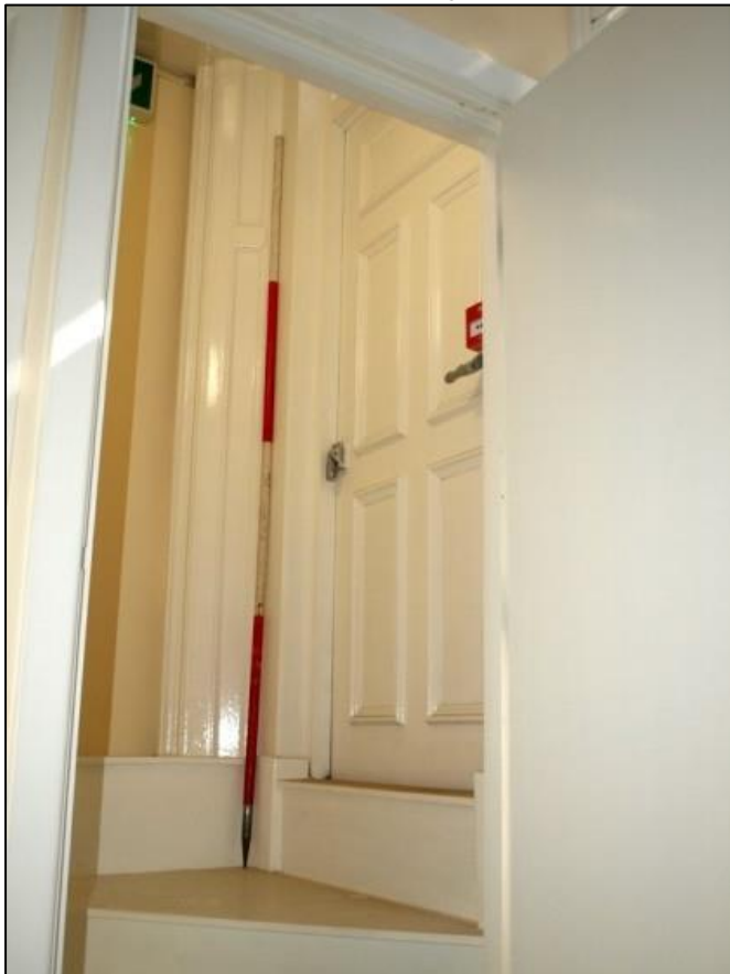
Plate 40: First floor door to fire escape
