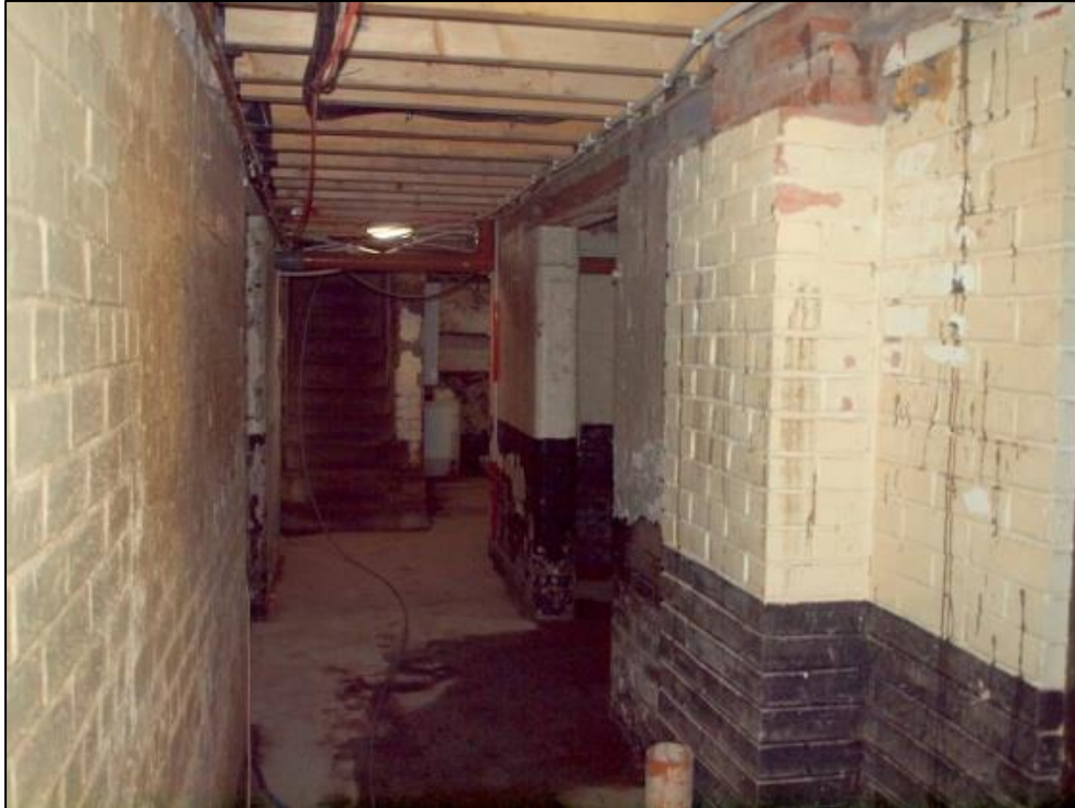
Plate 87: Basement room 4 northern end
