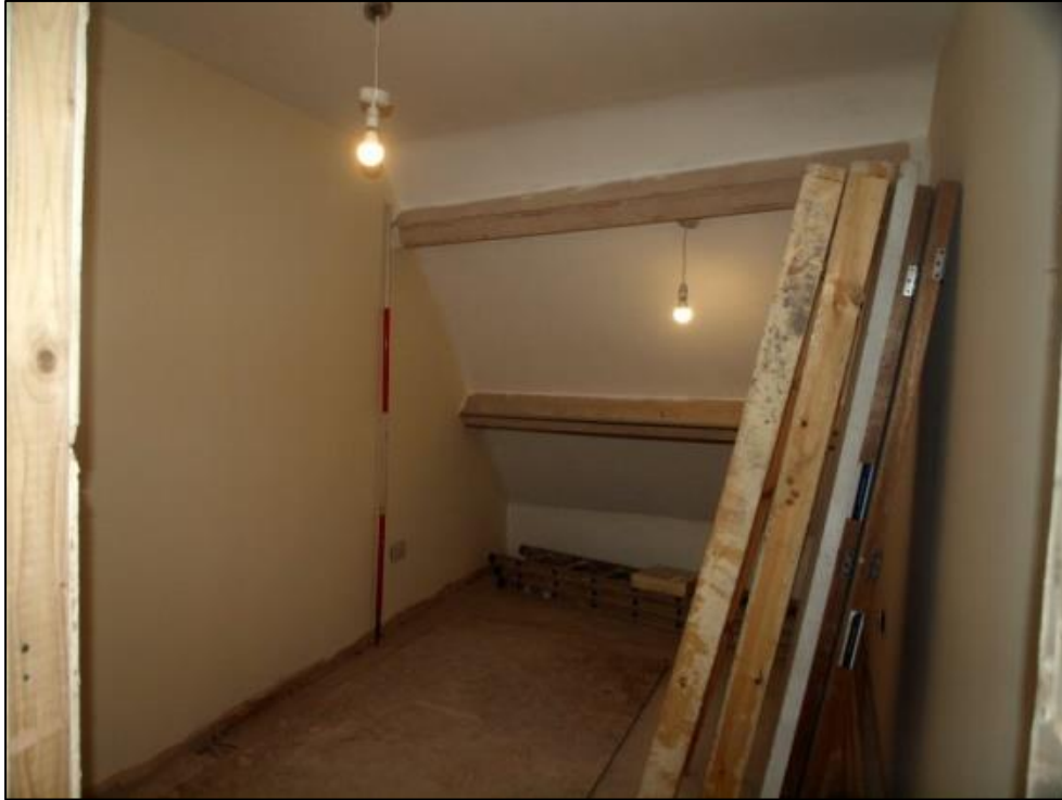
Plate 71: Converted attic space showing purlins
