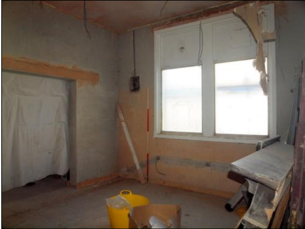
Plate 23: Ground floor room 6
