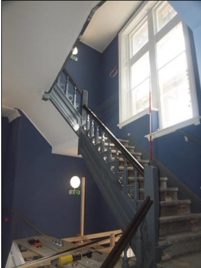
Plate 51: Main staircase to second floor
