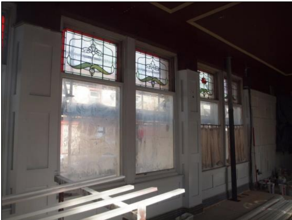
Plate 8; Ground floor room 1
