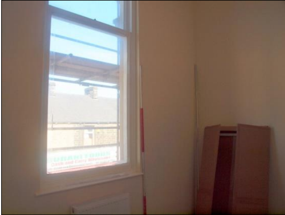
Plate 31: First floor room
