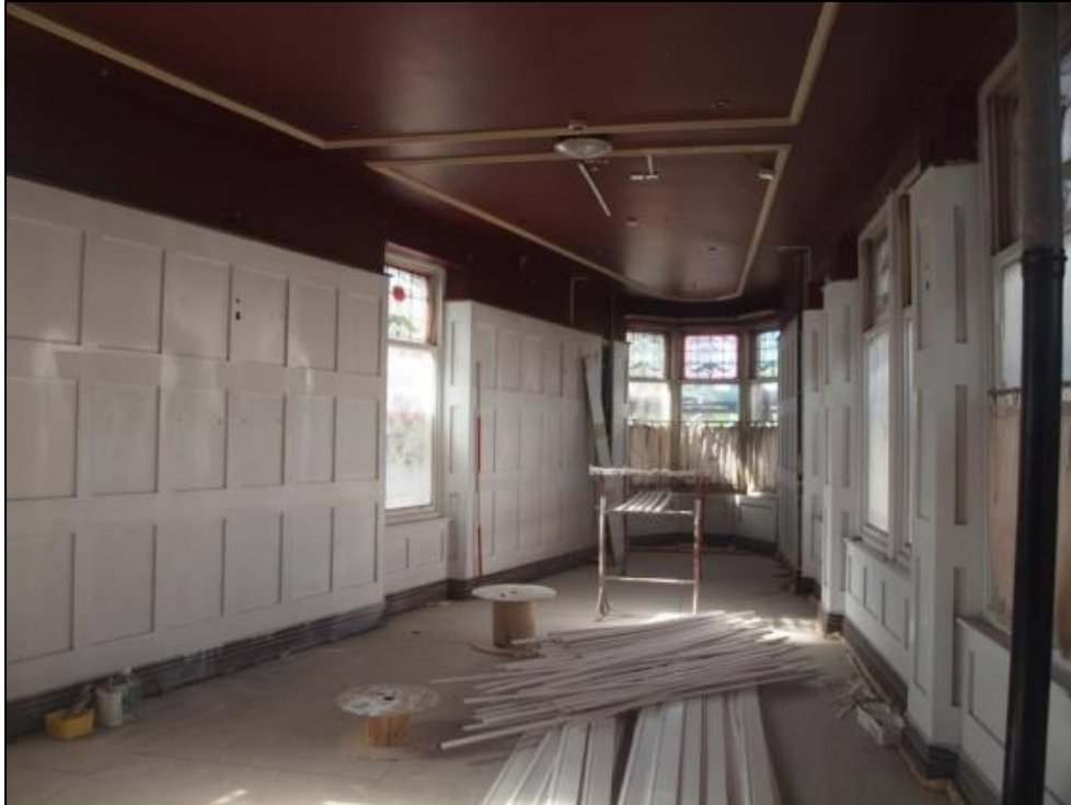
Plate 7: Ground floor room 1
