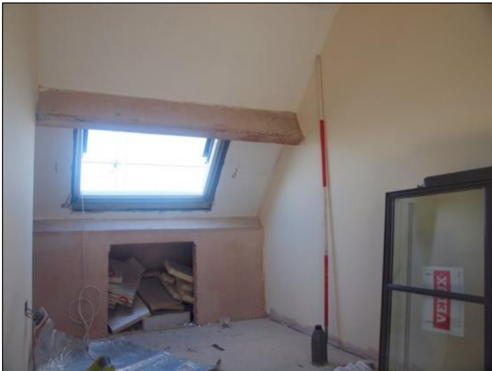
Plate 72: Converted attic space showing purlins
