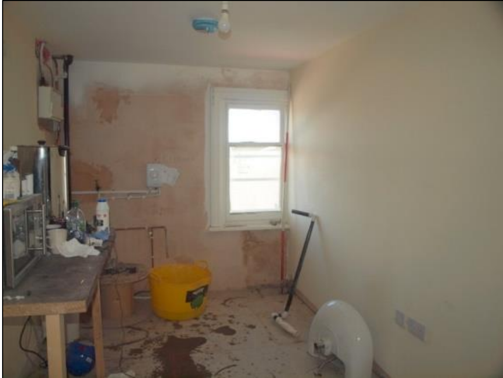
Plate 55: Second floor room showing window cut by inserted wall
