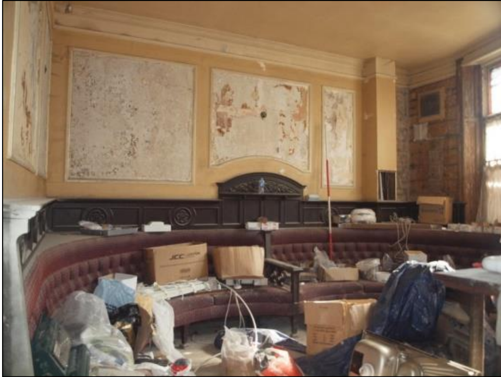
Plate 17: Ground floor room 4
