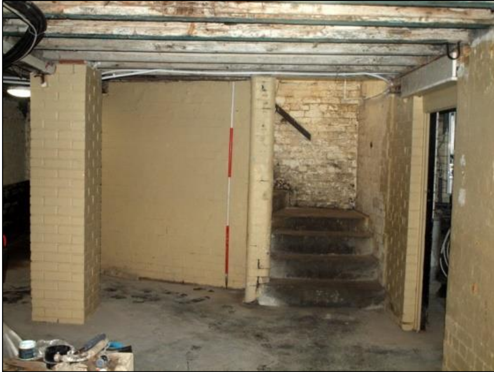
Plate 83: Basement room 4 southern end showing main staircase
