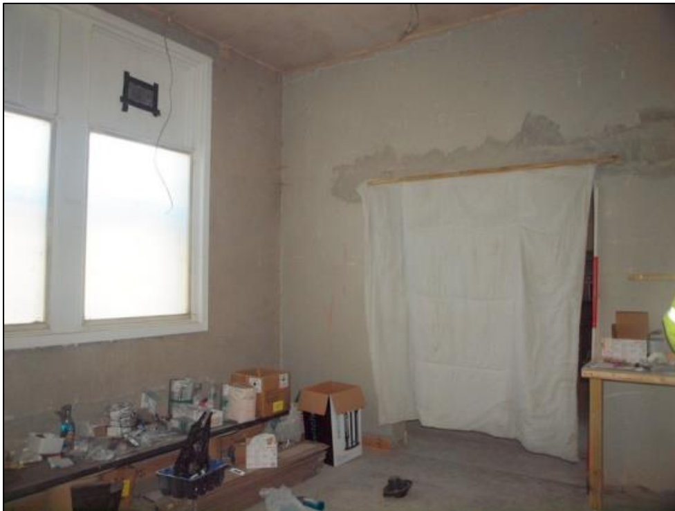
Plate 22: Ground floor room 6
