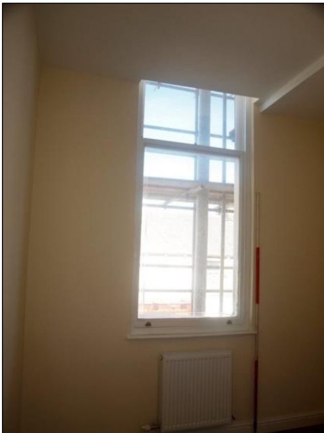
Plate 30: First floor window
