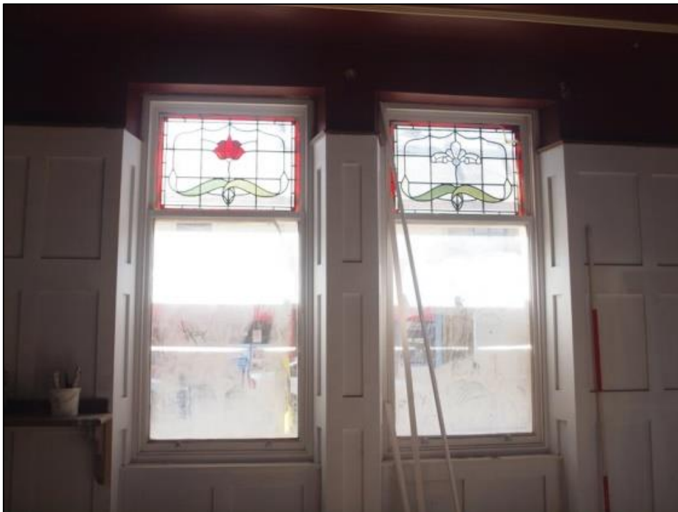
Plate 10: Ground floor room 1 windows
