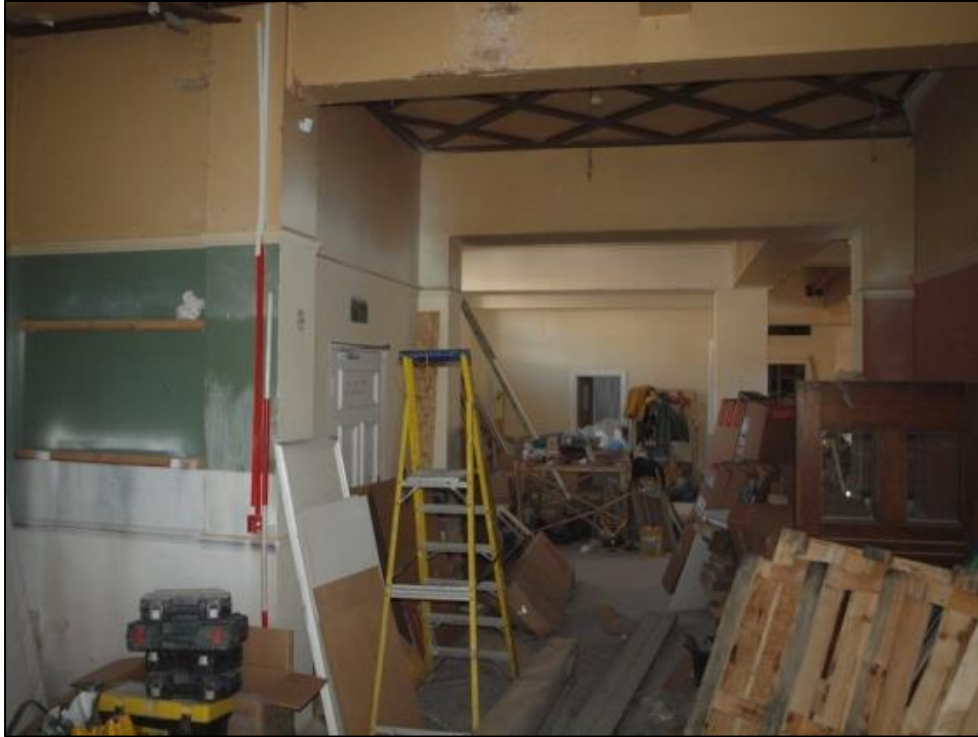
Plate 11: Ground floor room 2
