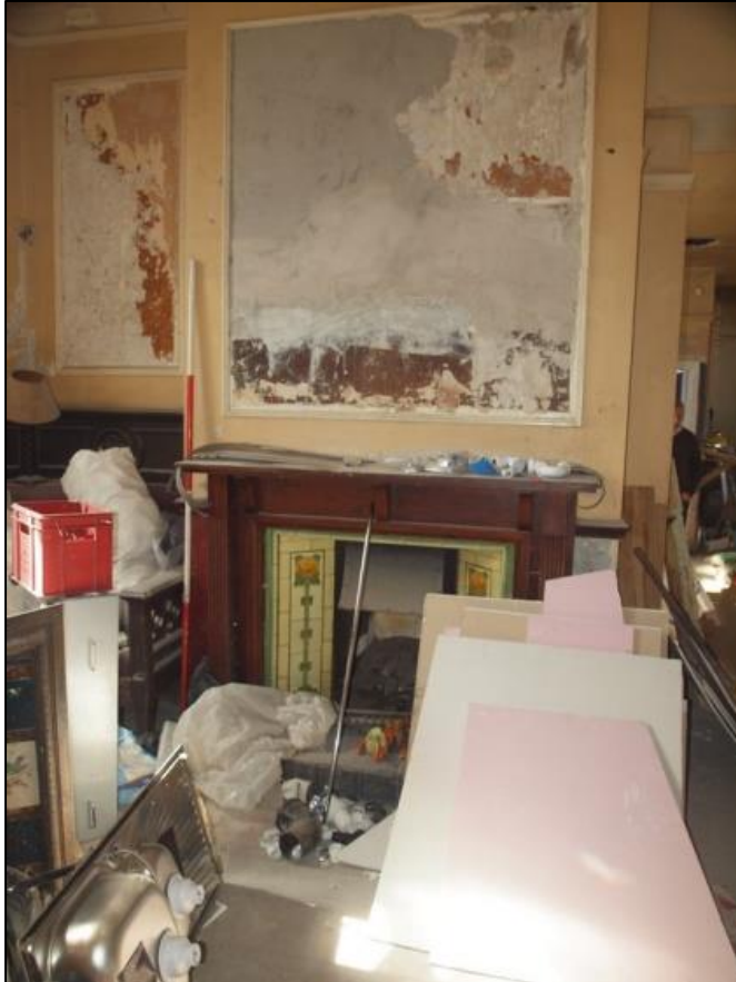
Plate 19: Ground floor room 4 fireplace
