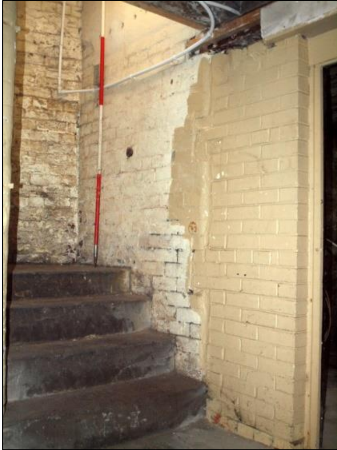
Plate 85: Basement room 4 main staircase
