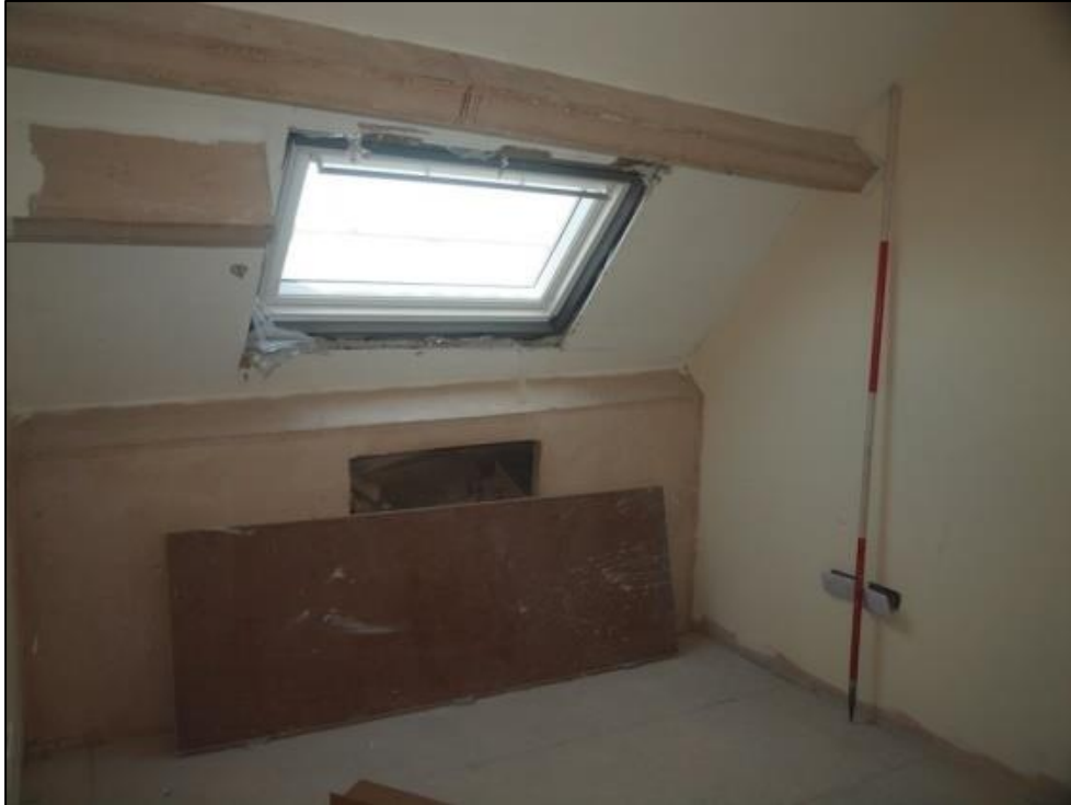
Plate 73: Converted attic space showing purlins
