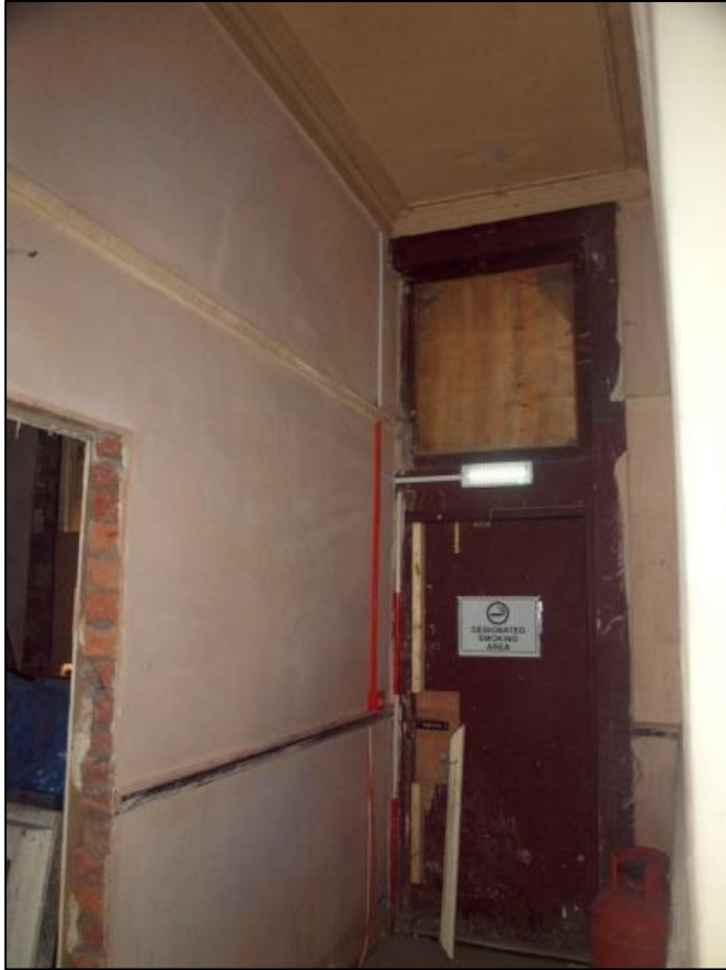
Plate 21: Ground floor room 5
