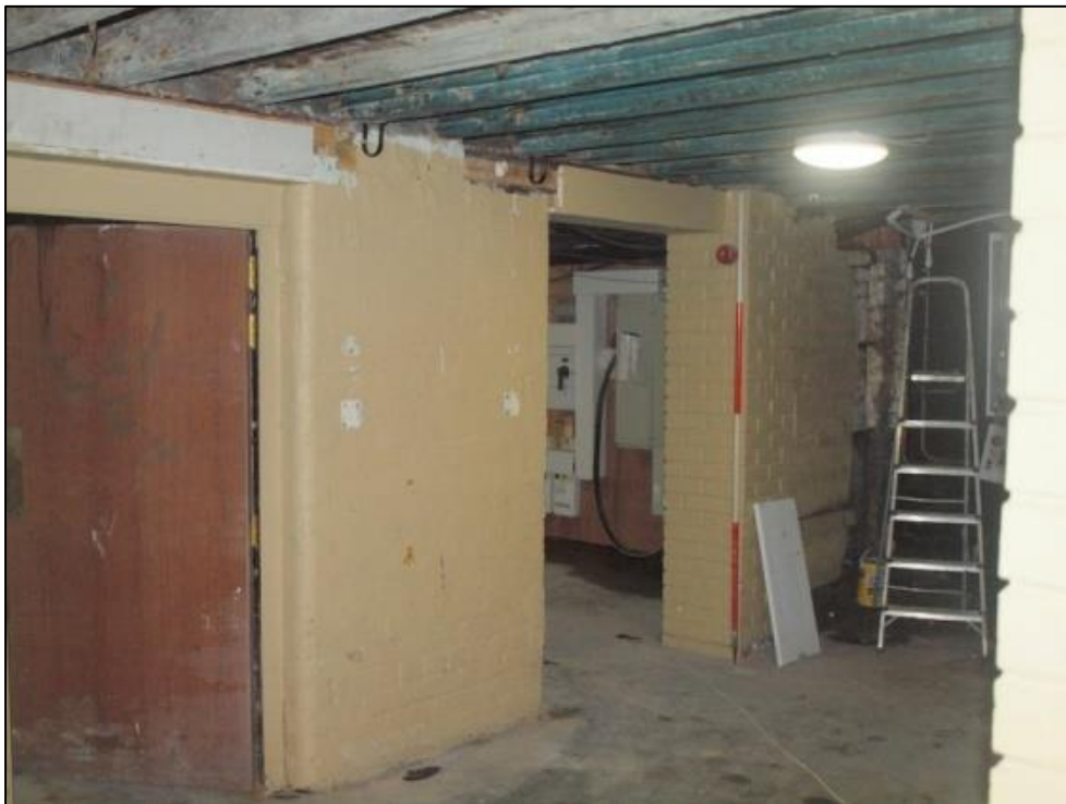
Plate 84: Basement room 4 southern end
