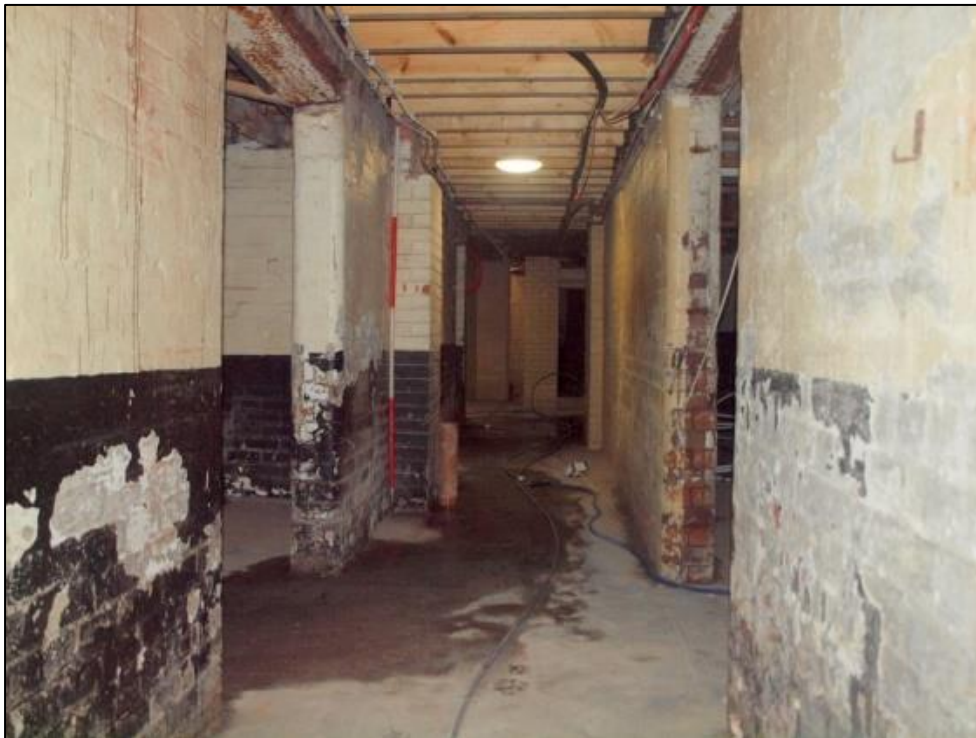
Plate 86: Basement room 4 northern end
