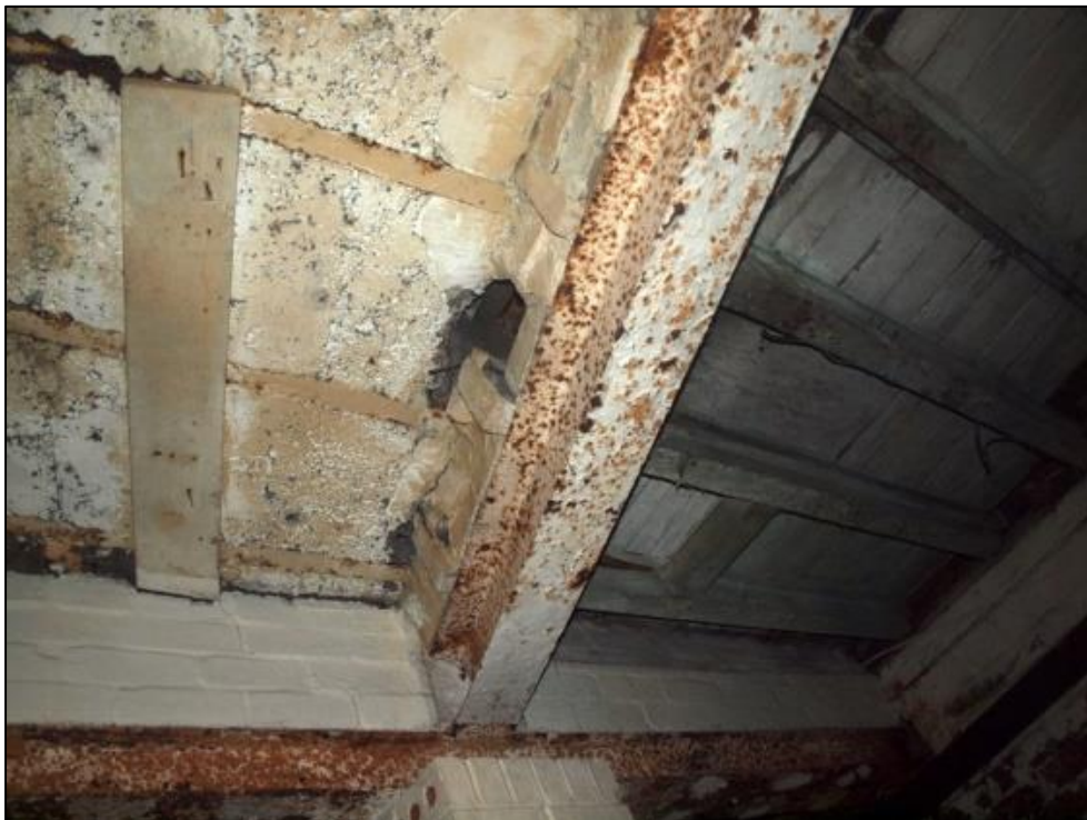
Plate 76: Ceiling of basement room 1
