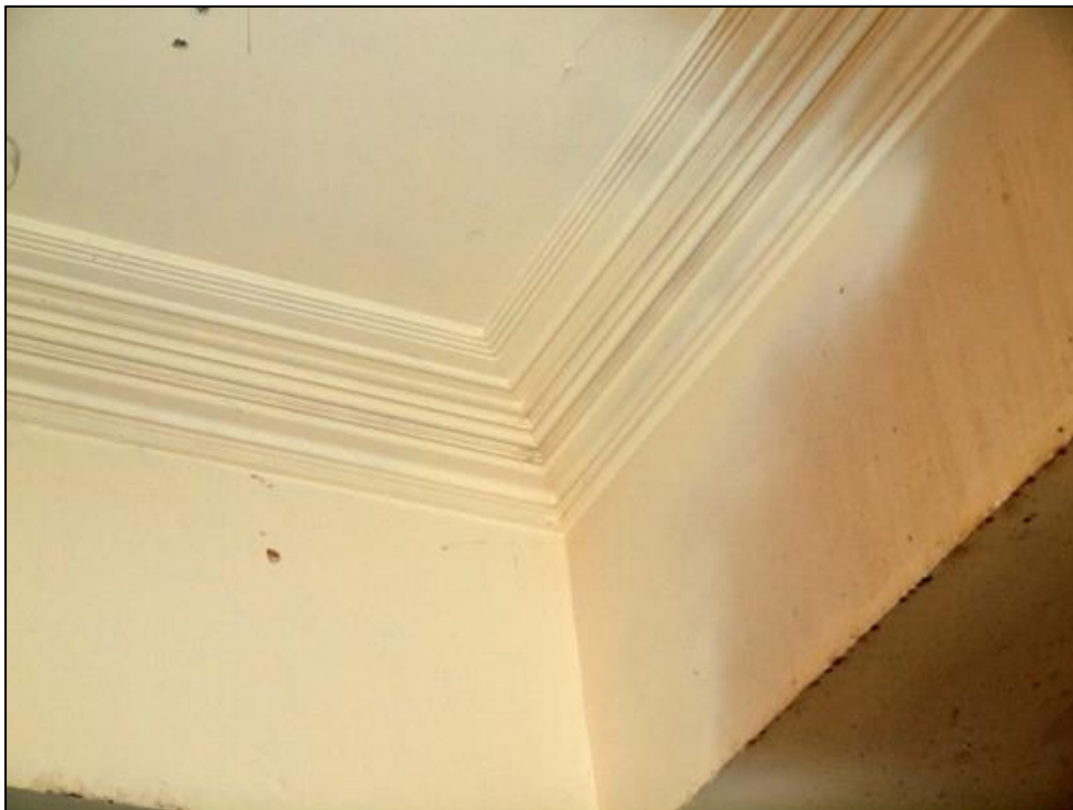
Plate 14: Detail of cornice C1
