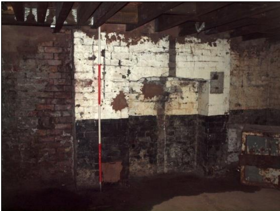
Plate 96: Basement room 9 detail
