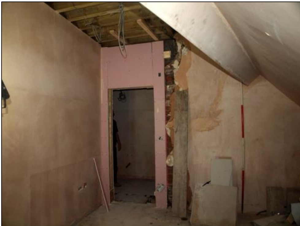
Plate 68: Converted attic space
