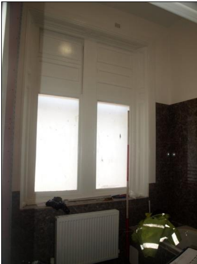
Plate 32: First floor room
