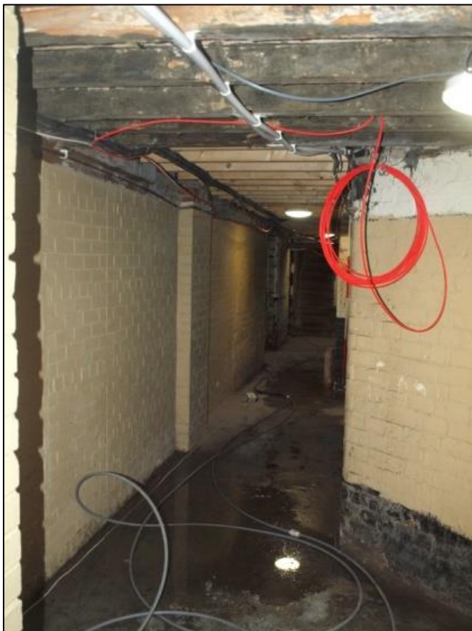
Plate 82: Basement room 4 southern end
