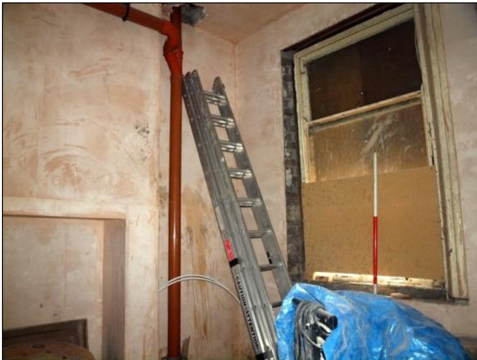
Plate 24: Ground floor room 7
