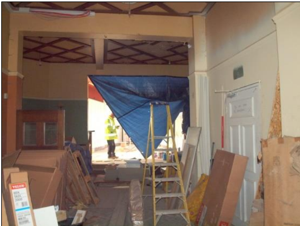
Plate 12: Ground floor room 2
