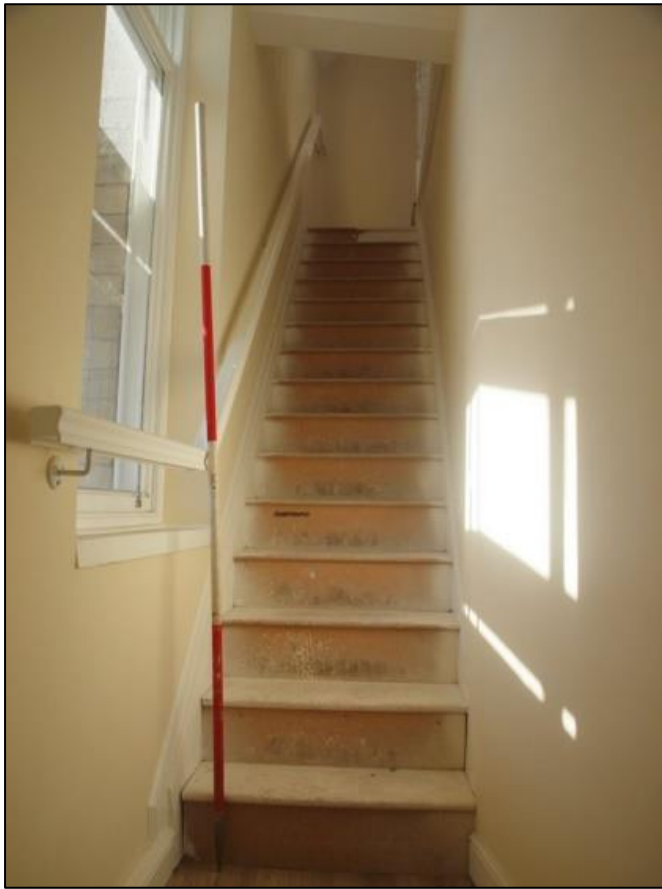
Plate 47: Staircase at southern end to second floor
