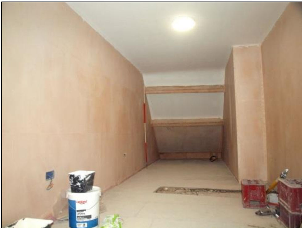
Plate 66: Converted attic space
