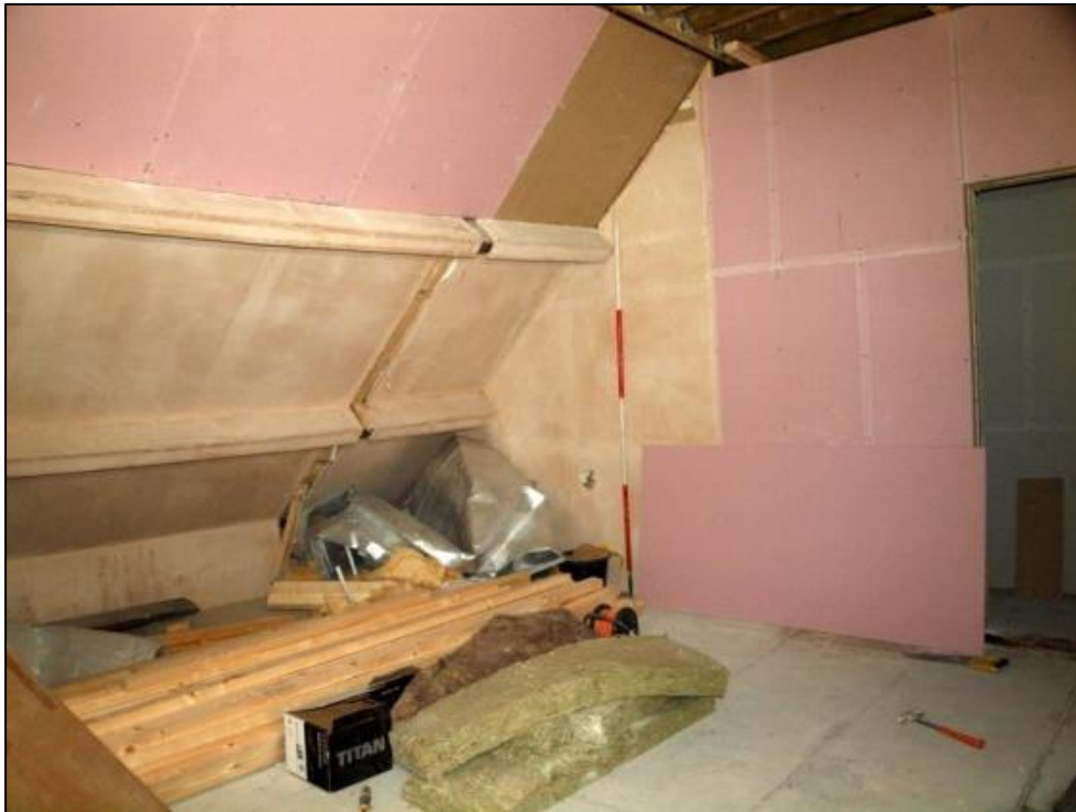
Plate 69: Converted attic space showing purlins
