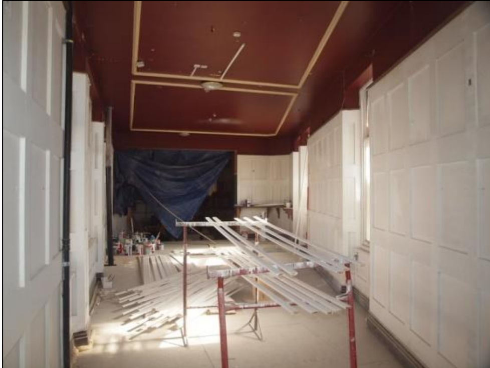
Plate 9: Ground floor room 1
