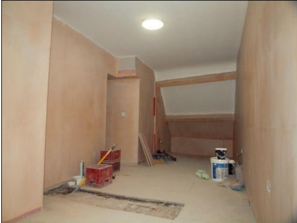
Plate 67: Converted attic space
