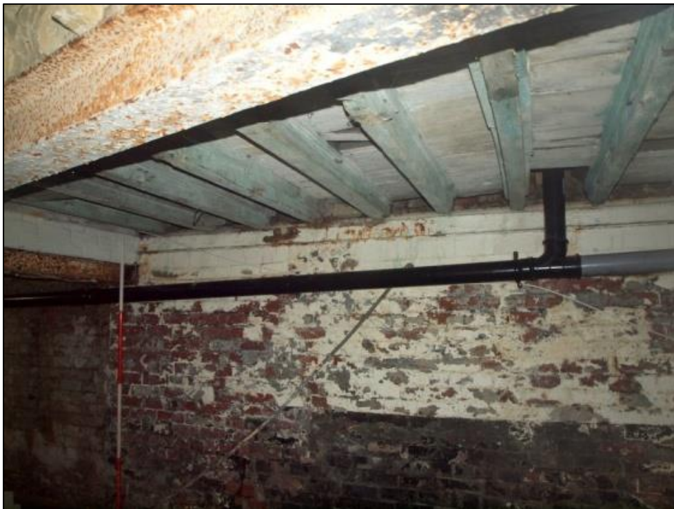
Plate 78: Blocked openings in basement room 1
