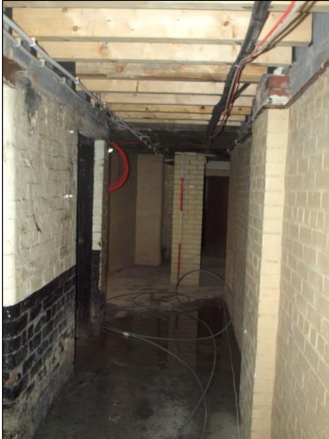
Plate 81: Basement room 4 southern end
