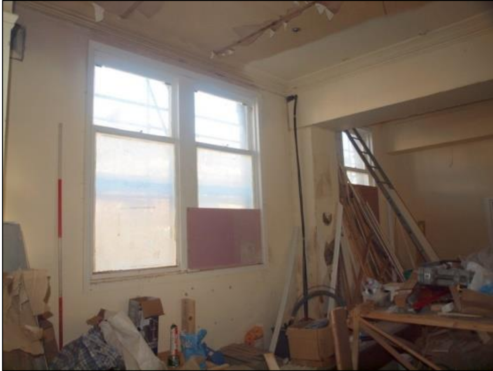
Plate 15: Ground floor room 2
