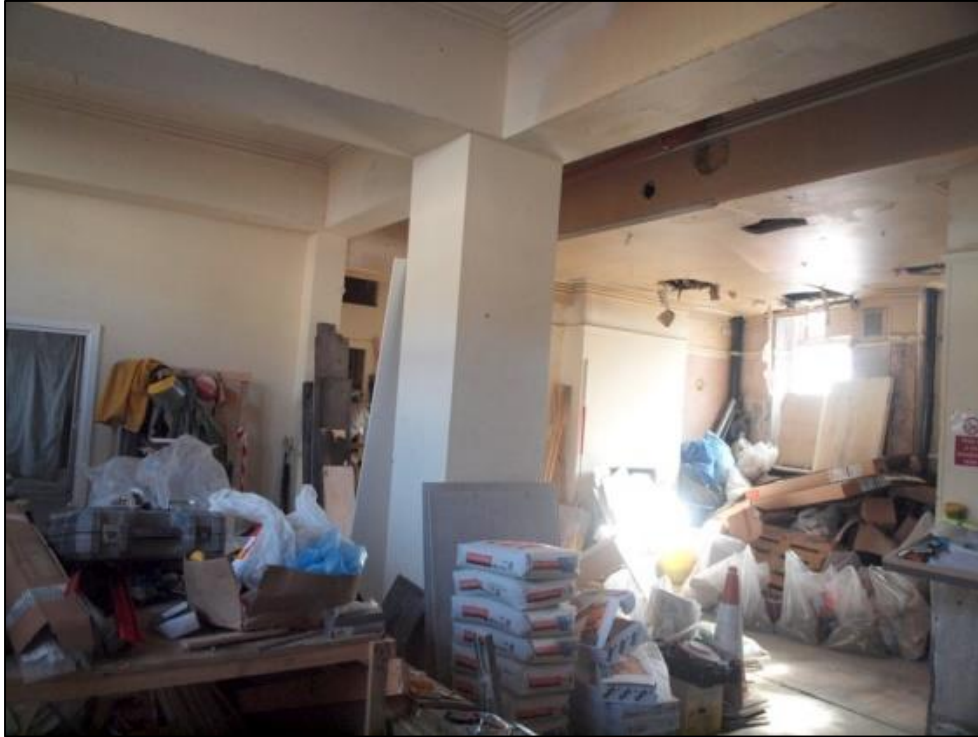
Plate 13: Ground floor room 2
