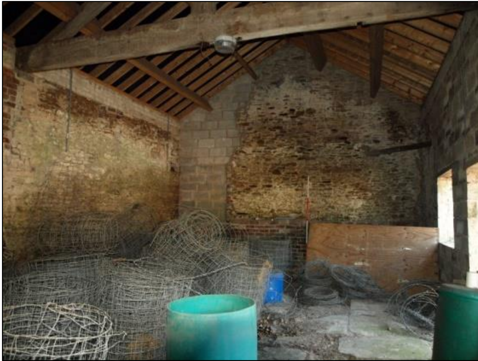
Plate 45: Room 2 showing blocked openings
