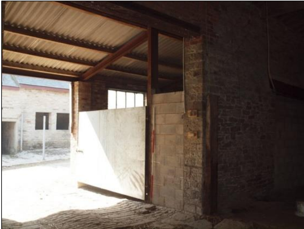
Plate 27: Passageway showing entrance southern lean-to room
