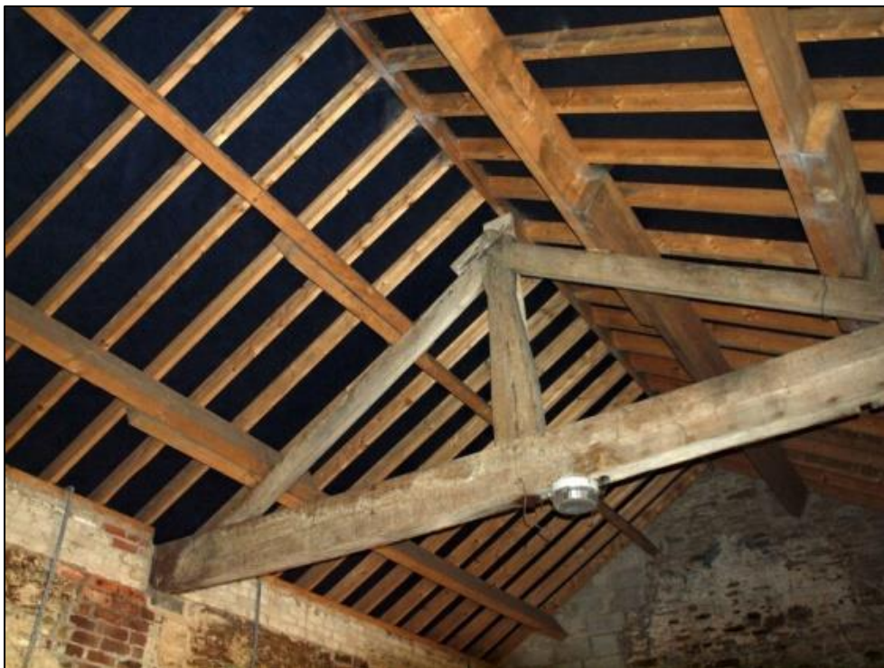
Plate 46: King post truss in room 2
