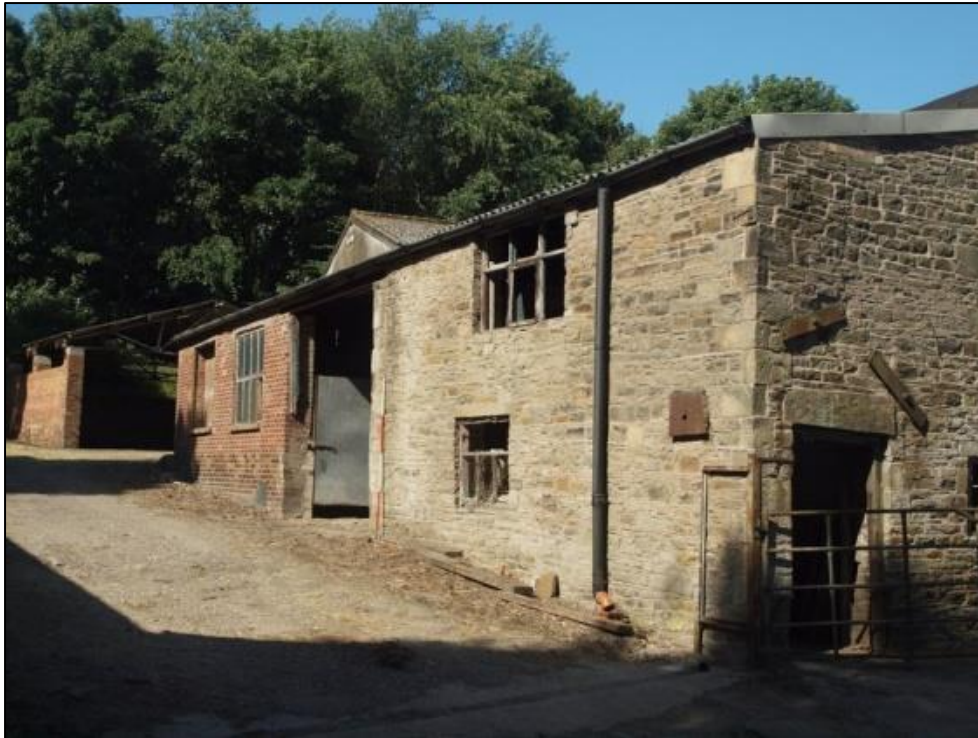
Plate 7: Southeast elevation from east
