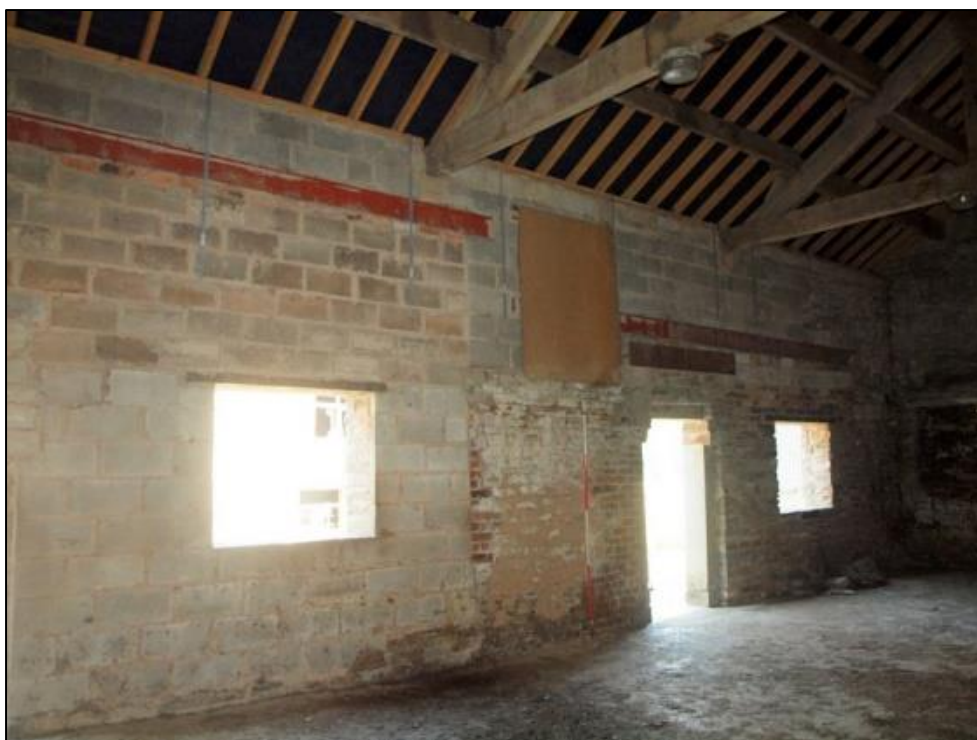
Plate 43: Room 1 interior showing rebuilt northwest wall
