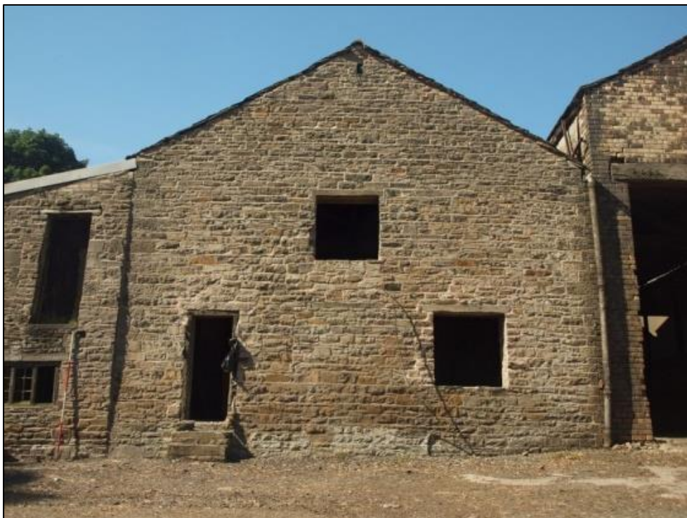
Plate 6: Barn northeast elevation
