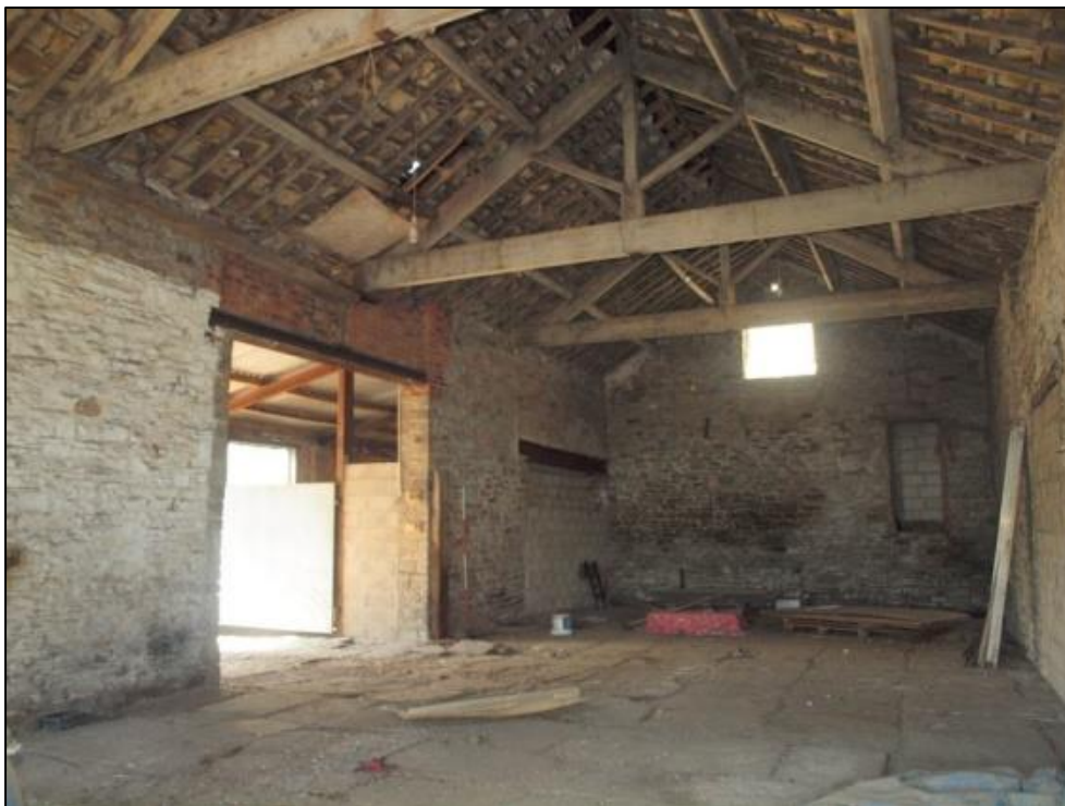
Plate 18: Barn interior showing barn door to passage
