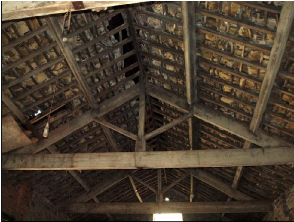
Plate 21: Detail of king post truss
