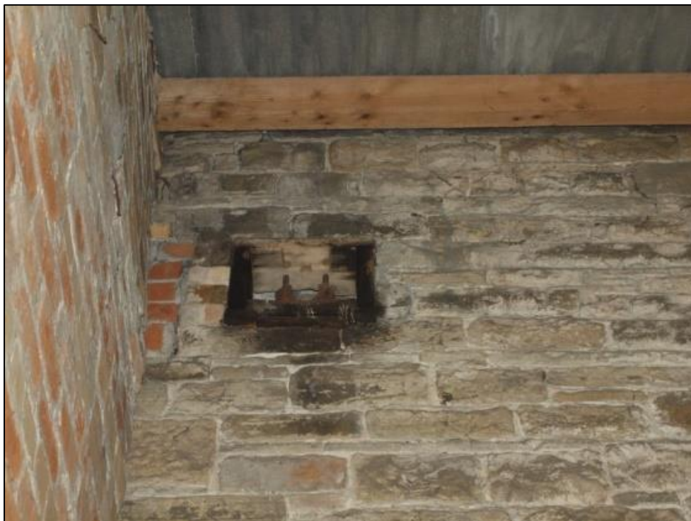
Plate 25 : Transmission window in eastern lean-to room
