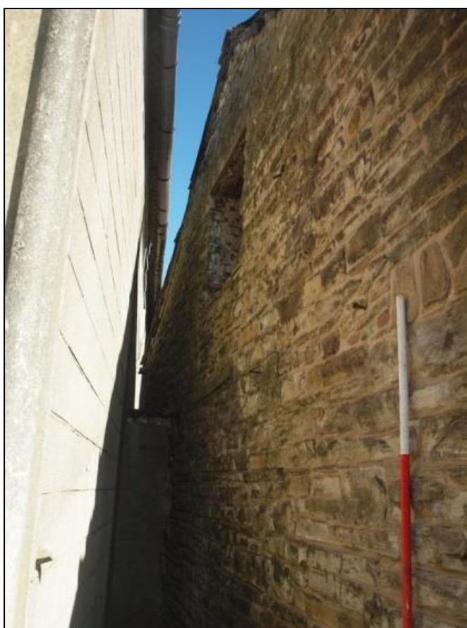
Plate 10: Detail of window in southwest elevation of barn
