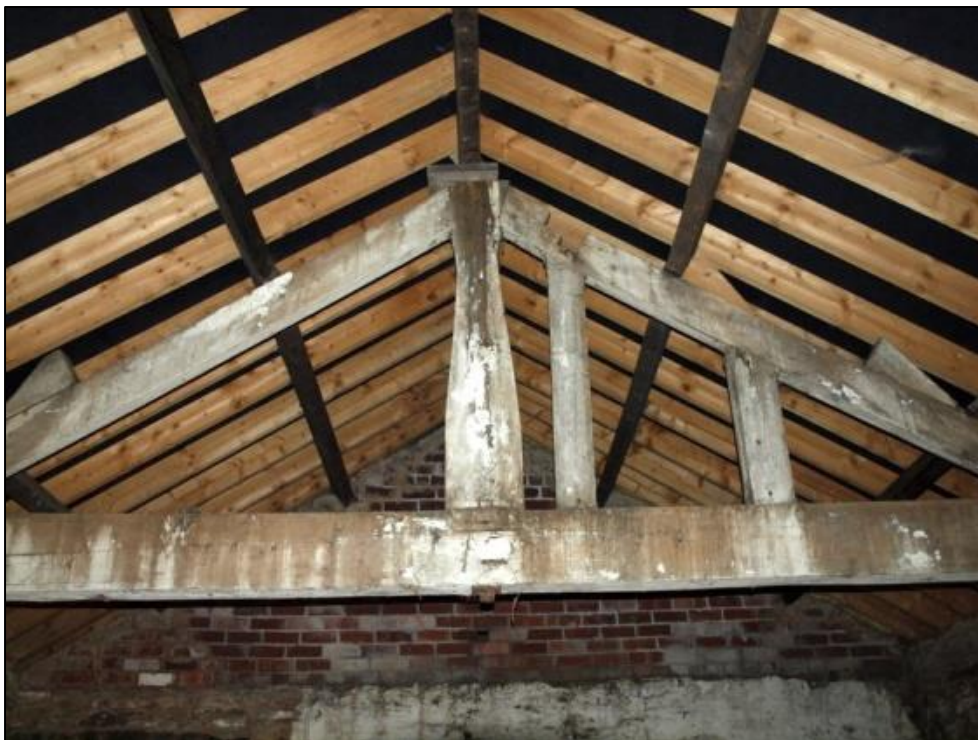
Plate 52: King post truss in room 4
