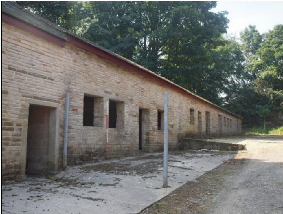
Plate 33: Northwest elevation, looking west
