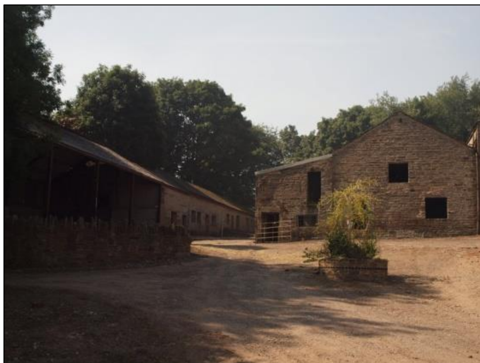
Plate 1: General shot of Barn 1 (right) and Barn 2 (left)
