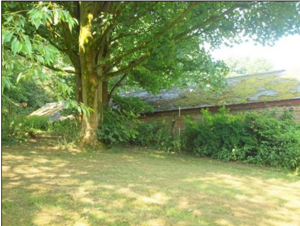
Plate 37: Southwest elevation west end
