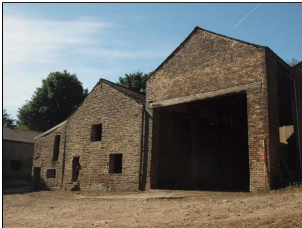
Plate 2: Barn 1 northeast elevation
