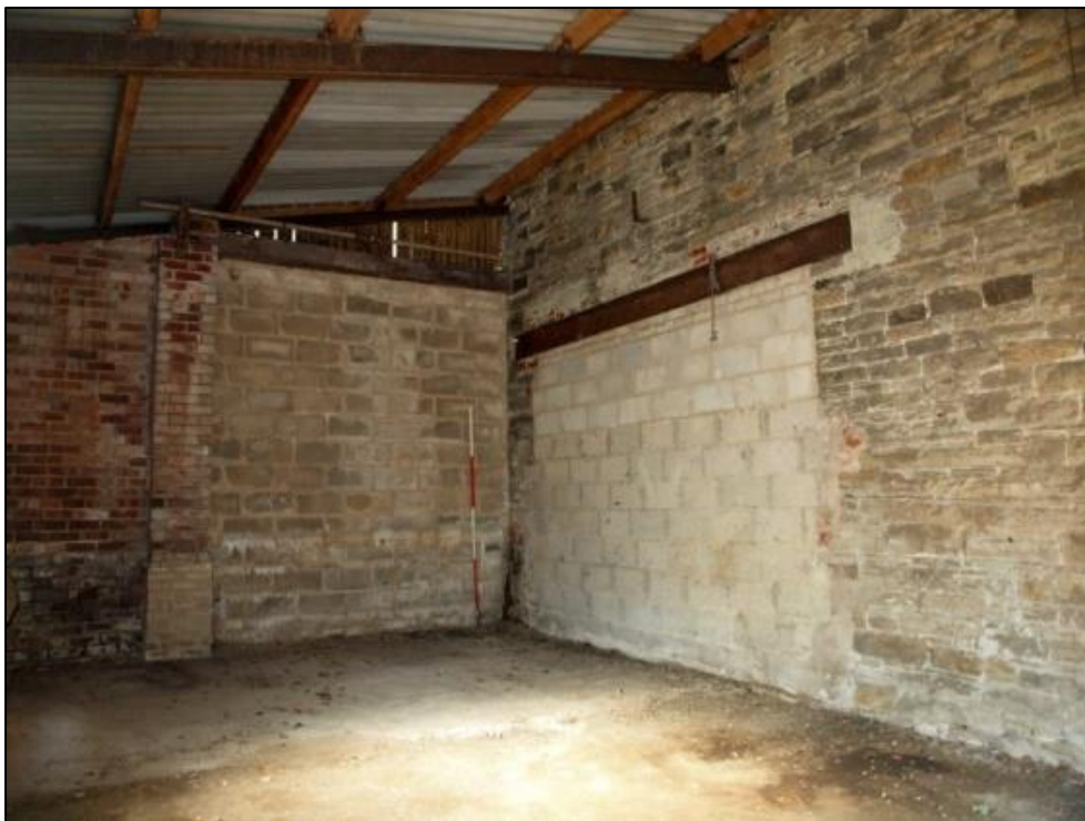
Plate 28: Southern lean-to room
