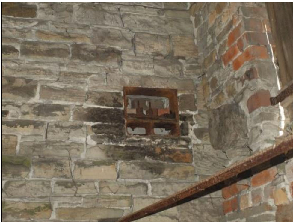
Plate 24: Transmission window in eastern lean-to room
