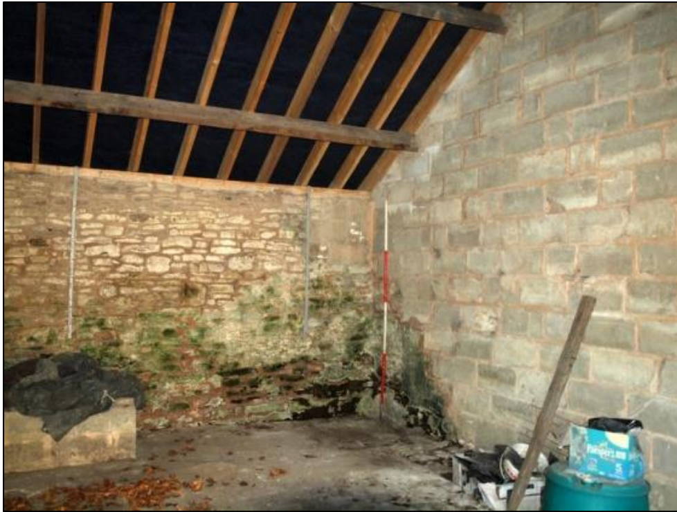
Plate 55:Room 5 showing rebuilt gable wall
