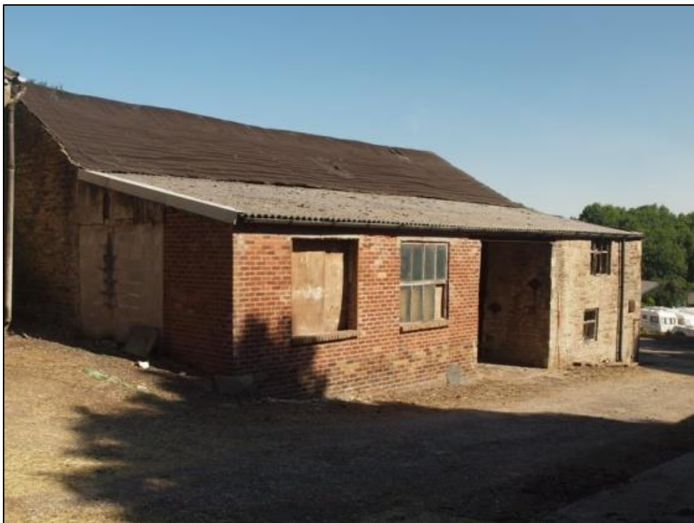
Plate 8: Southeast elevation from south
