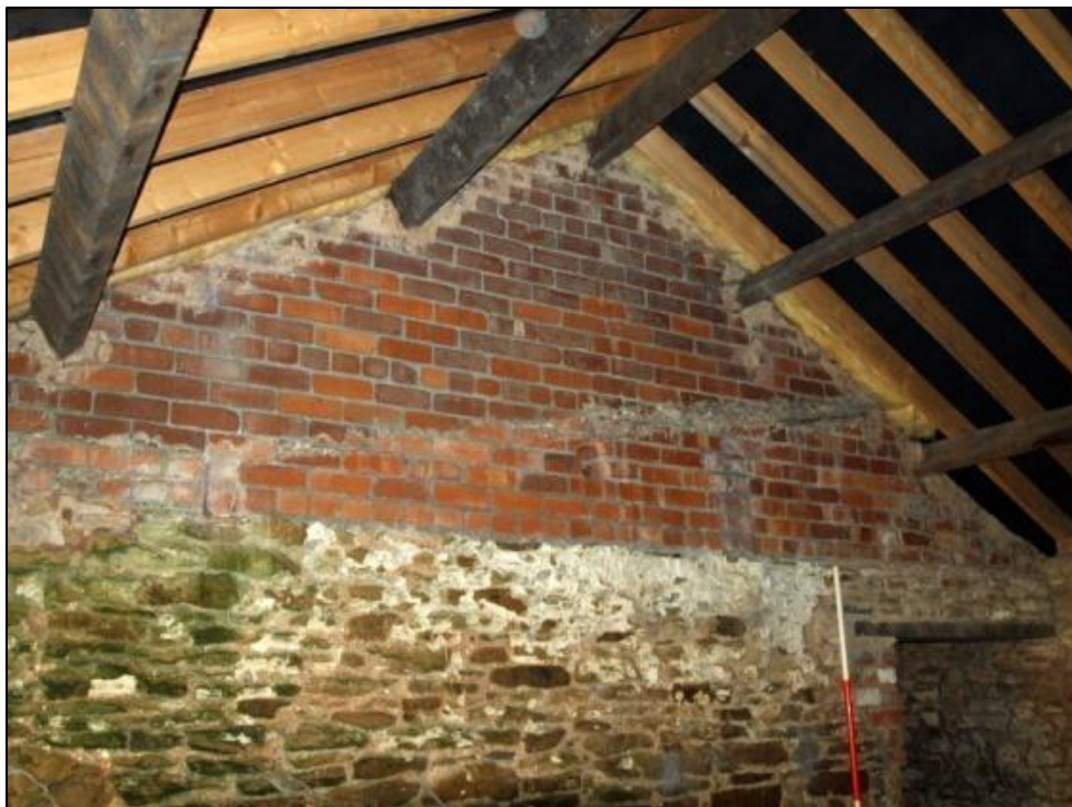
Plate 54: Detail of ghost of roof line
