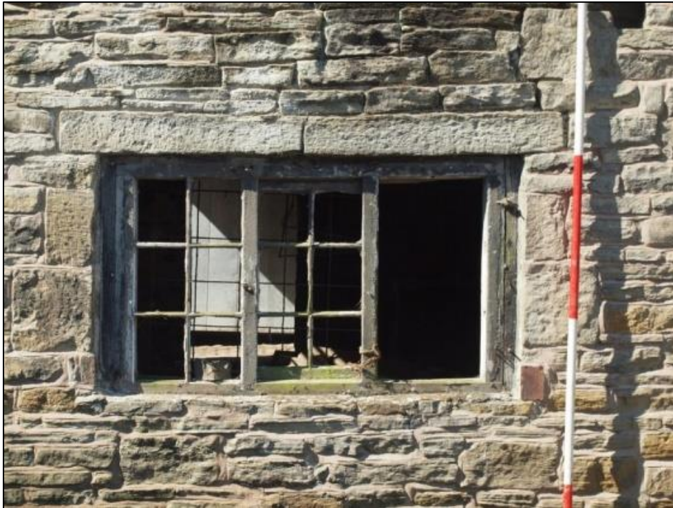
Plate 5: Lean-to window detail
