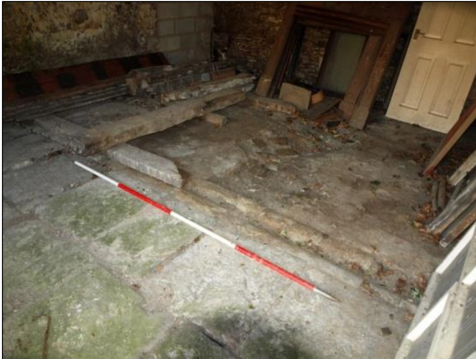
Plate 49: Detail of drains in floor of room 3
