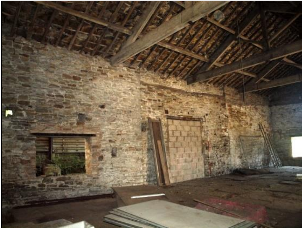
Plate 17: As above also showing inserted window
