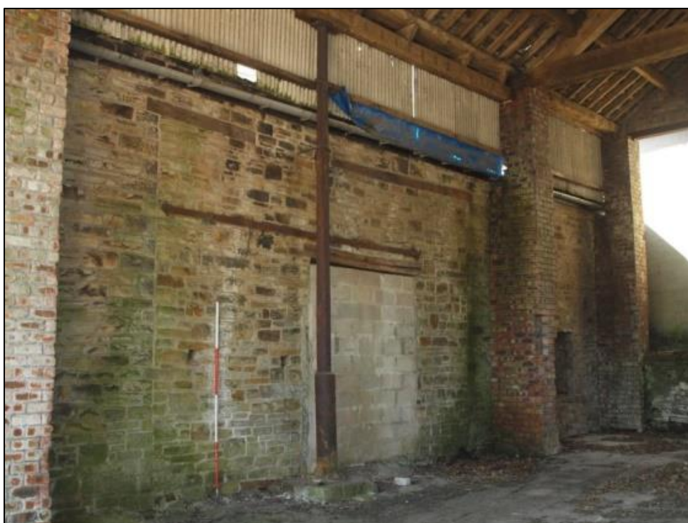
Plate 12: Interior of Dutch barn showing blocked loading door within blocked barn door of barn
