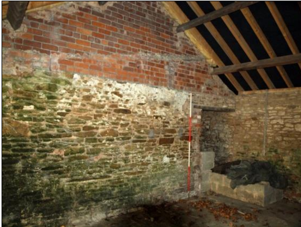
Plate 53: Room 5 showing rebuilt party wall
