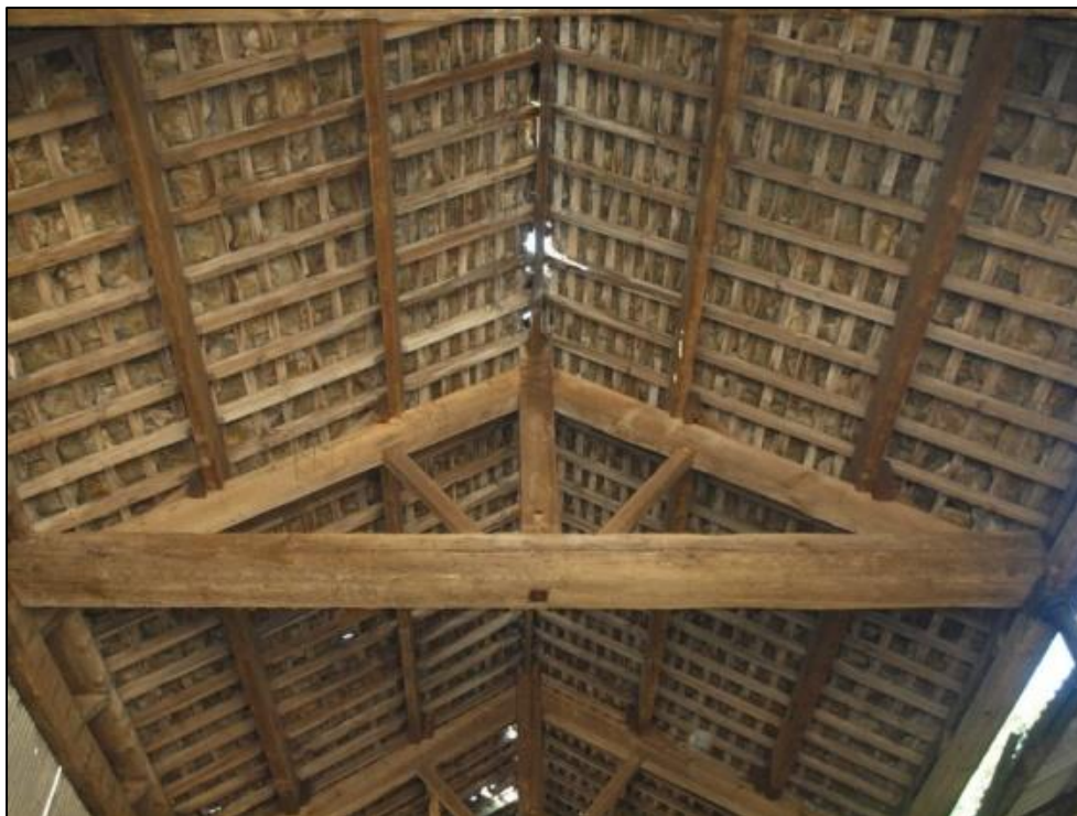
Plate 15: King post truss of Dutch barn
