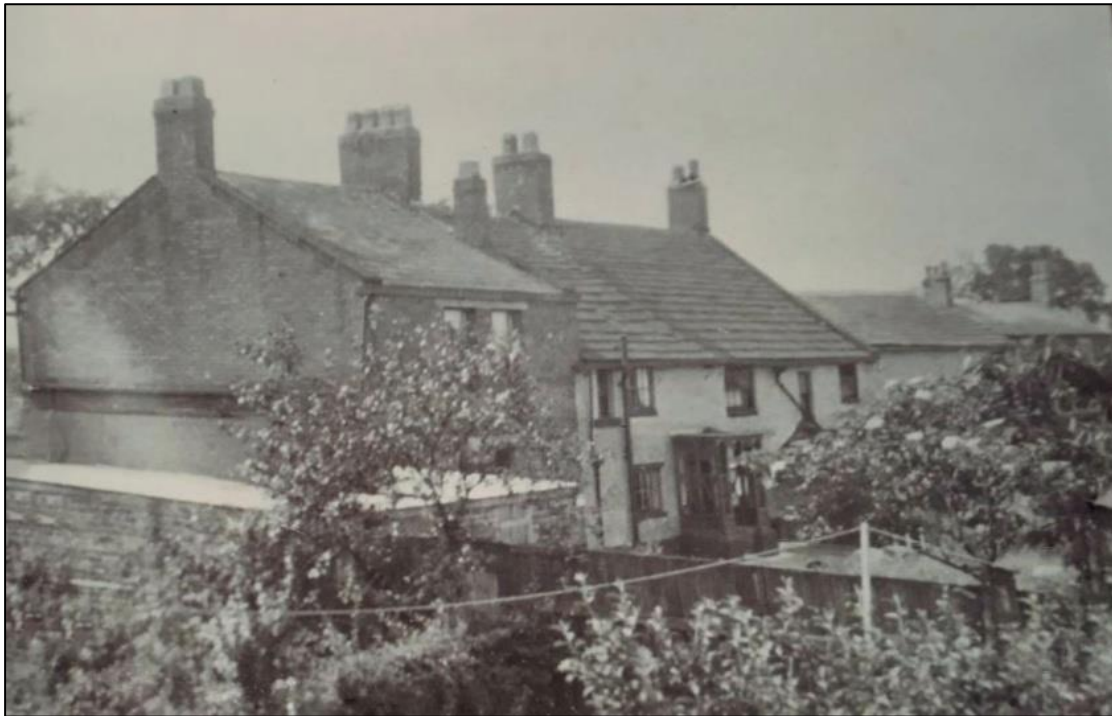
Figure 15: Rear of the Inn before the alterations of 1937
