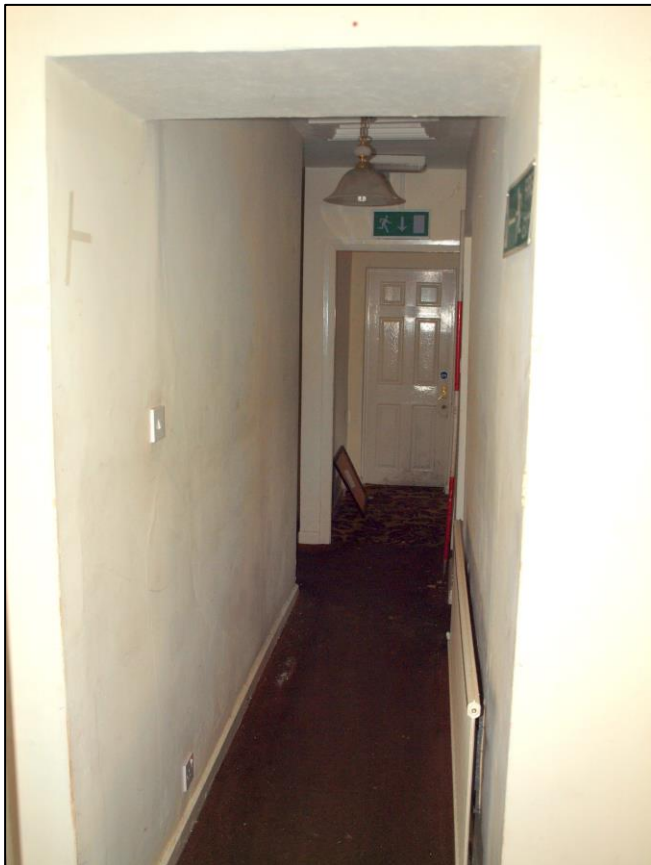
Plate 30: First floor corridor
