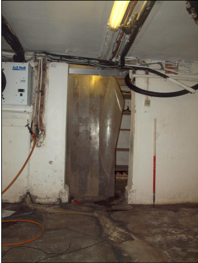
Plate 51: Doorway to storage area
