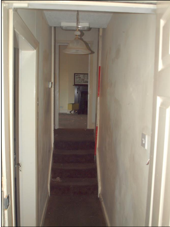
Plate 31: First floor corridor showing stairs to bay 4
