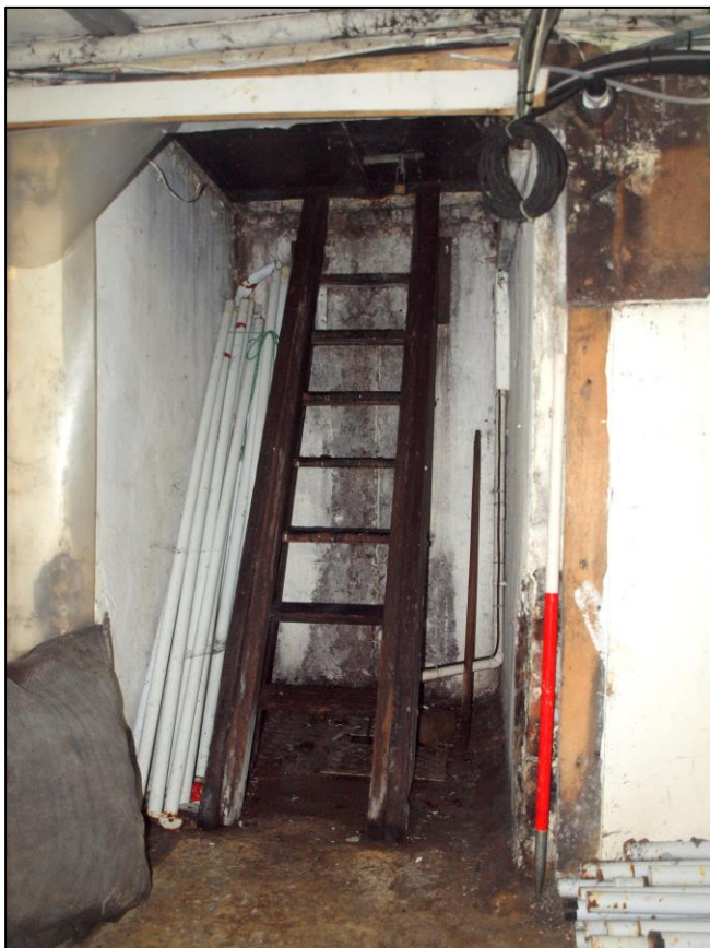
Plate 50: Ladders to hatch
