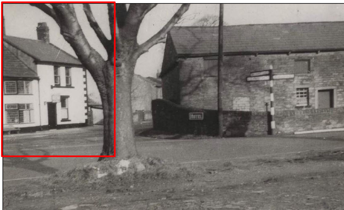
Figure 16: Myerscough farm, with the Inn to the left. Note the bay windows are present
