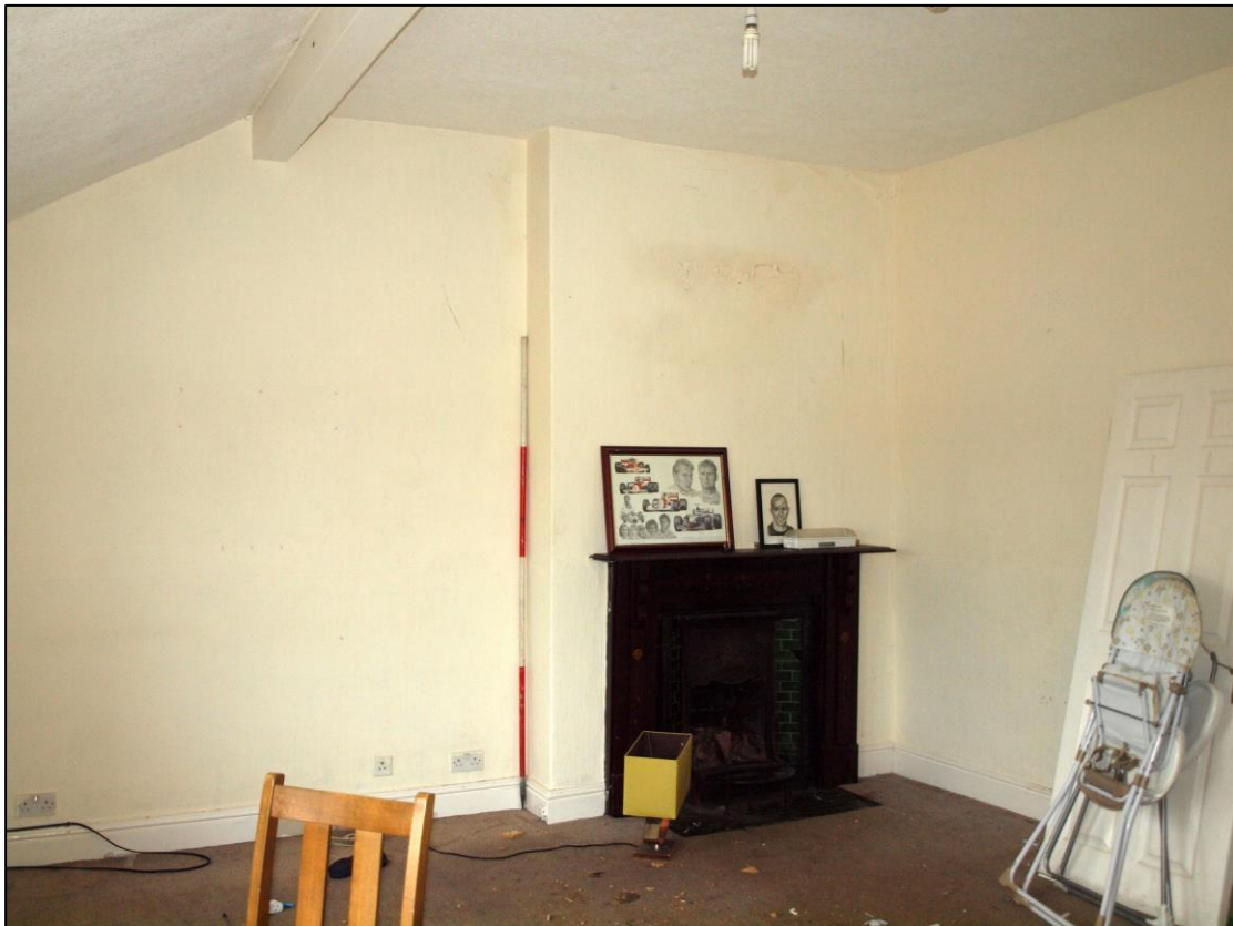
Plate 42: Bay 4 northwest bedroom
