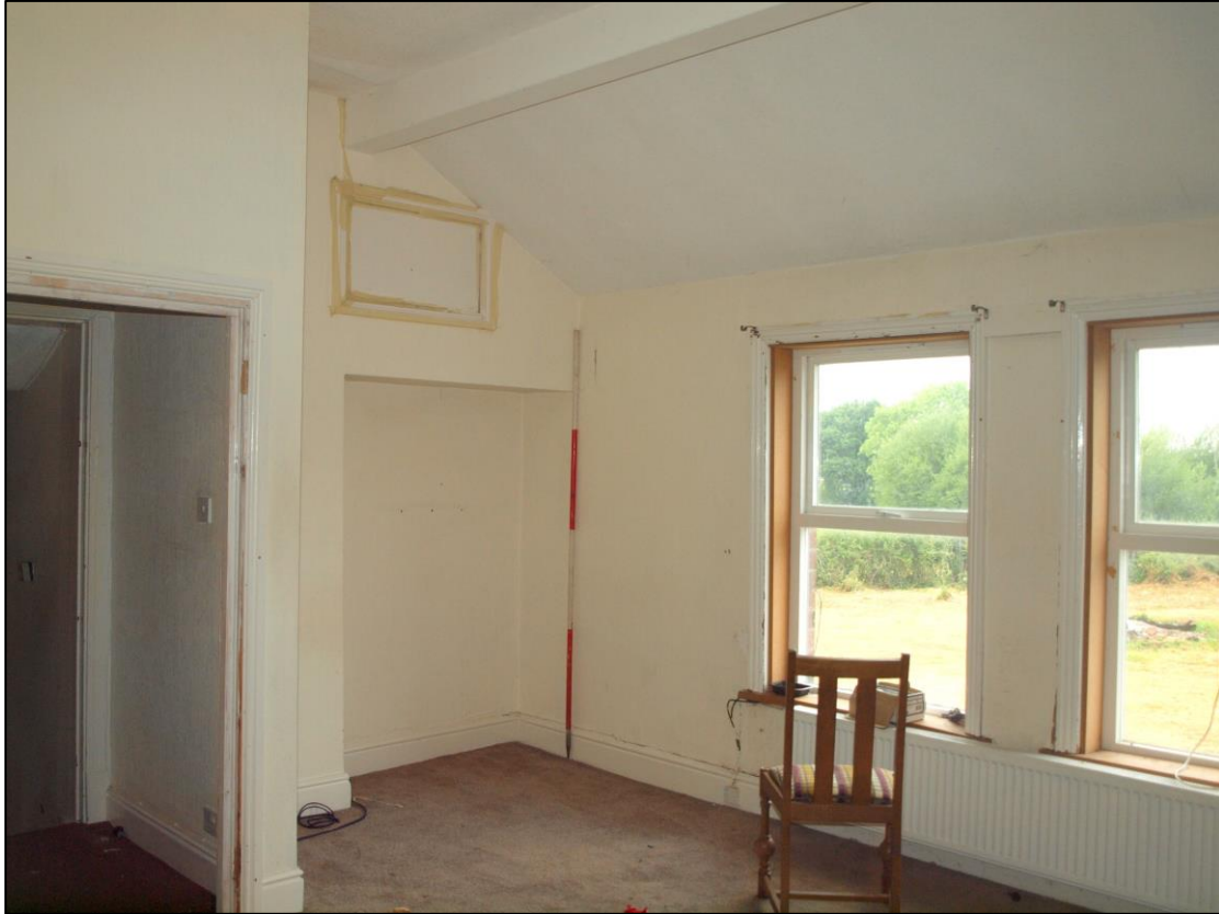
Plate 43: Bay 4 northwest bedroom
