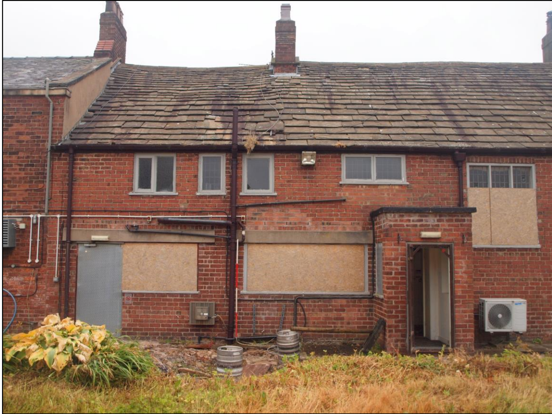
Plate 9: Northwest elevation detail
