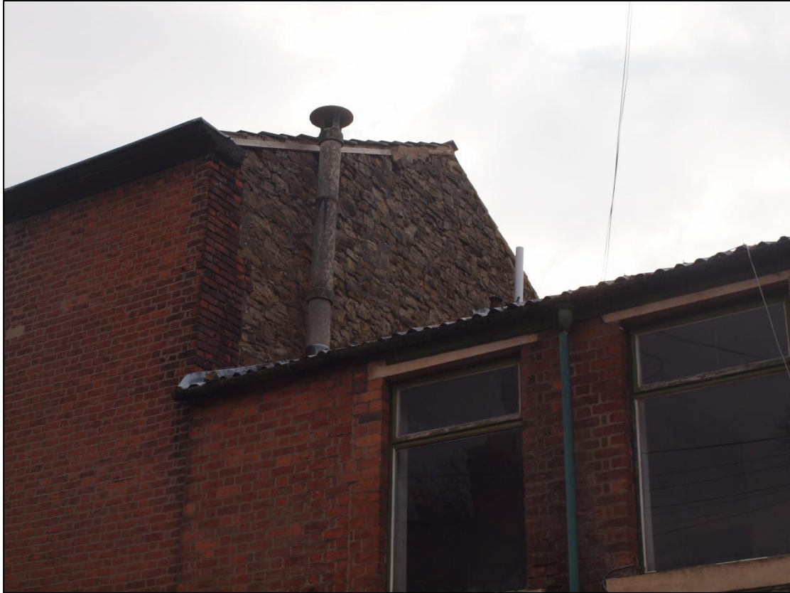
Plate 3: First floor of number 5 showing gable of adjacent building
