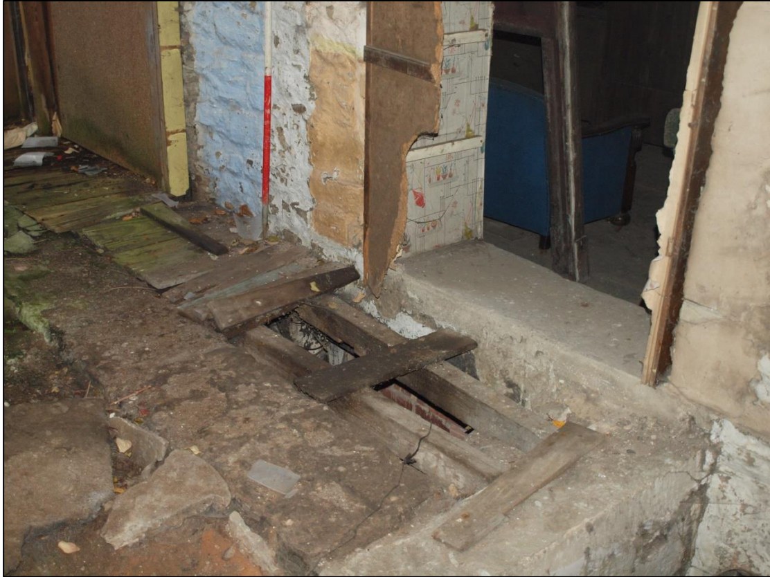
Plate 31: Top of cellar lights in rear yard
