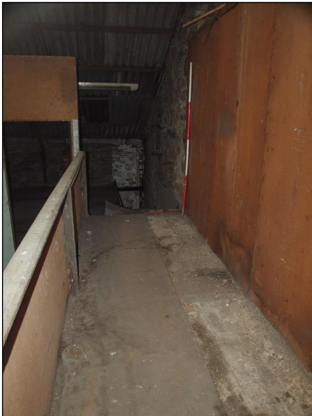
Plate 66: Walkway at first floor level
