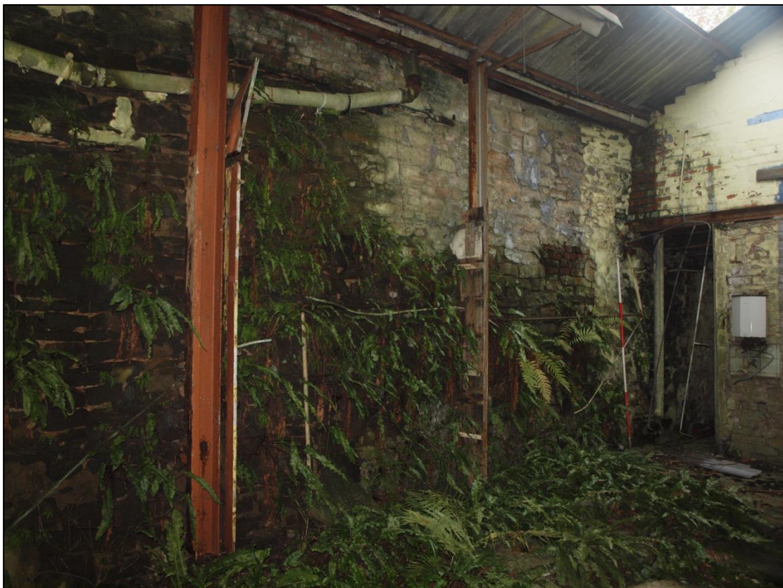
Plate 30: Southern wall of rear yard
