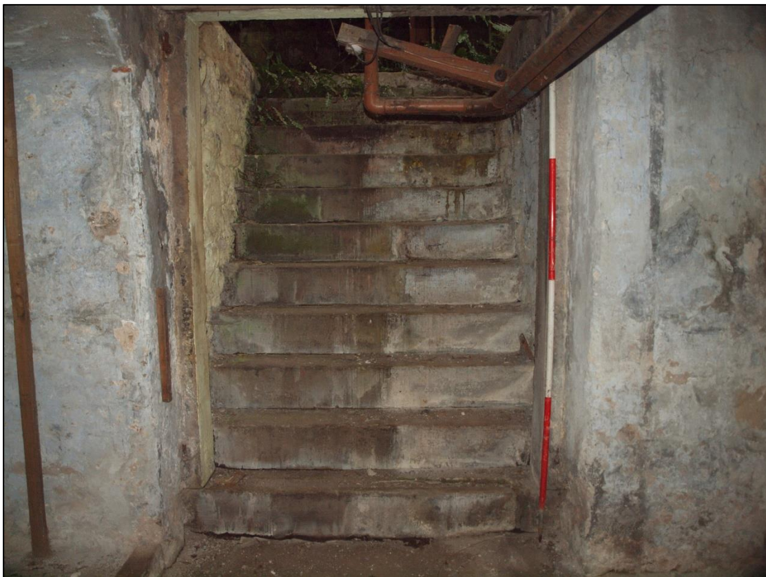
Plate 52: Concrete cellar steps
