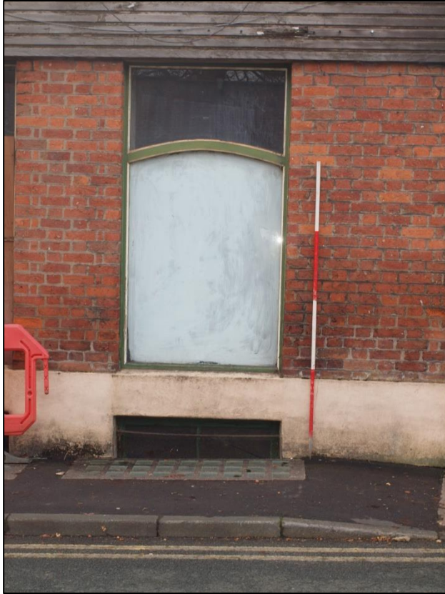
Plate 7: Detail of ground floor window 5 Queens Road
