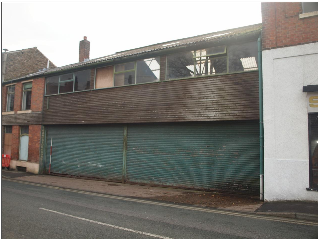
Plate 12: North elevation of 7 - 9 Queens Road
