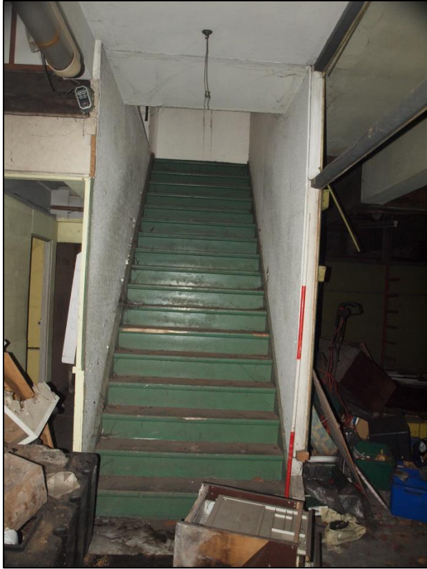
Plate 33: Large steps to first floor in number 7-9
