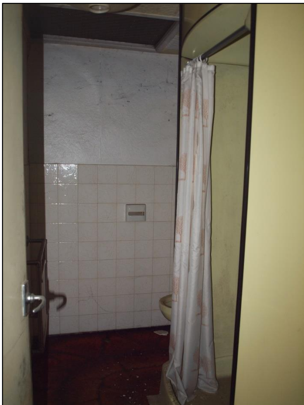
Plate 62: Bathroom at north end of number 5 first floor
