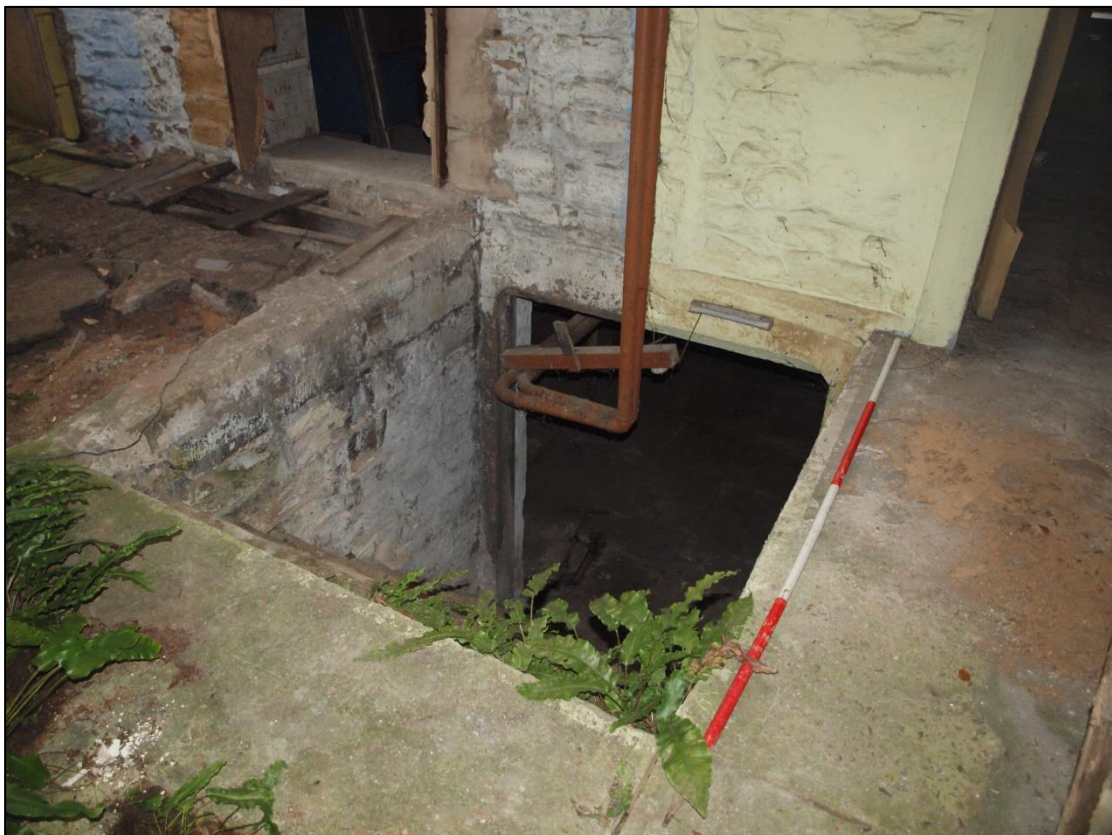
Plate 26: Inserted staircase to cellar in rear yard
