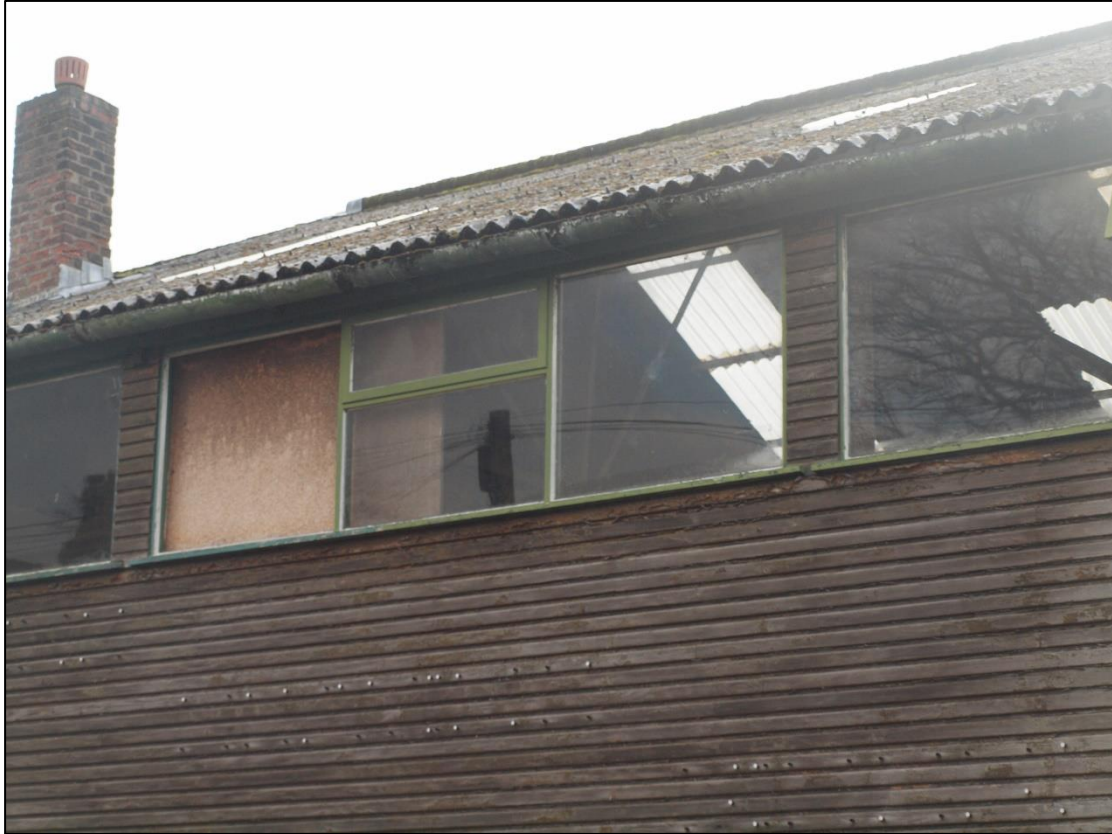
Plate 13: Detail of first floor windows of 7 - 9 Queens Road
