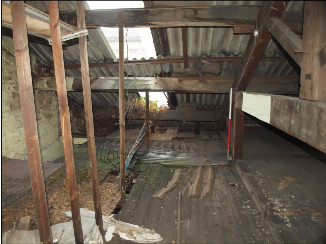
Plate 73: General shot of attic
