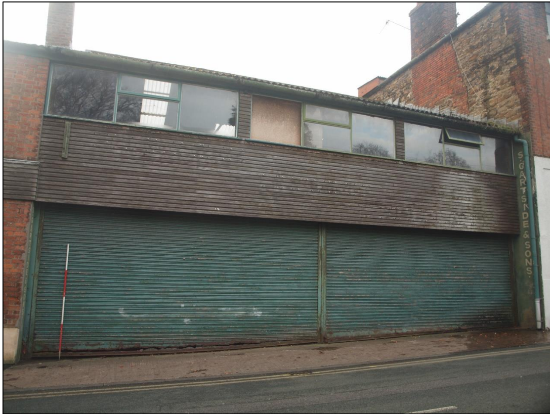
Plate 11: North elevation of 7 - 9 Queens Road
