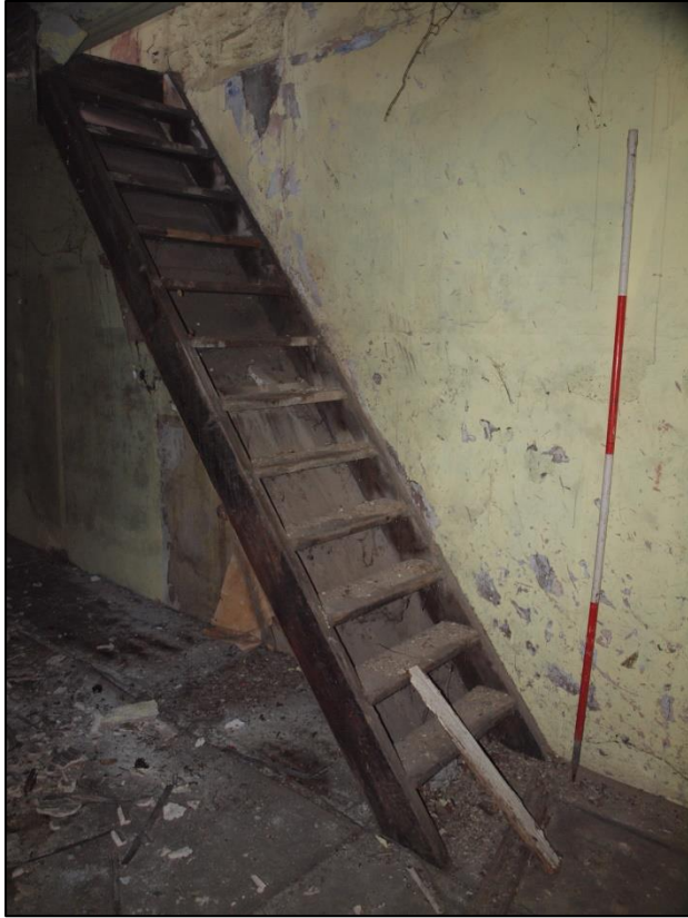
Plate 55: Staircase to attic
