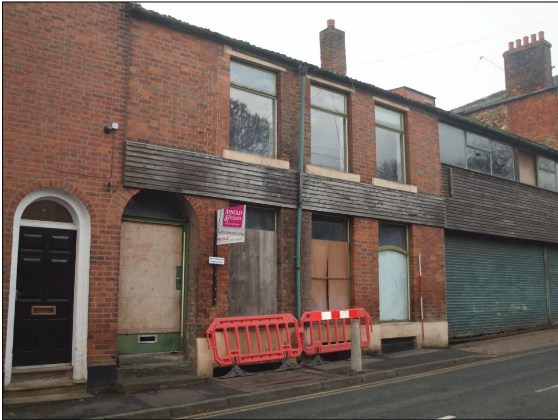
Plate 5: North elevation of 5 Queens Road
