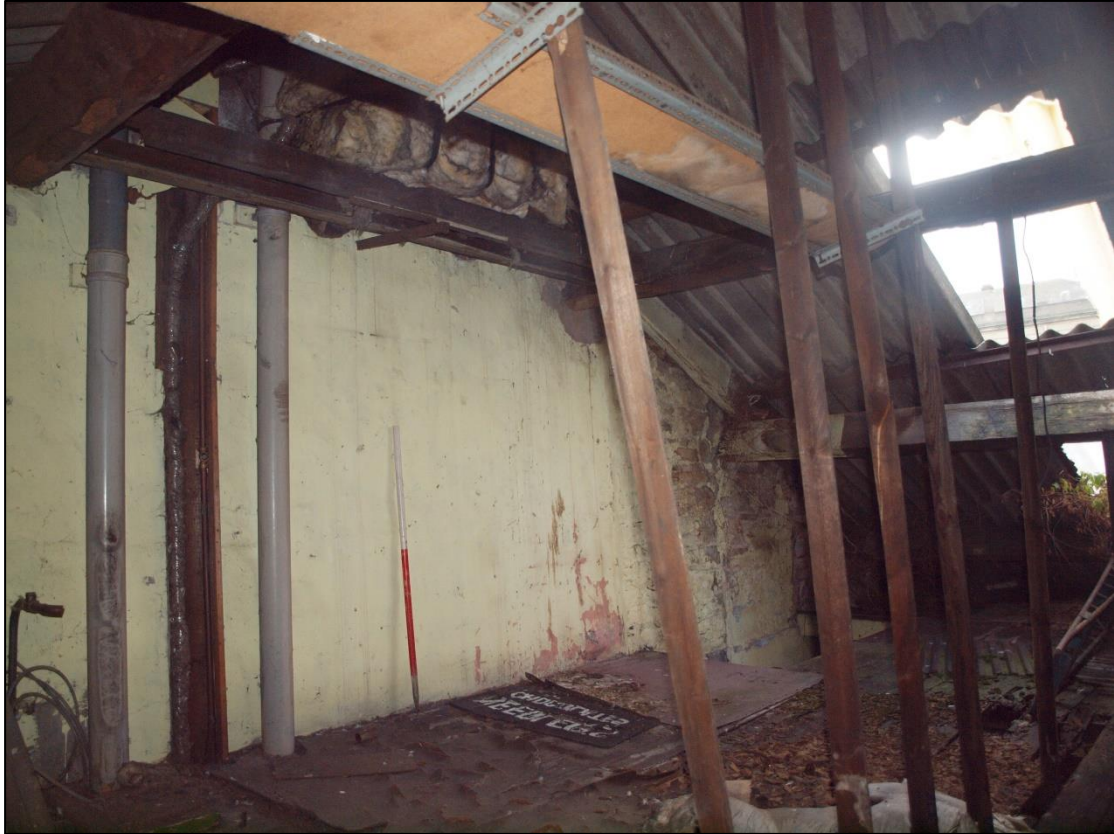
Plate 77: East gable in attic
