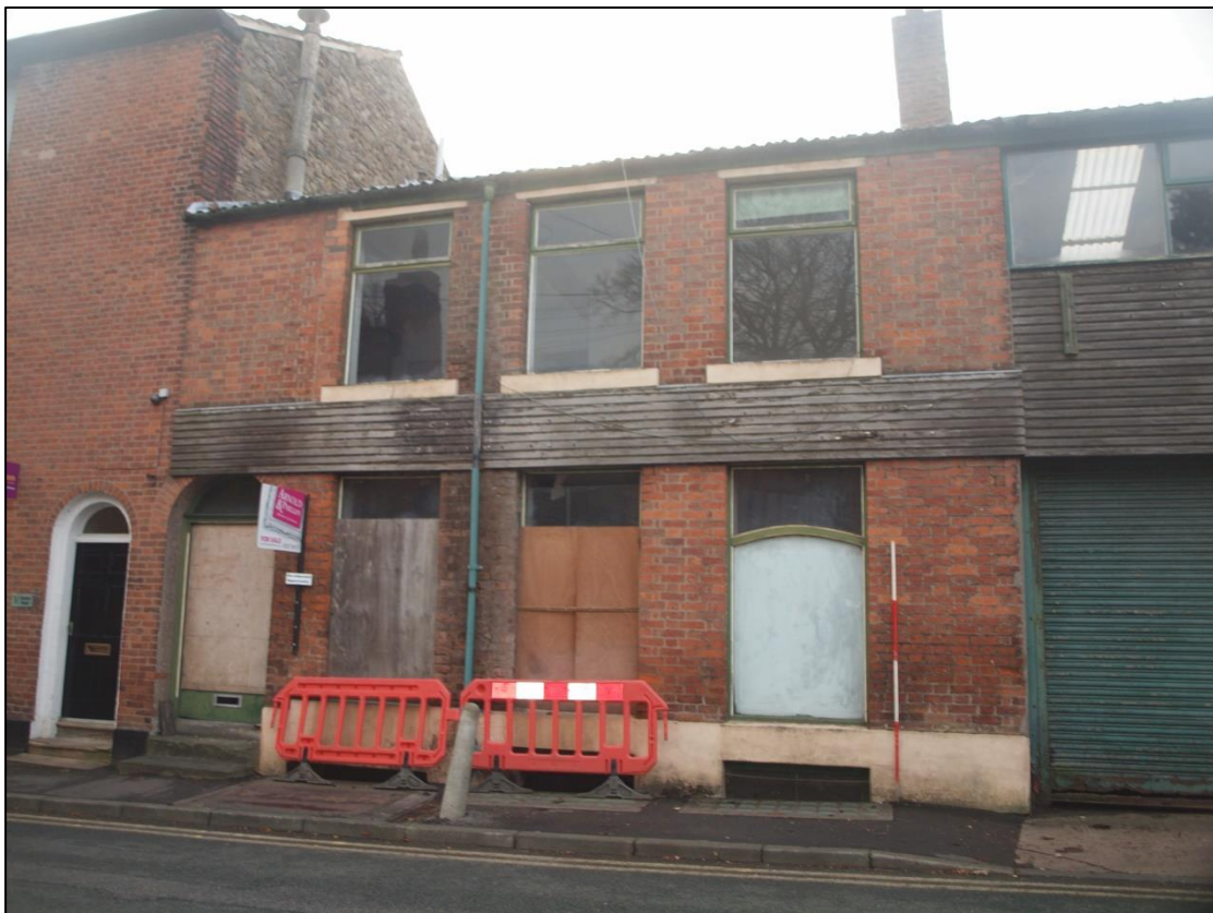
Plate 6: North elevation of 5 Queens Road
