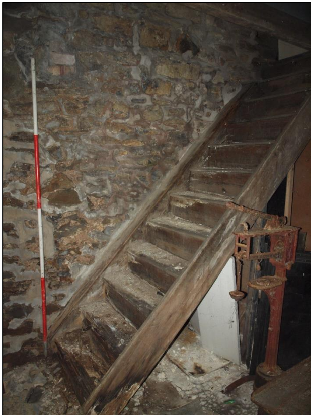
Plate 42: Staircase to first floor in Workshop
