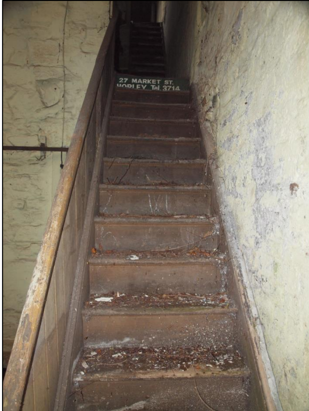
Plate 25: Staircase to first floor in rear yard of number 5
