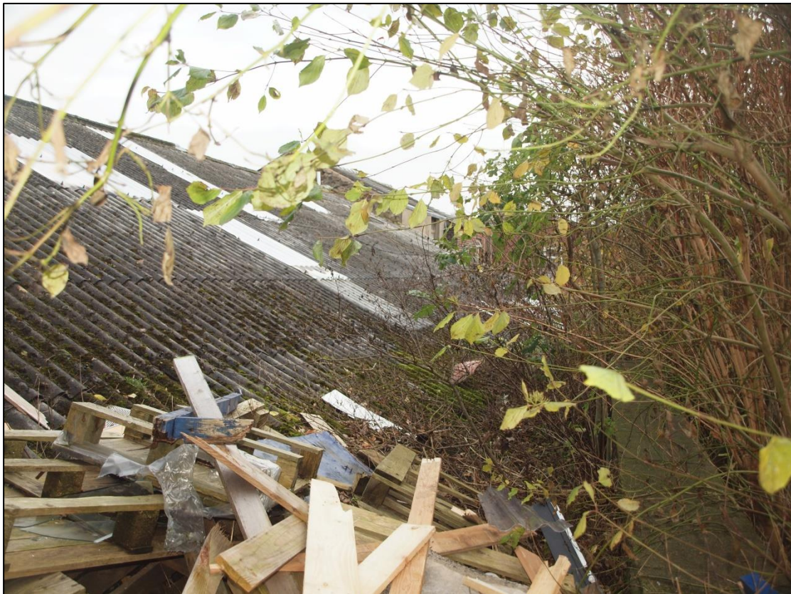
Plate 14: Corrugated asbestos roofing at rear of building
