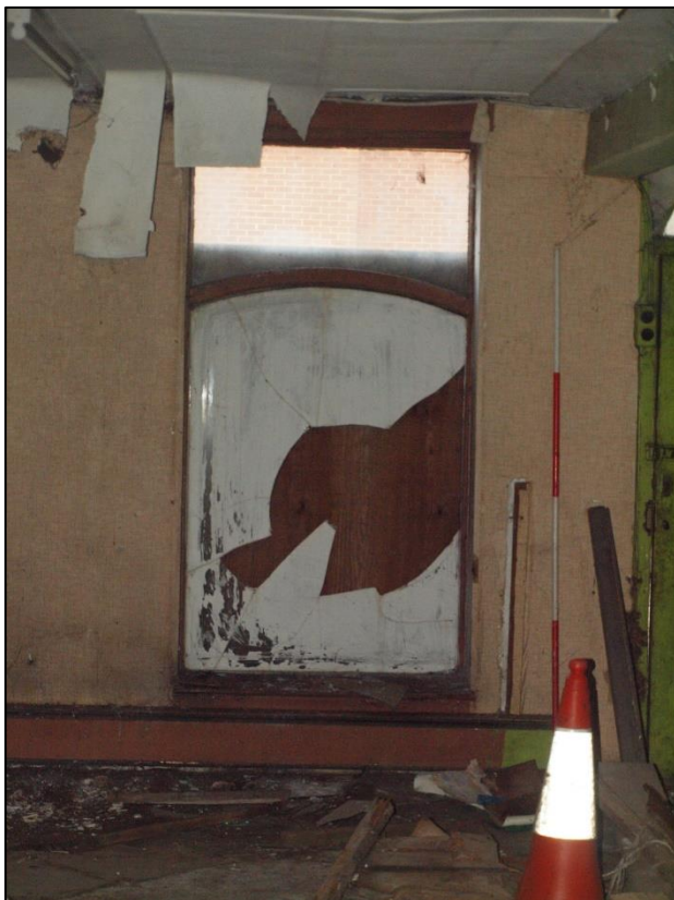
Plate 20: Ground floor of number 5 window
