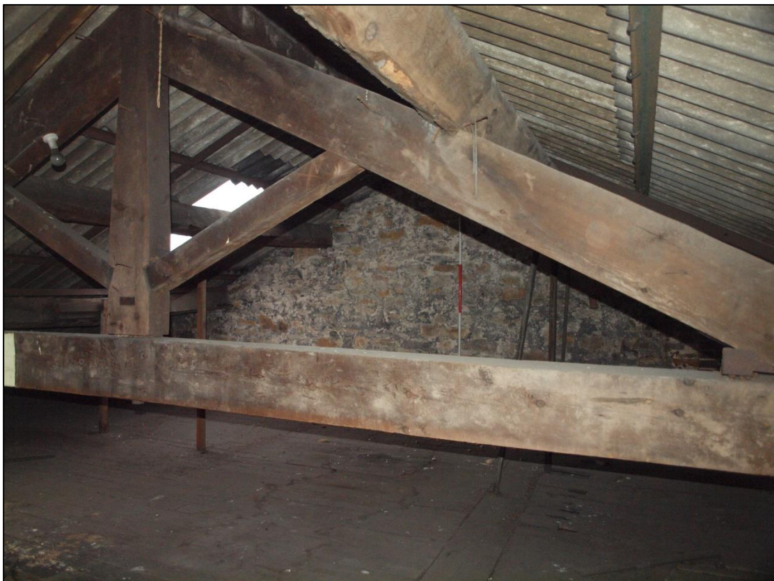
Plate 72: General shot of attic
