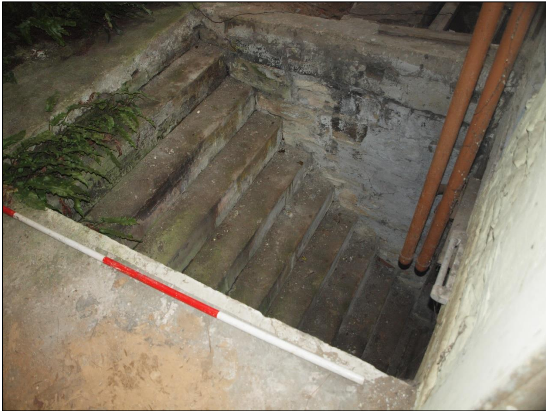
Plate 27: Inserted staircase to cellar in rear yard
