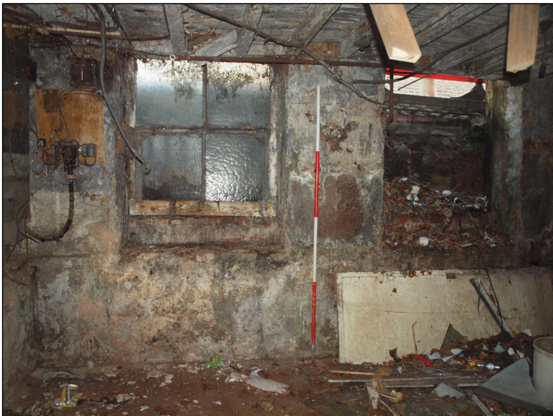
Plate 46: Detail of cellar windows
