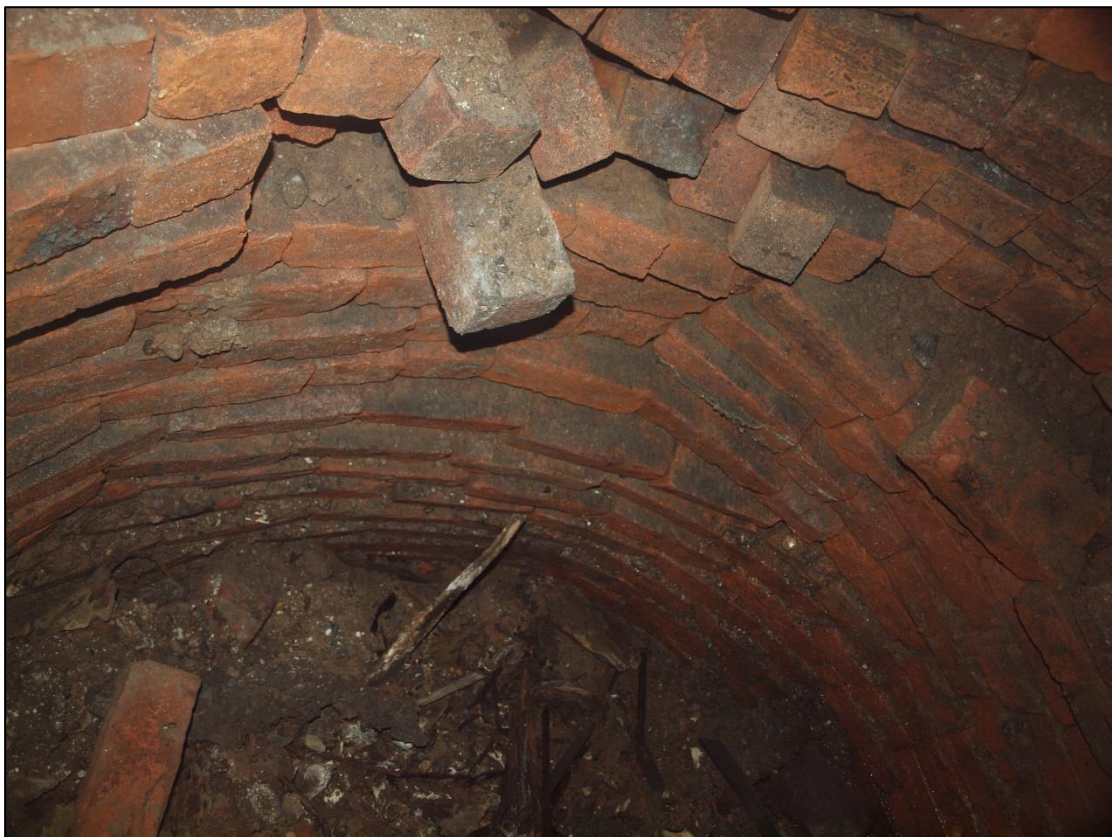
Plate 48: Well below flagstone in cellar
