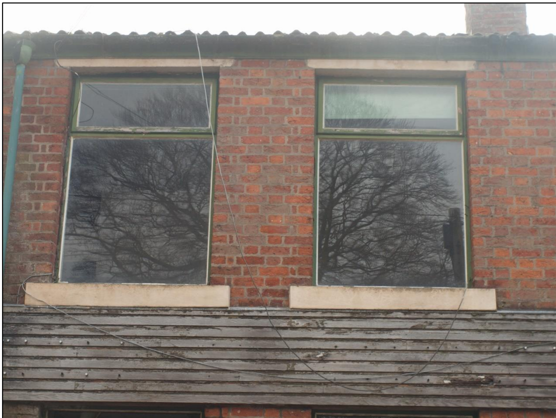
Plate 10: Detail of first floor windows of 5 Queens Road
