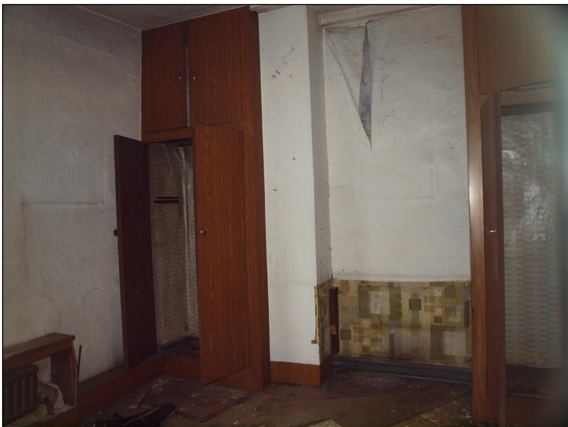
Plate 60: Livingroom at north end of number 5 first floor
