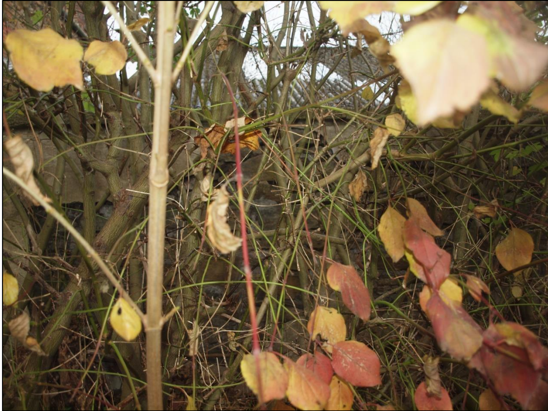
Plate 15: Stone wall hidden by hedge at south elevation
