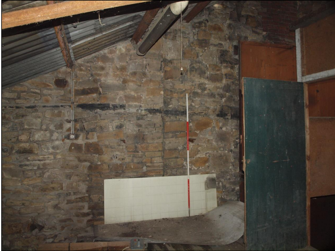
Plate 69: Detail of west wall showing straight joint
