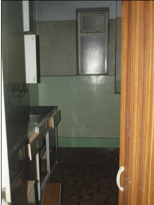
Plate 61: Kitchen at north end of number 5 first floor
