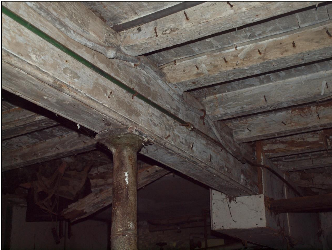
Plate 47: Detail of moulded timber beam in cellar
