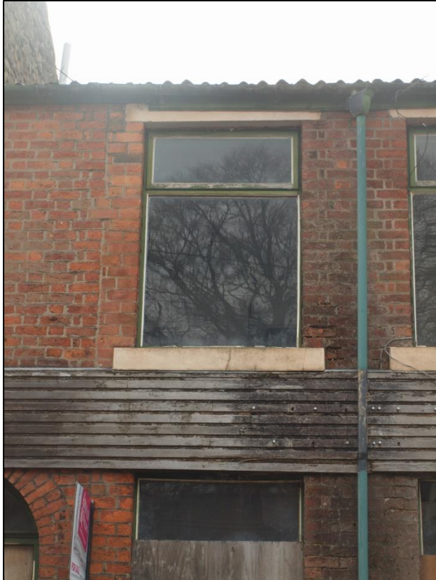
Plate 9: Detail of first floor windows of 5 Queens Road showing straight joint
