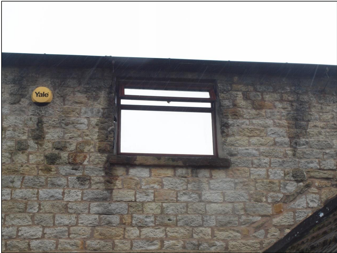
Plate 9: Bay 4 first floor window
