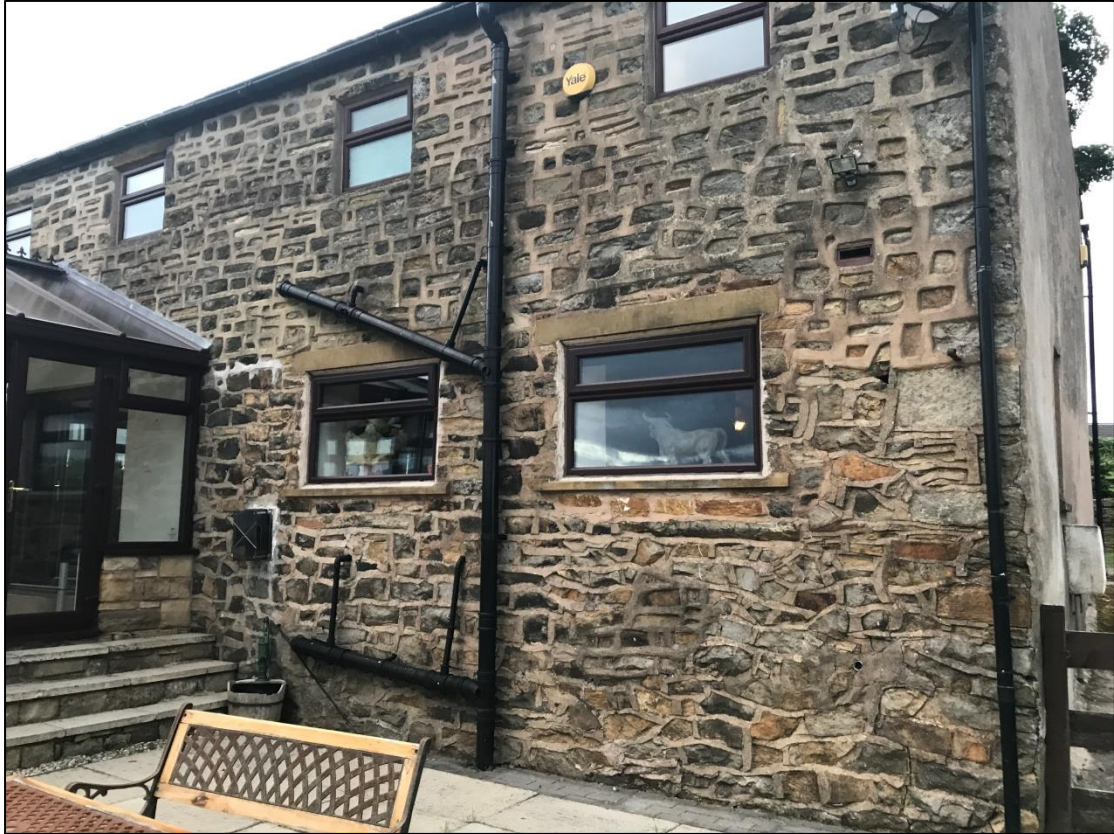
Figure 9: Rear of Standhill farm prior to demolition (courtesy of Marcus Walsh)
