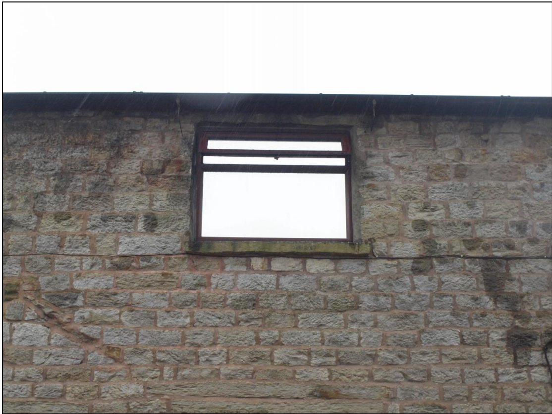
Plate 5: Bay 2 first floor window
