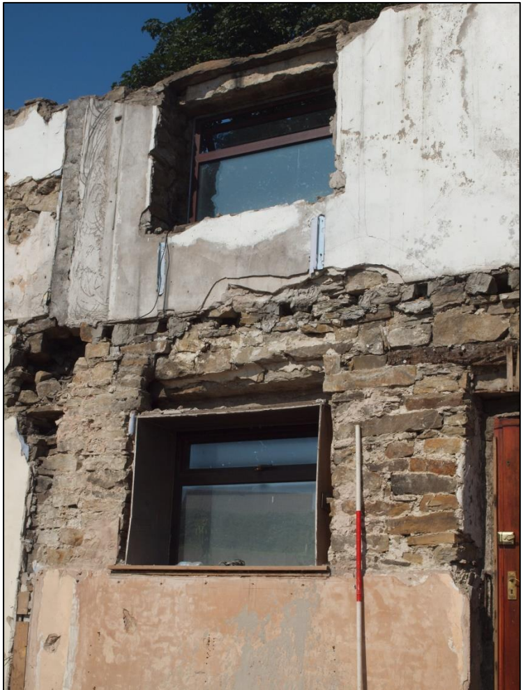
Plate 19: Bay 2 showing exposed stonework
