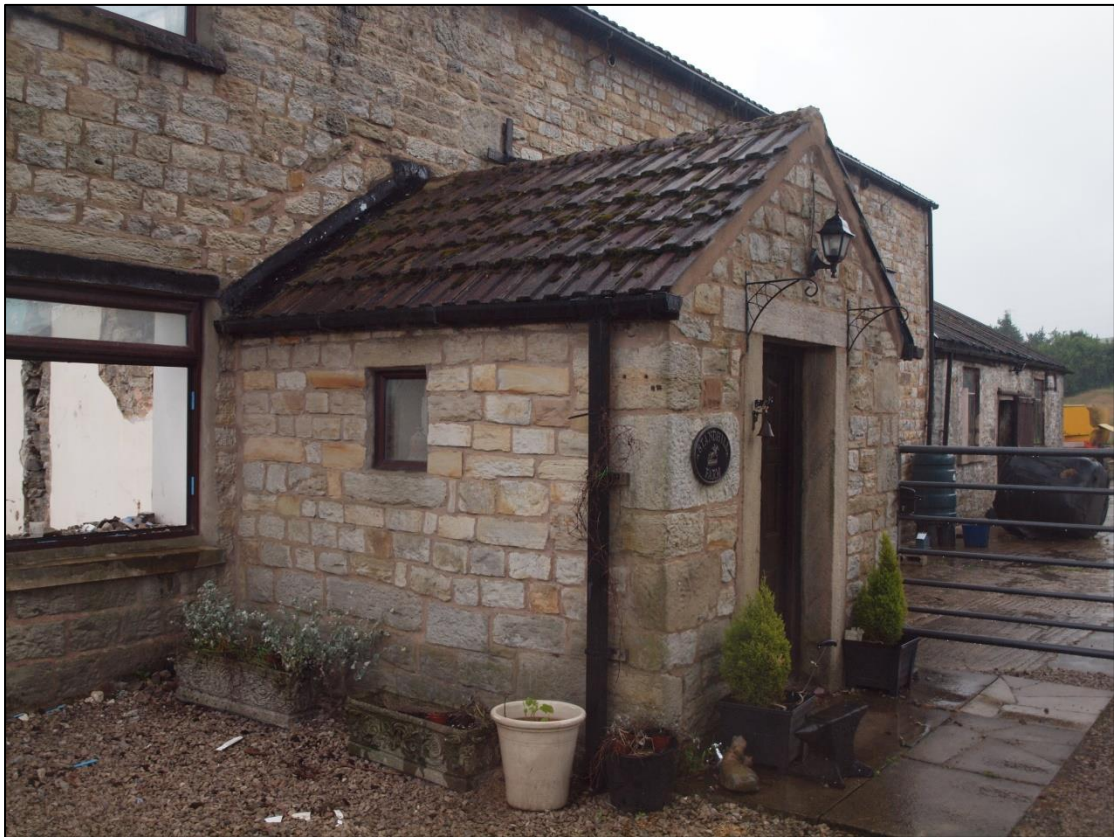
Plate 10: Porch butting face of bay 5
