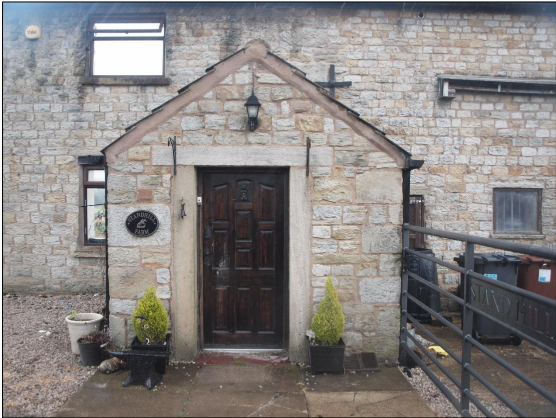
Plate 11: Front of porch in bay 5
