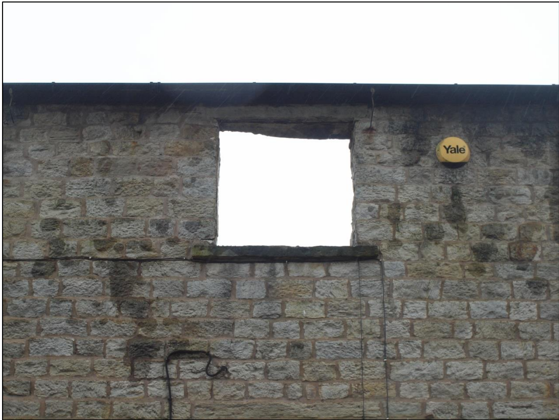
Plate 7: Bay 3 first floor window
