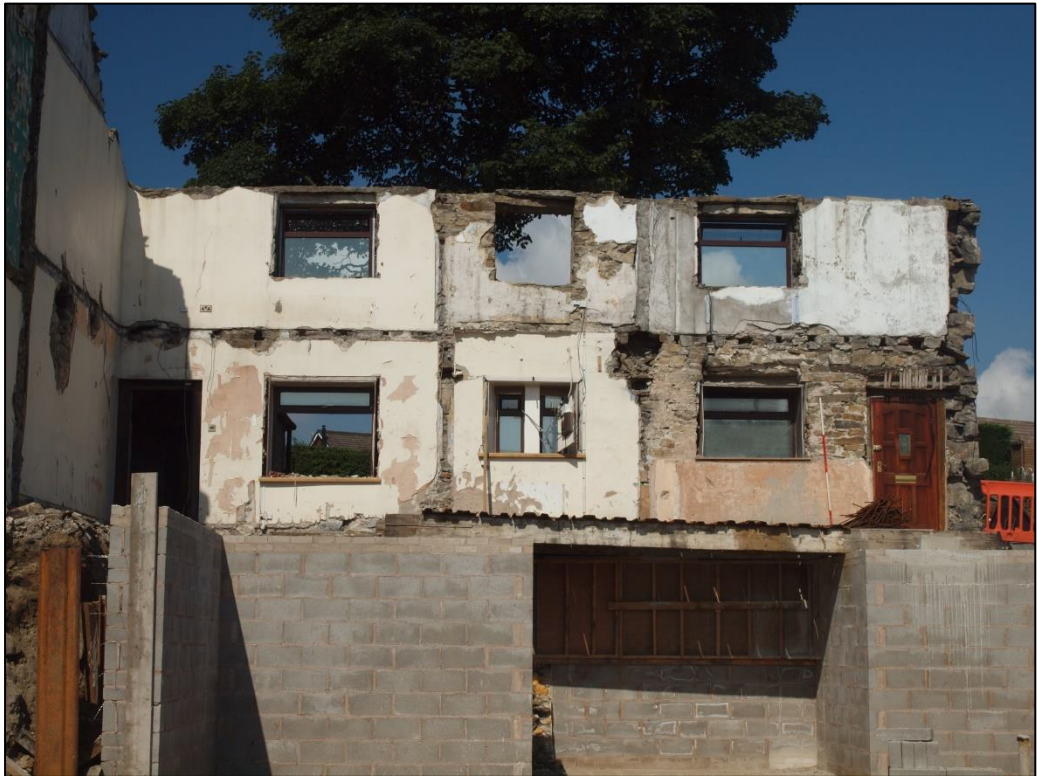
Plate 20: General shot of rear of wall showing lies of former walls and first floor
