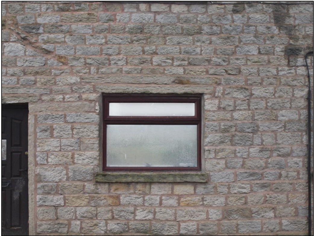
Plate 4: Bay 2 ground floor window
