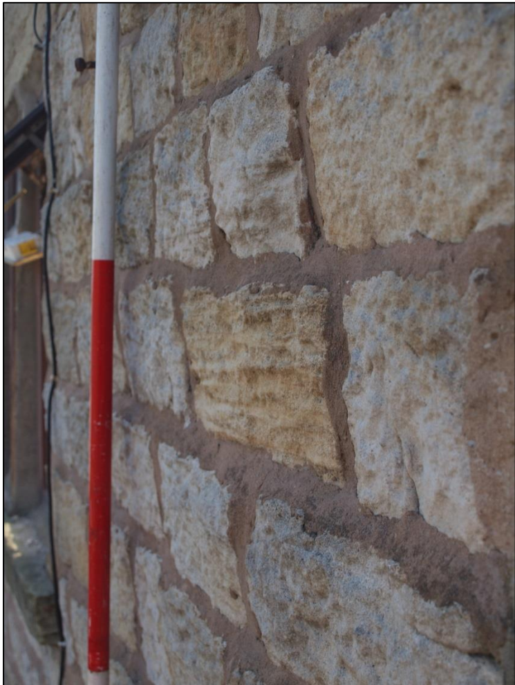
Plate 13: Detail of watershed sandstone
