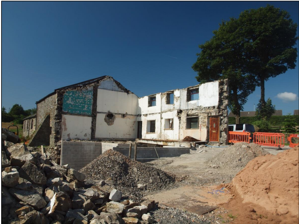
Plate 14: General shot of rear of wall in relation to barn gable
