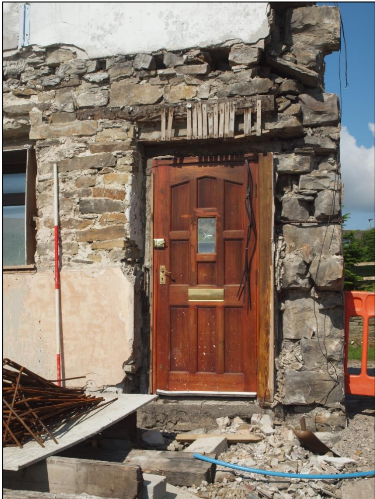
Plate 17: Detail of doorway in bay 1
