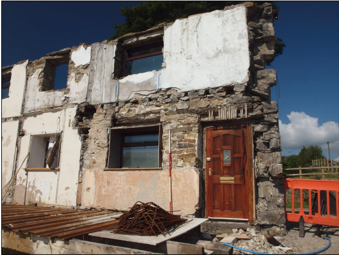
Plate 16: Rear of wall, bays 1 -3
