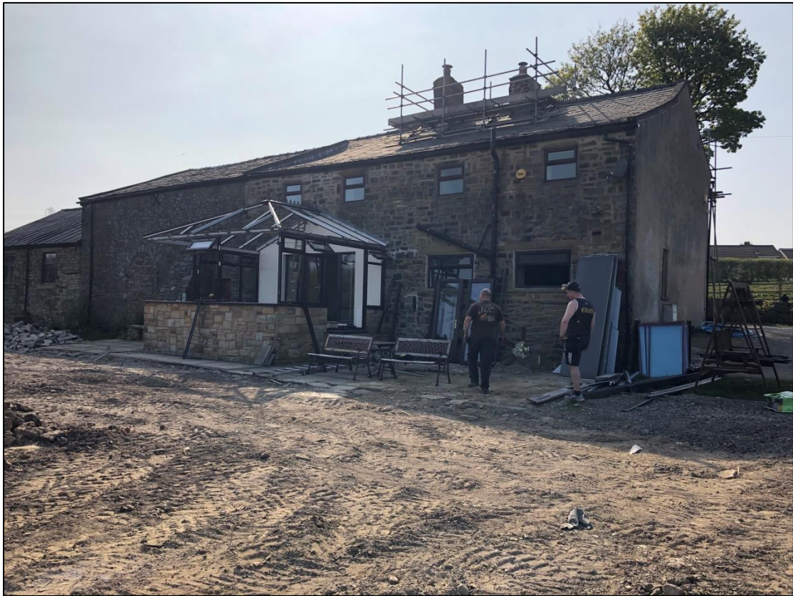
Figure 7: Rear of Standhill farm prior to demolition (courtesy of Marcus Walsh)
