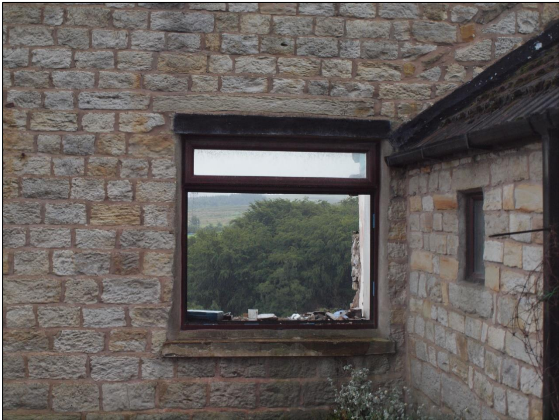
Plate 8: Bay 4 ground floor window
