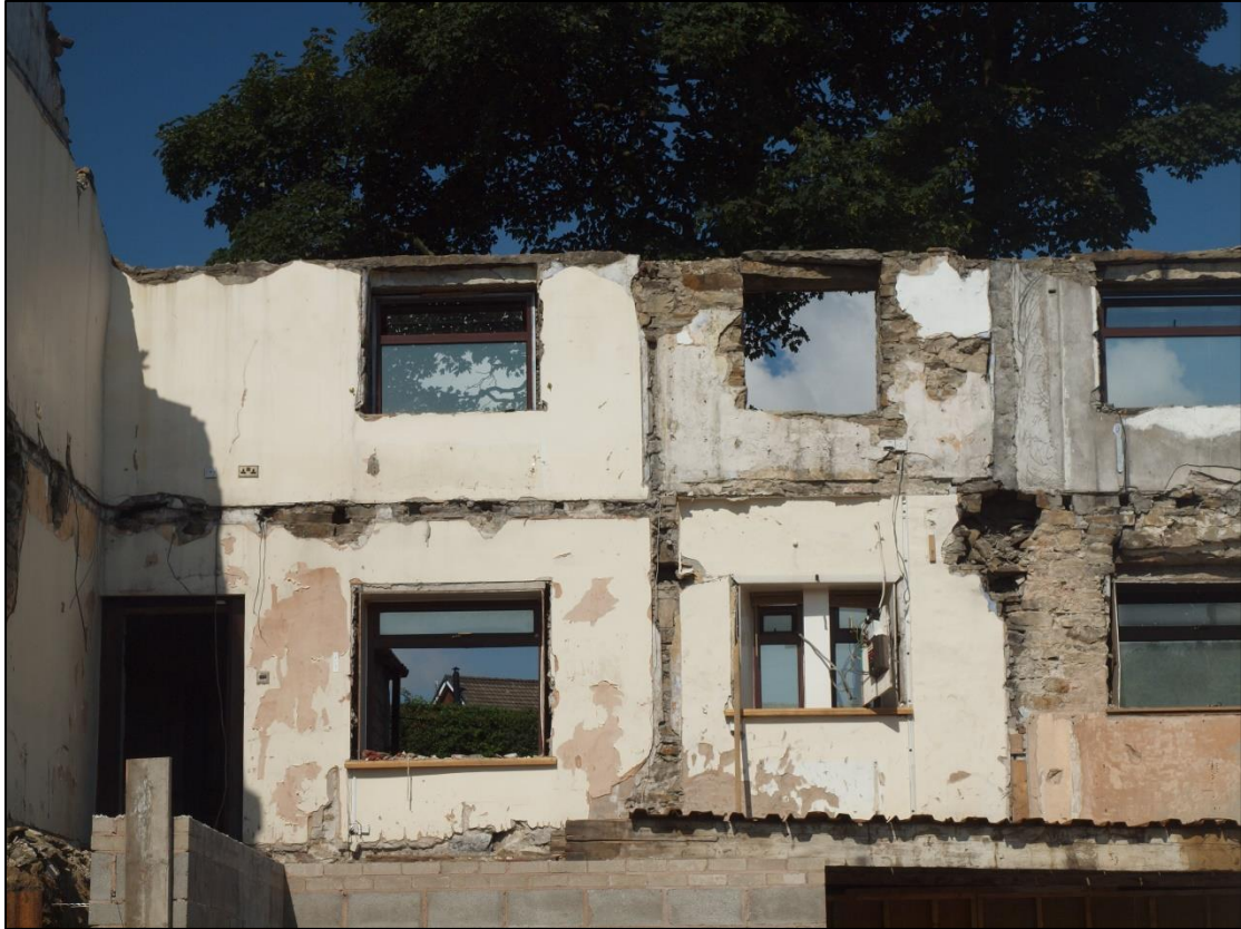
Plate 21: Rear of walls showing bays 2 - 5
