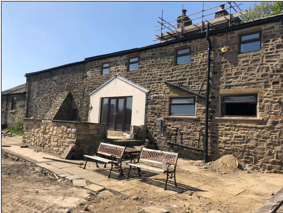
Figure 8: Rear of Standhill farm prior to demolition (courtesy of Marcus Walsh)
