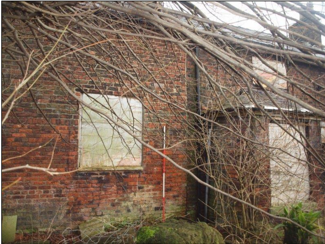
Plate 5: South elevation of west extension
