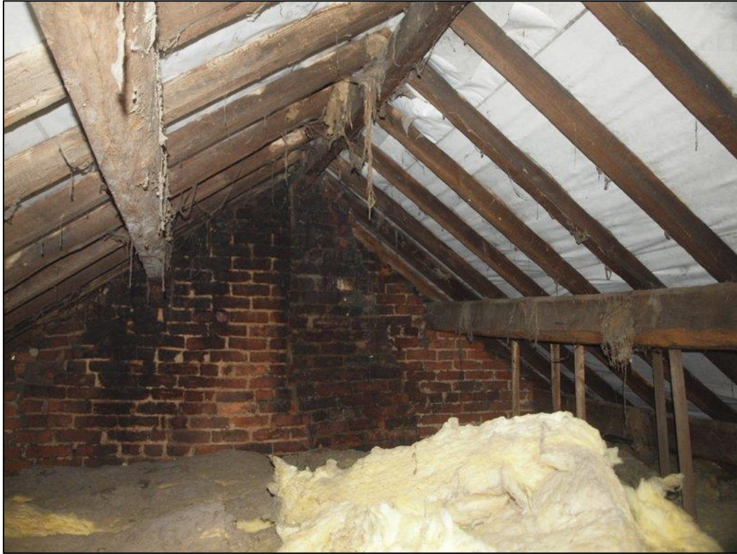
Plate 59: Eastern cottage extension roof space
