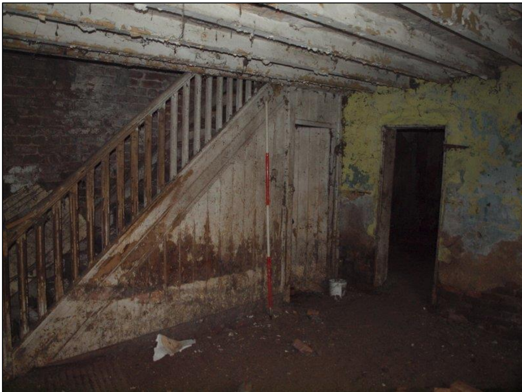
Plate 38: Southern room of east extension
