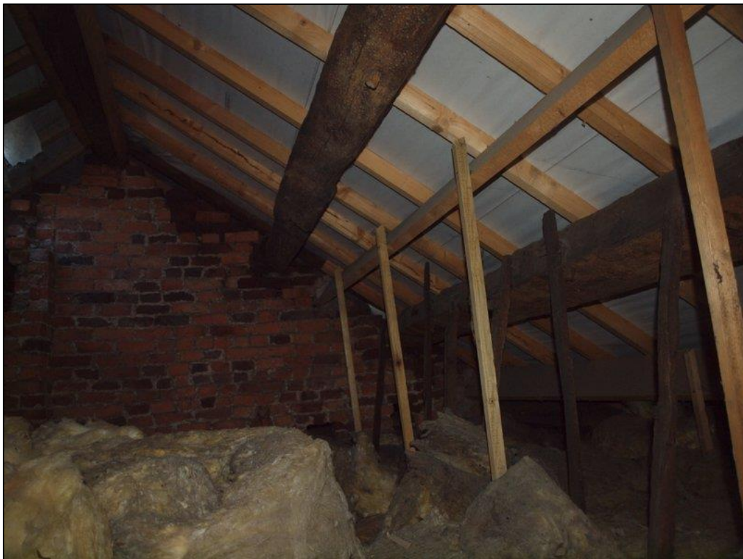
Plate 58: As above showing purlins
