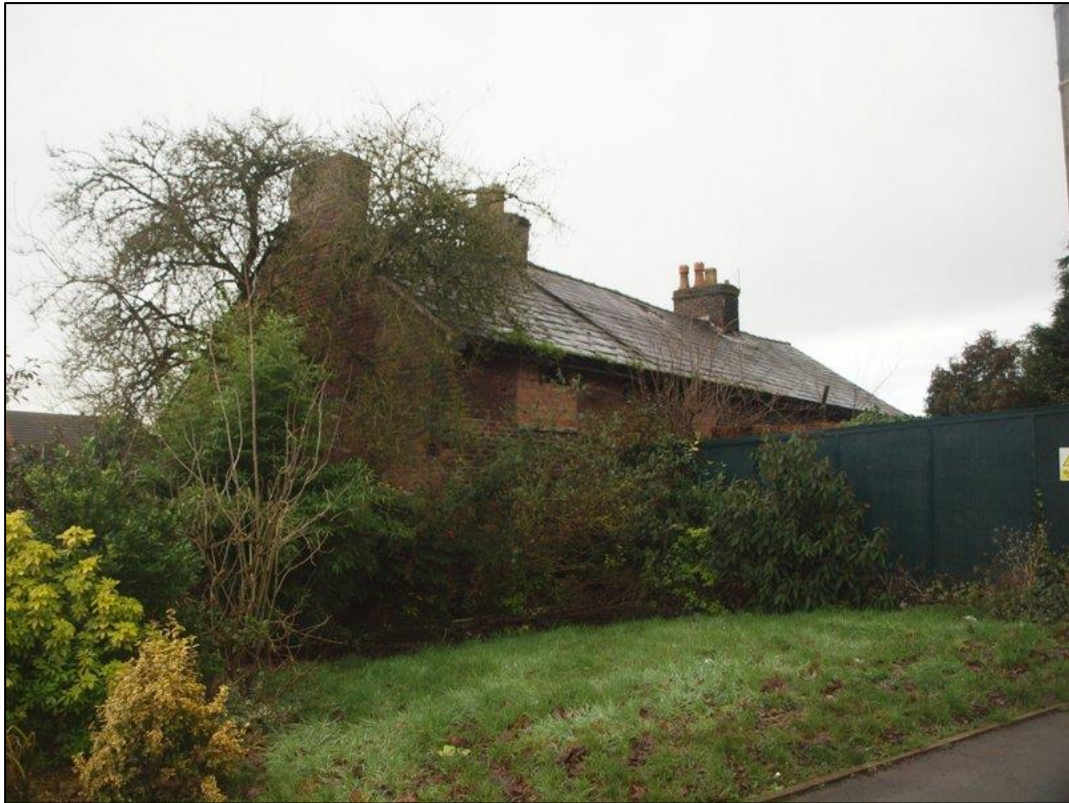
Plate 13: General shot of north elevation
