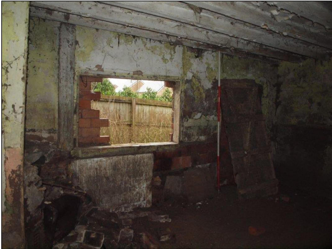
Plate 39: Southern room of east extension
