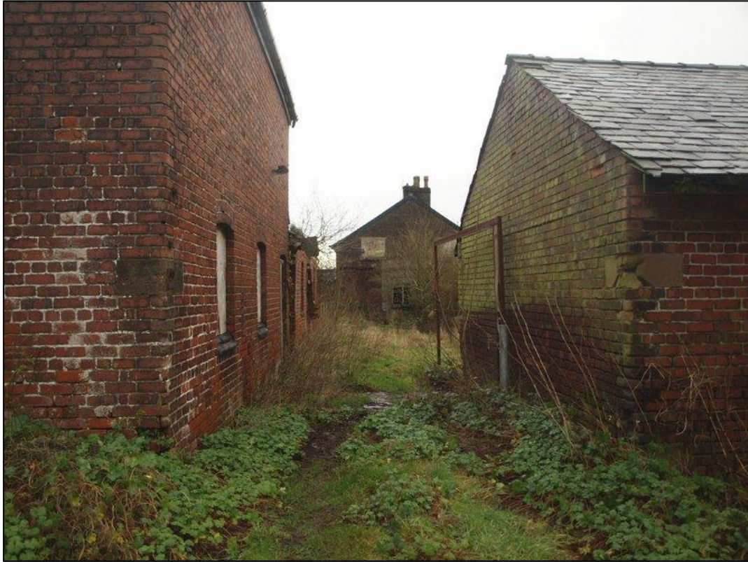
Plate 1: General shot of the farm showing the farmhouse (centre) with shippon (left) and piggery (right)
