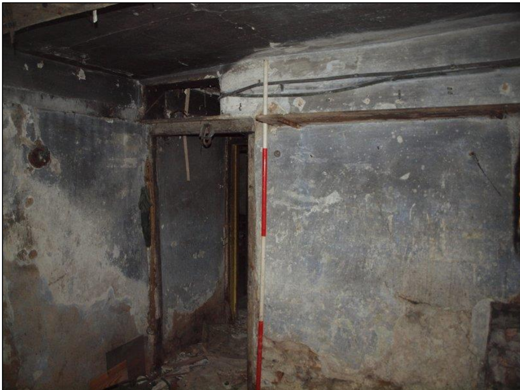
Plate 34: Northeast room of main building
