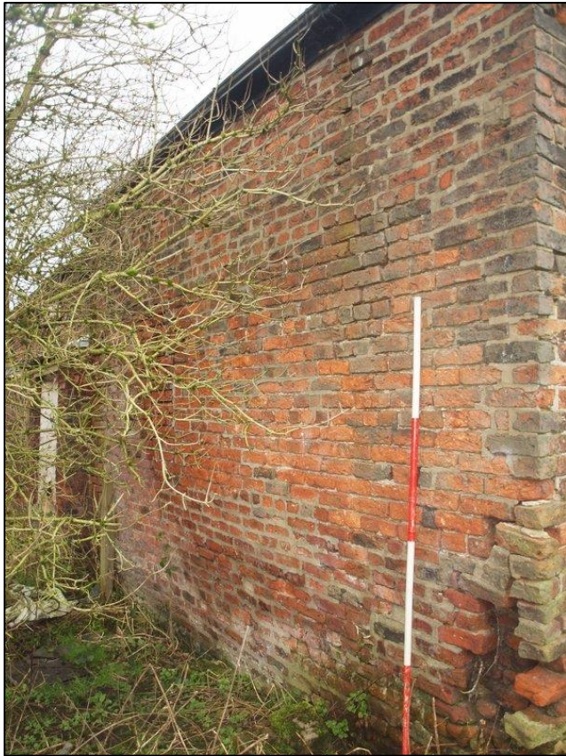
Plate 9: South elevation of east extension
