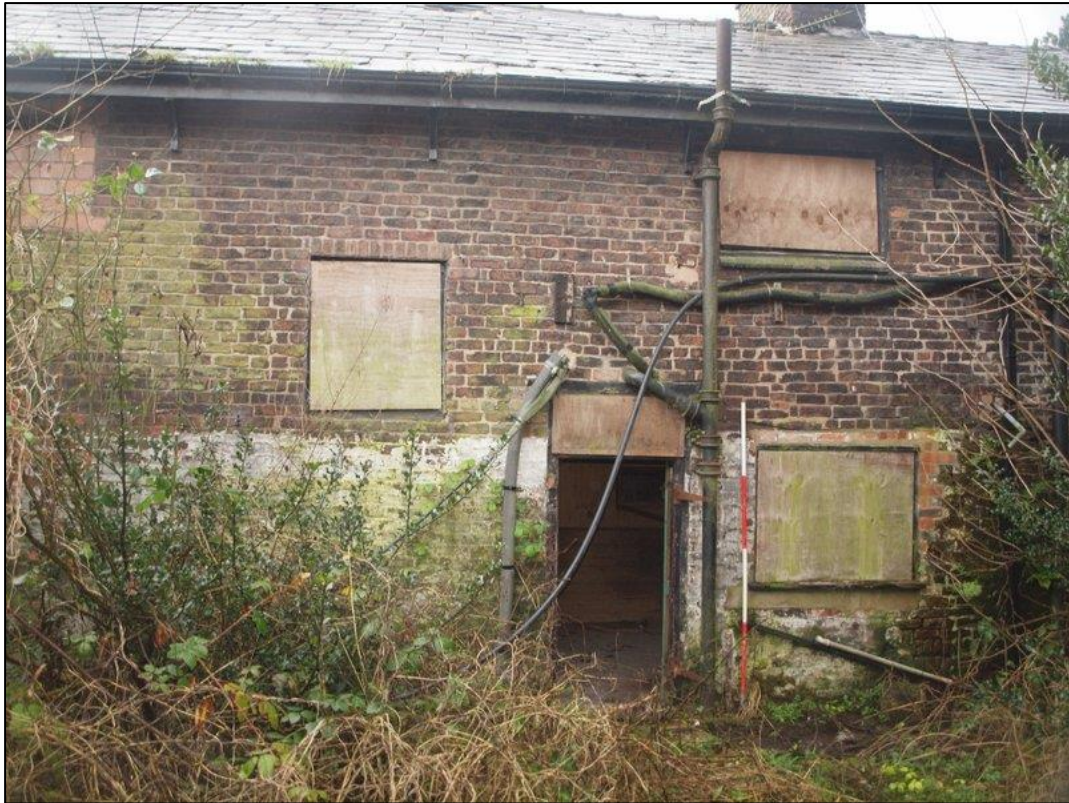
Plate 15: North elevation showing back door
