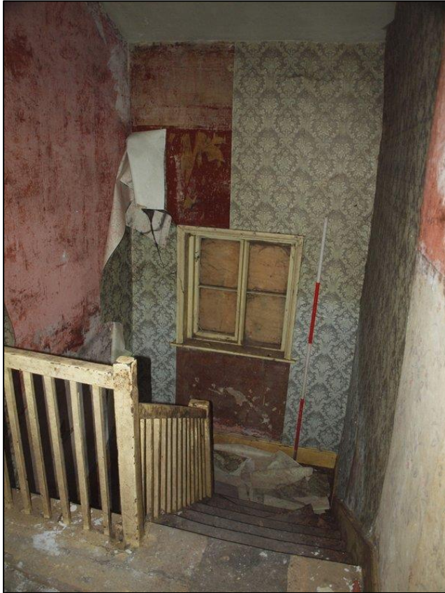
Plate 43: Main stairs landing
