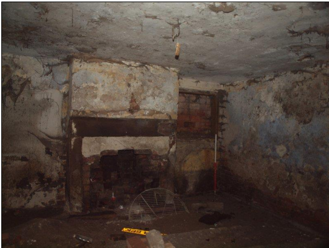
Plate 42: Northern room of east extension
