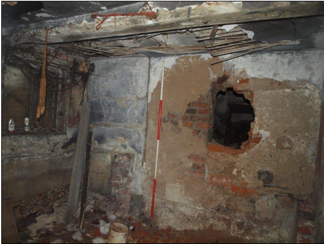
Plate 33: Northeast room with blocked doorway to eastern extension
