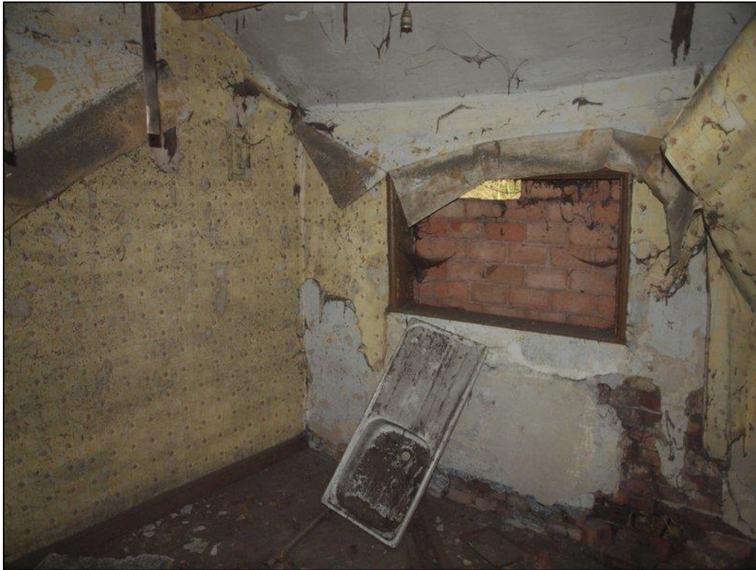
Plate 53: Bedroom in main building accessed from east extension
