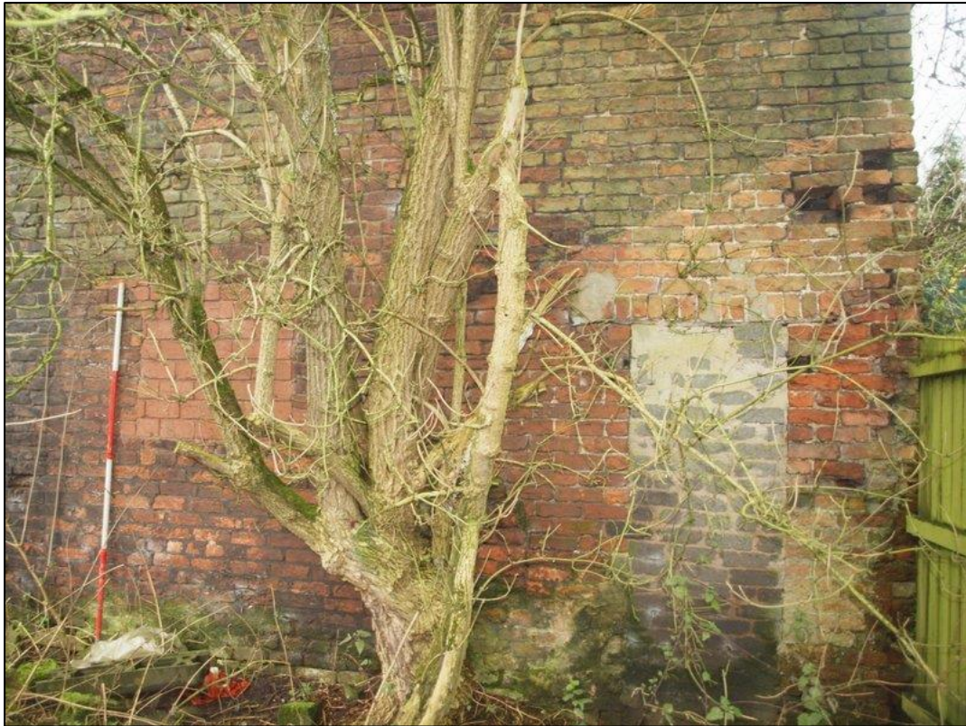
Plate 11: Northern end of east elevation
