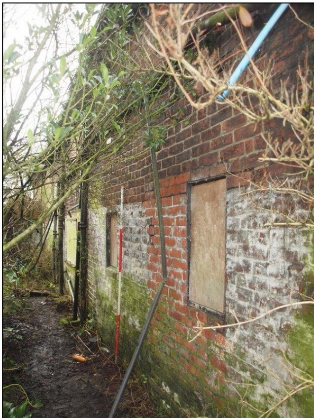
Plate 18: North elevation of west extension
