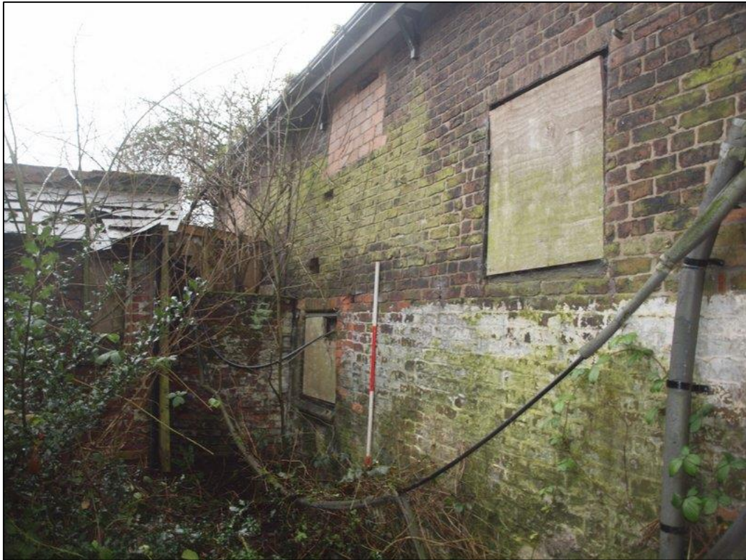
Plate 17: North elevation to the east of the doorway
