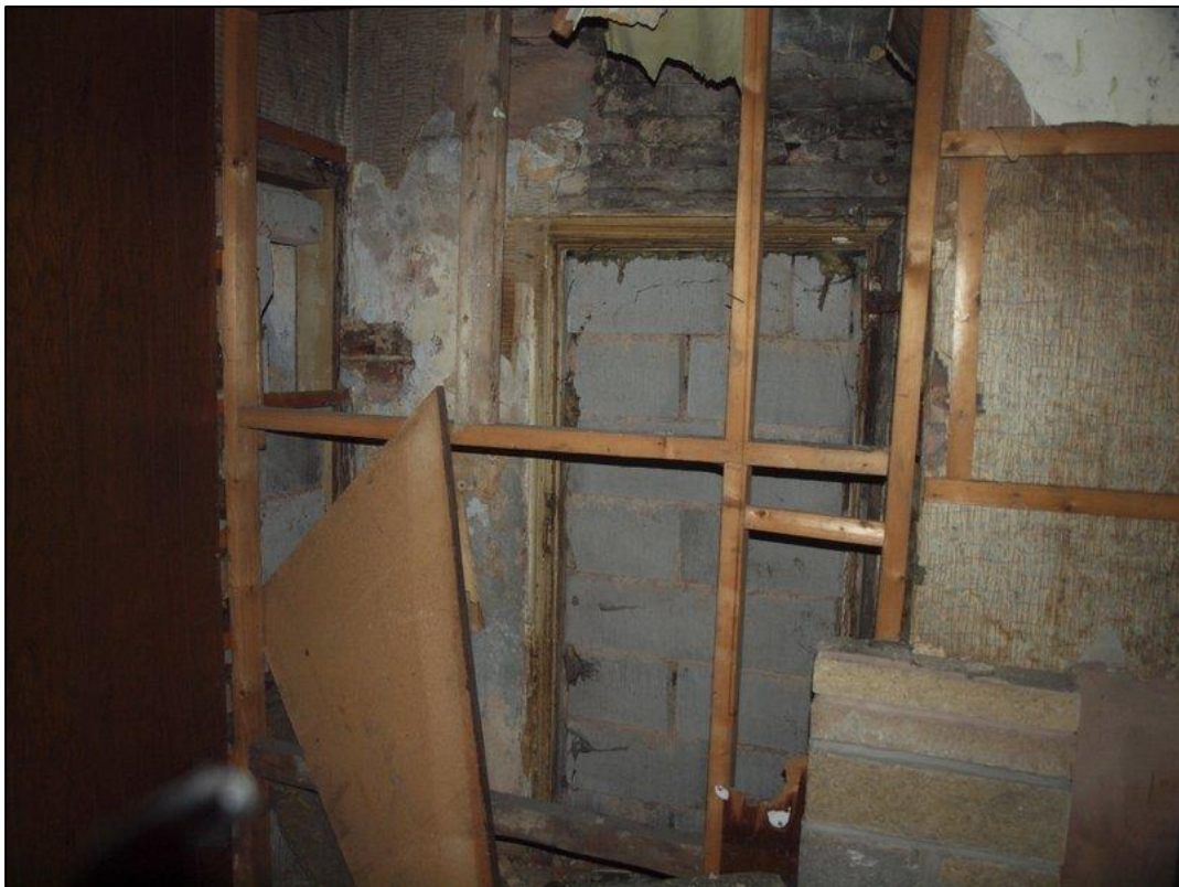
Plate 30: Blocked doorways in above
