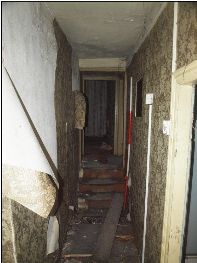
Plate 44: First floor corridor to west
