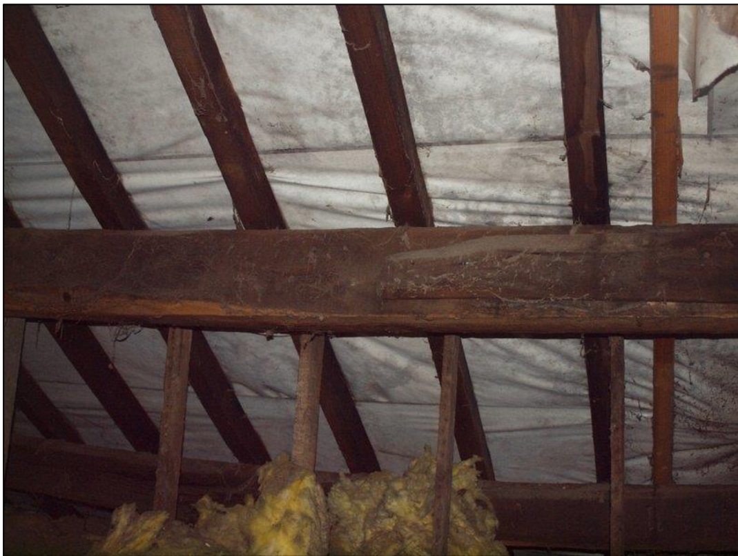
Plate 60: As above showing purlins
