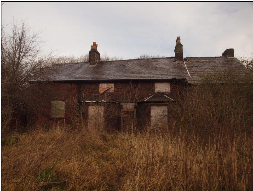
Plate 4: South elevation of building 1
