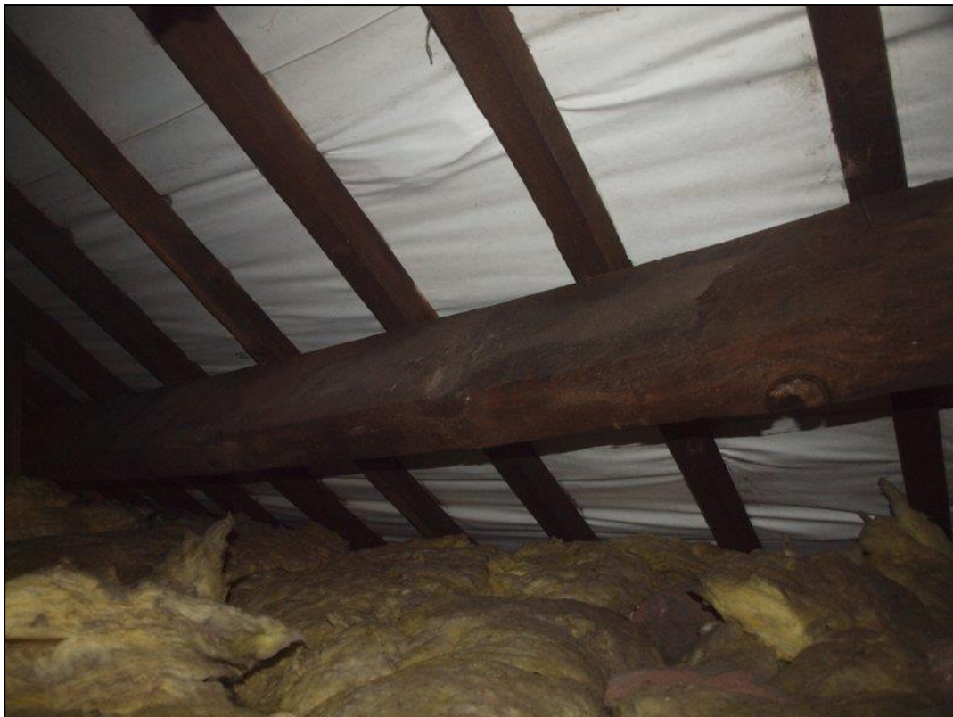
Plate 62: As above showing purlins
