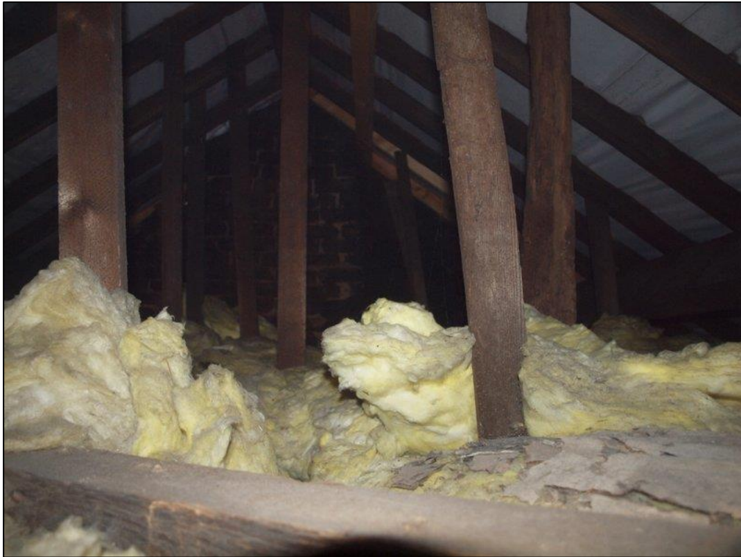
Plate 61: Western extension roof space
