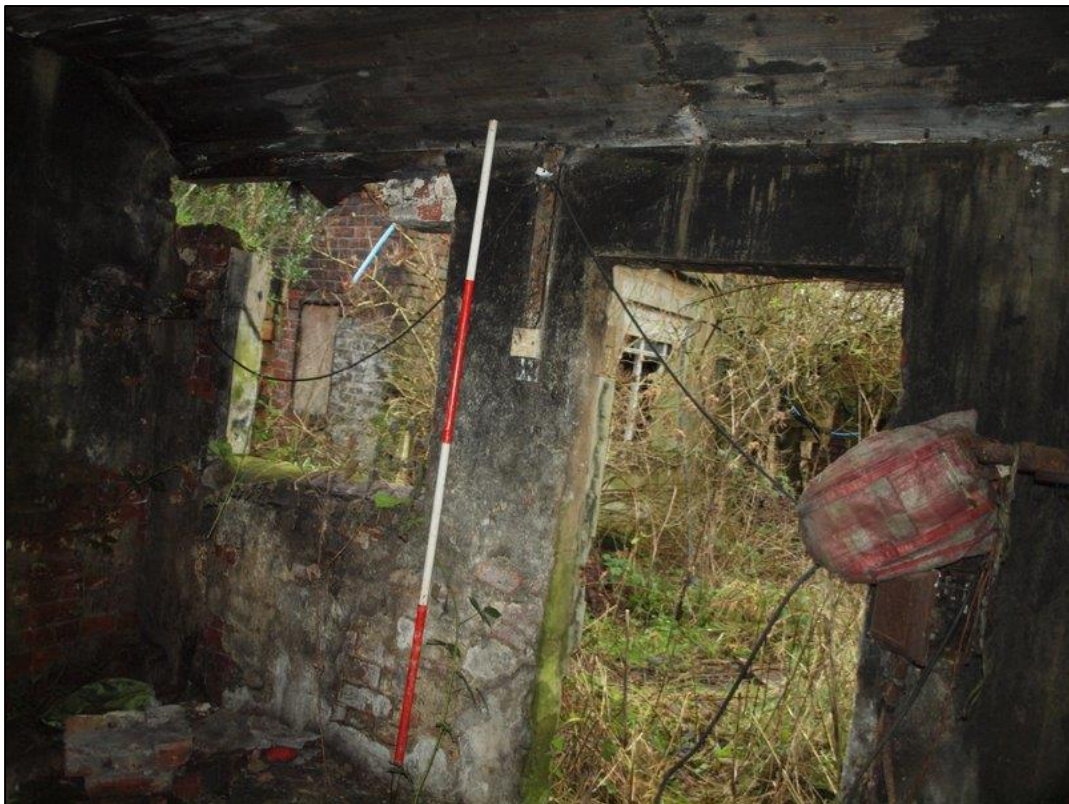
Plate 76: East room interior
