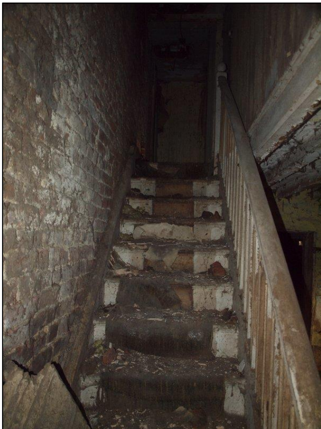
Plate 40: Detail of staircase in above
