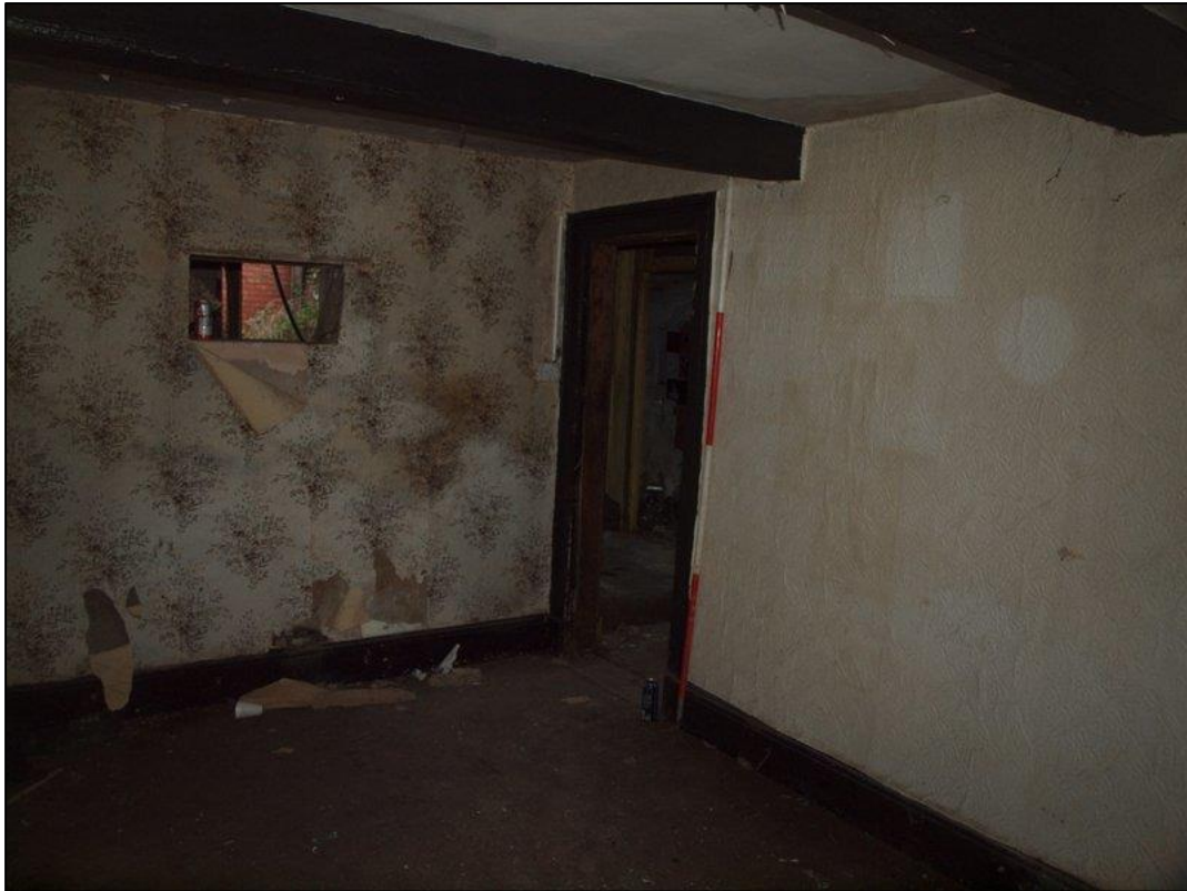
Plate 27: Western room of main house
