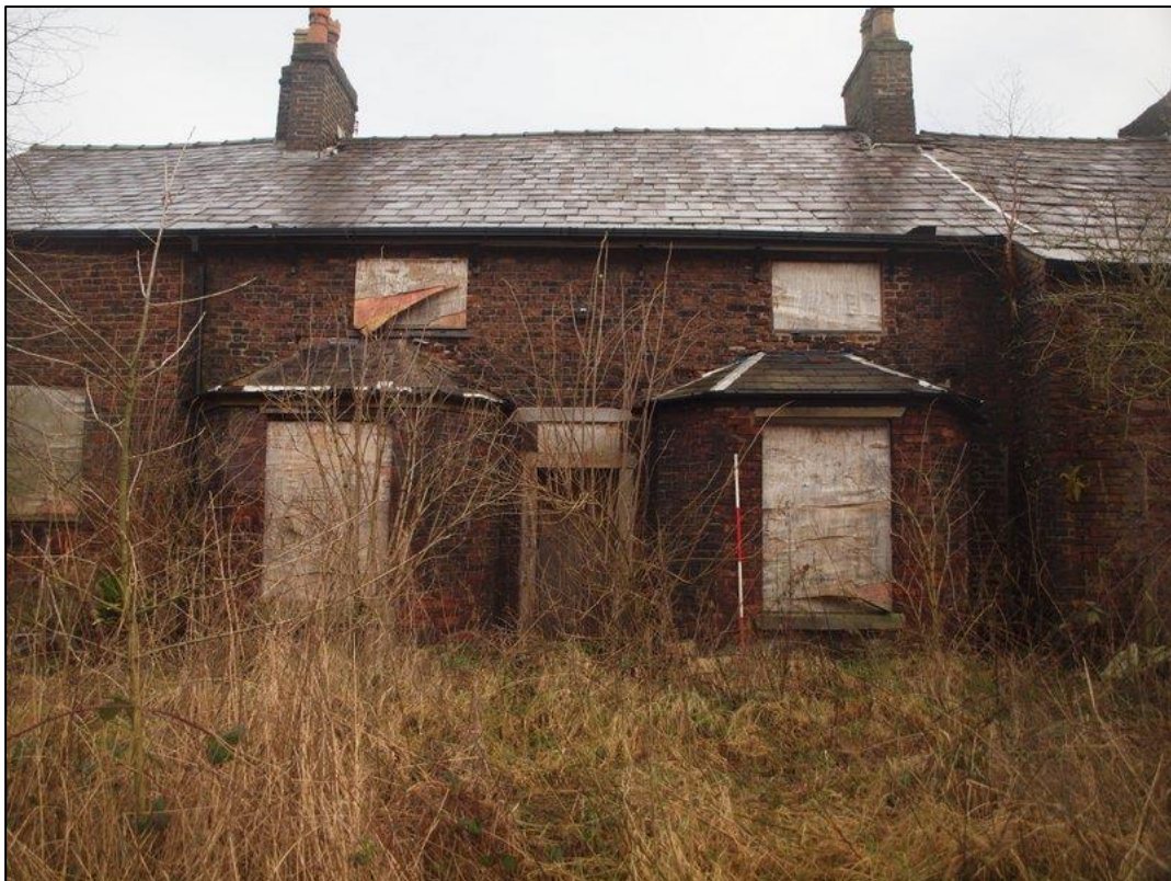
Plate 6: South elevation of original part of building 1
