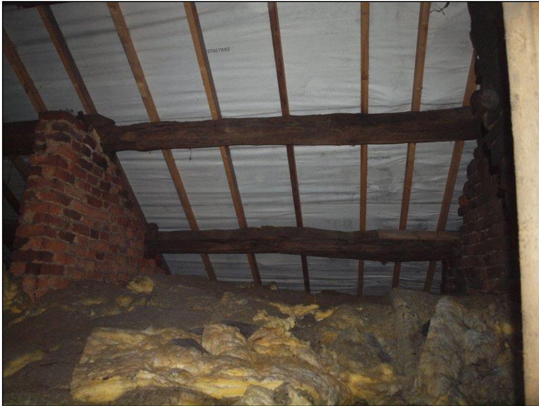
Plate 55: As above showing purlins
