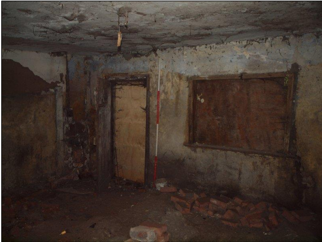
Plate 41: Northern room of east extension
