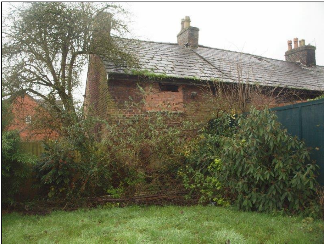
Plate 14: East end of north elevation
