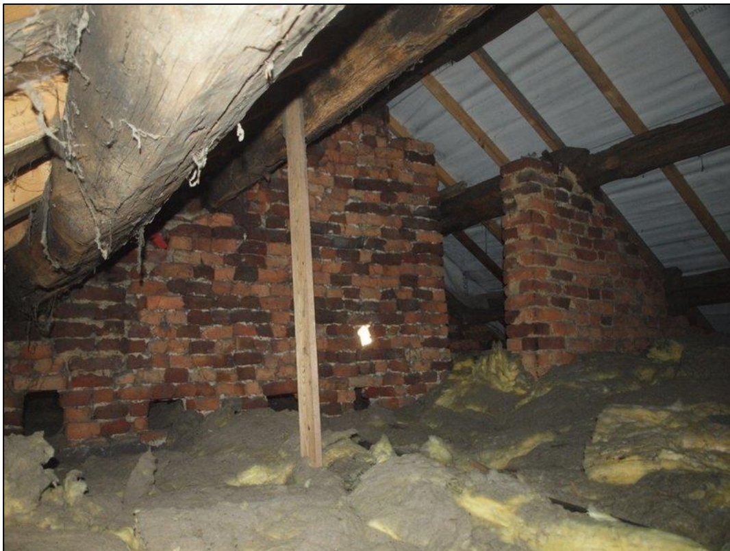
Plate 54: Eastern end of main building roof space
