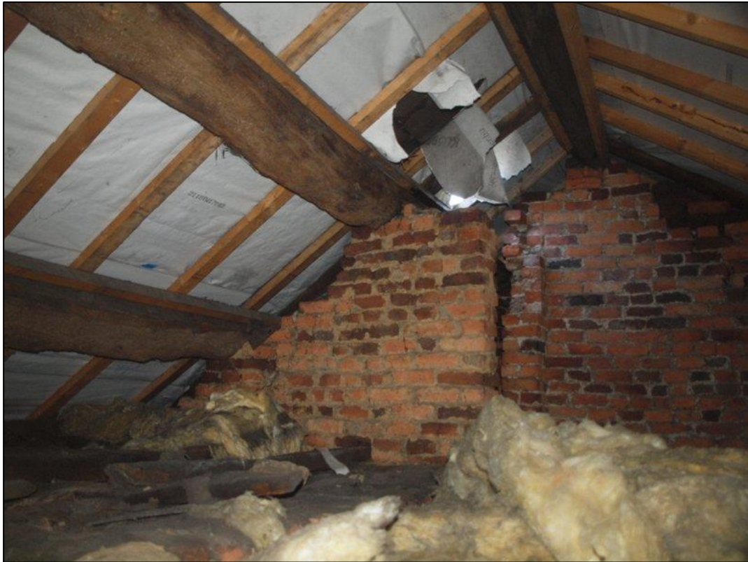
Plate 57: Western end of main building roof space
