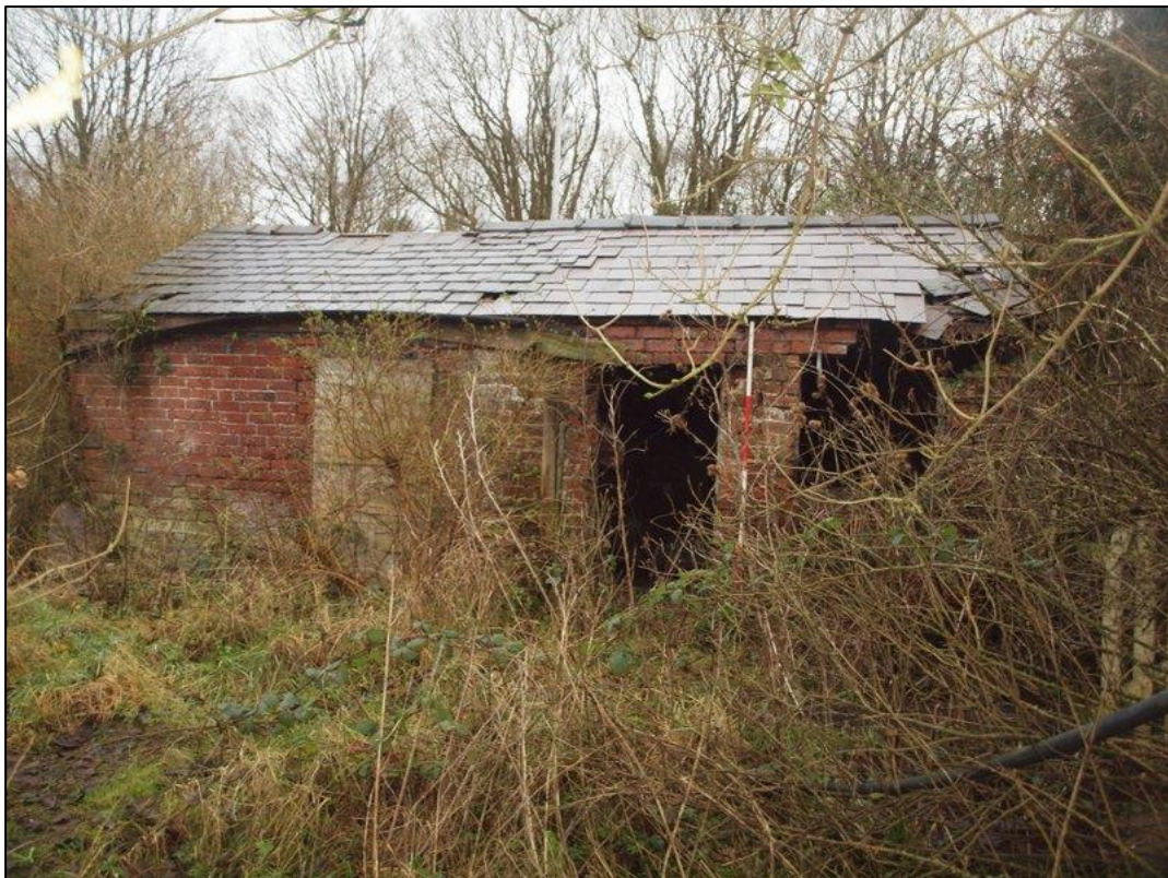
Plate 70: South elevation of building 3
