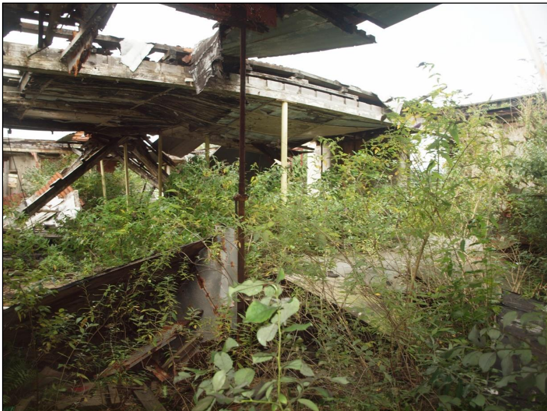
Plate 48: Second floor looking west from stair tower
