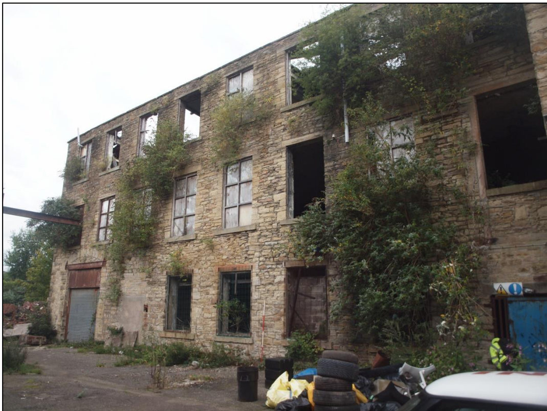
Plate 8: General shot of Southeast elevation
