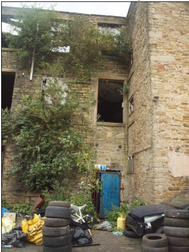
Plate 10: Detail of north end of elevation showing bay 8
