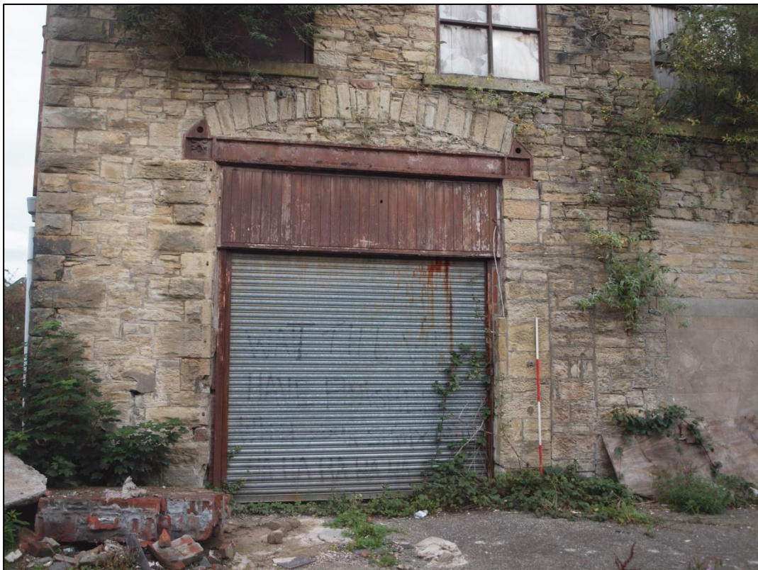
Plate 4: Loading bay to bays 1 and 2
