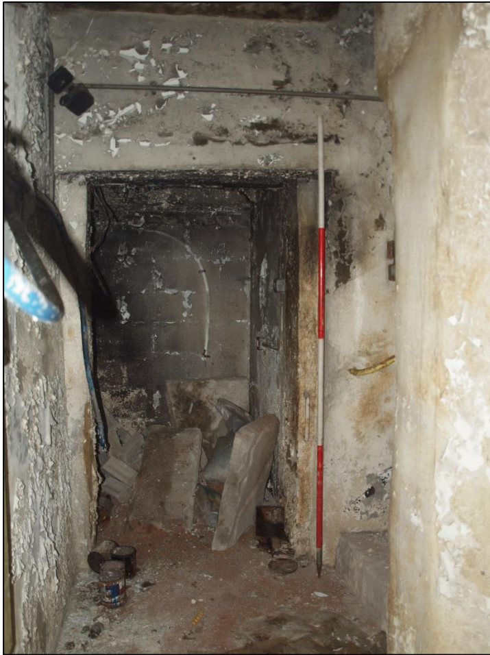
Plate 29: Bottom of stair tower showing blocked doorway
