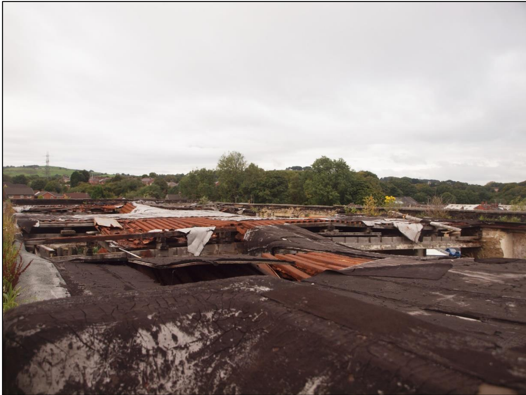
Plate 53: Detail of roof
