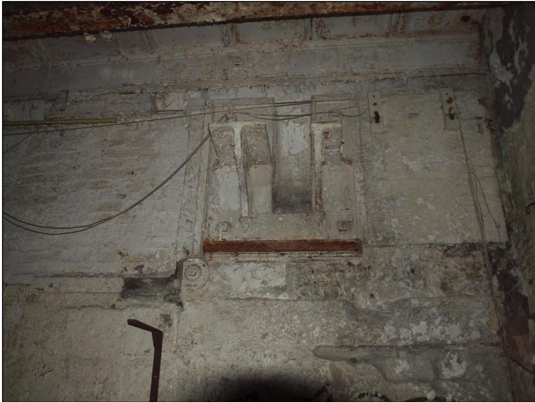
Plate 37: Detail of above
