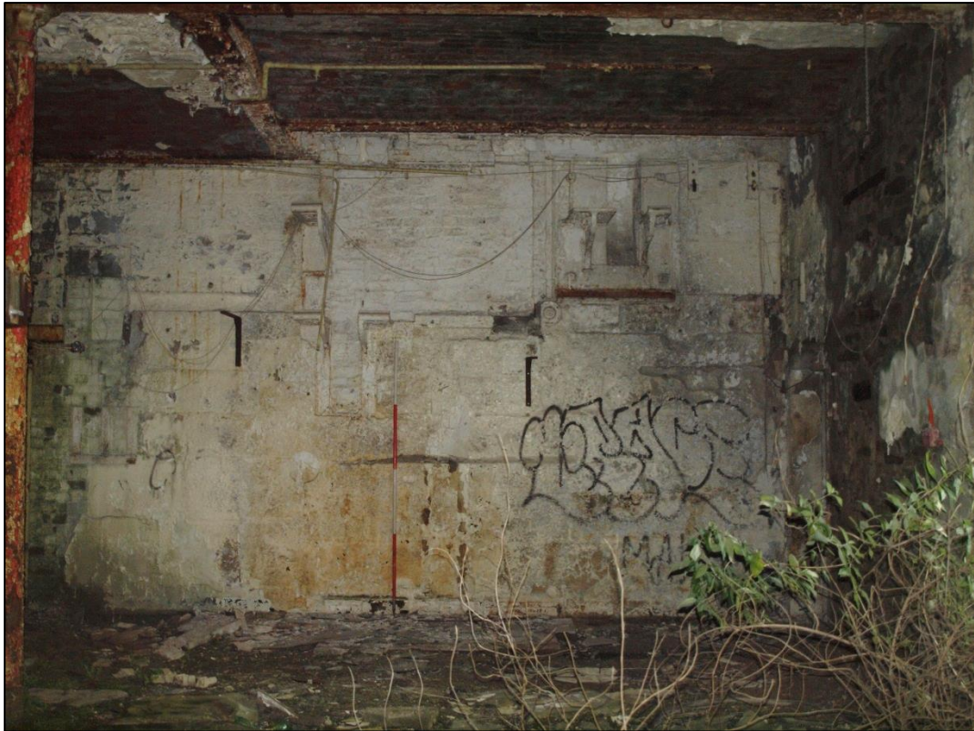
Plate 33: First floor northeast wall
