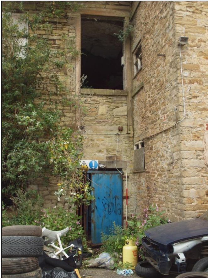
Plate 11: Detail of doorway in bay 8 with window above
