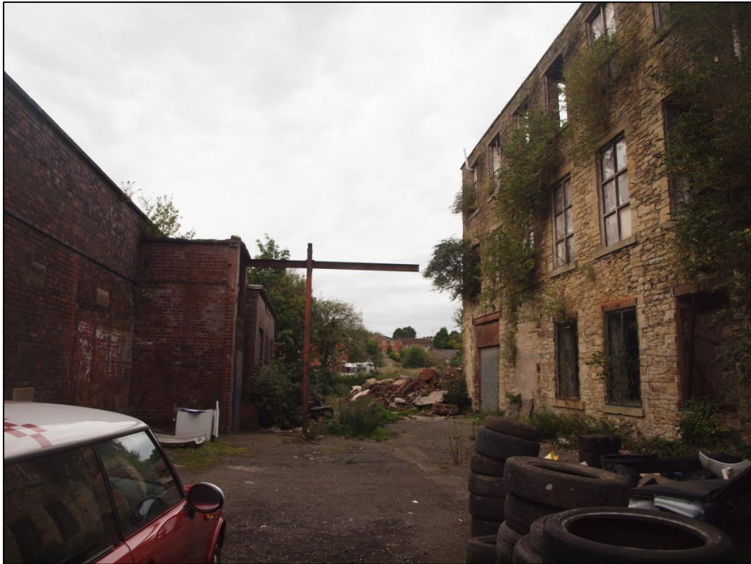
Plate 1: General shot showing Albert Mill (right) and Lower Darwen Mill (left)
