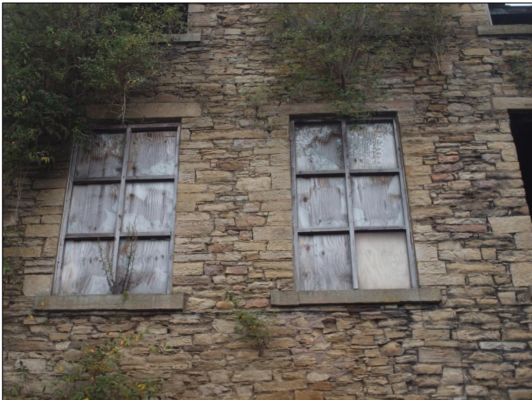
Plate 6: Detail of first floor windows
