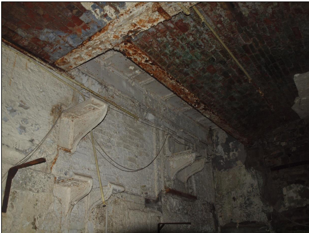
Plate 38: Hatch in ceiling above transmission window
