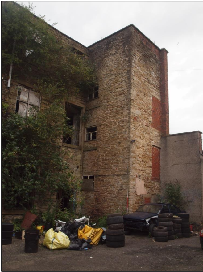
Plate 9: North end of elevation showing stair tower
