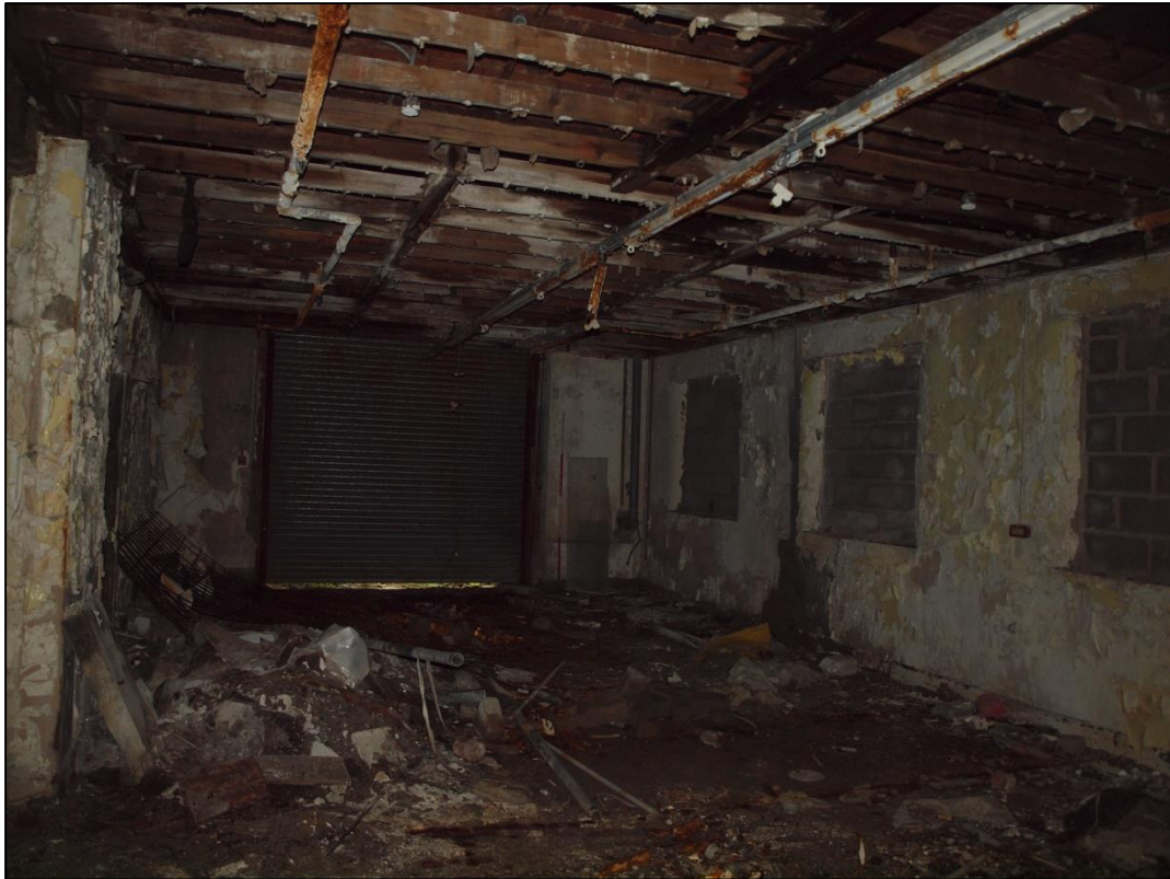
Plate 27: Southwestern end of ground floor
