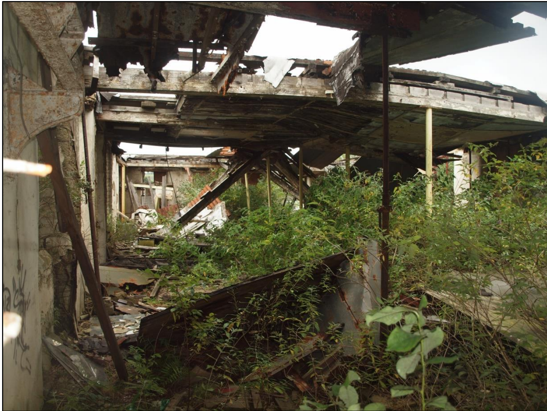
Plate 47: Second floor looking southwest from stair tower
