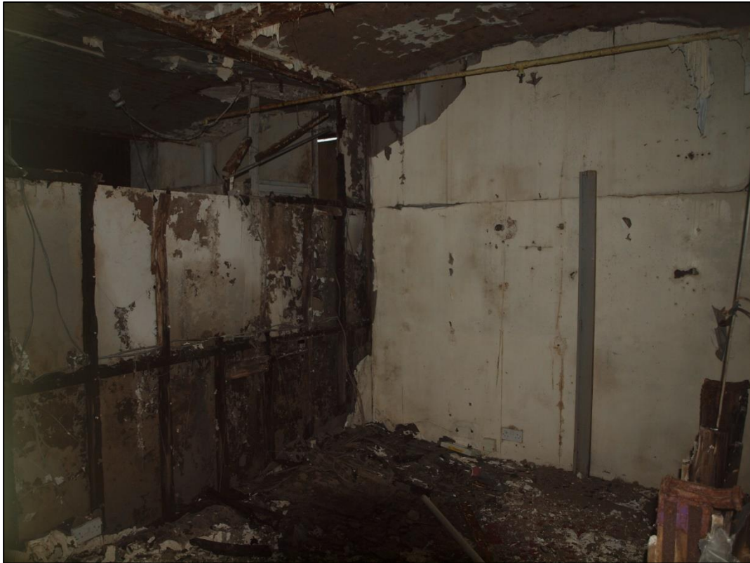
Plate 45: Detail of office interior
