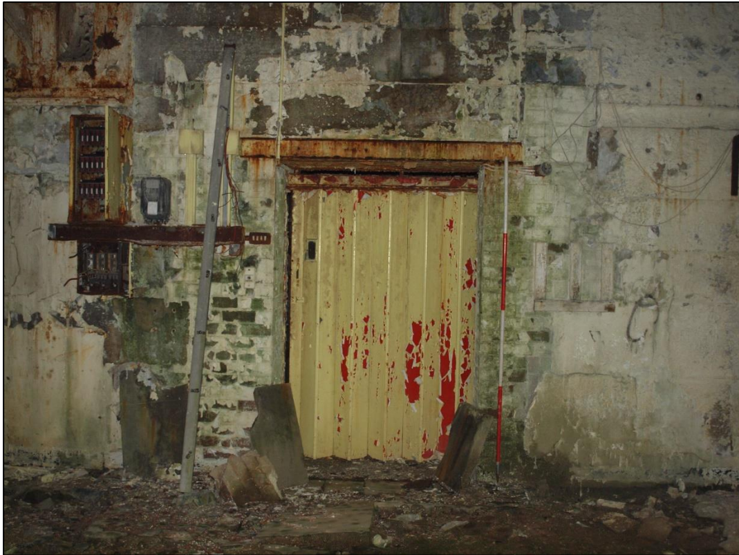
Plate 41: Inserted lift shaft
