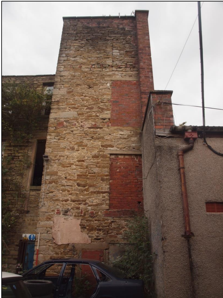
Plate 14: Blocked doorways at upper floors of stair tower
