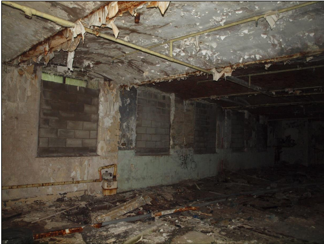
Plate 21: Blocked windows in ground floor
