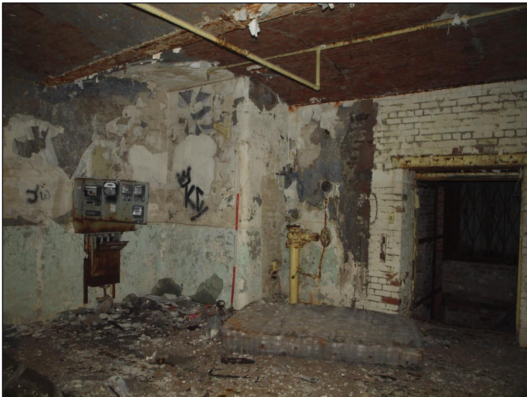
Plate 22: Northern corner of ground floor showing inserted lift shaft
