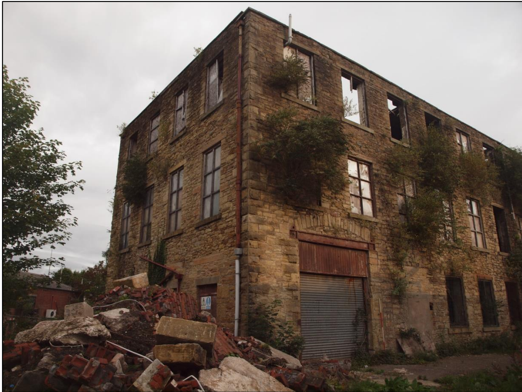
Plate 15: Southwest elevation of mill
