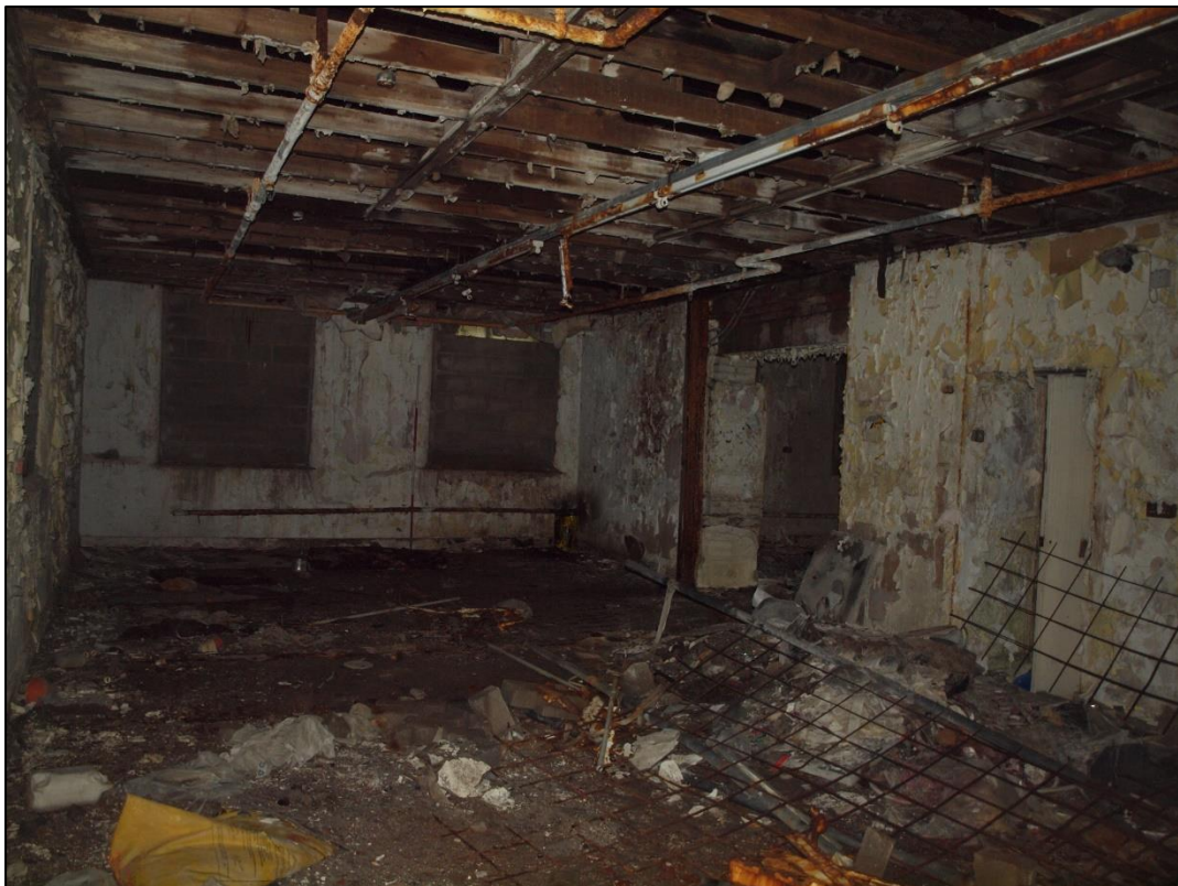
Plate 28: Southwestern end of ground floor
