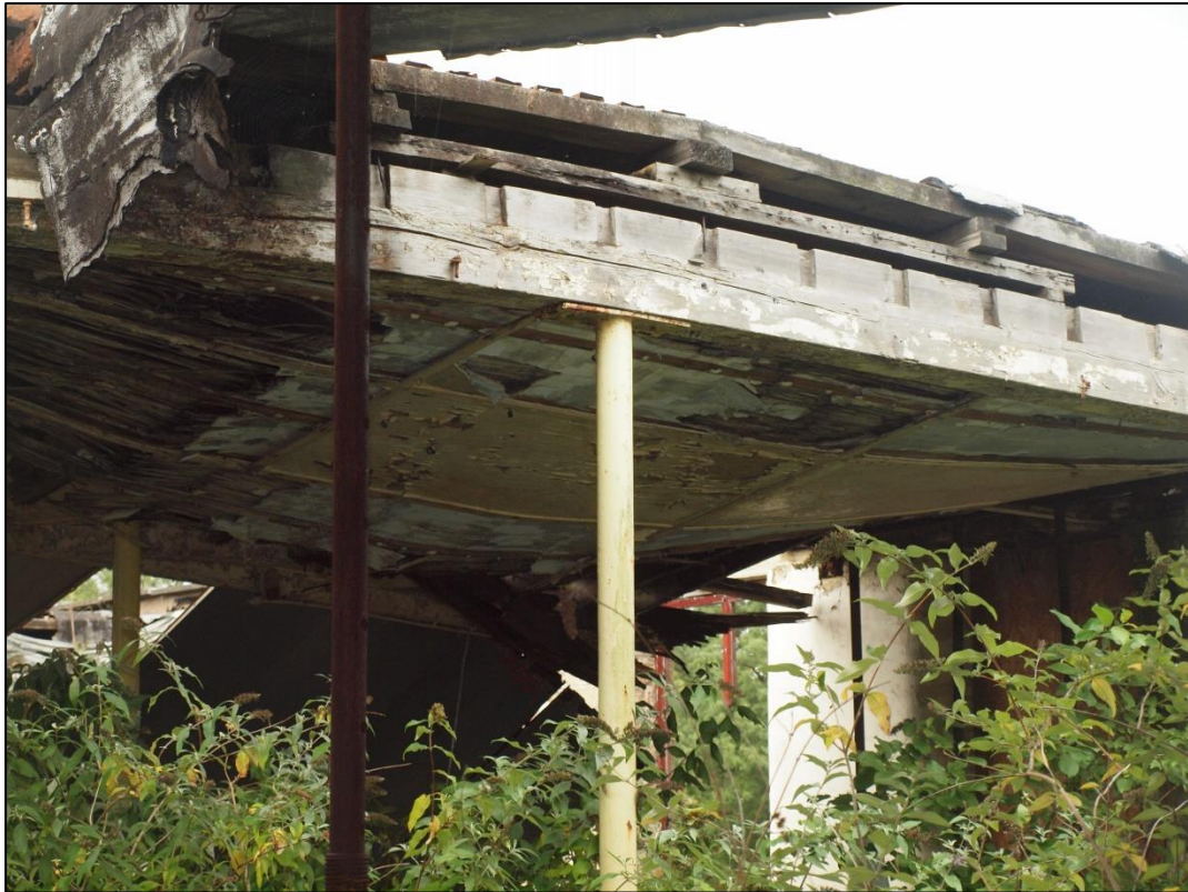
Plate 51: Detail of second floor stanchion
