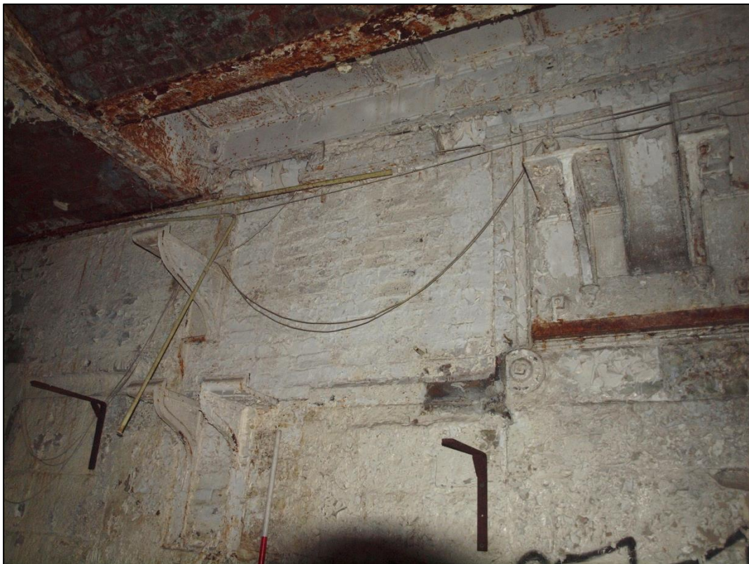
Plate 36: As above showing brackets and wheel slot to the right
