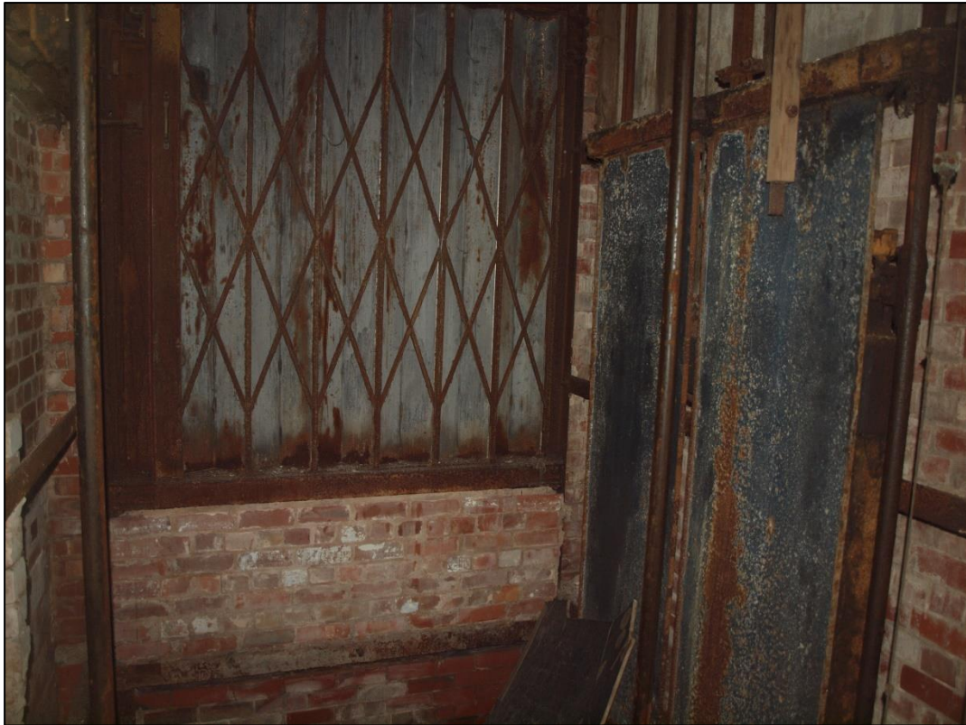
Plate 23: Interior of lift shaft
