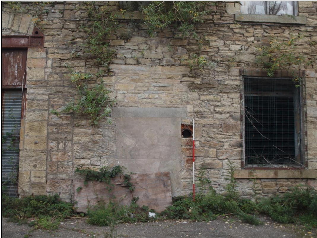
Plate 5: Blocked doorway to bay 3
