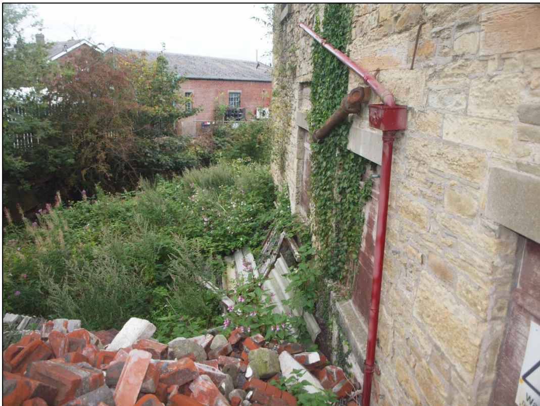
Plate 16: Windows and stonework of southwest elevation
