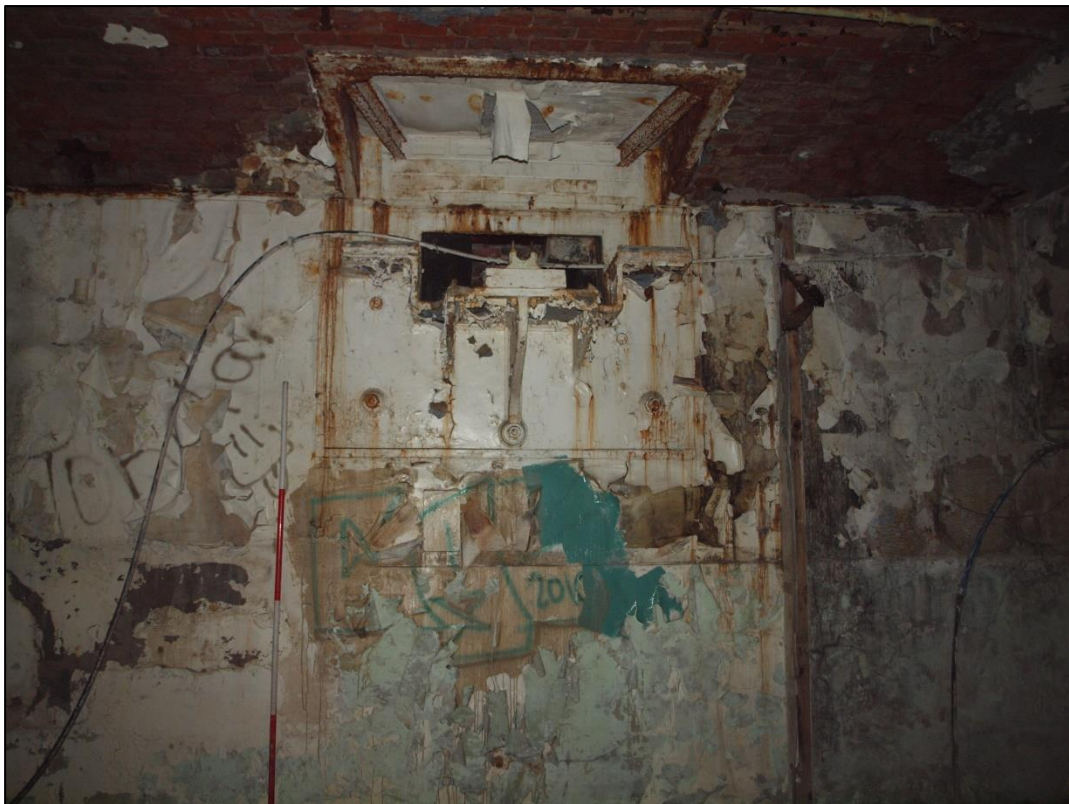
Plate 24: Transmission window in northeast wall
