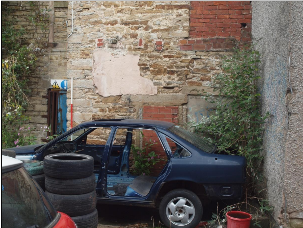
Plate 13: Ground floor of stair tower showing blocked doorway and window
