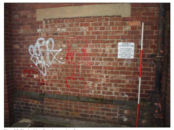
Plate 20: Blocked loading door to bay 6
