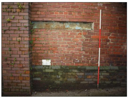
Plate 23: Blocked loading door to bay 9
