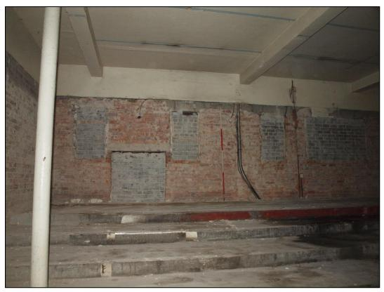
Plate 35: North wall of first floor showing blocked openings
