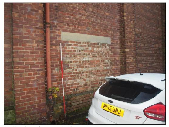
Plate 6: Blocked loading door to bay 6
