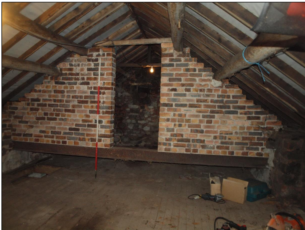
Plate 58: Modern supporting wall on beam supporting roof
