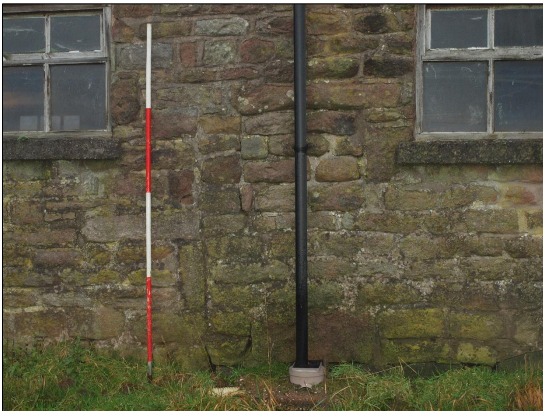
Plate 26: Detail of blocked doorway
