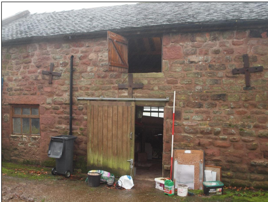
Plate 10: Doorway to bay 2 with pitching eye over
