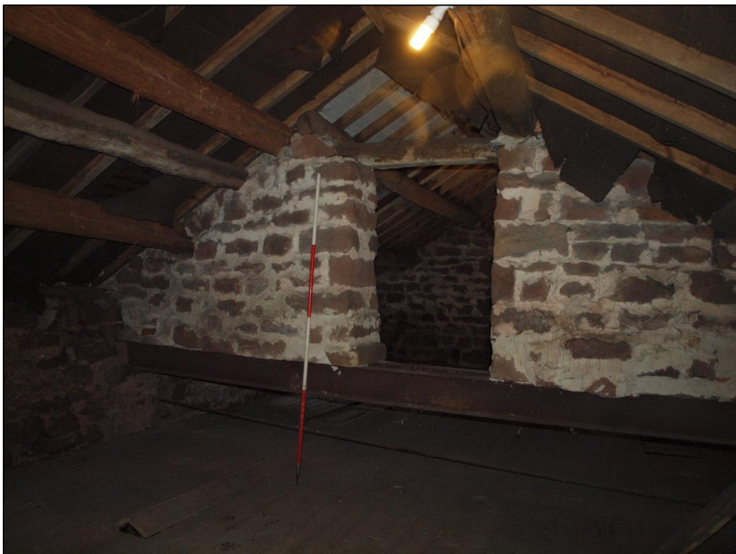
Plate 48: East end of first floor showing inserted beam carrying the remains of former cross wall
