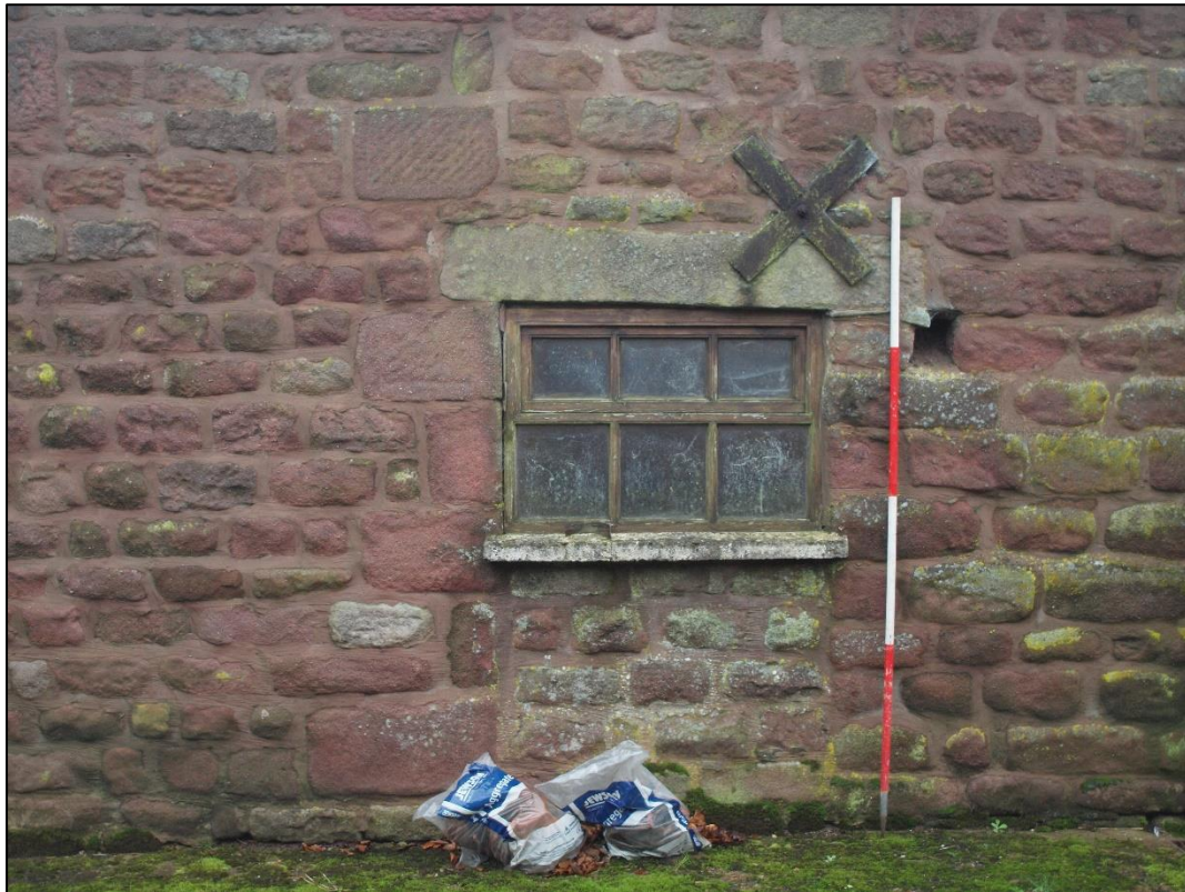
Plate 13: Detail of window with blocking below
