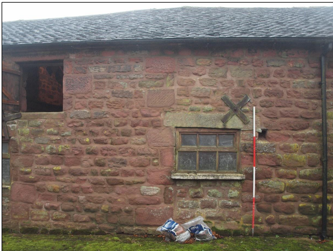
Plate 12: Straight joint between bays 3 and 4 with window to bay 4
