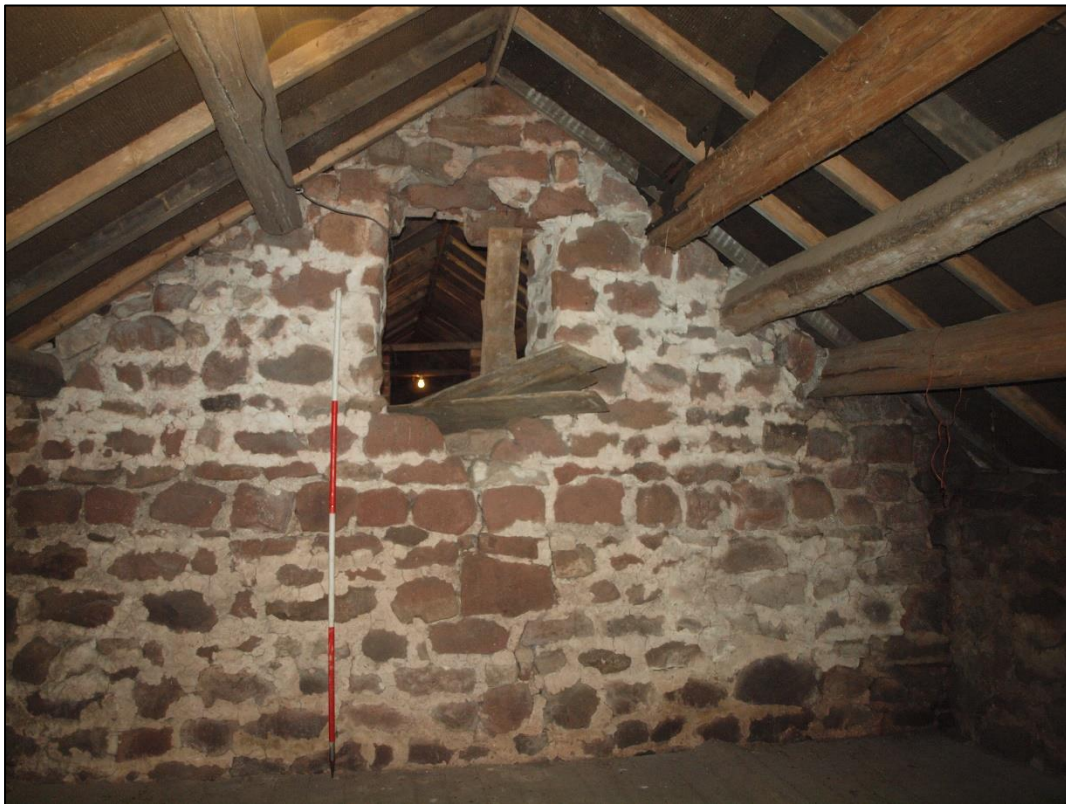
Plate 56: Former end gable wall with pitching eye to bay 4
