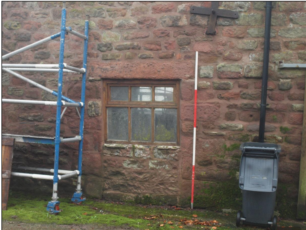
Plate 9: Detail of above showing blocking beneath
