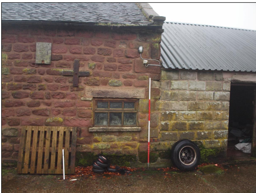
Plate 16: Detail of window with blocking below
