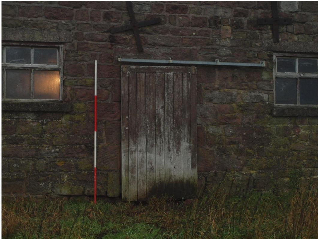
Plate 27: Doorway to bay 3
