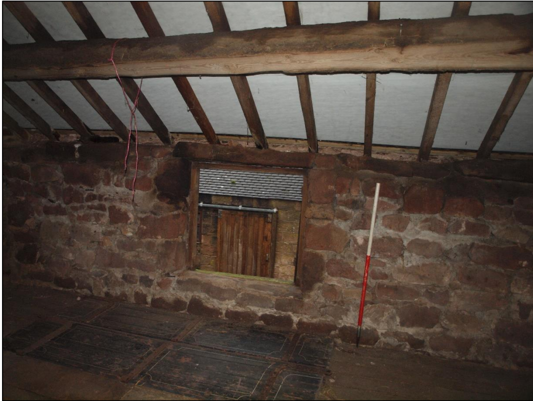
Plate 55: Pitching eye to north elevation from the inside
