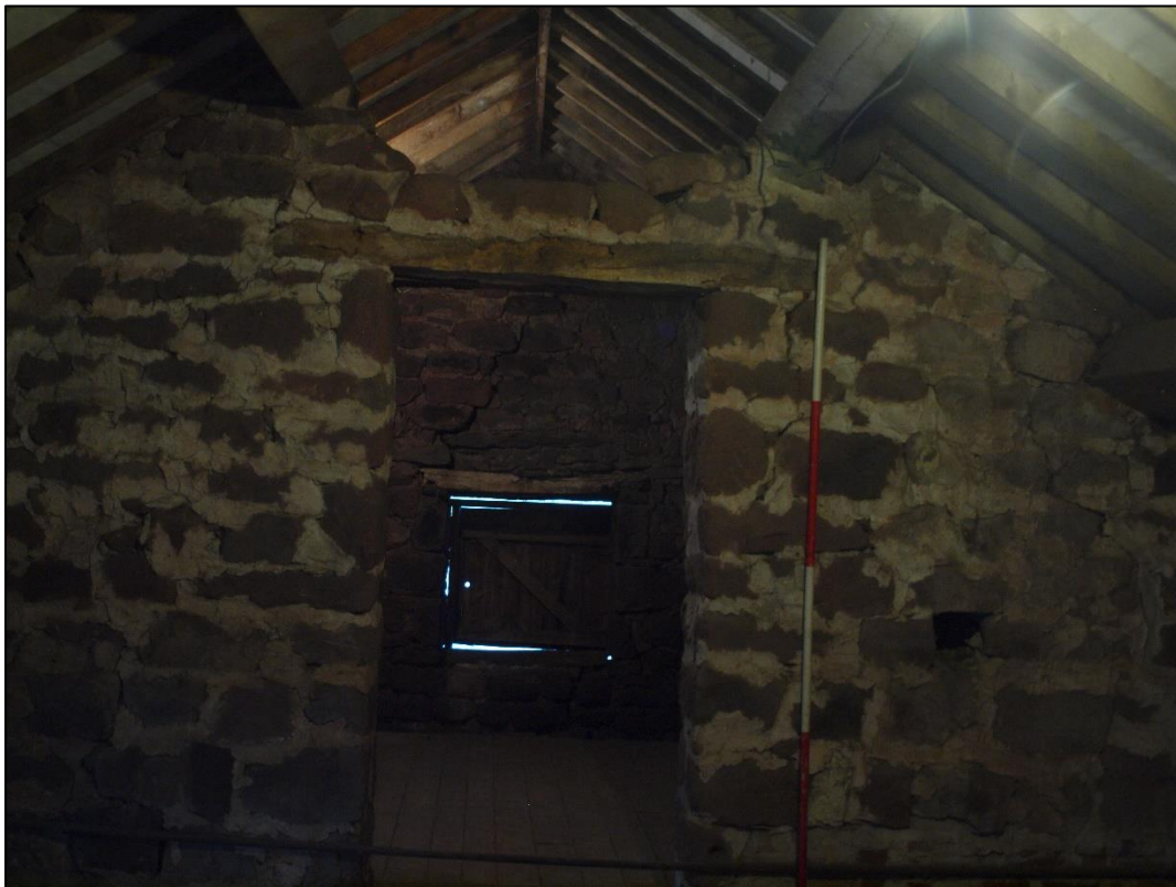
Plate 52: Detail of doorway
