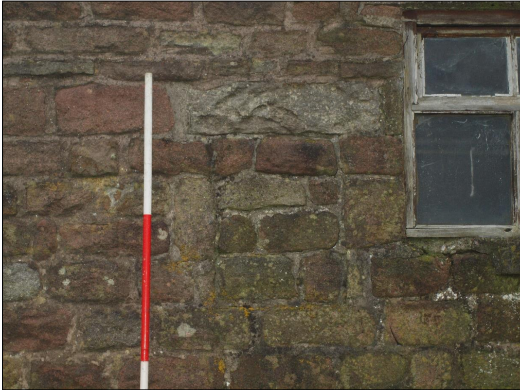
Plate 23: Detail of small blocked window to bay 1
