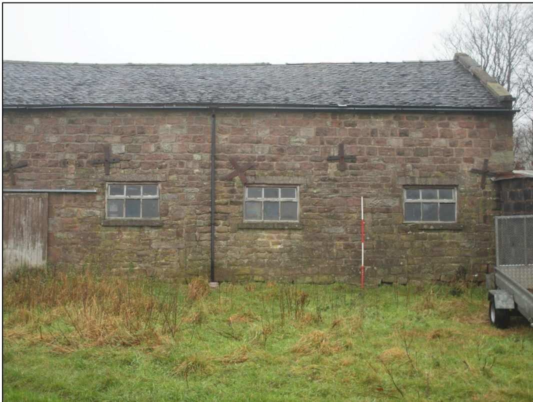
Plate 22: Inserted windows to bays 1 and 2
