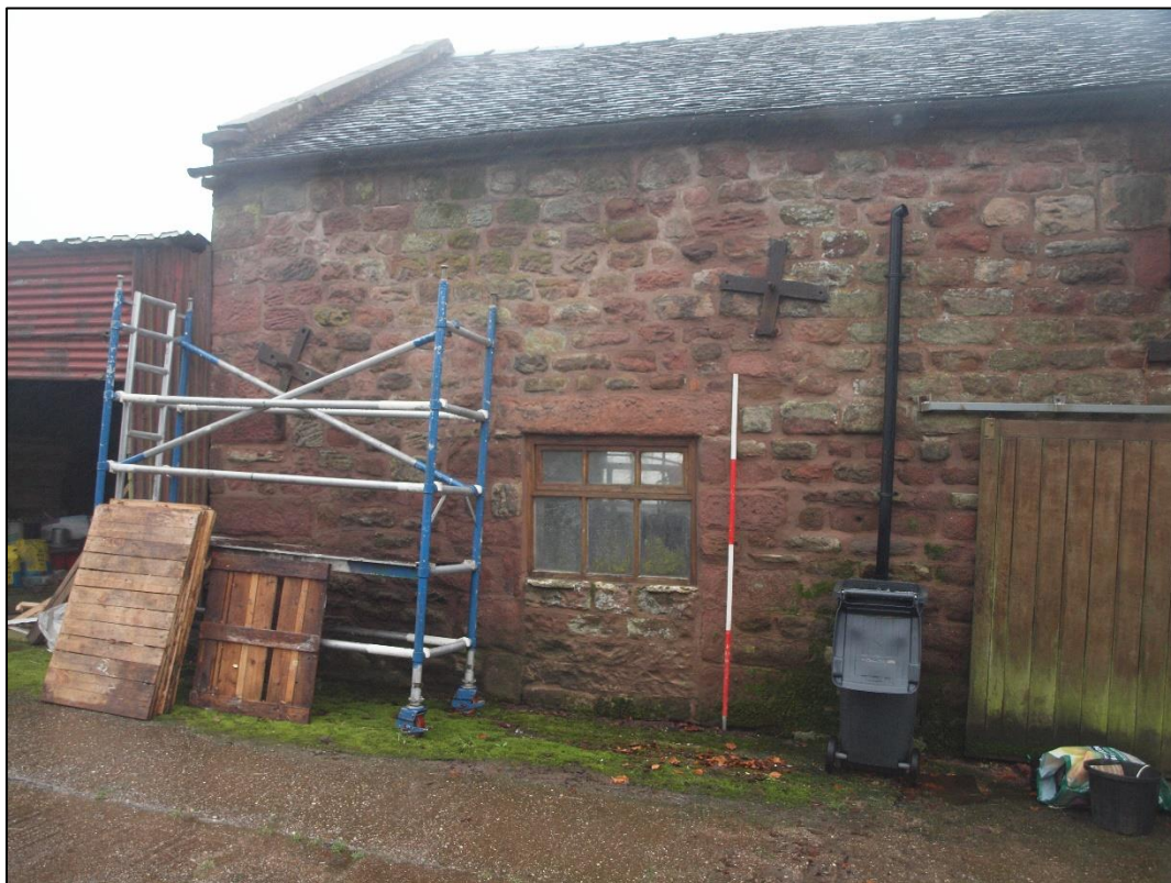
Plate 8: Window to bay 1
