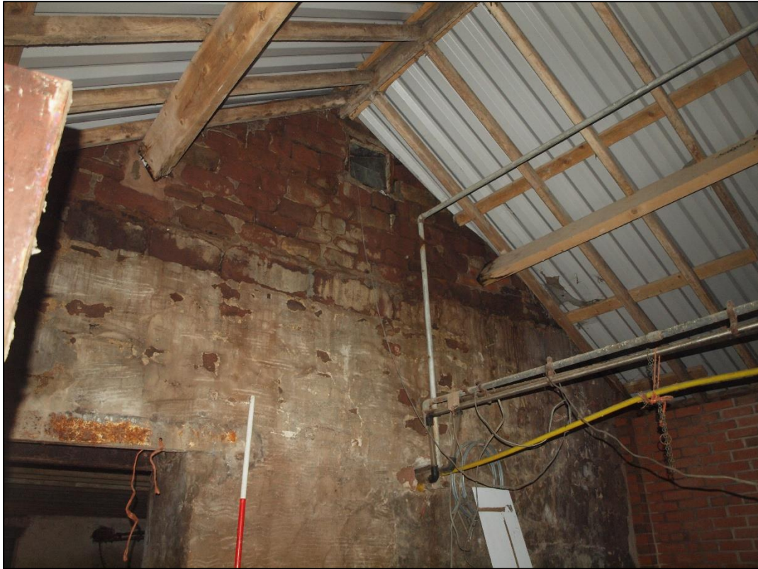
Plate 19: As above showing small window to first floor
