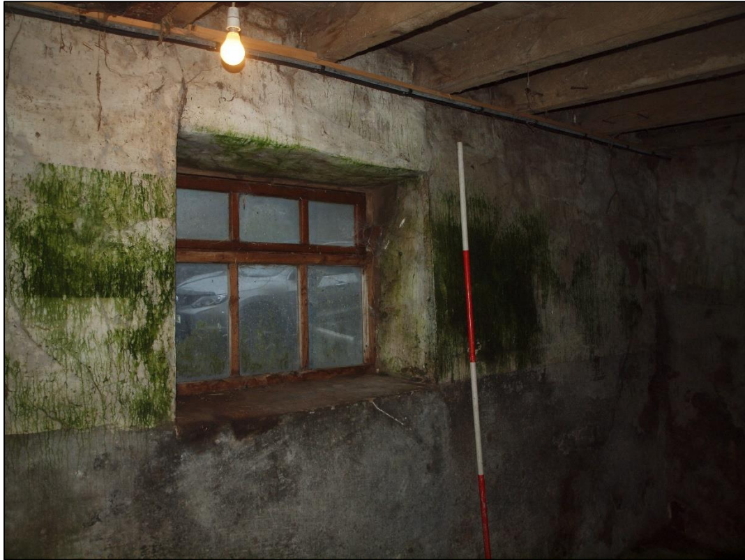
Plate 39: Detail of inserted window to north wall
