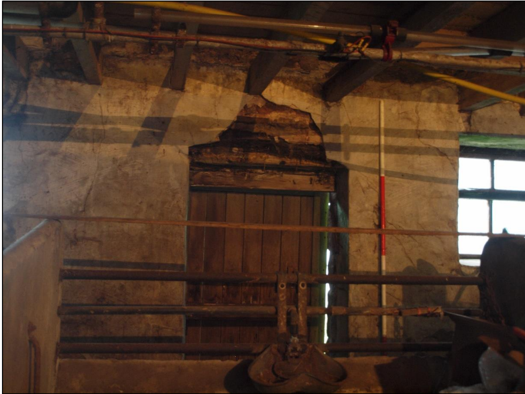
Plate 45: Doorway in south wall to bay 2
