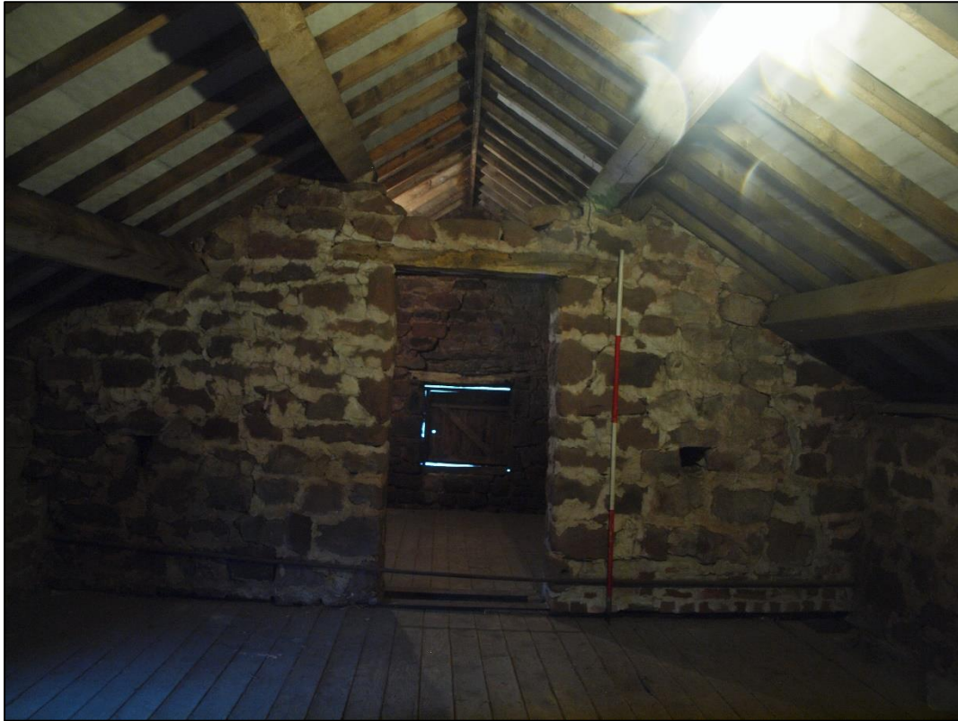
Plate 51: Surviving cross wall at first floor level between bays 1 and 2
