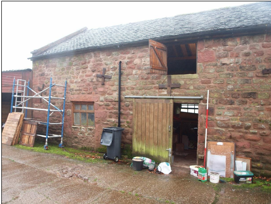
Plate 7: East end of north elevation showing bays 1 and 2
