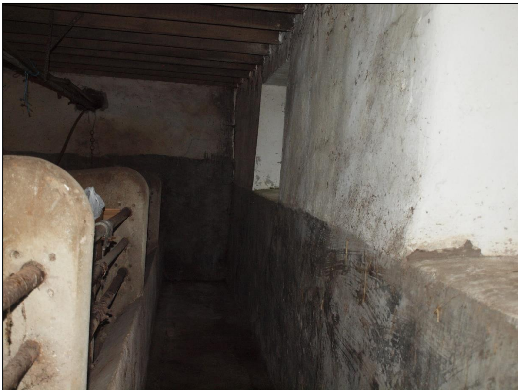
Plate 42: View down feeding passage in west extension
