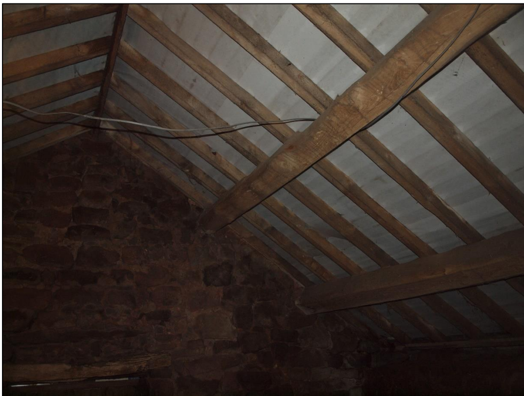
Plate 54: Purlins to bay 1
