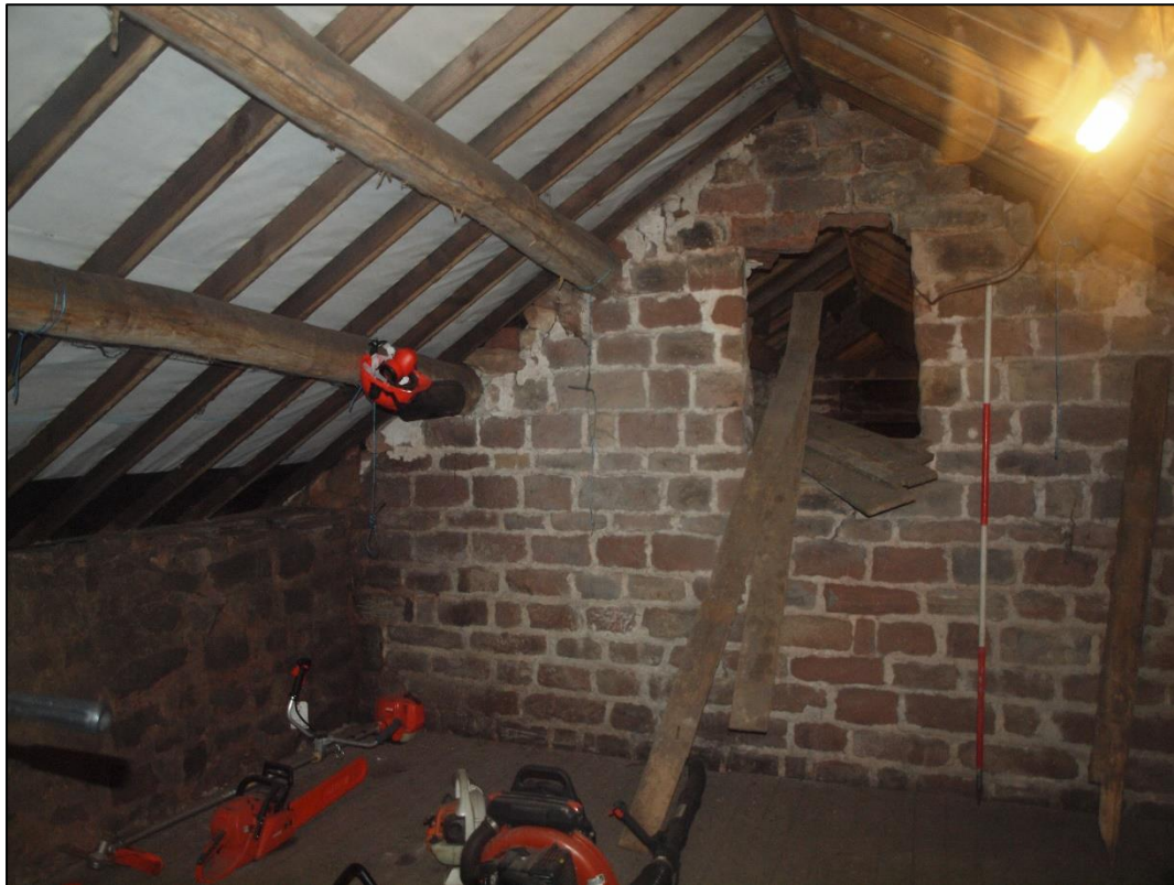
Plate 57: As above from bay 4 in west extension
