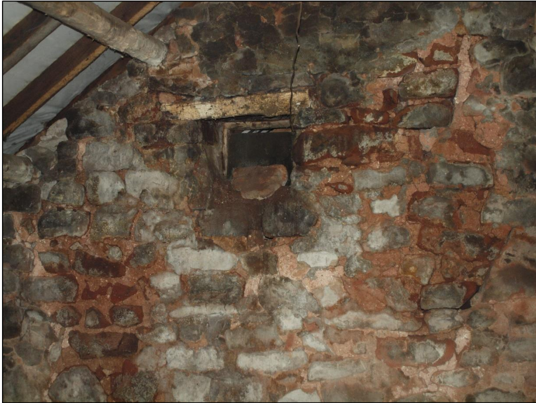
Plate 61: Detail of window above
