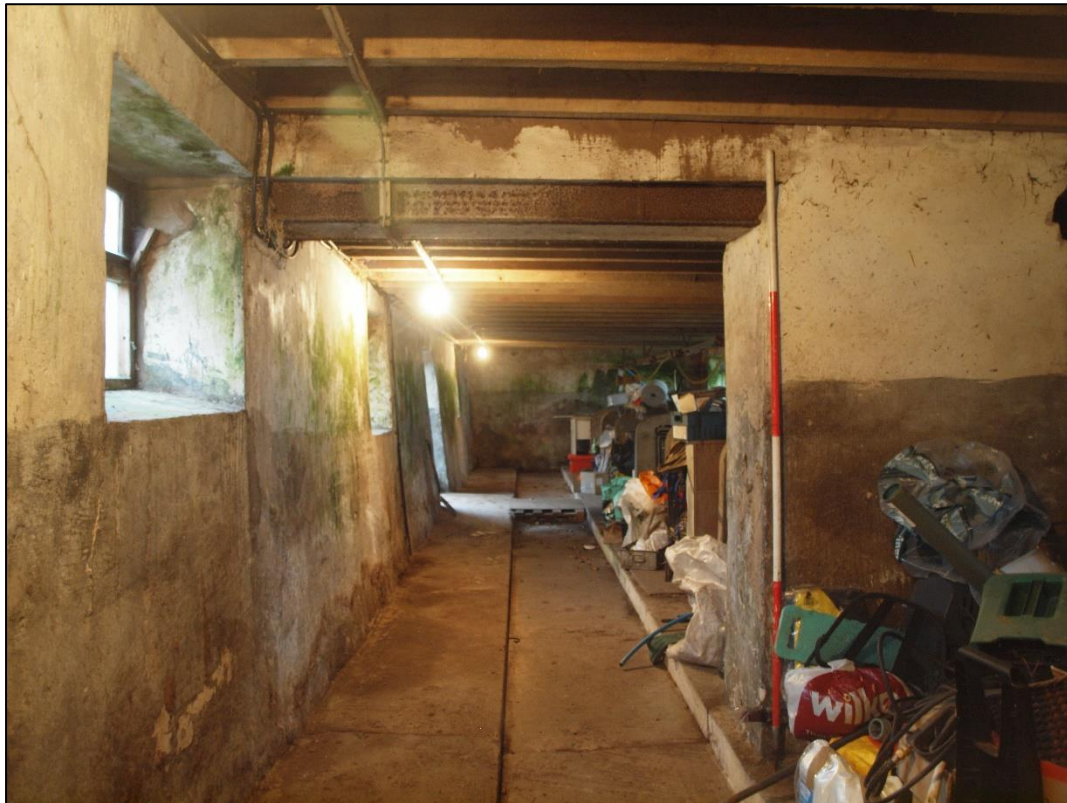
Plate 37: Inserted opening in cross wall
