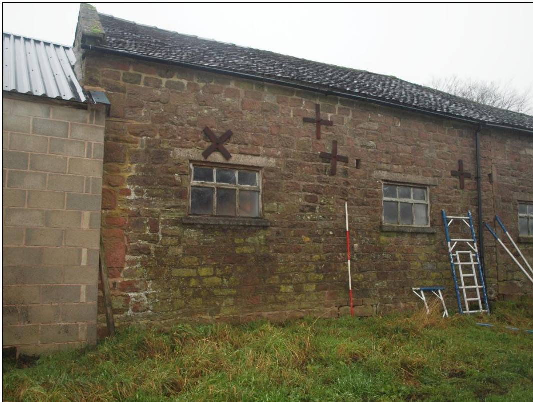
Plate 30: Western extension, bays 4 and 5
