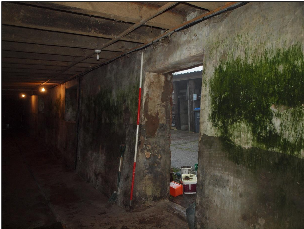
Plate 41: Detail of doorway to bay 2
