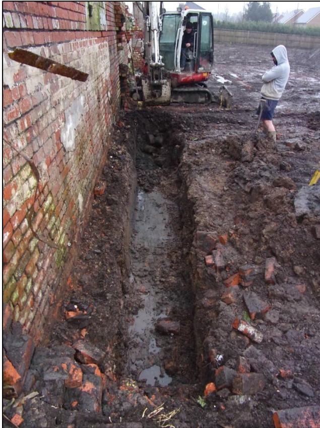
Plate 1: initial opening of wall foundation trench
