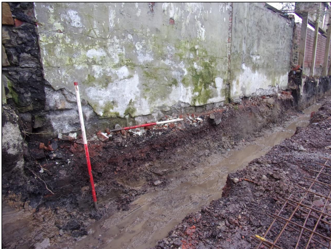
Plate 6: General shot of trench looking east
