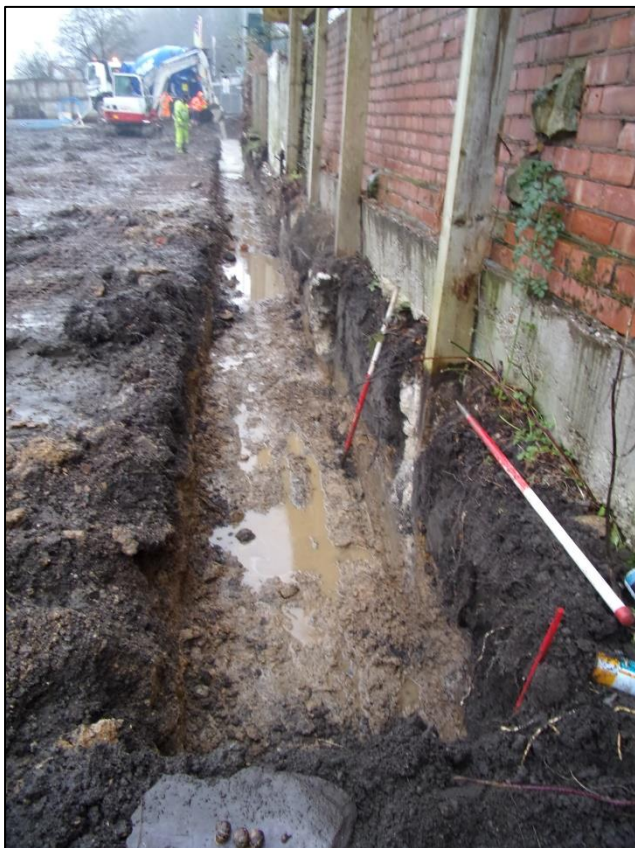
Plate 8: Completed trench looking west
