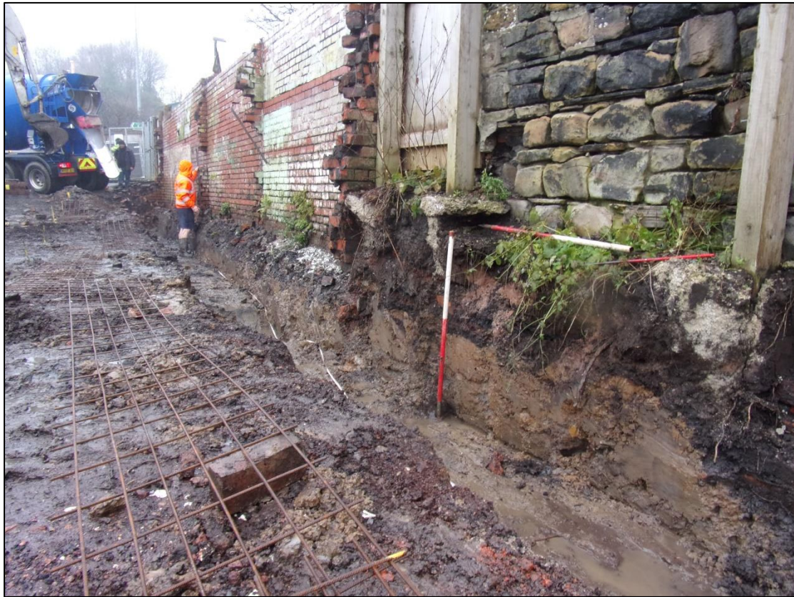
Plate 5: General shot of trench looking west
