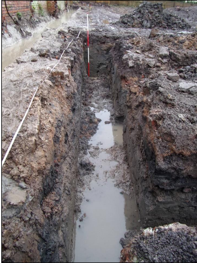
Plate 11: Norther trench looking east
