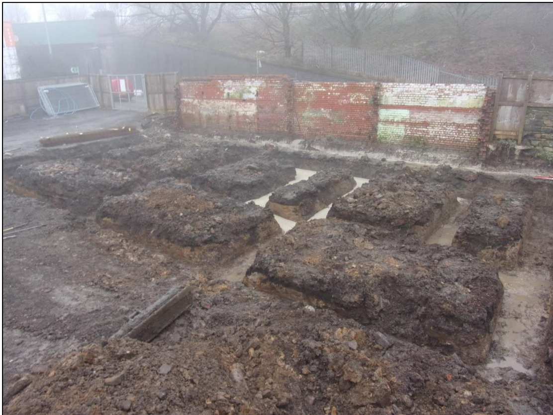
Plate 16: Plots 1-3 after excavation
