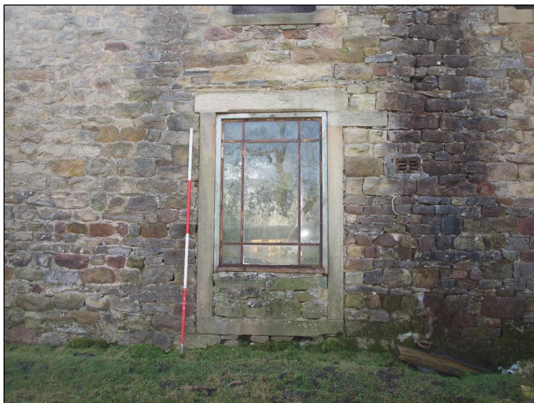
Plate 13: Former threshing door
