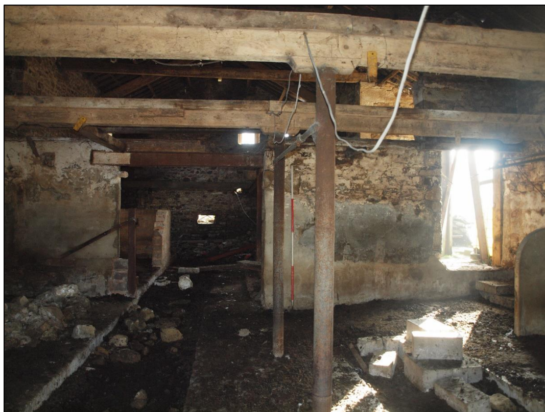
Plate 22: Interior from west end looking east
