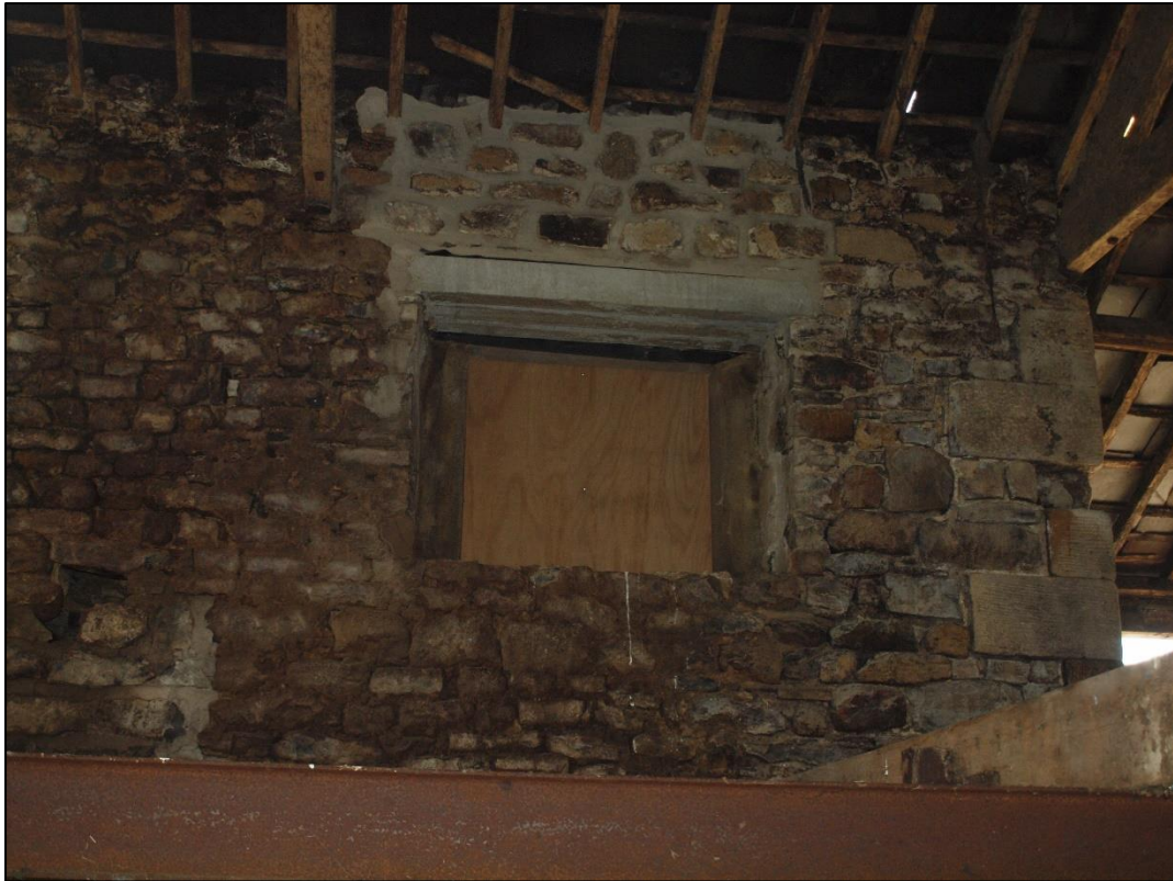
Plate 35: Detail of inserted first floor window above
