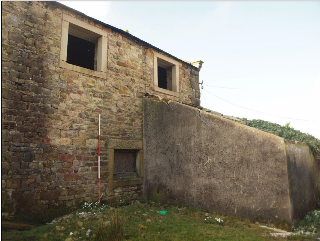
Plate 15: West end of north elevation
