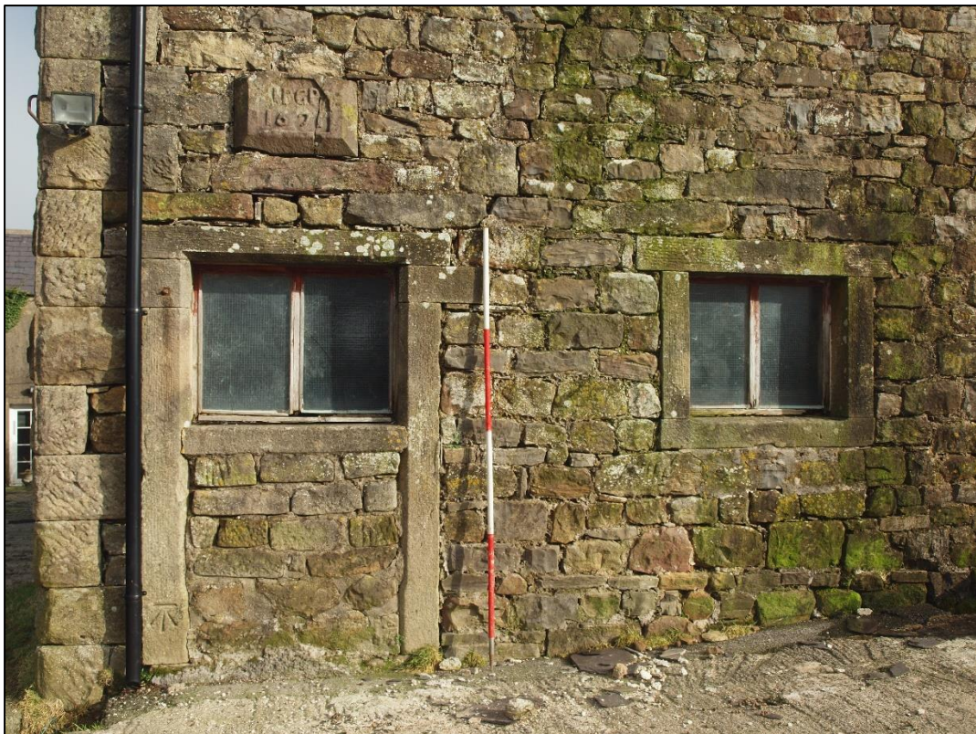
Plate 4: West end of south elevation
