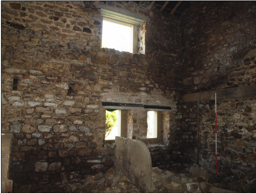
Plate 33: Inserted boskins and windows in north wall of eastern end
