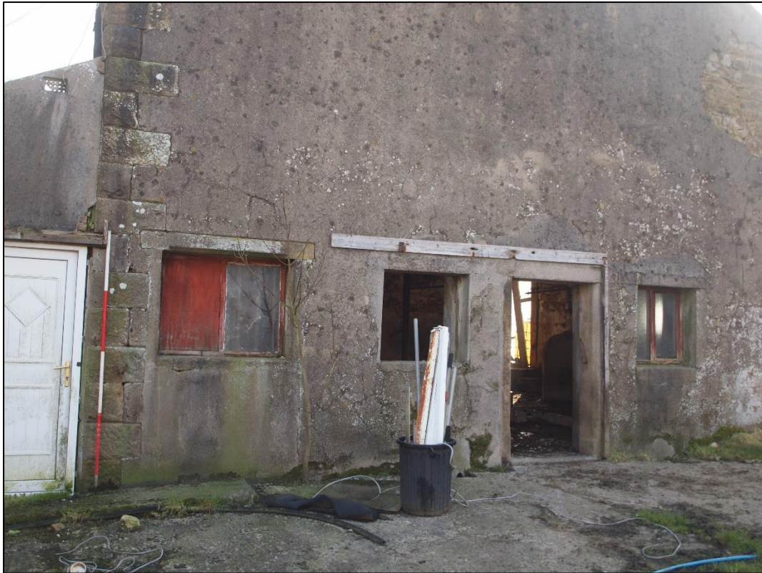
Plate 19: Ground floor openings in west elevation
