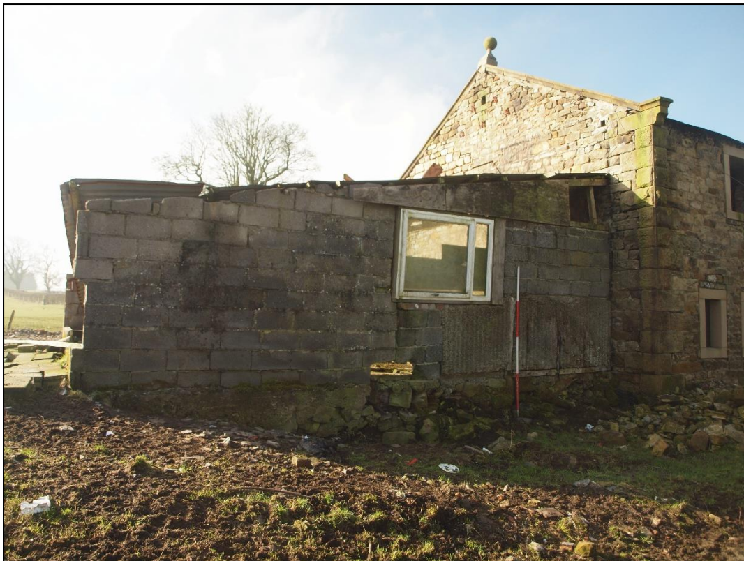
Plate 10: North elevation of eastern extension
