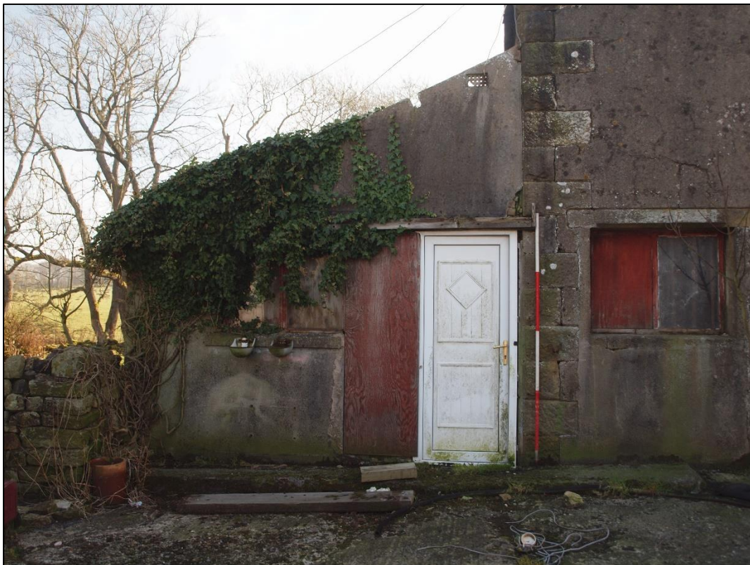
Plate 18: West elevation of modern extension
