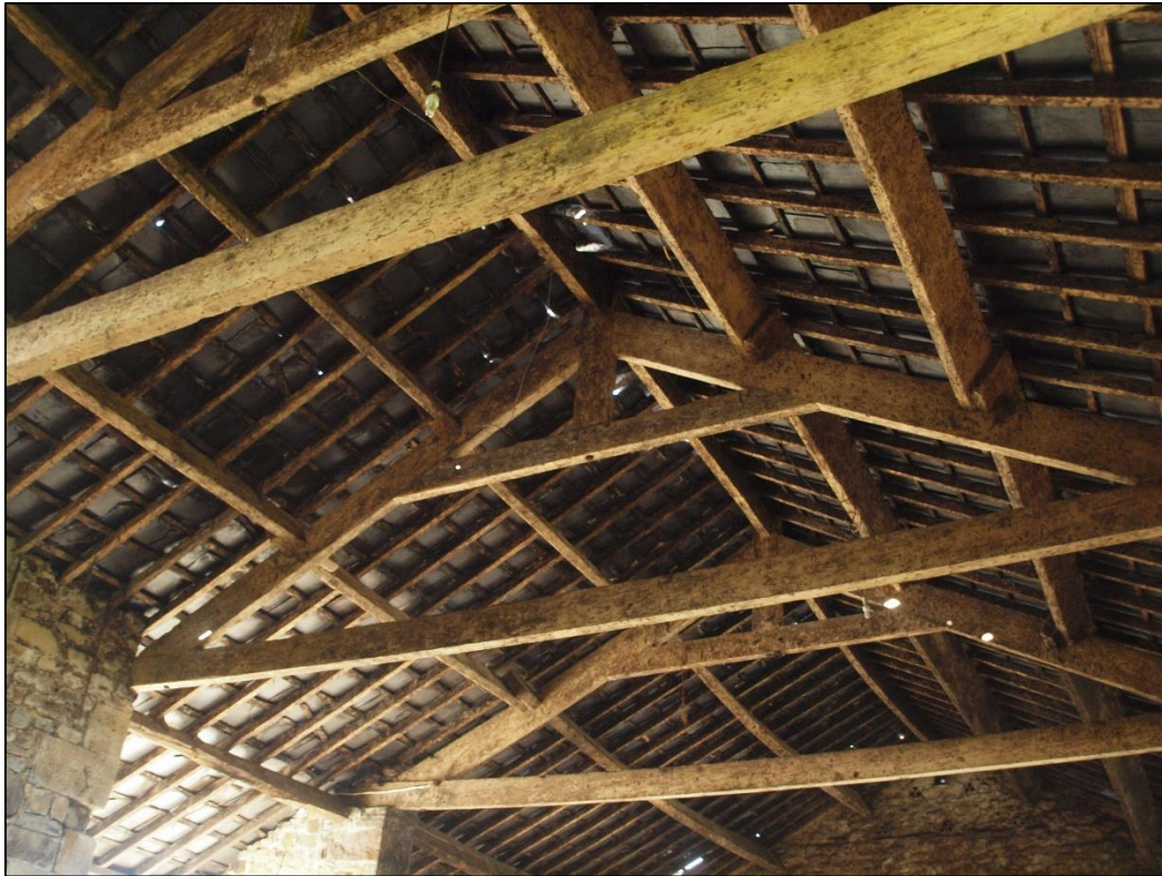
Plate 37: General shot of machine cut timber roof structure
