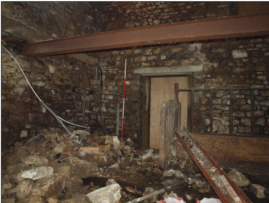
Plate 34: Inserted boskins and door in south wall of eastern end
