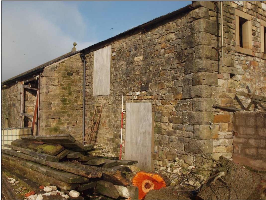
Plate 7: East end of south elevation
