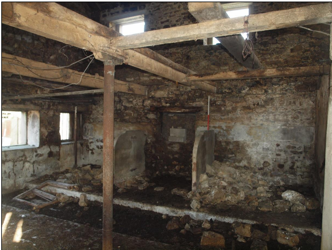
Plate 26: As above showing timber original window
