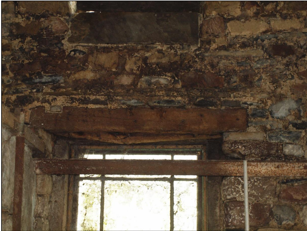
Plate 29: Detail of above showing hand cut timber lintel
