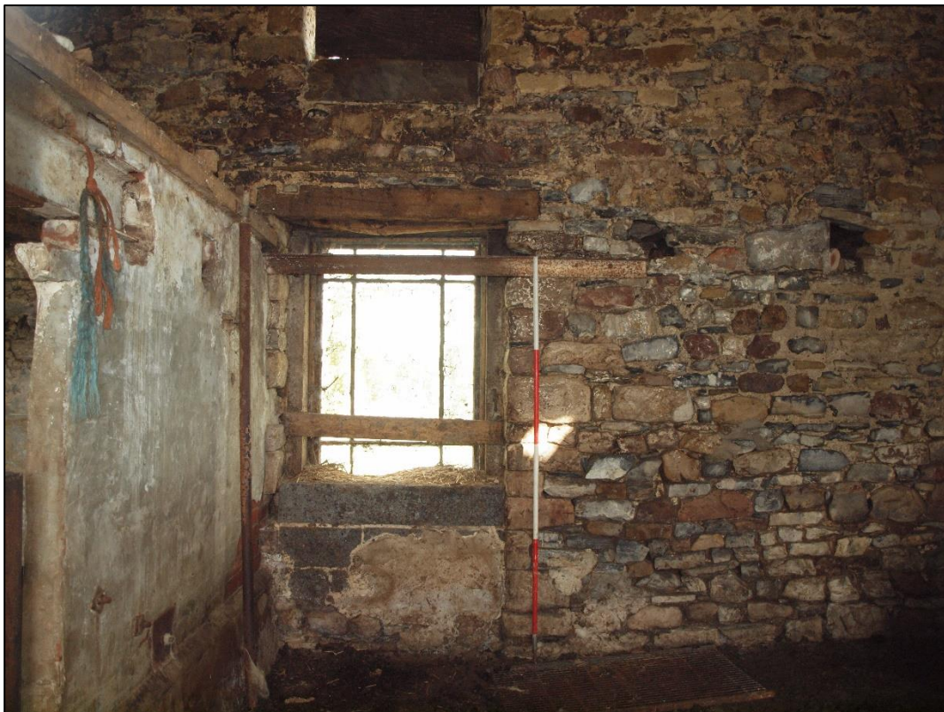
Plate 28: Former threshing door
