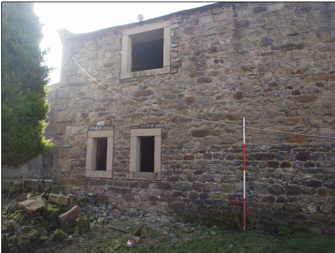
Plate 12: East end of north elevation showing inserted windows
