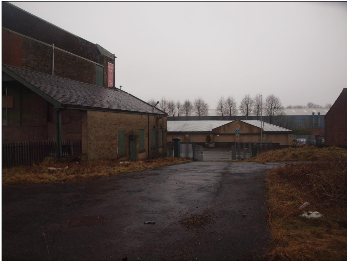
Plate 7: West side of Dale Mill looking south towards Dale Street
