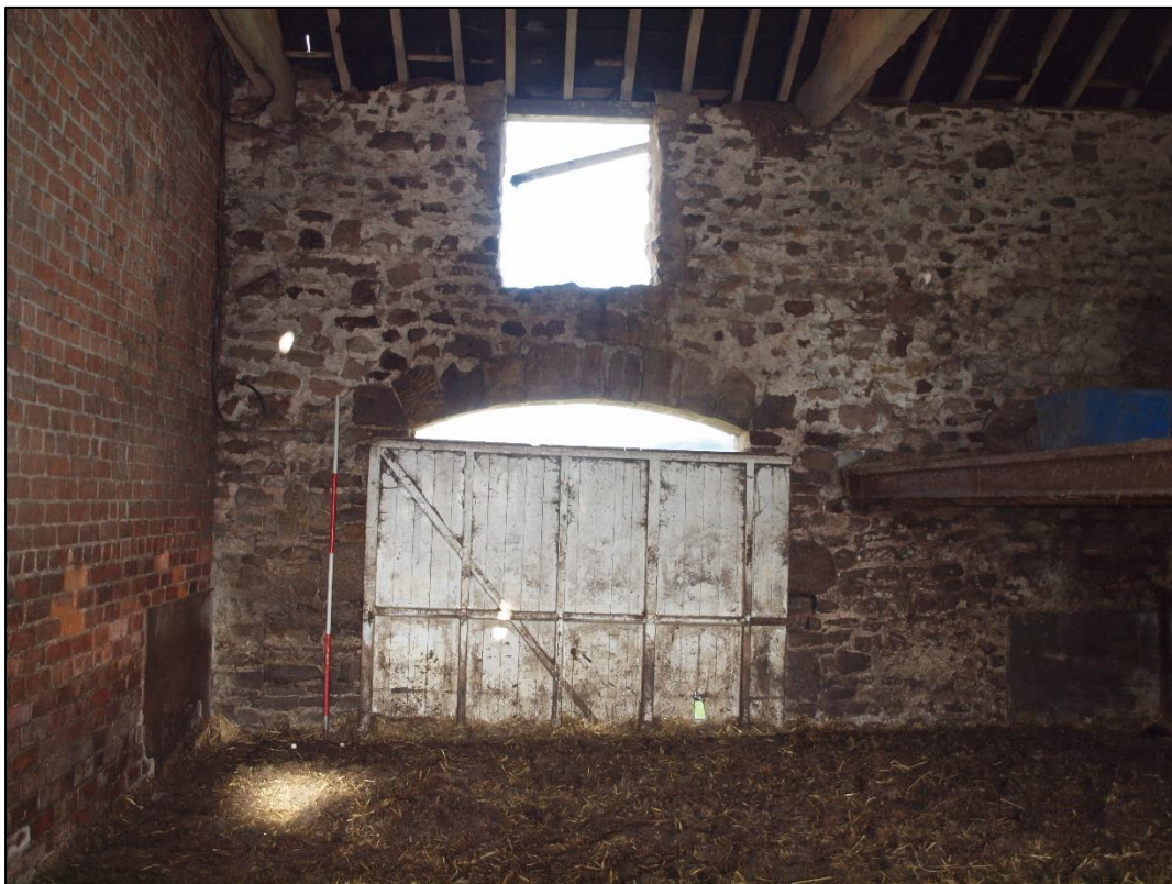
Plate 24: Barn door in northwest wall
