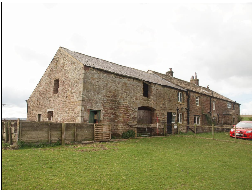
Plate 4: General shot of northwest elevation of whole building
