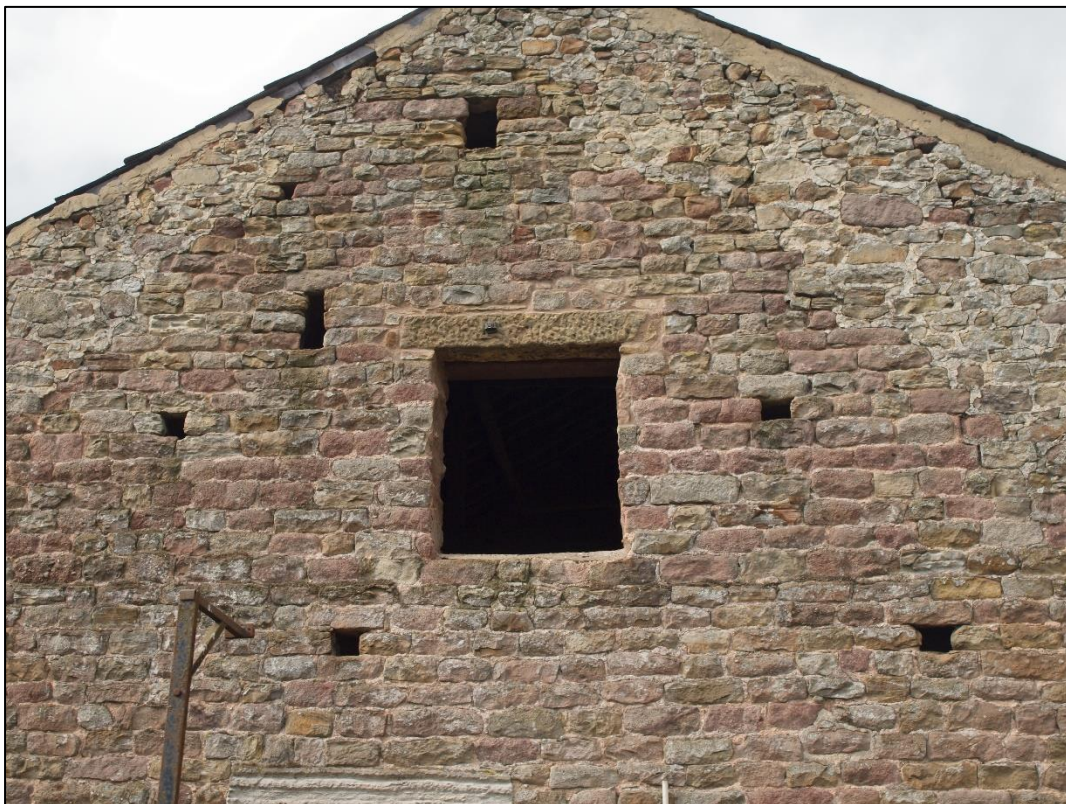
Plate 12: First floor pitching eye and differing stonework showing former roof pitch.
