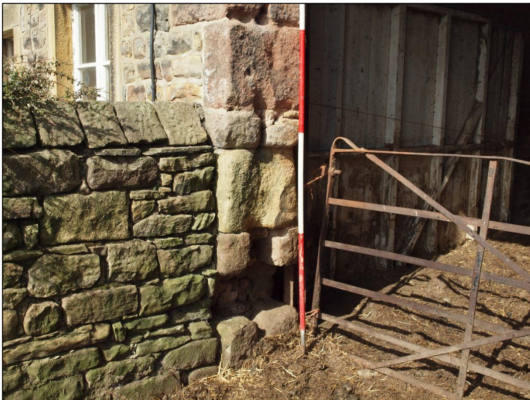
Plate 18: Slot for board in jamb
