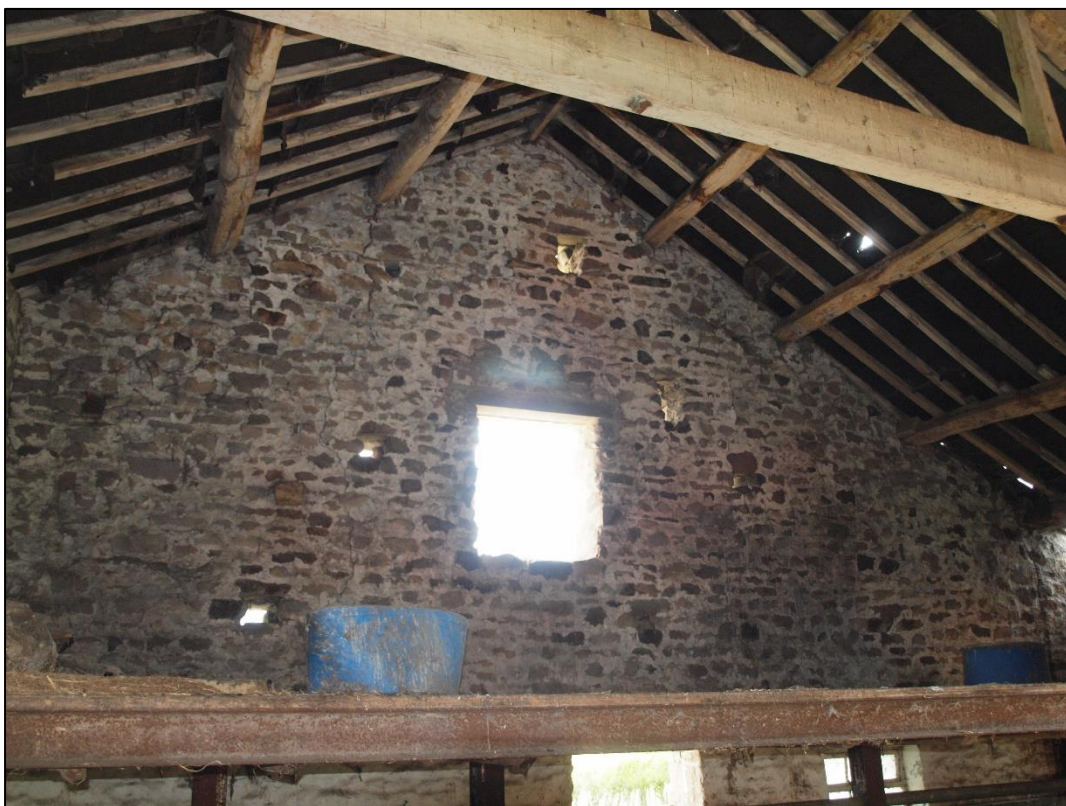
Plate 28: First floor looking northeast
