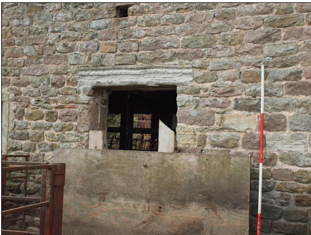
Plate 10: Ground floor doorway
