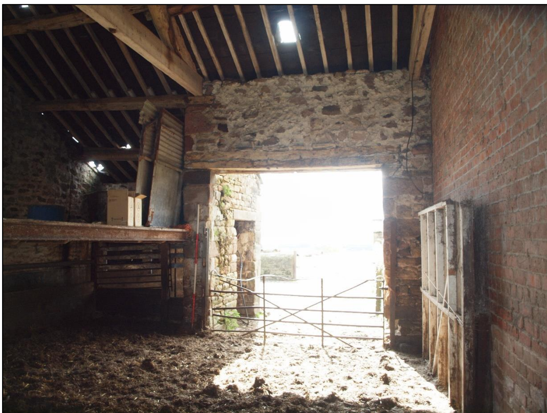
Plate 26: Barn door in southeast wall
