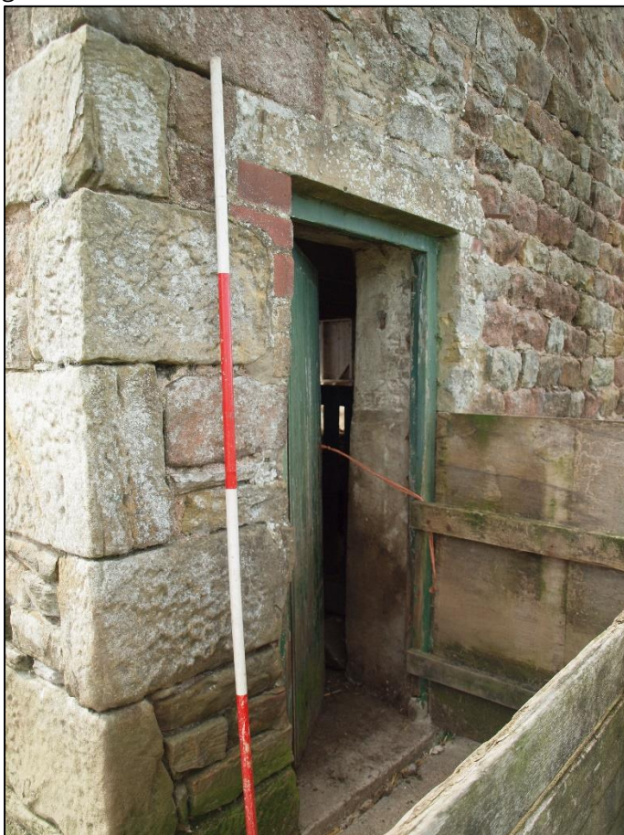
Plate 8: Inserted doorway to north side
