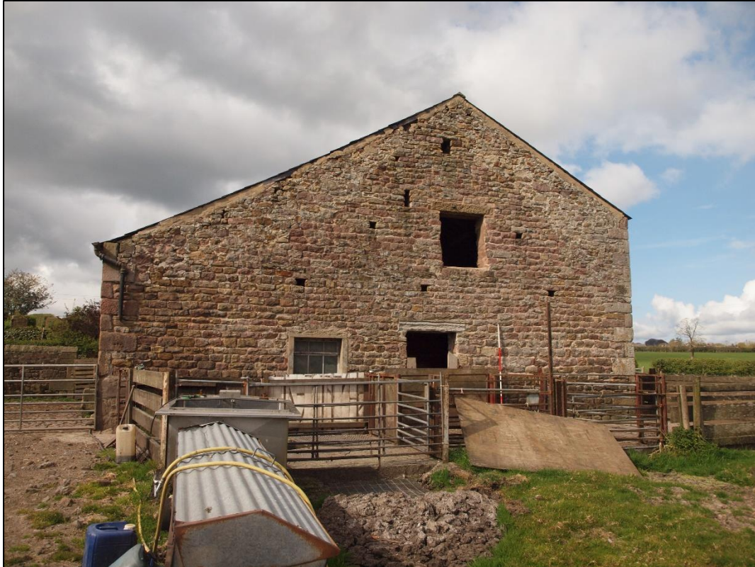
Plate 9: General shot of northeast gable
