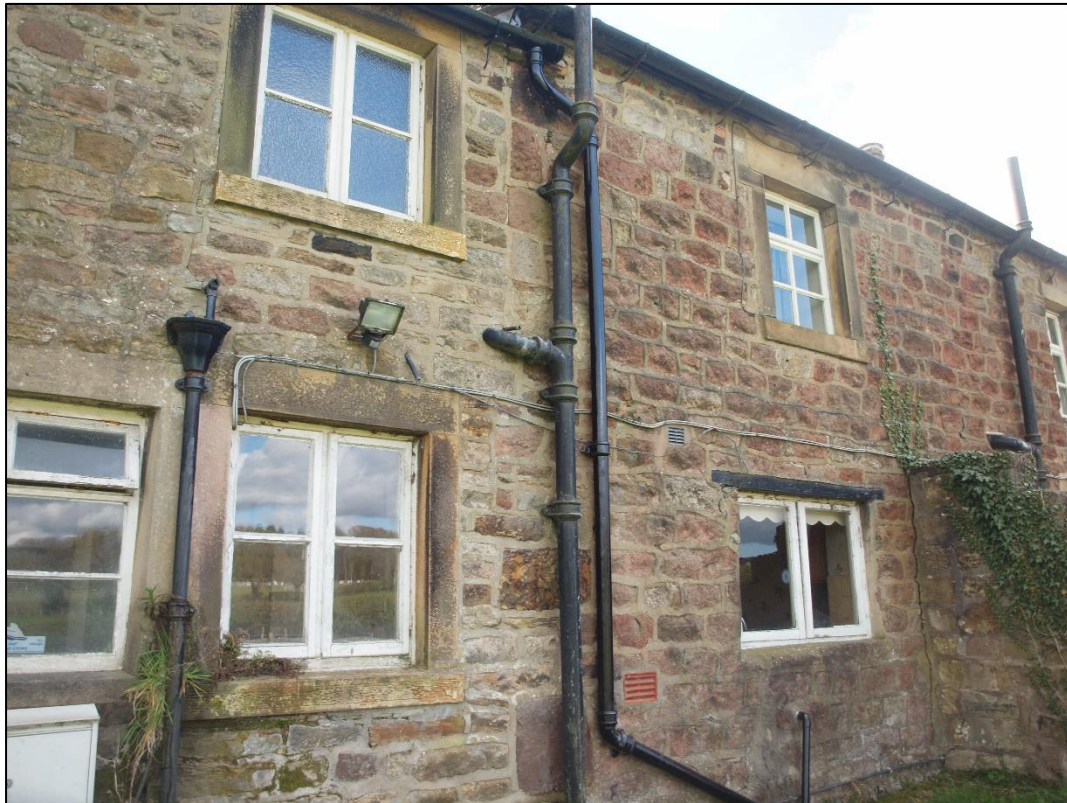
Plate 3: Junction between barn (left) and house (right) showing quoins to the house
