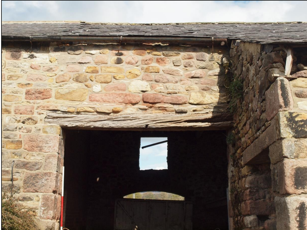
Plate 17: Detail of timber lintel
