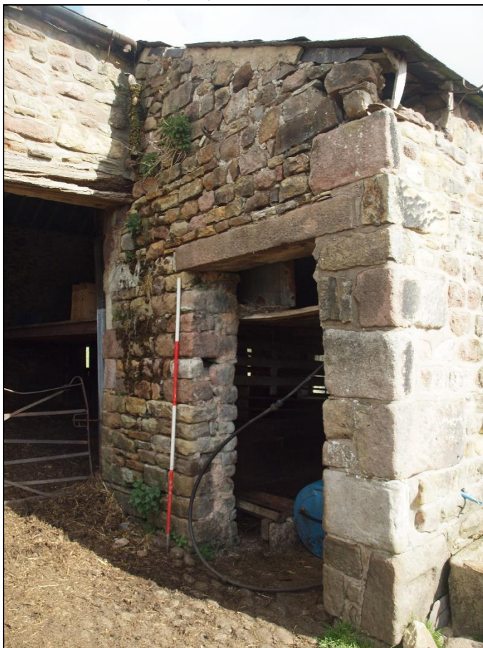
Plate 20: Southwest elevation of lean-to
