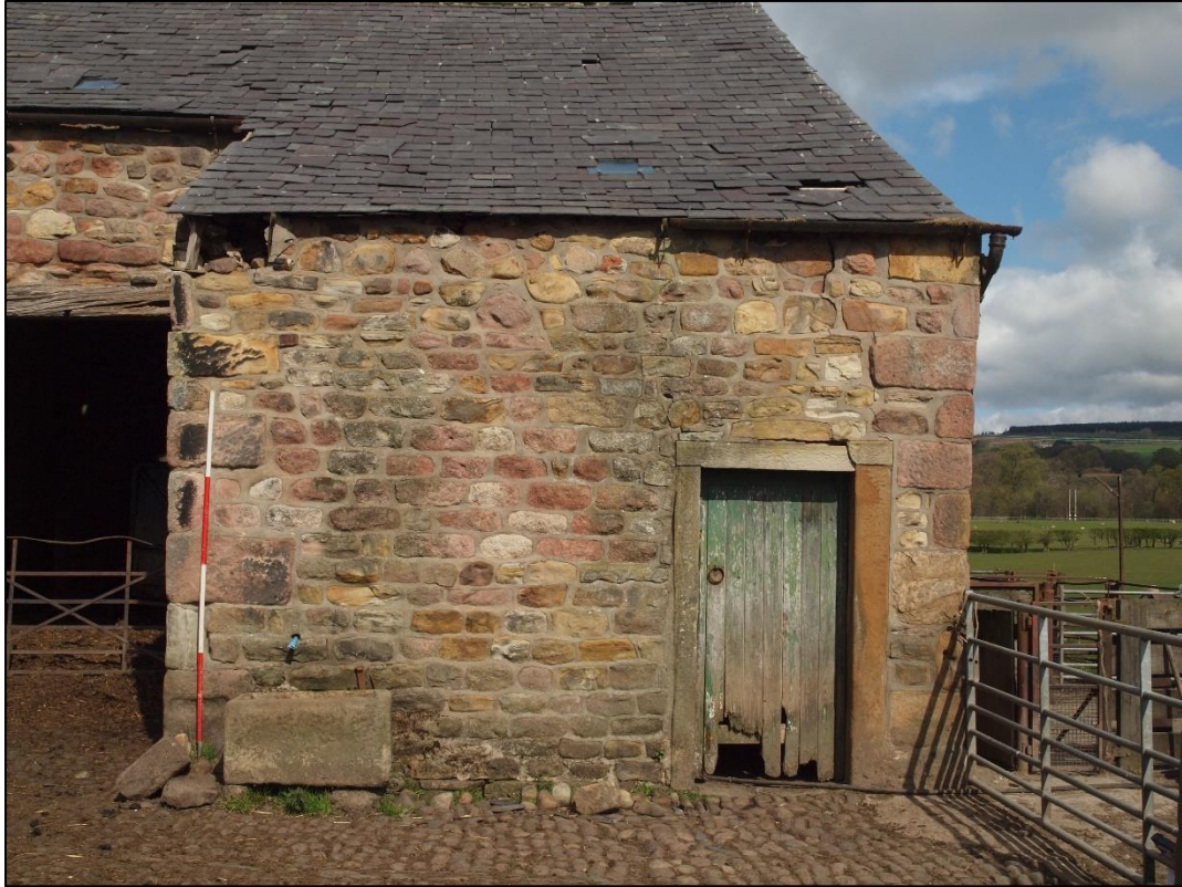
Plate 15: Detail of lean-to
