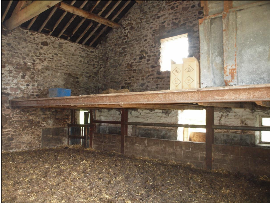
Plate 23: General interior shot looking north
