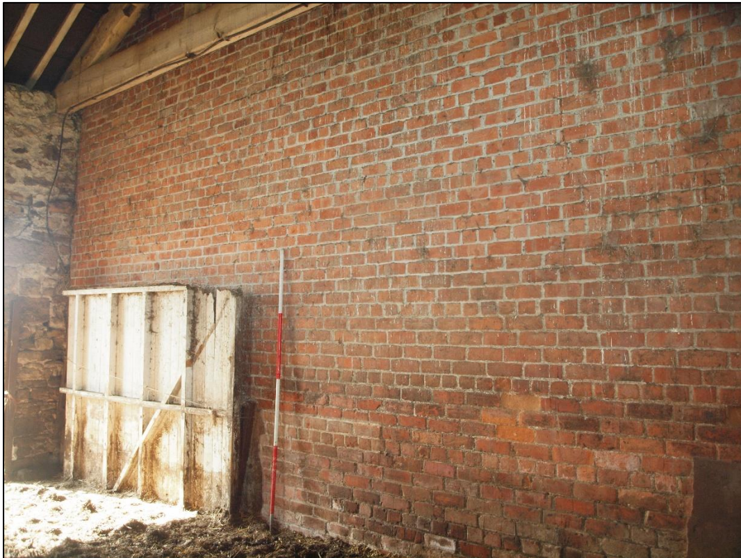
Plate 27: Inserted brick wall to southwest
