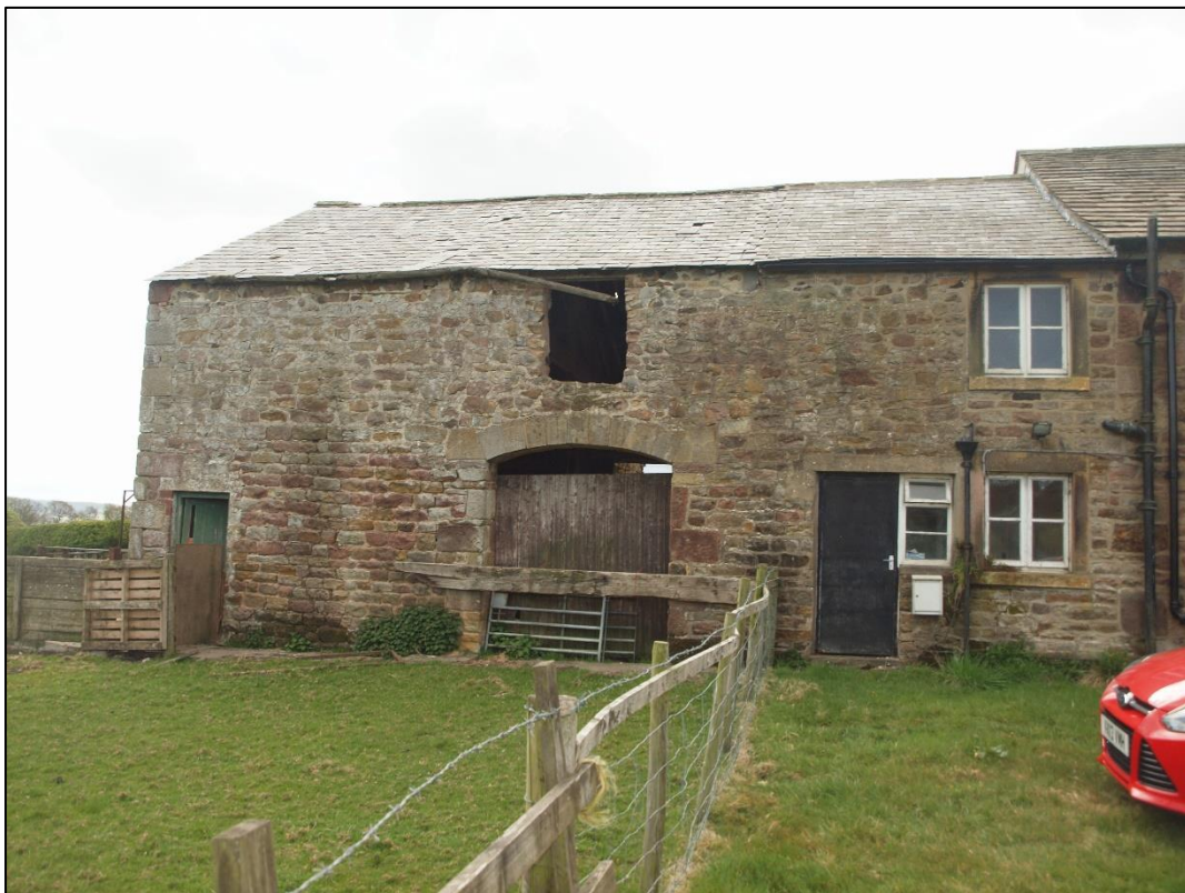
Plate 6: Northwest elevation of barn. Fence marks the boundary of the survey
