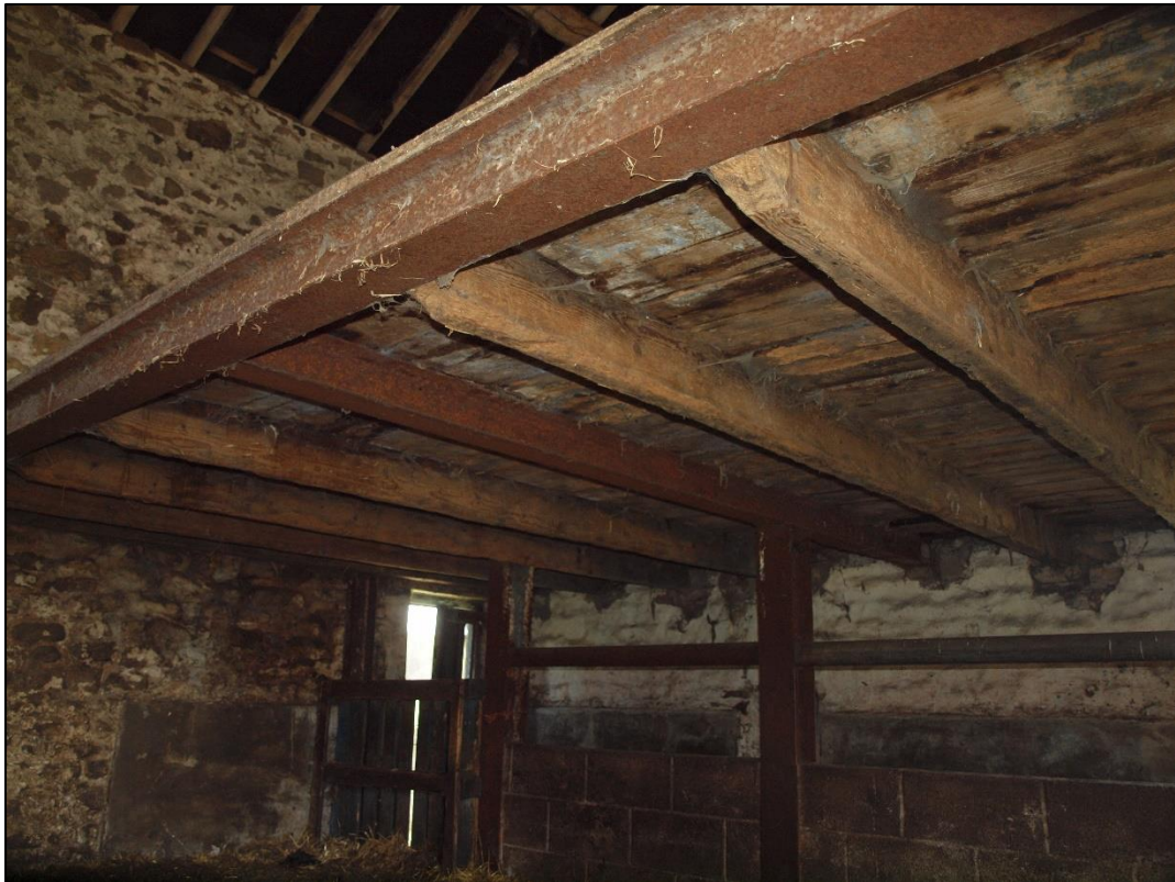
Plate 29: Detail of inserted first floor and concrete feeding passage
