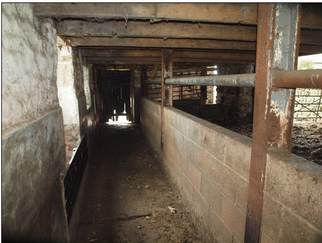
Plate 32: Inserted feeding passage along northeast wall, looking southeast
