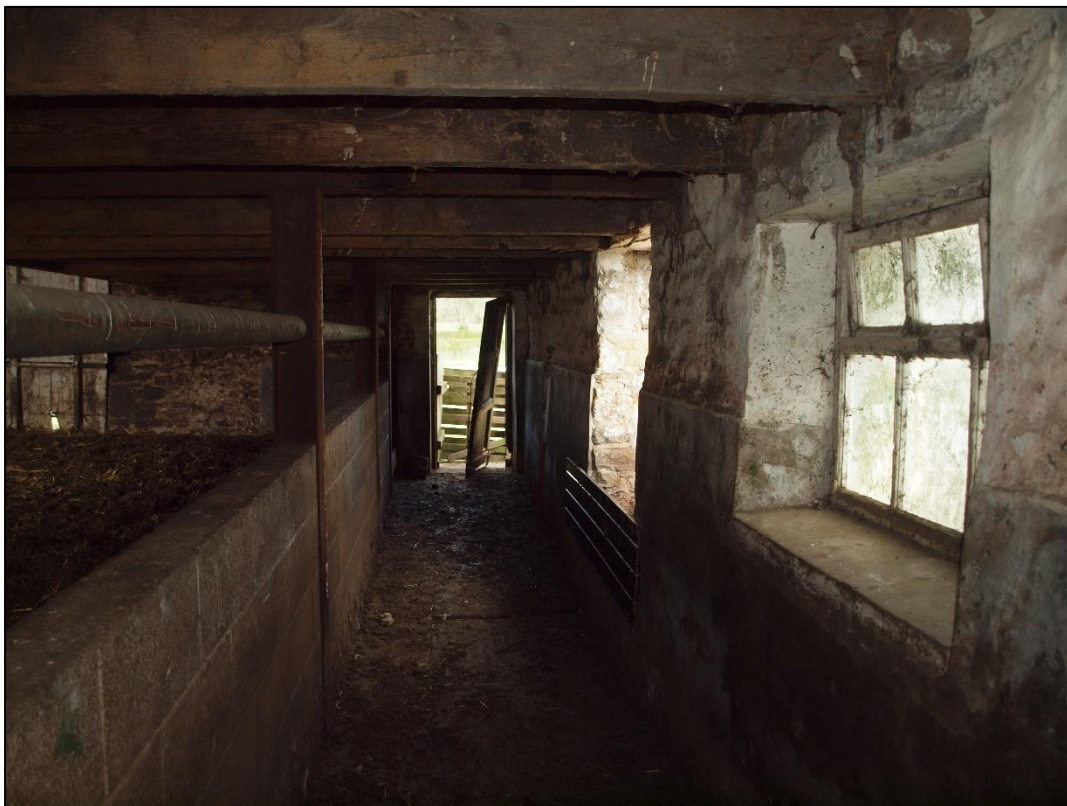
Plate 34: Feeding passage looking northwest
