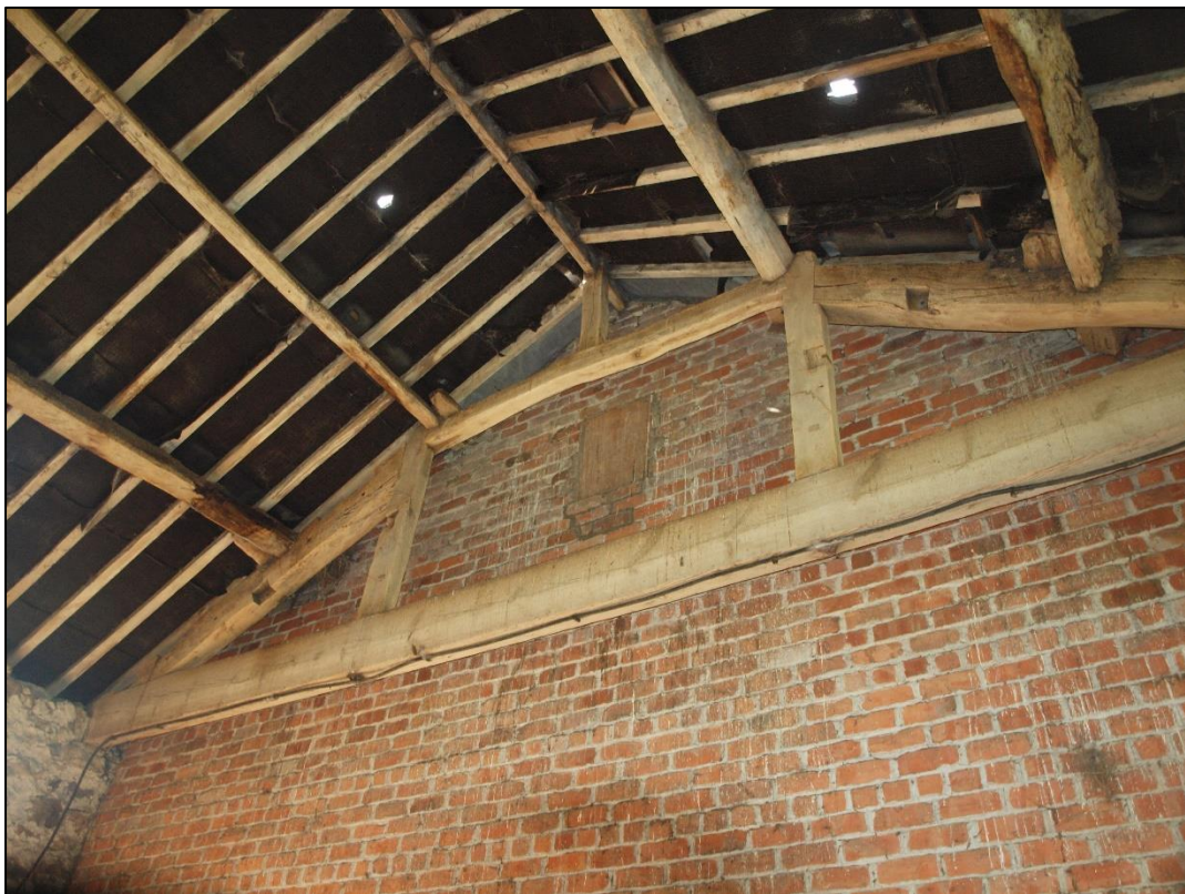
Plate 22: Southern queen post truss and brick wall
