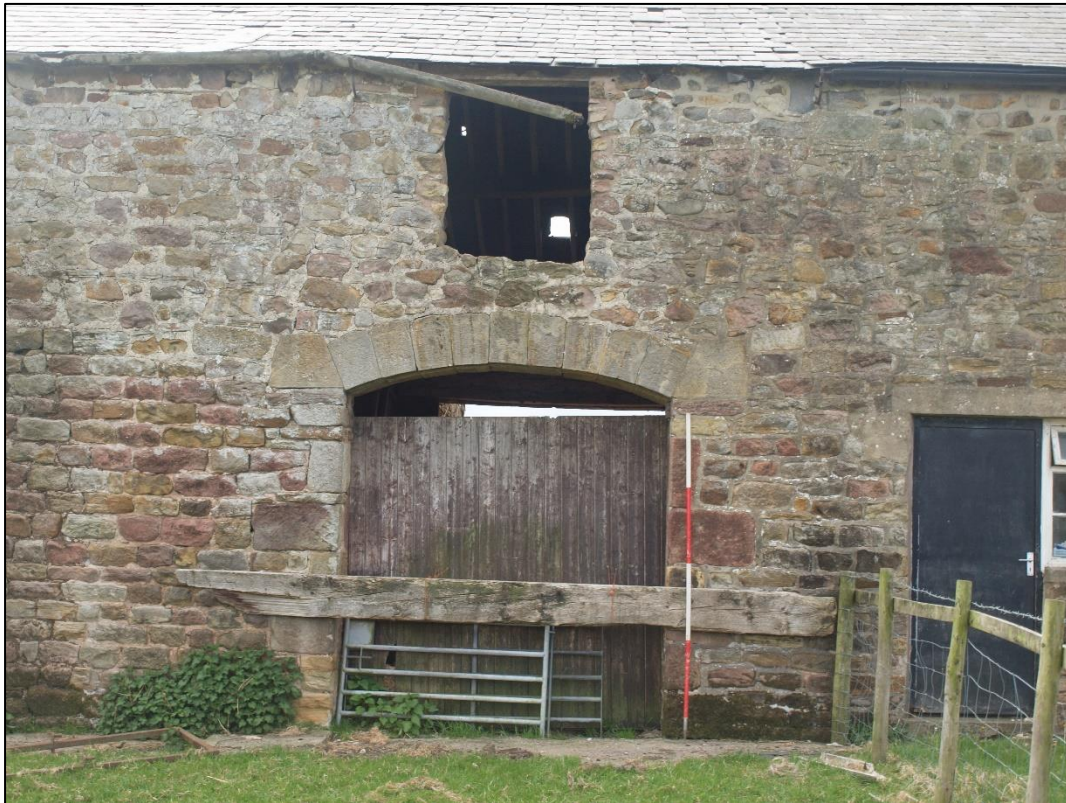
Plate 7: Barn door and pitching eye over. Note the change in stonework between ground and first floor
