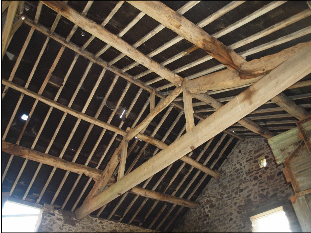
Plate 21: Queen post truss
