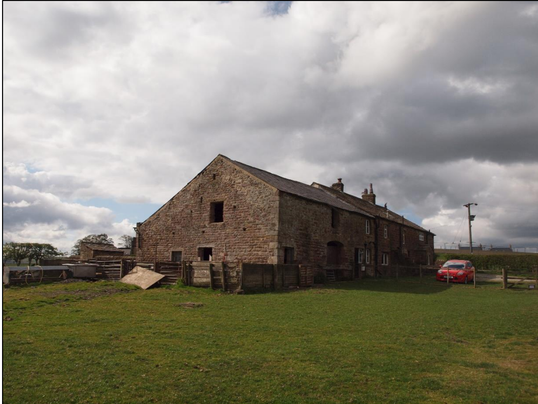
Plate 1: General shot of building from the north
