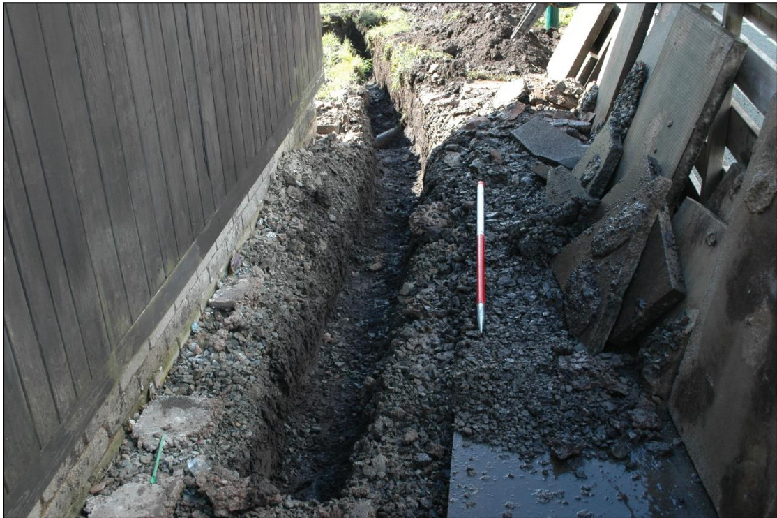
Plate 7: Service trench facing north
