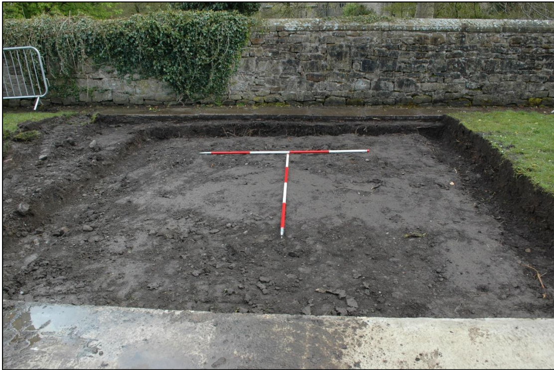
Plate 1: General shot of foundation trenches and stripped area
