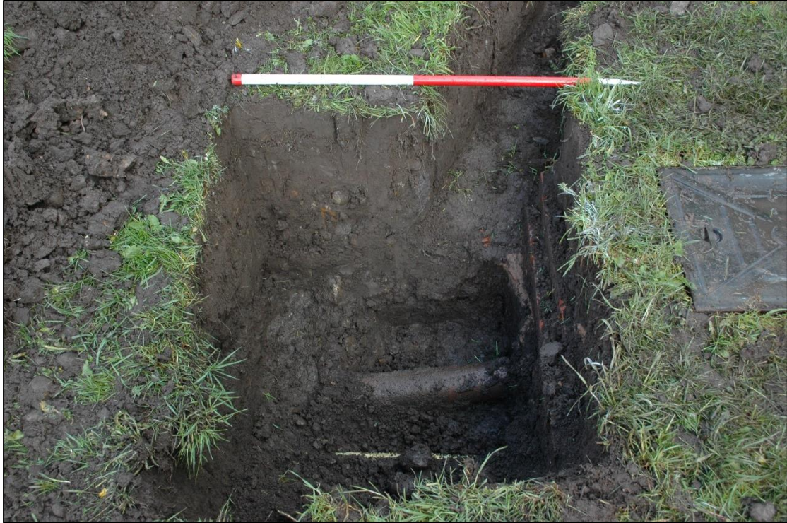
Plate 9: Manhole chamber facing south
