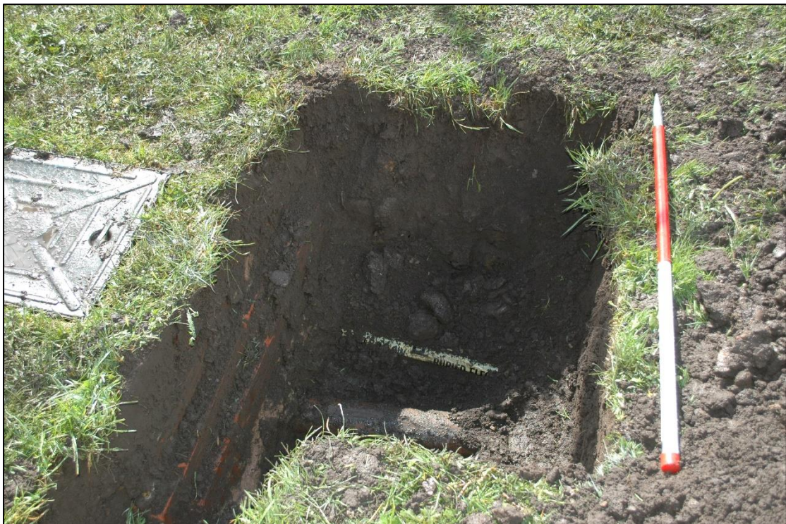
Plate 8: Manhole chamber facing north
