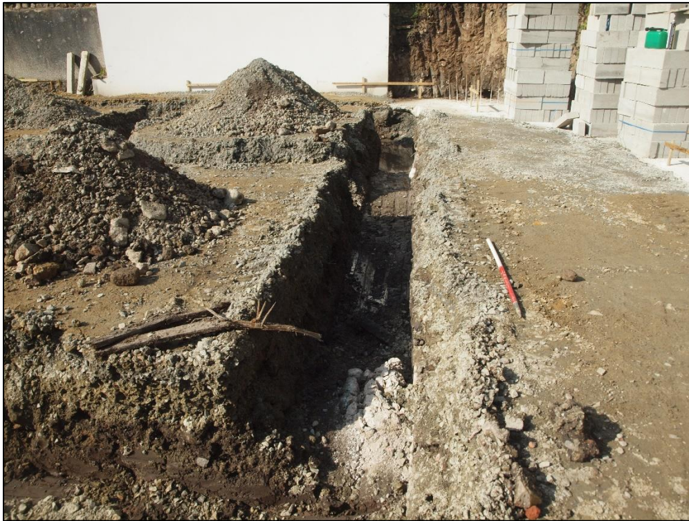
Plate 11: Eastern trench looking north showing concrete near base
