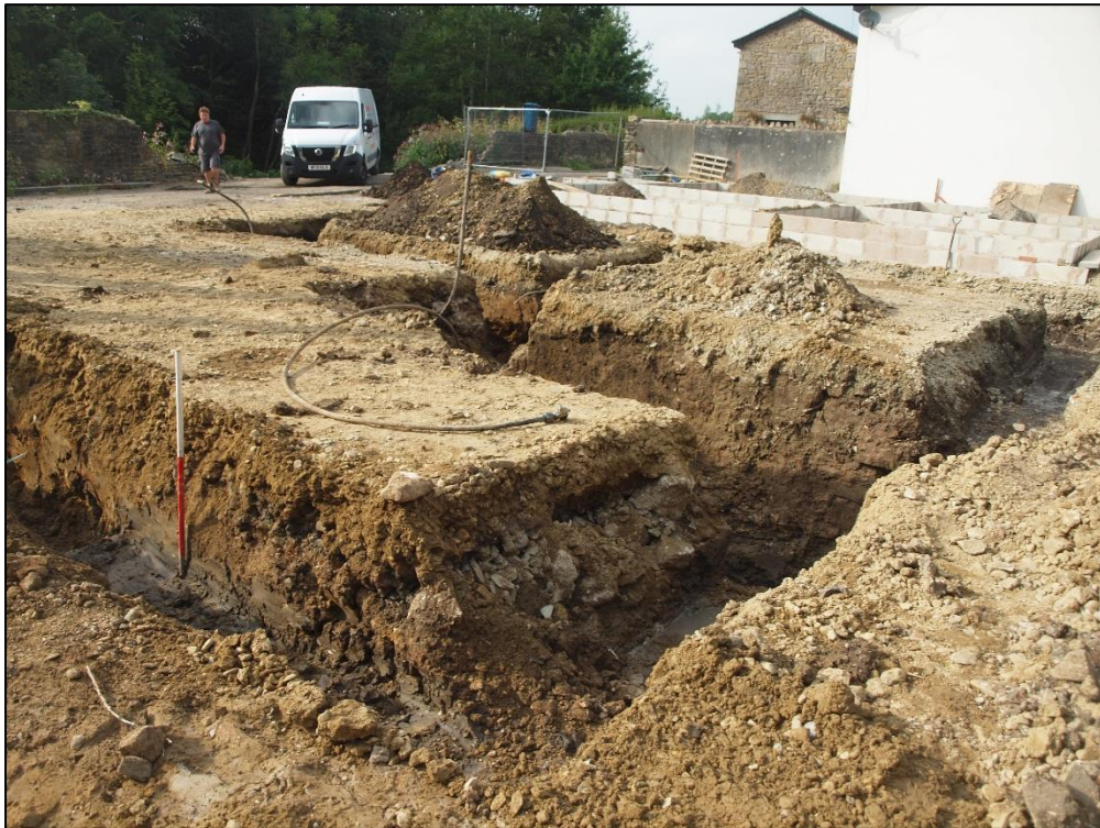
Plate 28: General shot looking northwest
