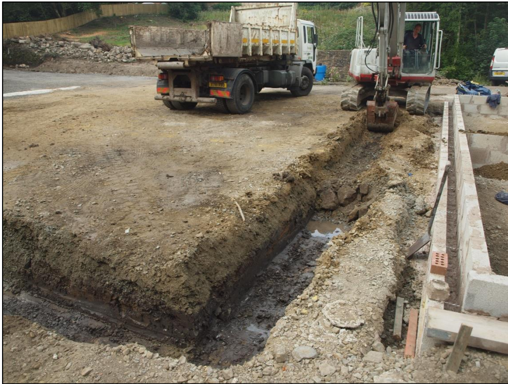
Plate 15: Working shot looking west
