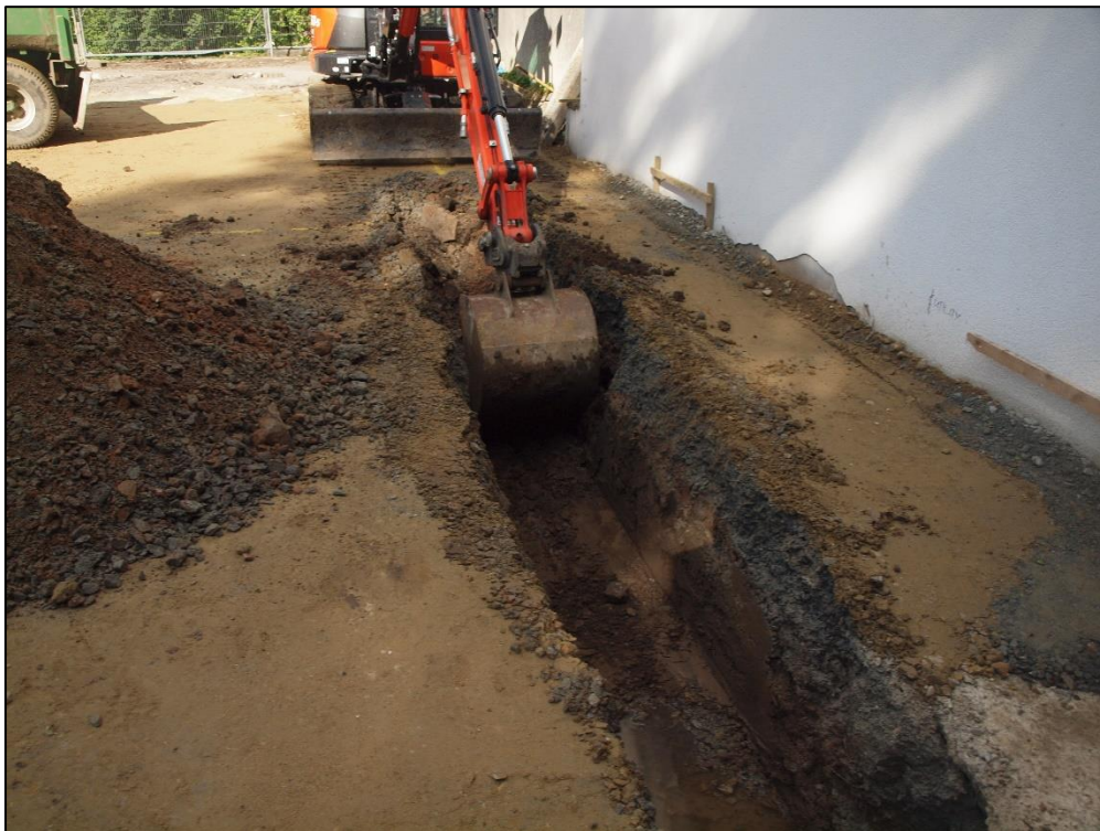
Plate 2: Initial opening of foundations
