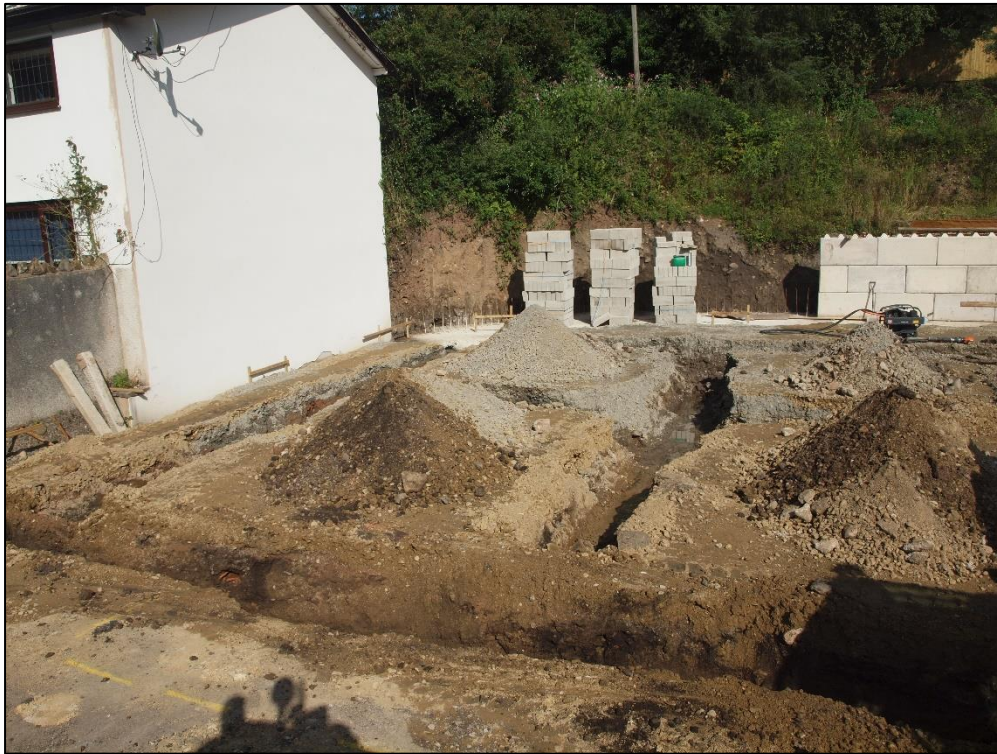
Plate 9: General shot of finished trenches looking northeast
