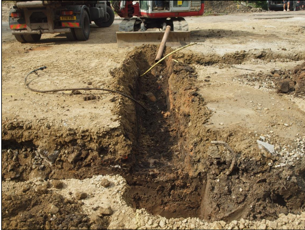
Plate 17: Initial opening of central trench looking west
