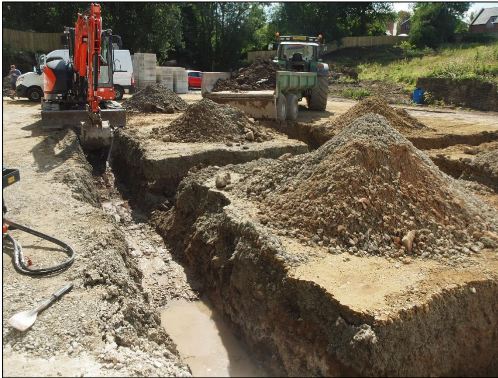
Plate 7: Working shot looking south
