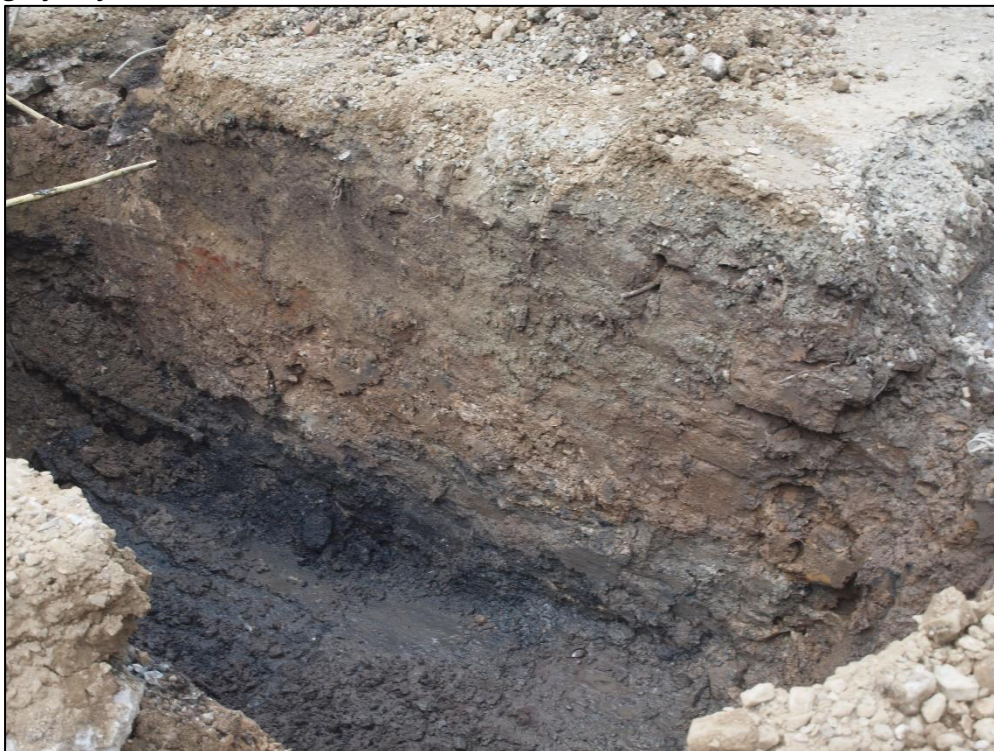
Plate 20: Detail of south facing section, showing wall (06) with bricks to the west (left) and stone to the east (right)
