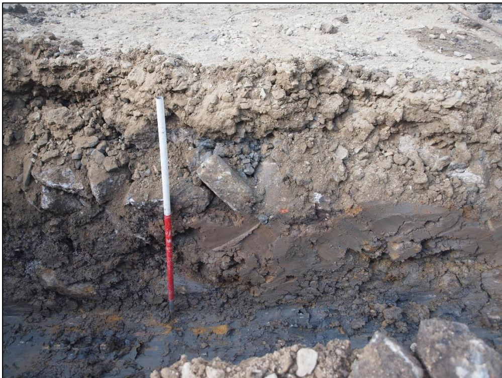
Plate 30: Example section at southern end showing grey clay (04) coming through at base at trench
