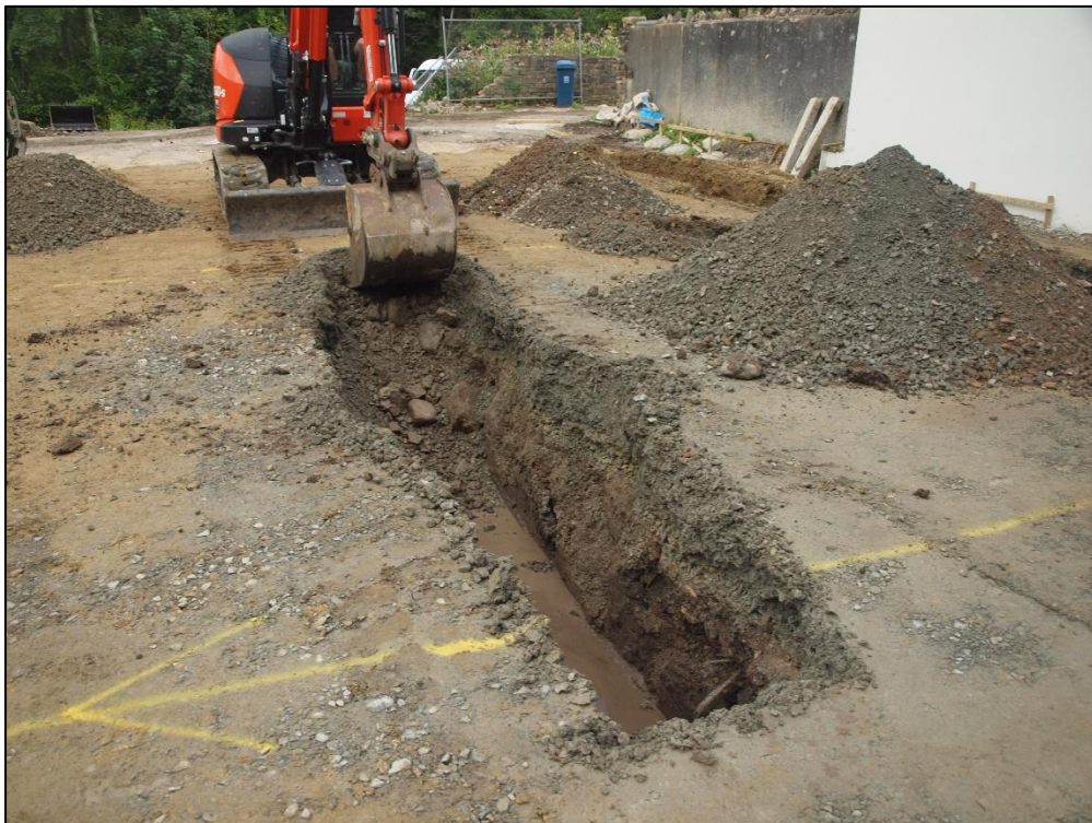
Plate 4: Working shot looking west
