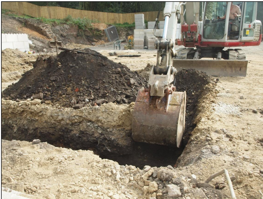
Plate 26: Working shot looking south
