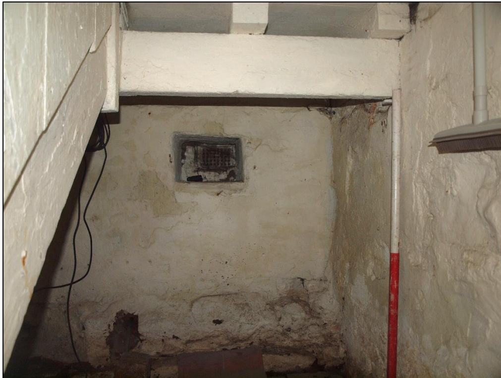
Plate 39: Storage area below stairs
