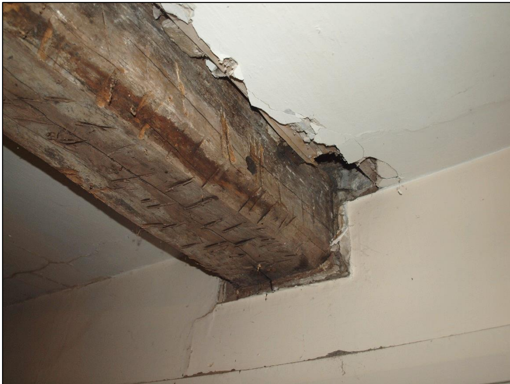
Plate 54: Detail of beam
