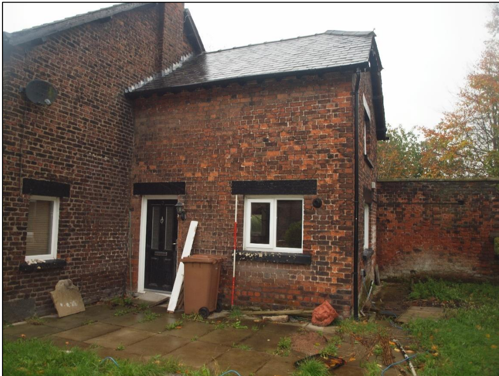
Plate 8: Southwest elevation of extension
