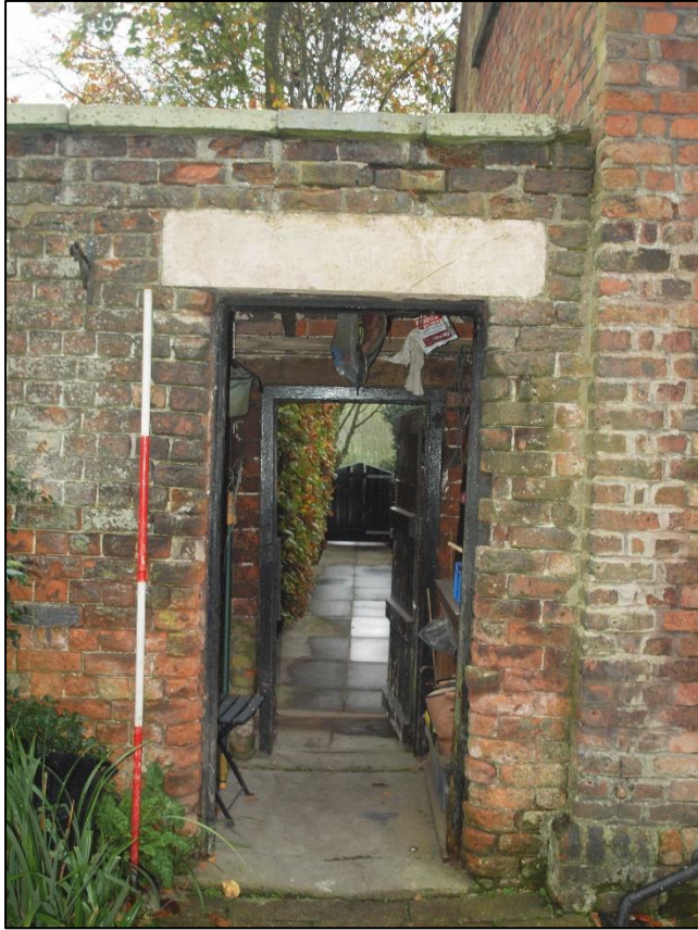
Plate 11: Eastern end of southwest elevation of outbuilding
