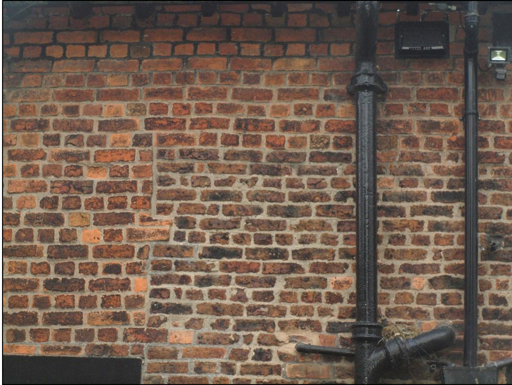
Plate 19: Detail of above showing straight joint and difference in brickwork
