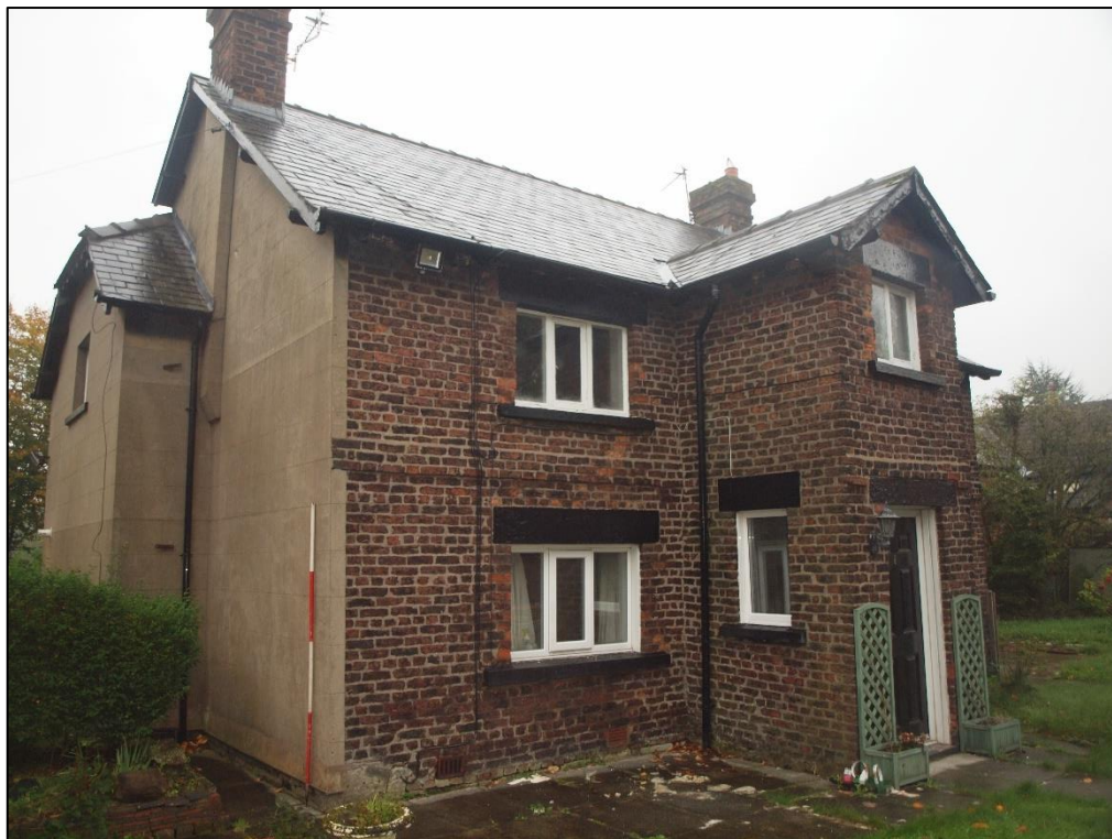
Plate 2: Southwest and Northwest elevations
