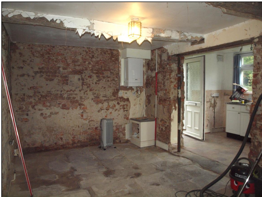
Plate 40: Kitchen to north corner of house
