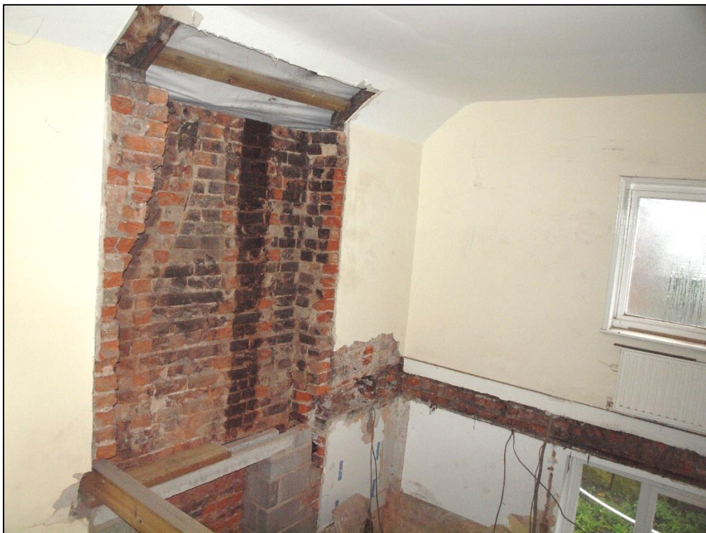
Plate 76: Extension showing removed fireplace
