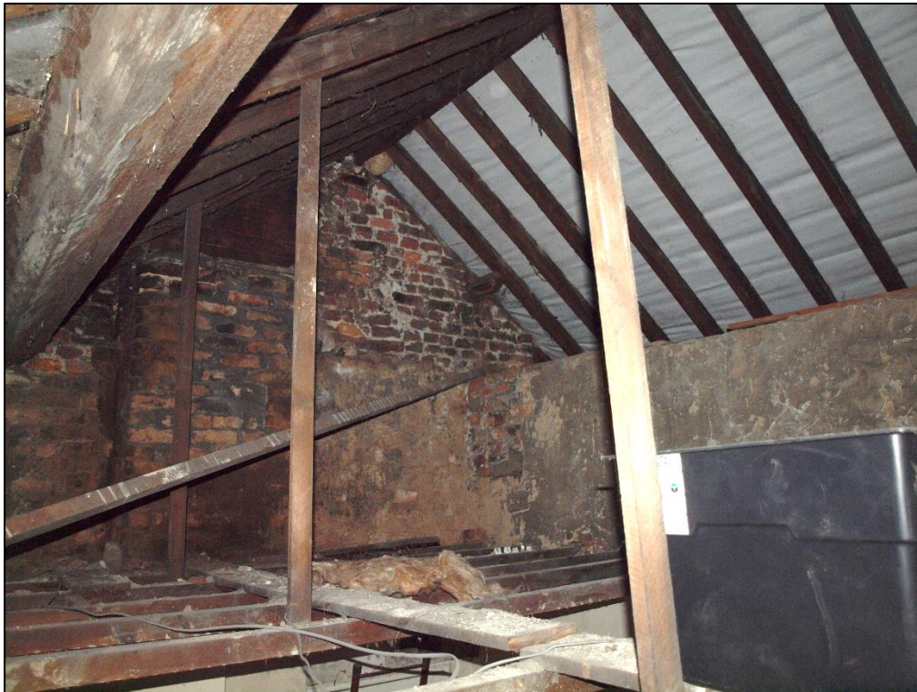
Plate 65: Detail of roof space above showing modern roof
