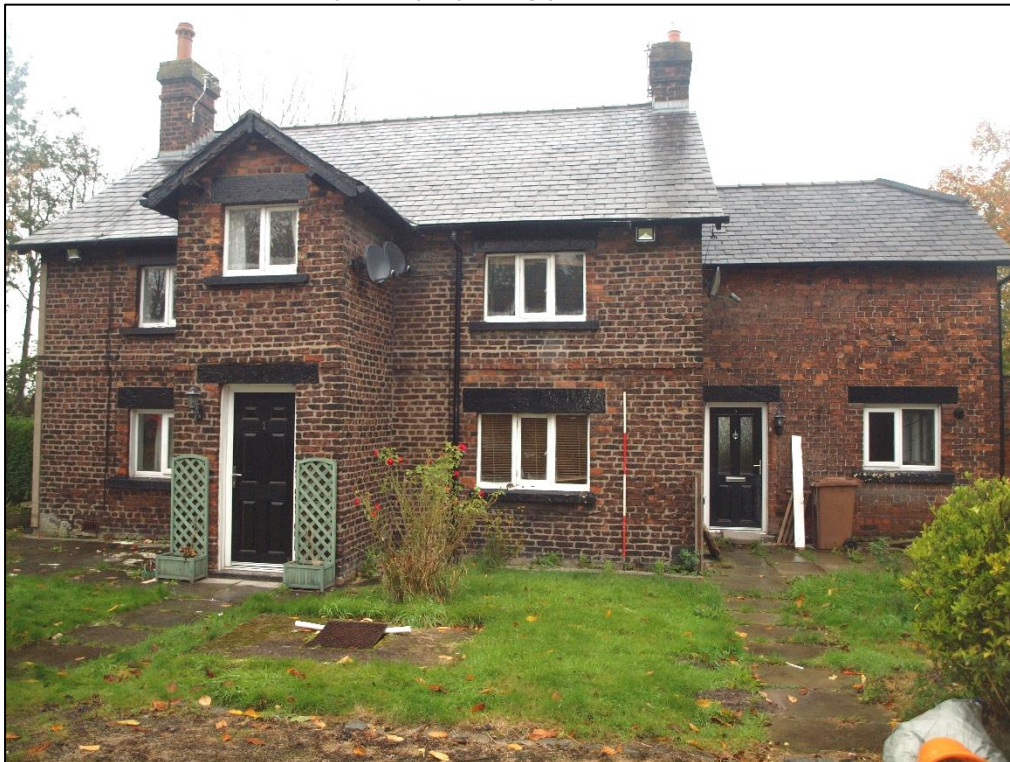
Plate 6: Southwest elevation showing extension
