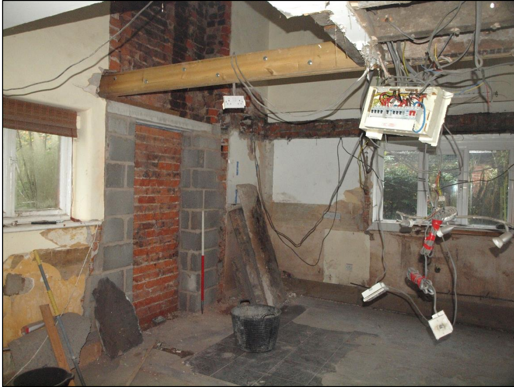
Plate 47: Interior of extension showing removed fireplace and ceiling
