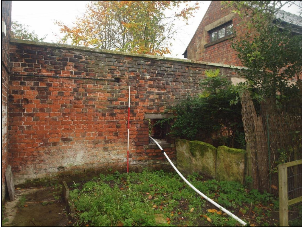
Plate 9: Southwest elevation of outbuilding
