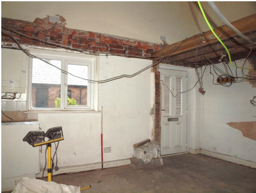
Plate 48: As above showing entrance to southwest elevation
