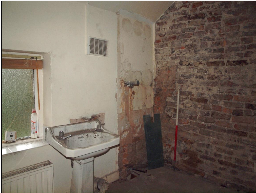
Plate 71: Bathroom to west corner of house
