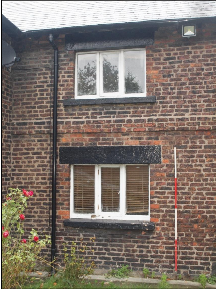
Plate 7: Detail of Bay 3 windows
