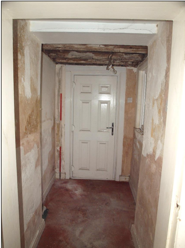
Plate 27: Interior of porch showing front door
