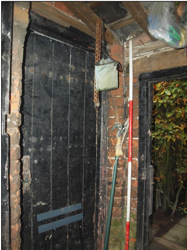
Plate 56: Interior of east end of outbuilding
