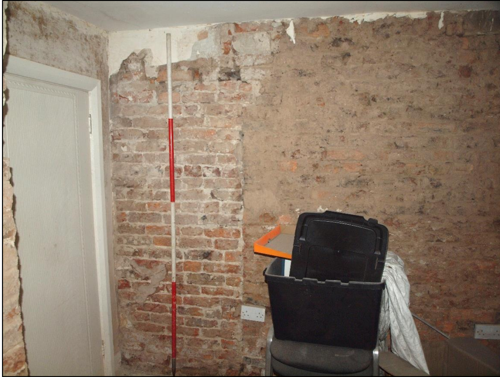
Plate 33: Detail of blocked doorway
