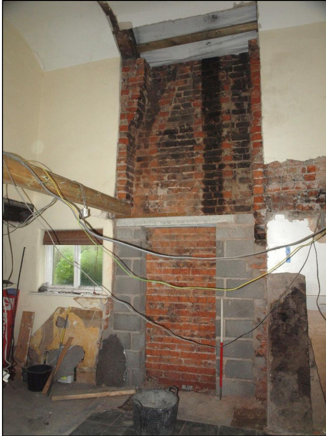
Plate 49: Removed ground and first floor fireplaces
