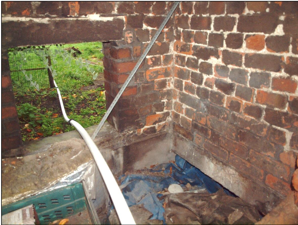
Plate 57: Interior of central room of outbuilding showing concrete beam supporting opening below adjacent toilet
