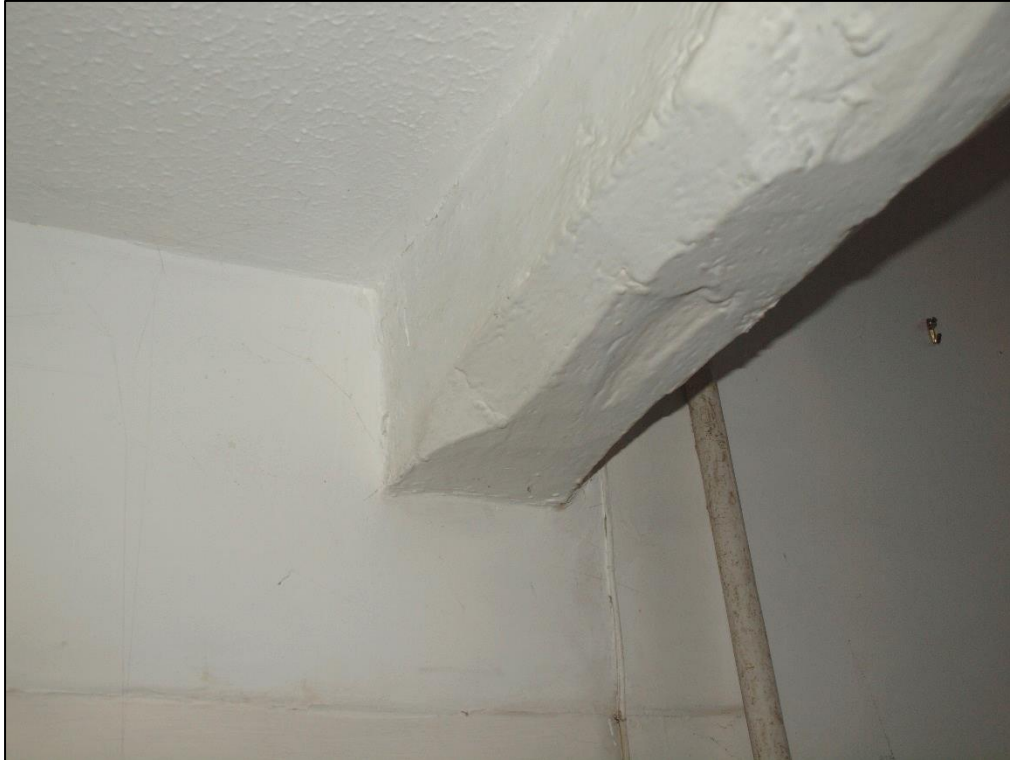
Plate 37: Reused beam in staircase showing blocked soffit
