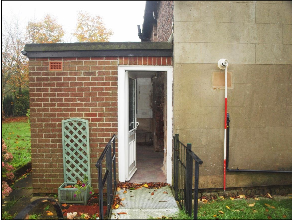
Plate 13: Northwest elevation of kitchen extension
