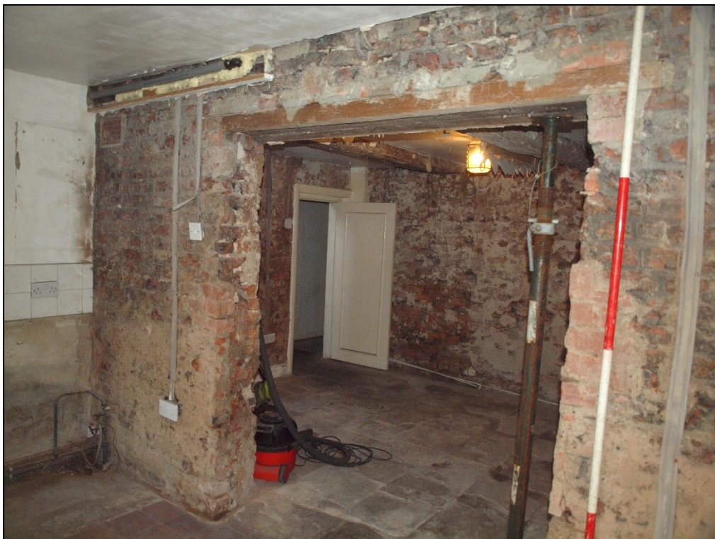
Plate 44: Inserted opening to kitchen extension
