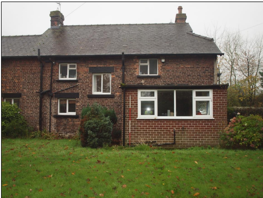
Plate 16: Northeast elevation of main house and kitchen extension
