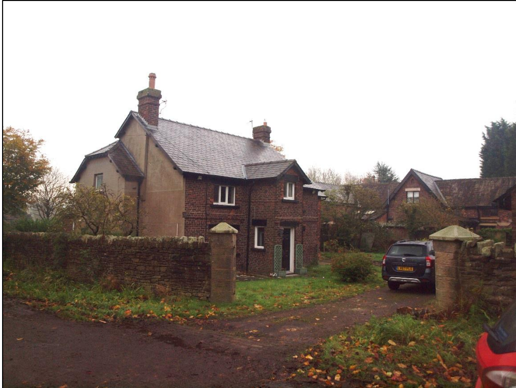
Plate 1: General shot of building
