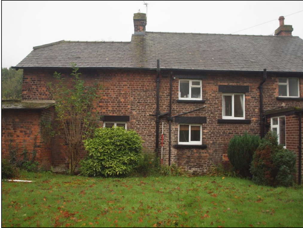
Plate 17: Northeast elevation showing extension
