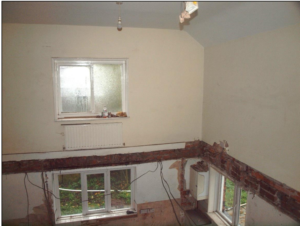
Plate 77: First floor of extension
