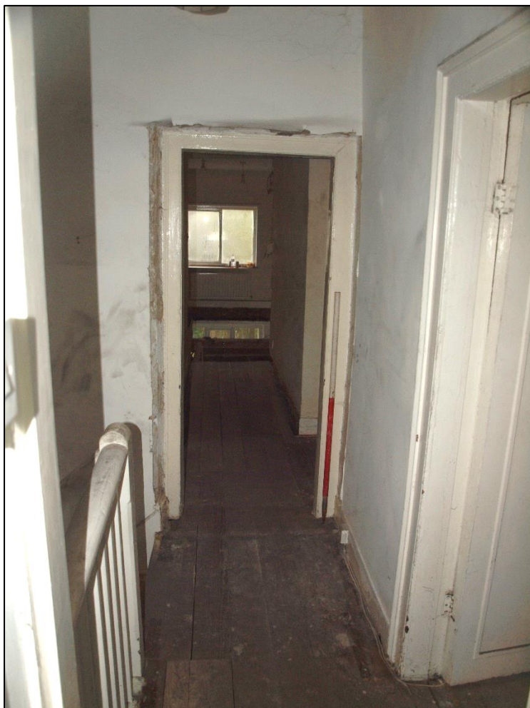
Plate 61: First floor landing
