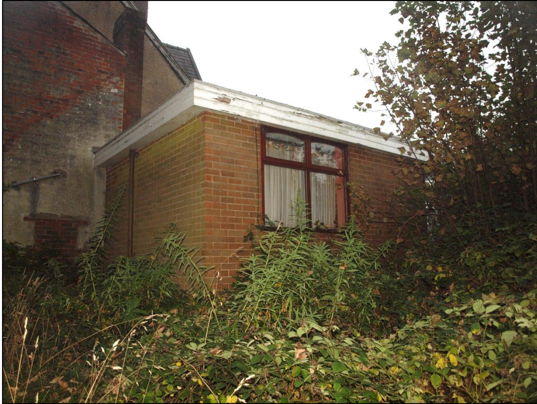
Plate 13: West elevation of western extension
