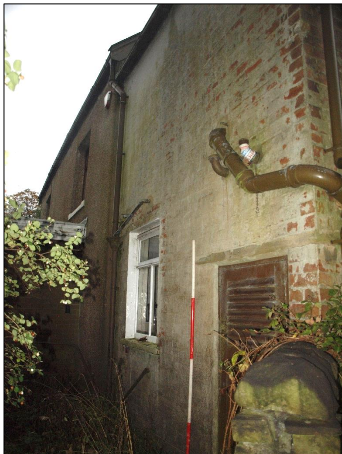
Plate 11: North elevation of west extension
