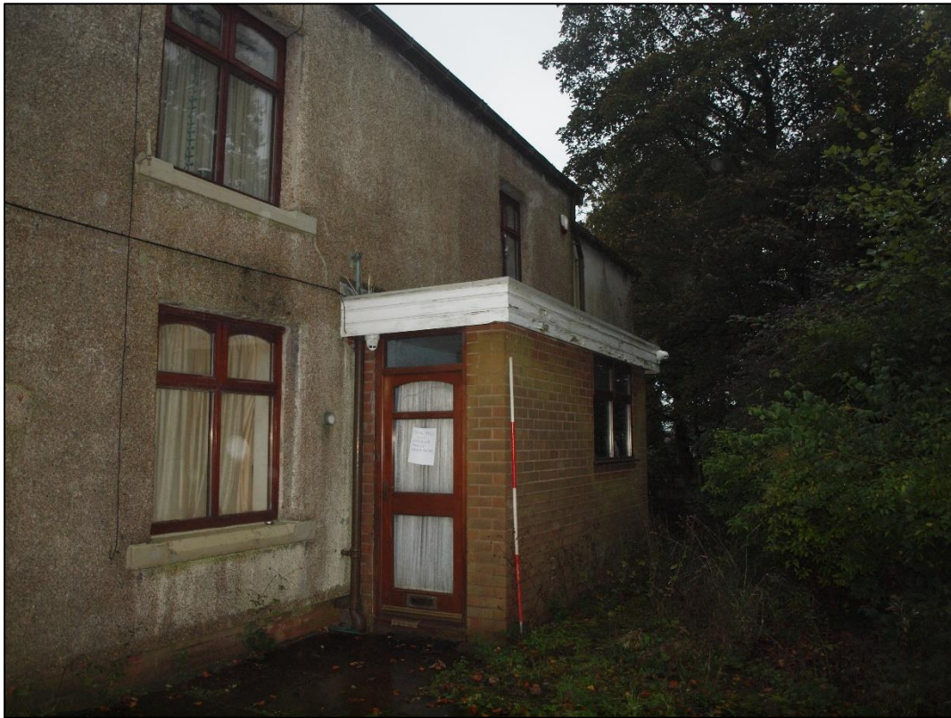
Plate 9: East elevation of northern porch extension
