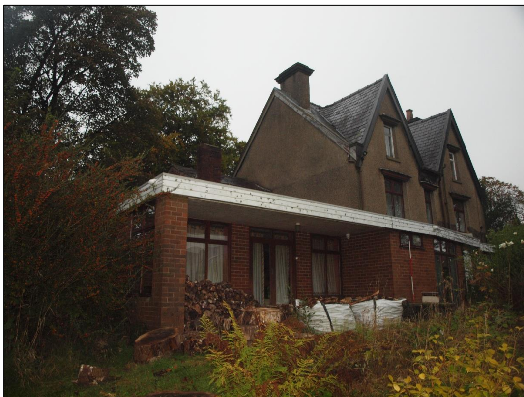
Plate 6: South elevation of extension
