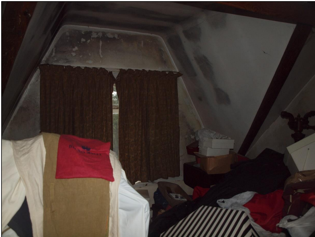
Plate 38: Bedroom to southwest corner
