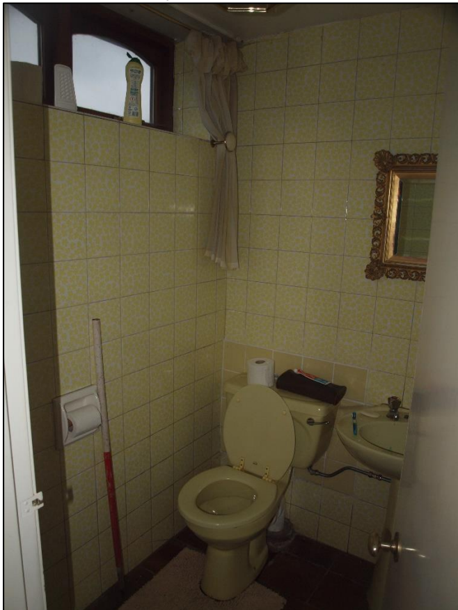
Plate 26: Toilet in southern porch extension
