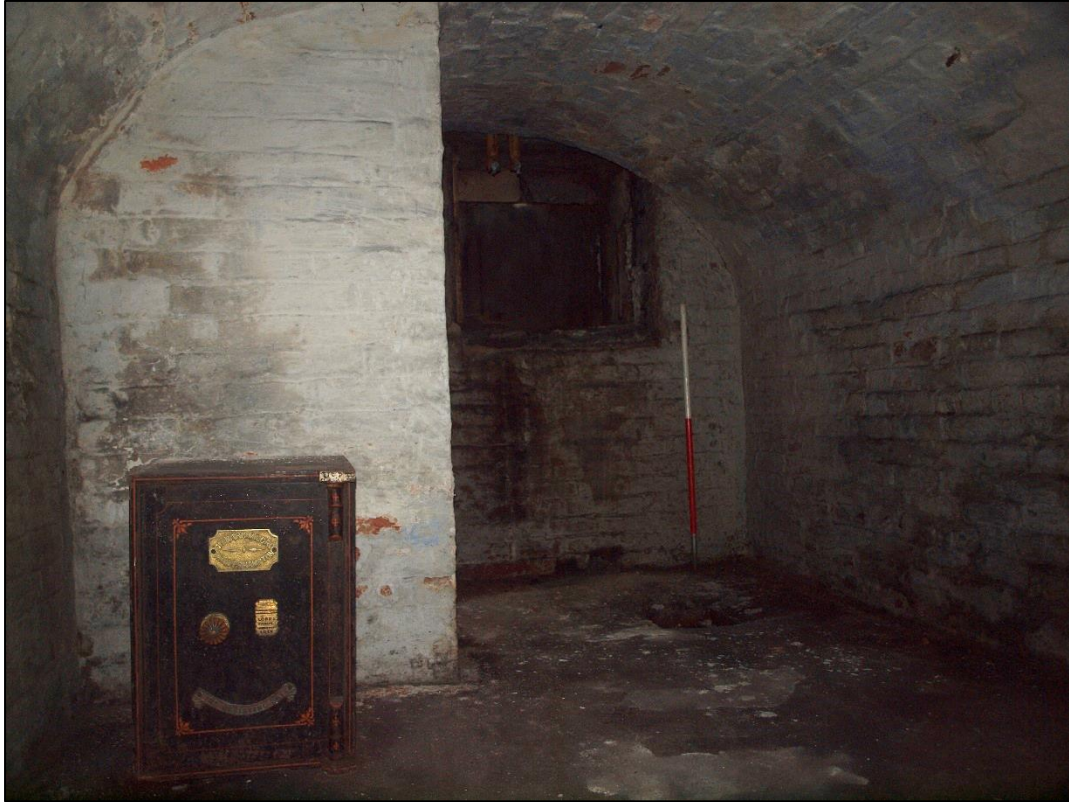
Plate 41: Basement looking south
