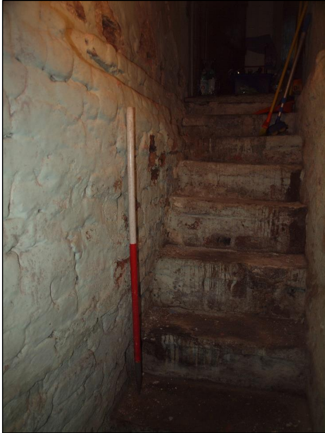
Plate 39: Stone and brick steps to basement
