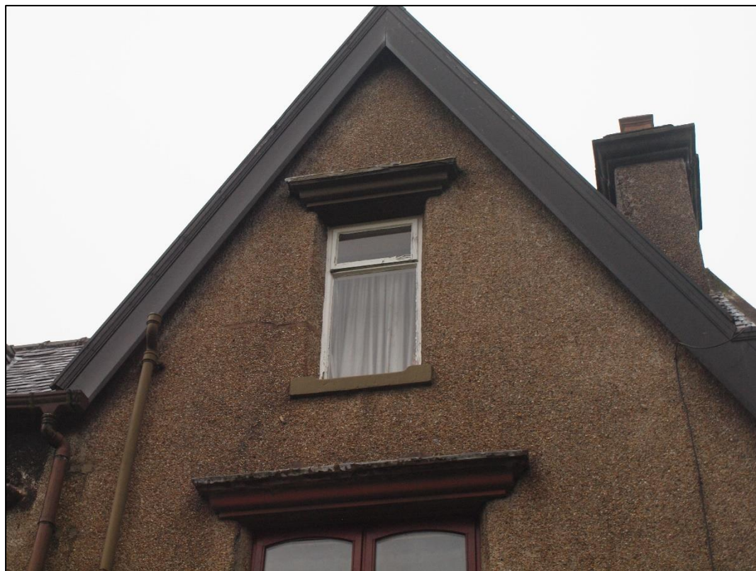
Plate 5: Detail of attic window
