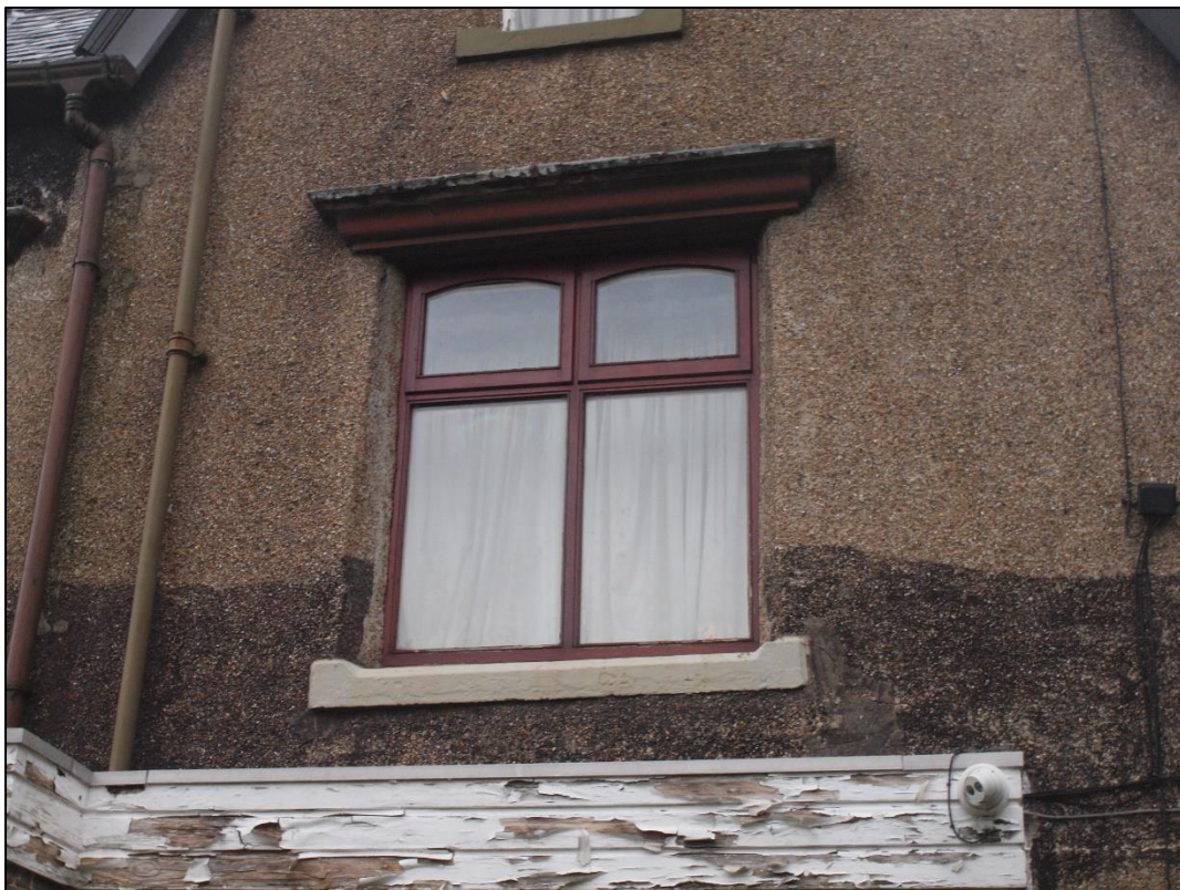
Plate 4: Detail of first floor window
