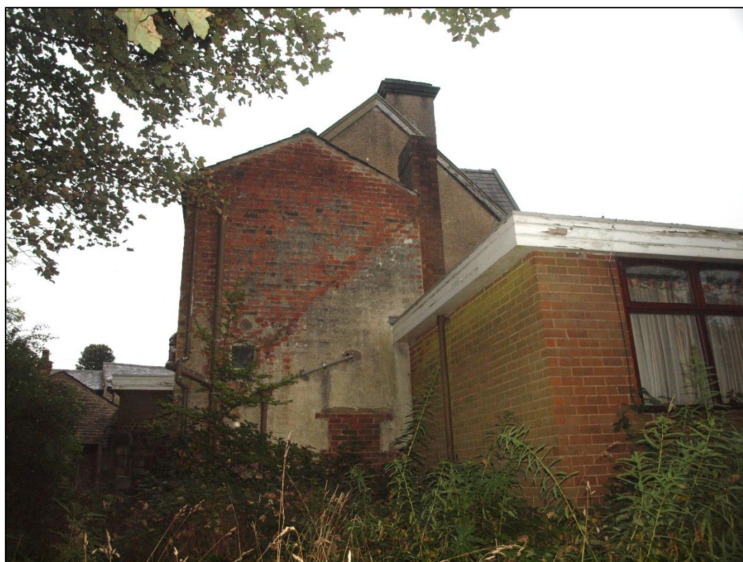
Plate 12: North elevation of later west extension and western gables
