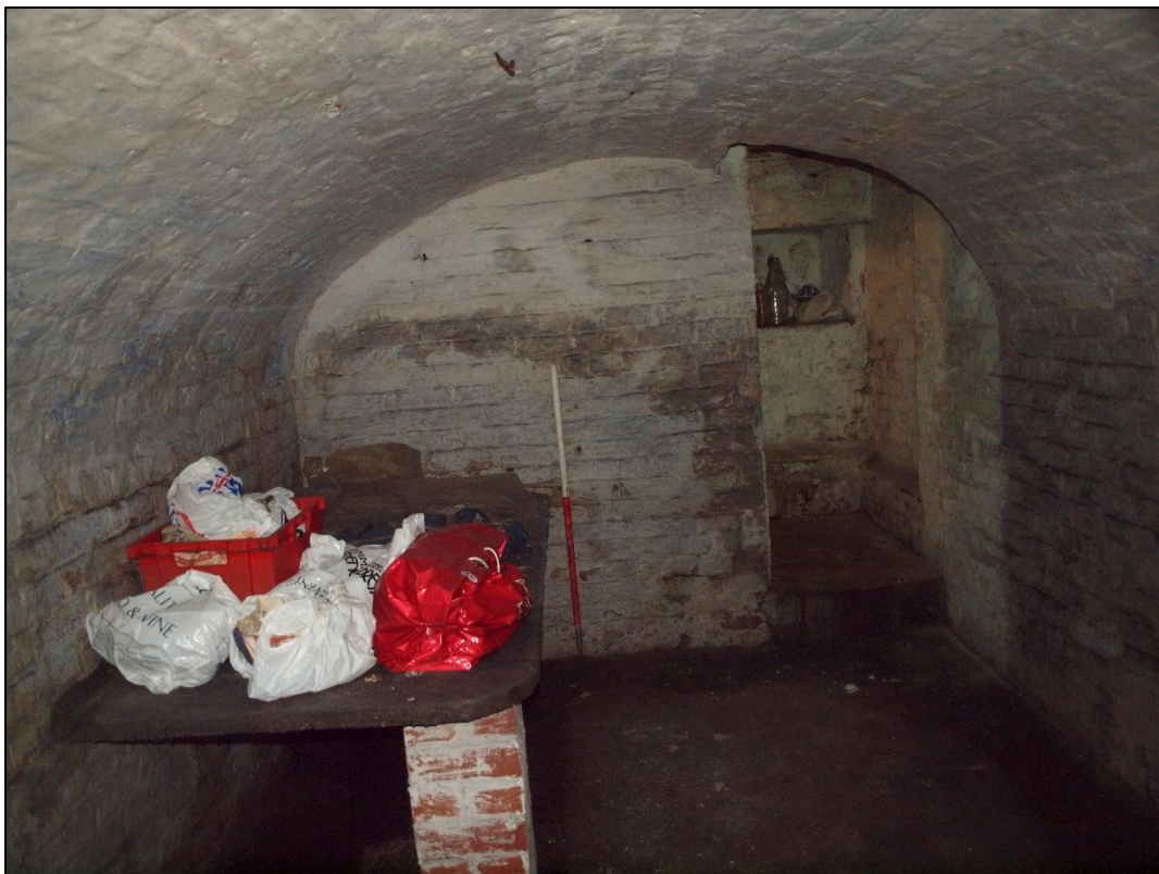
Plate 44: Basement looking north
