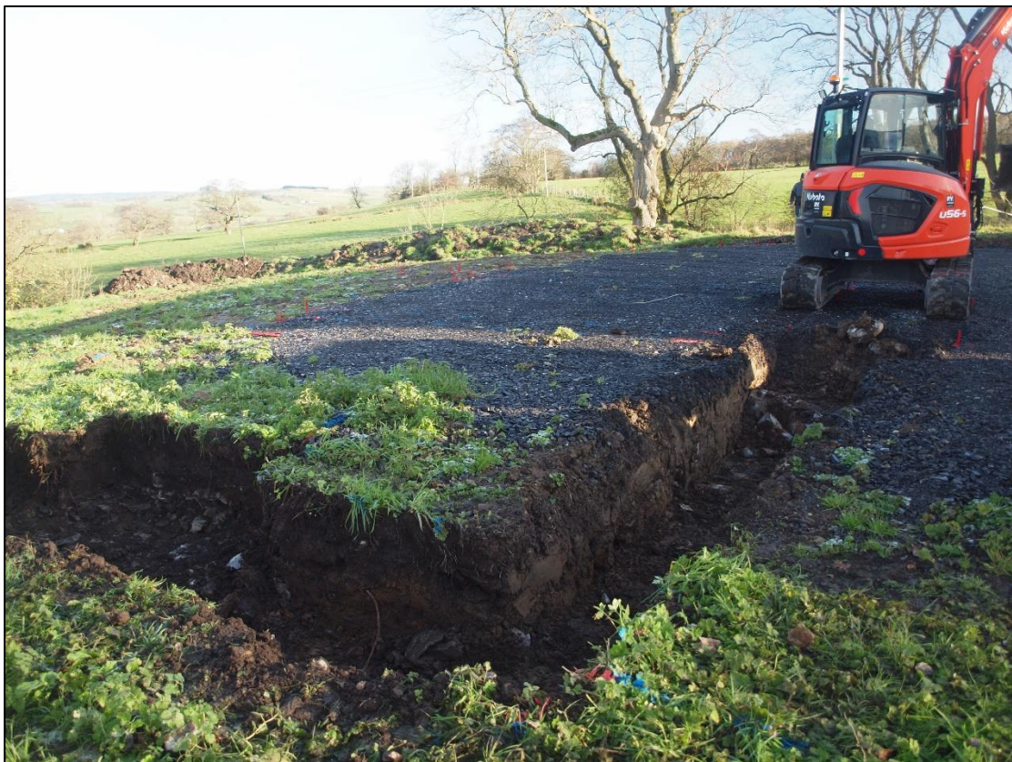
Plate 32: Further trench opening
