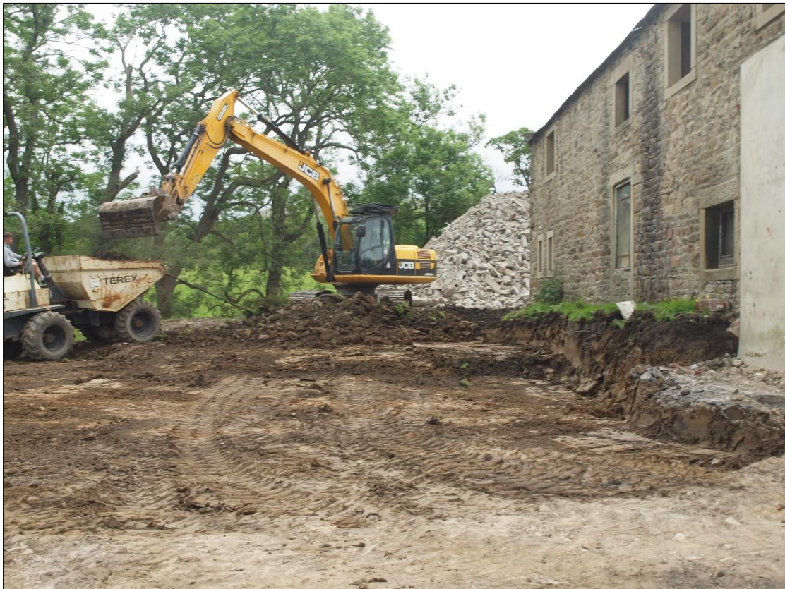
Plate 12: Working shot to northeast corner
