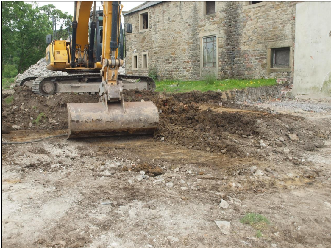
Plate 9: As above showing revealed natural clay (03)
