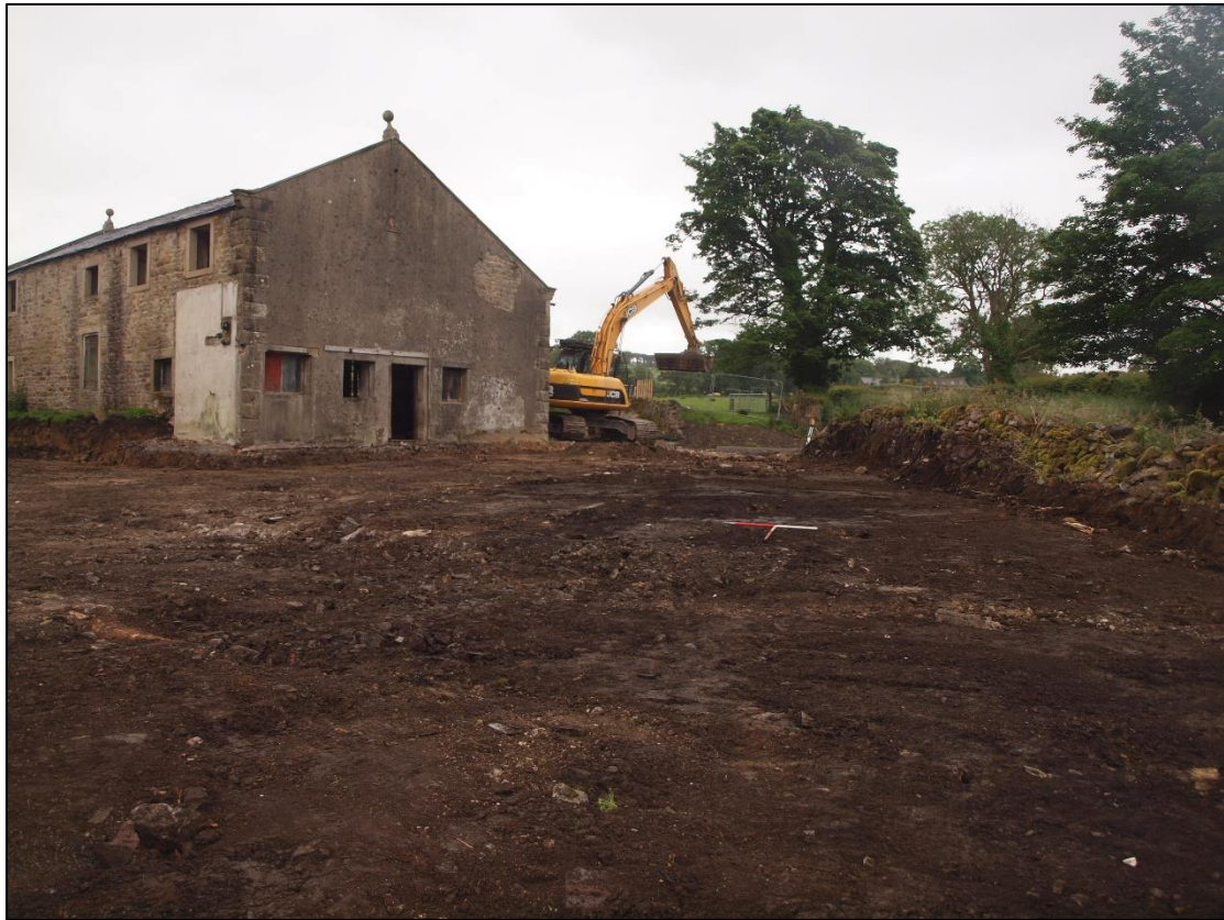
Plate 19: As above after clearance
