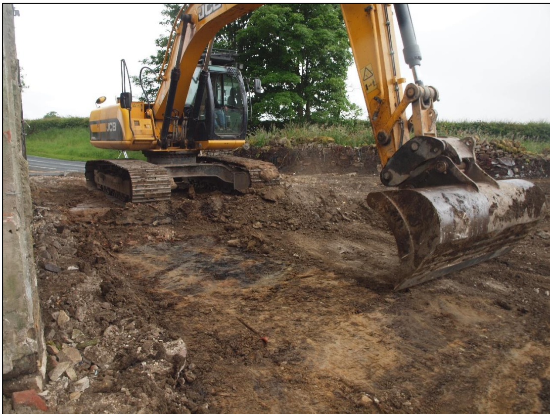
Plate 16: Clearance to west of barn
