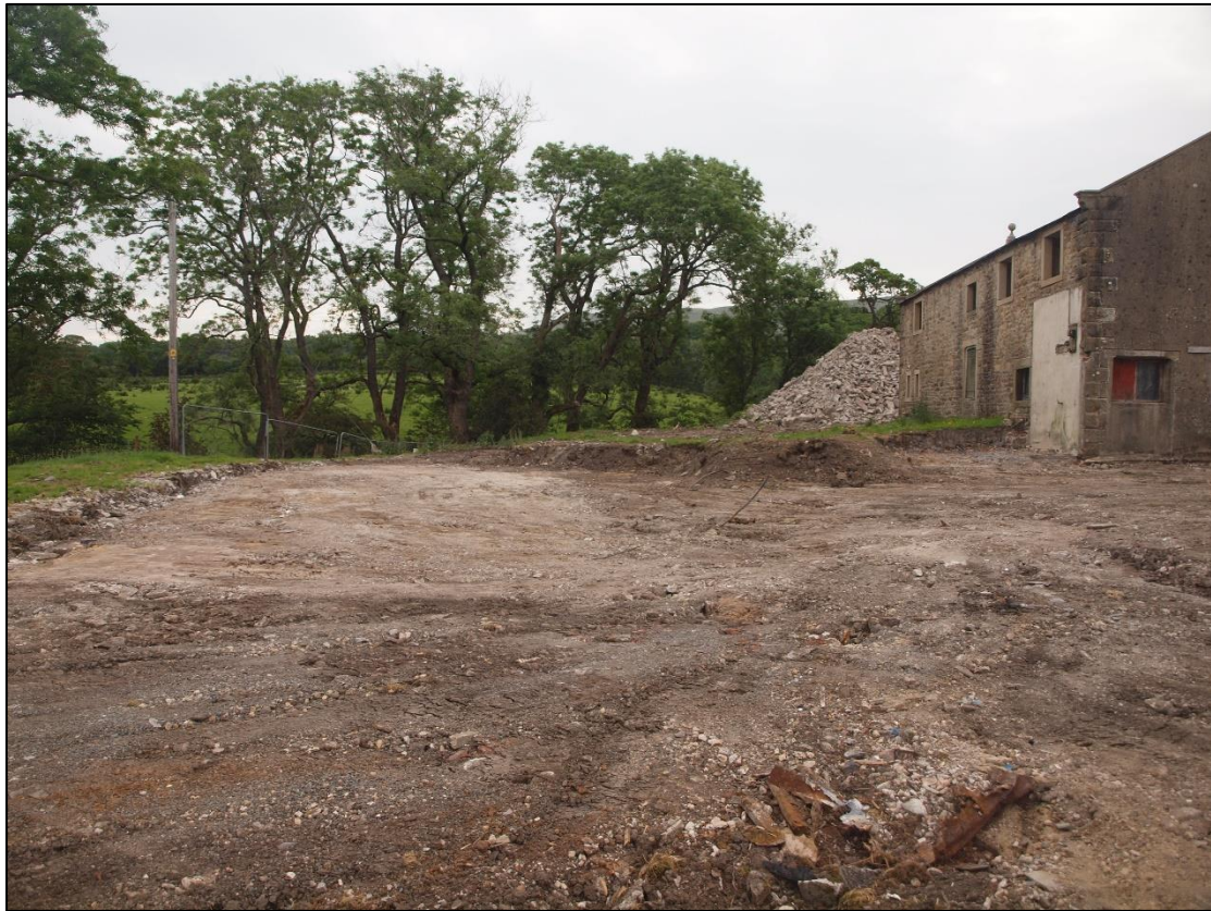
Plate 3: North side prior to clearance
