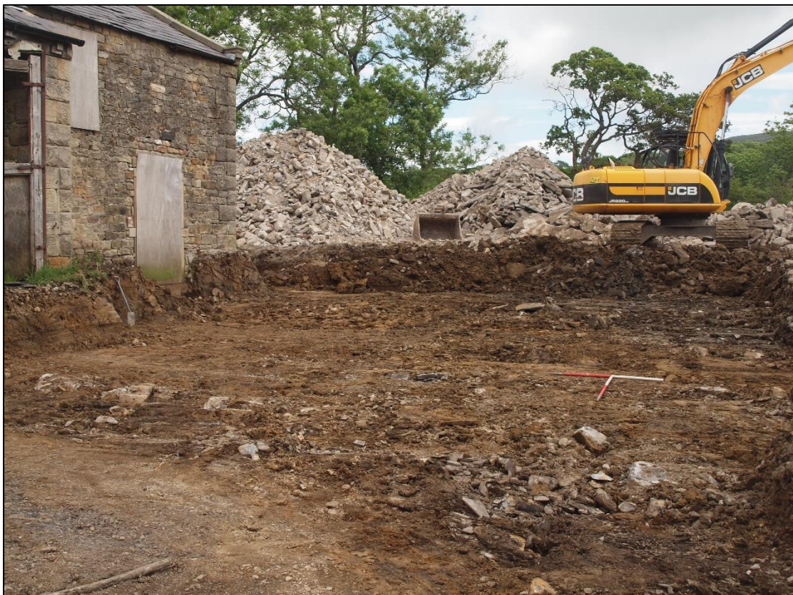
Plate 28: South side of site after clearance
