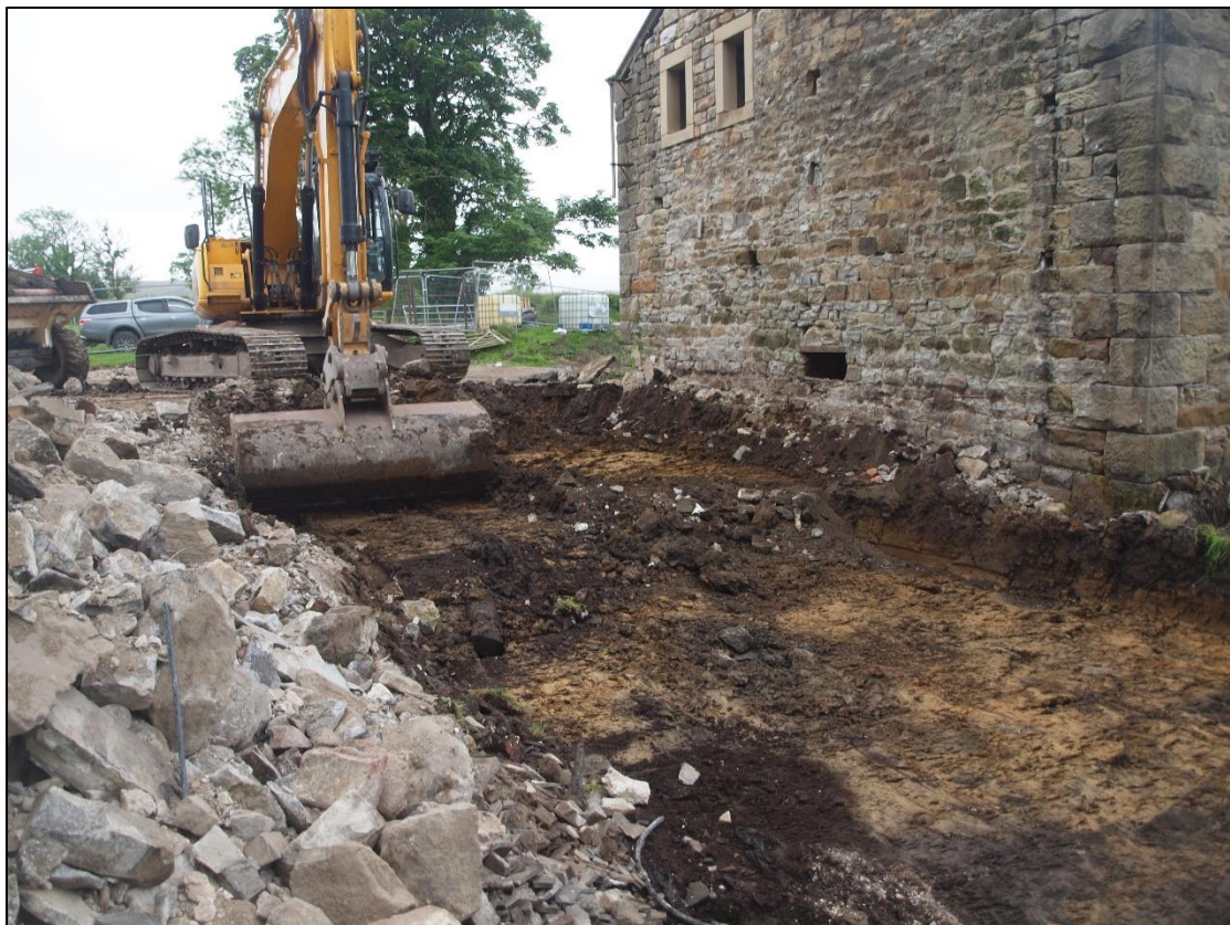
Plate 20: Clearance to east side of barn showing clay (03)
