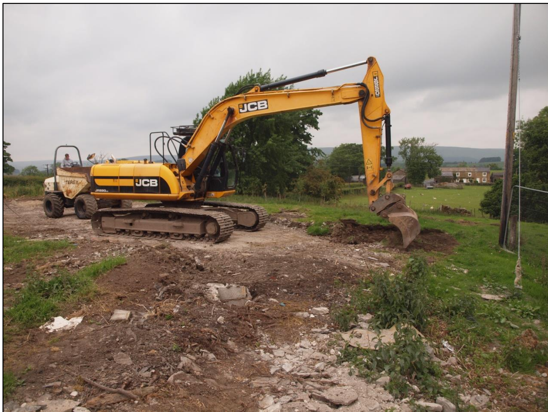
Plate 4: Northwest corner of site at commencement of clearance
