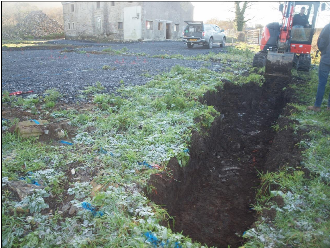
Plate 29: Initial trench opening
