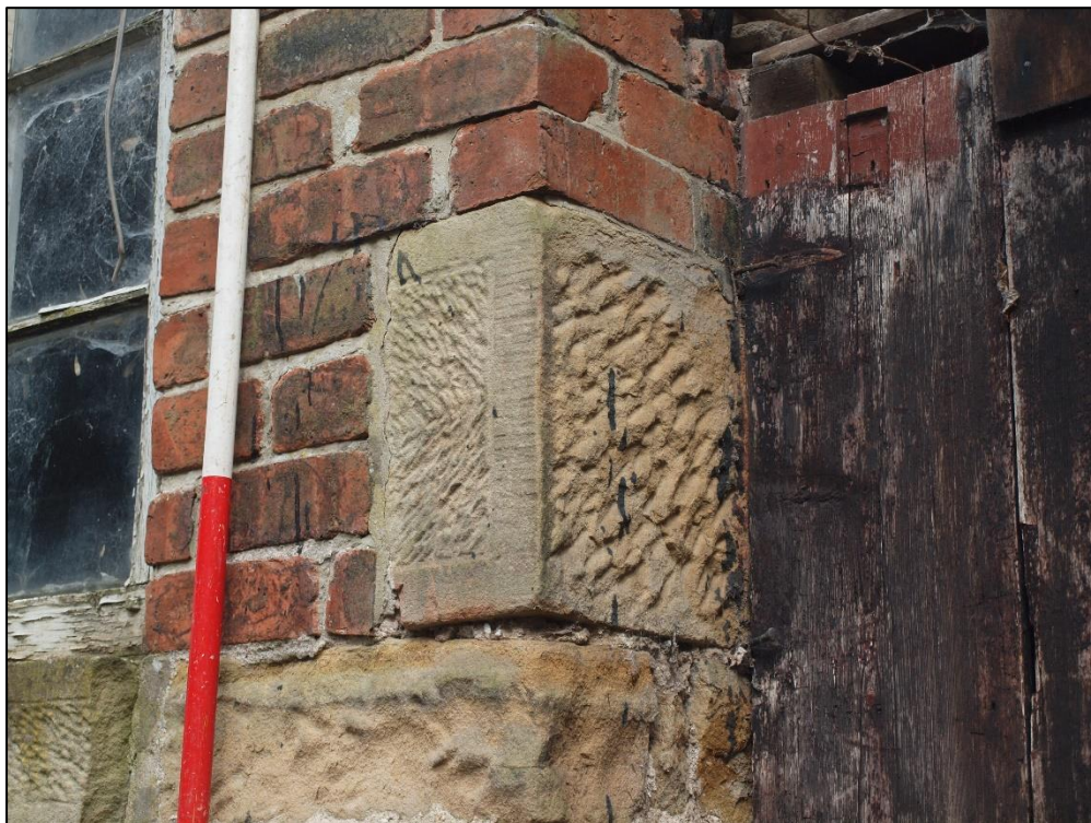
Plate 8: Detail of dressed sandstone quoin to corner
