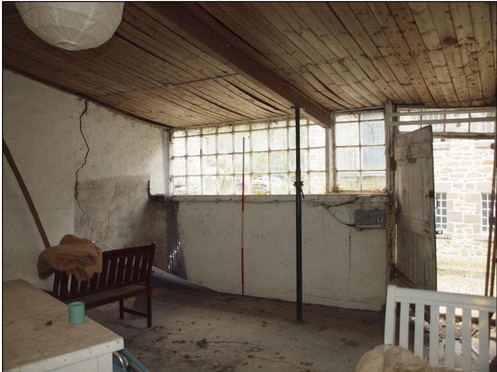
Plate 24: East end of southwest wall
