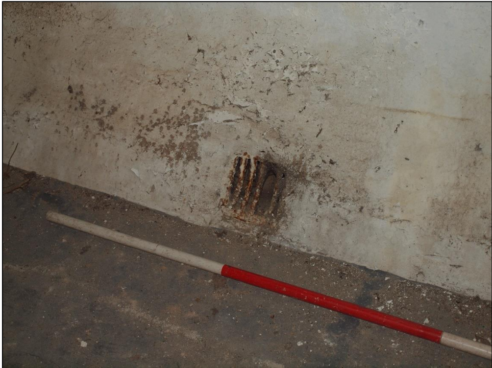
Plate 23: Drain hole in sloping base of northeast wall
