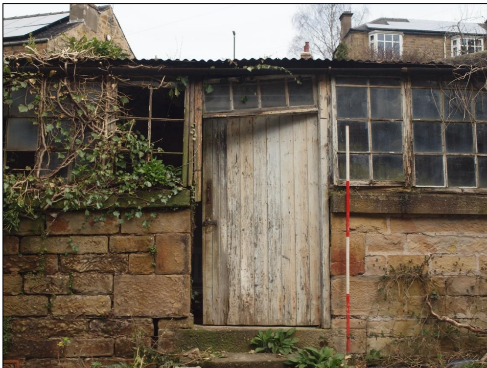
Plate 4: Central doorway detail
