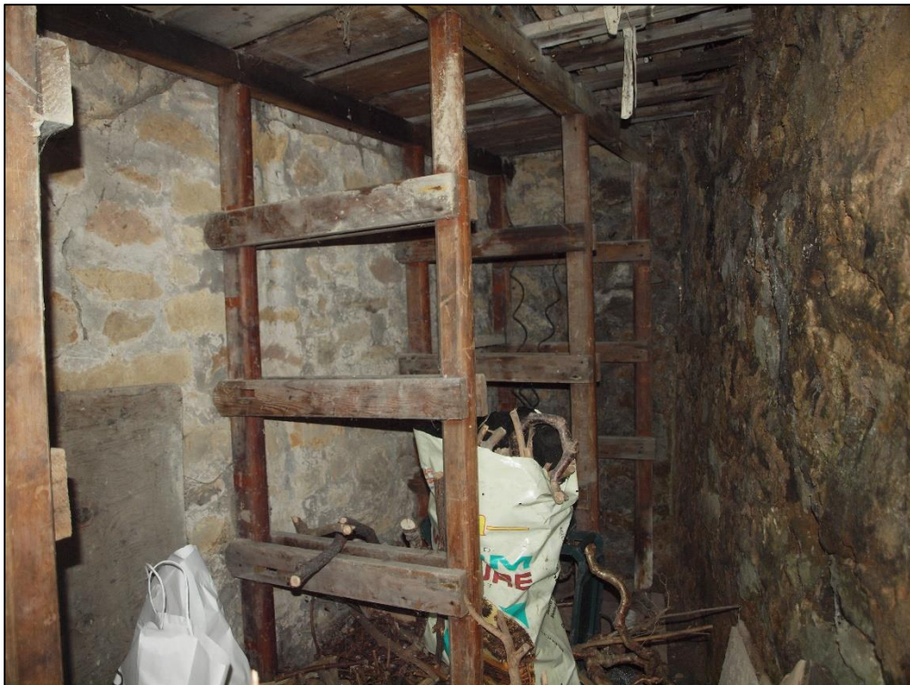
Plate 12: Southeast elevation beyond inserted timber door
