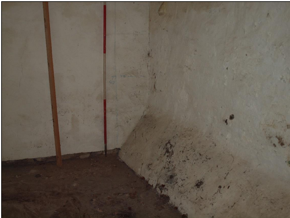
Plate 18: Detail of northeast wall showing sloping base
