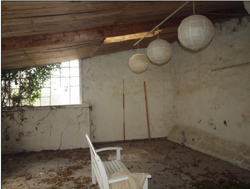
Plate 17: General shot of interior looking west
