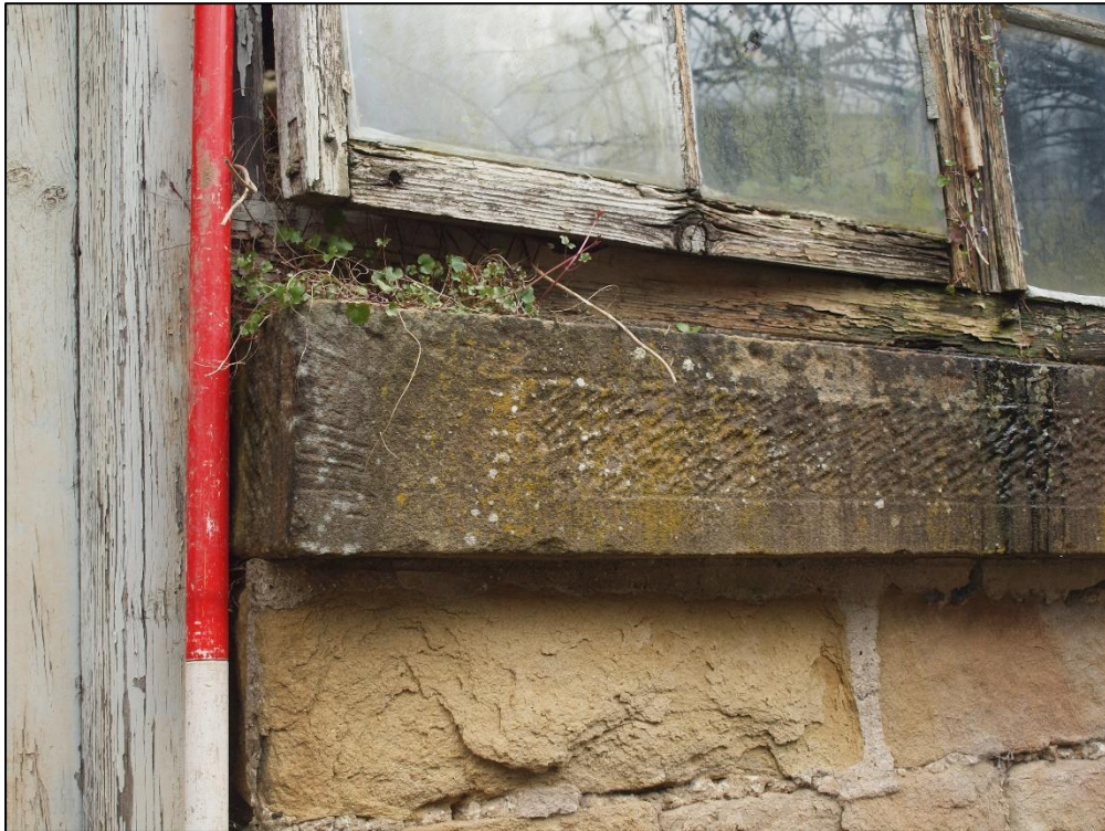
Plate 9: Detail of dressed sandstone window cills
