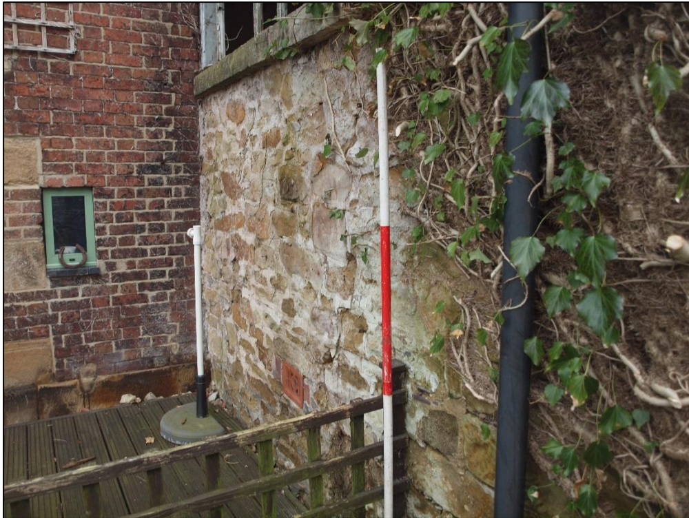
Plate 11: Wall detail showing rough rubble construction
