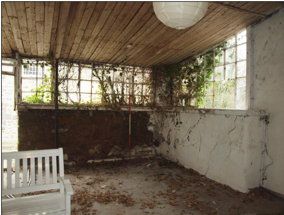
Plate 19: Western end of southwest wall showing windows
