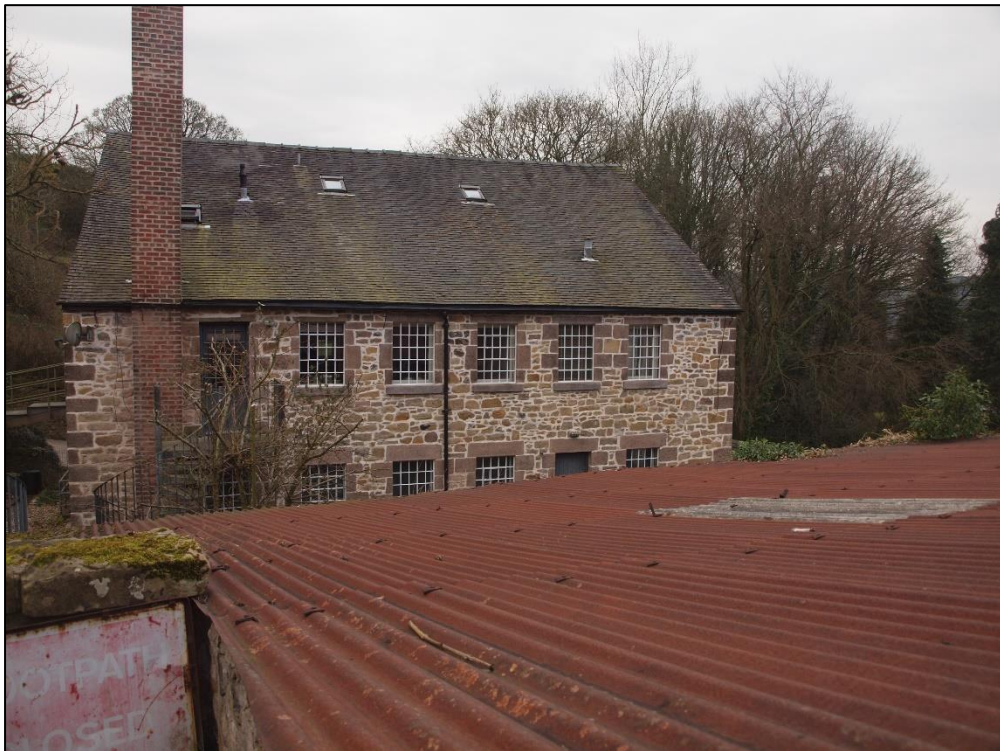
Plate 26: External shot of corrugated metal roof, showing Providence Mill beyond
