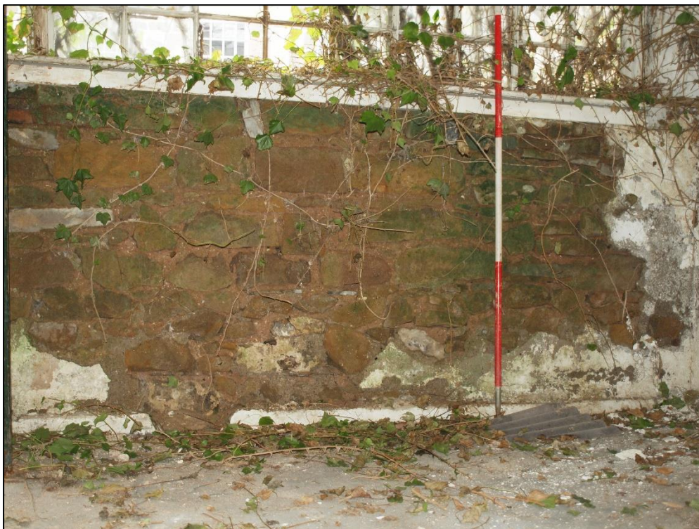
Plate 20: Detail of wall shown above, showing rough rubble construction
