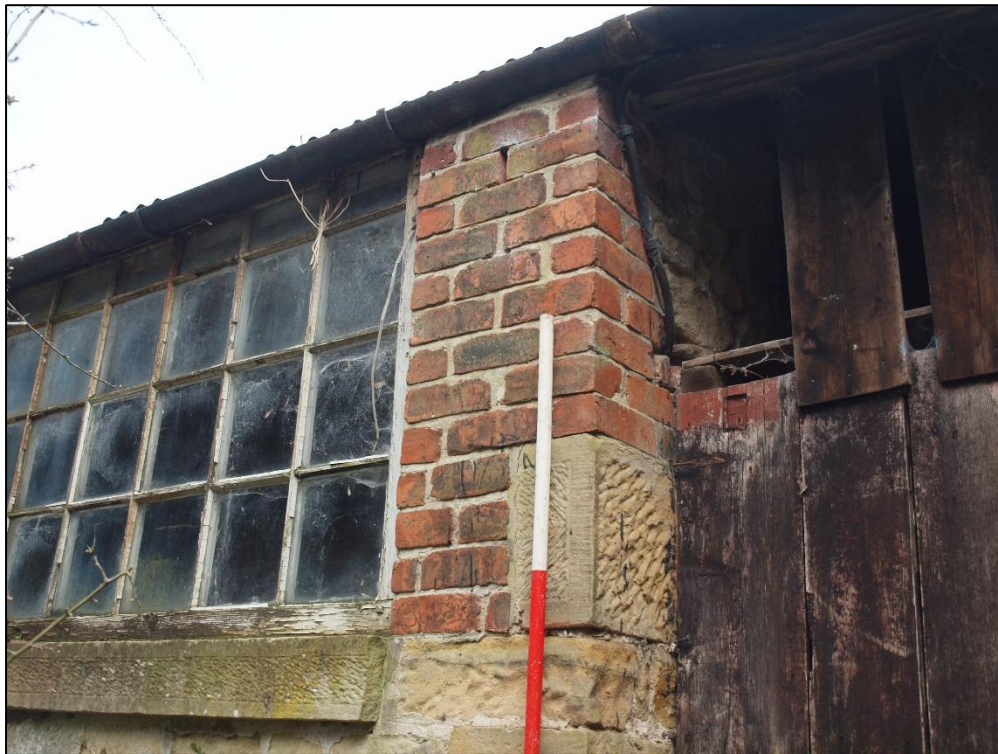
Plate 7: Detail of brick rebuilding to corner
