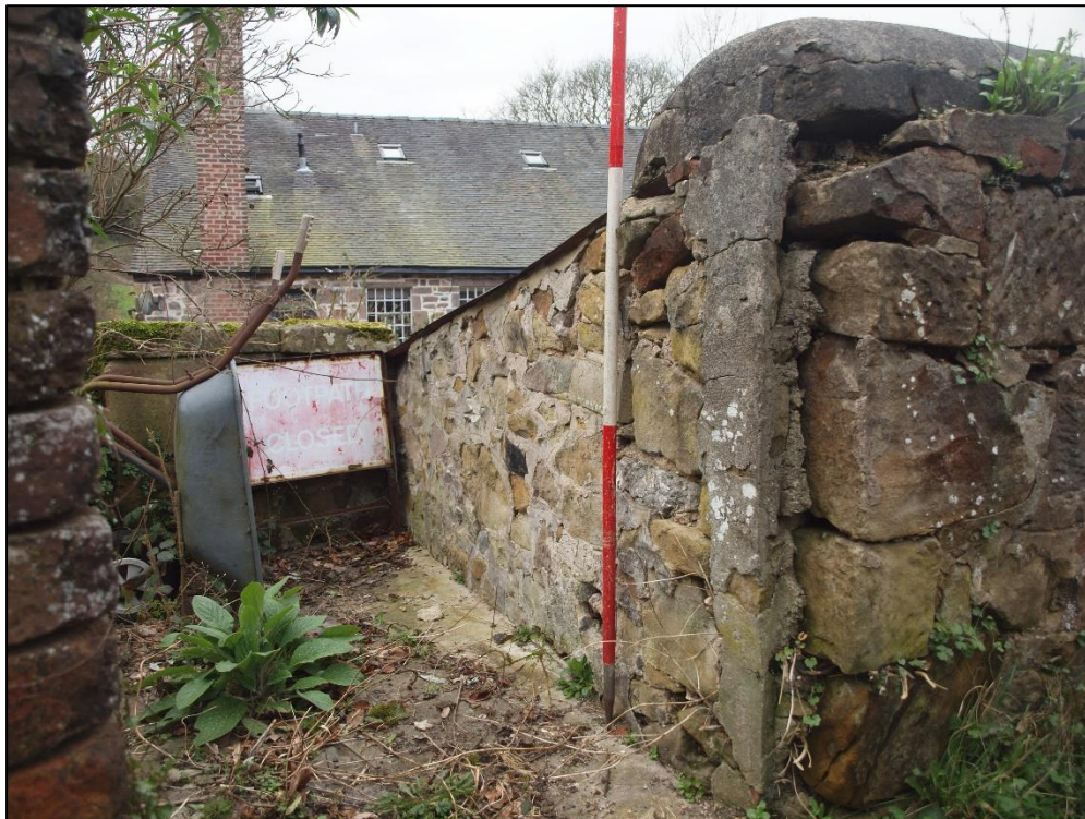
Plate 13: Southeast elevation, northern end
