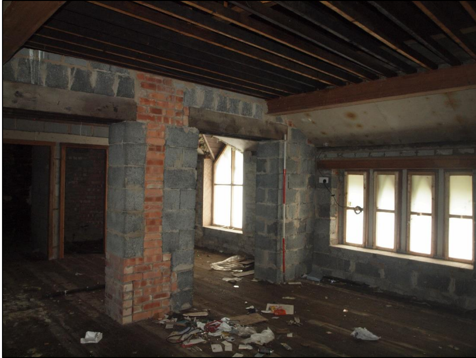
Plate 65: First floor showing southwest room
