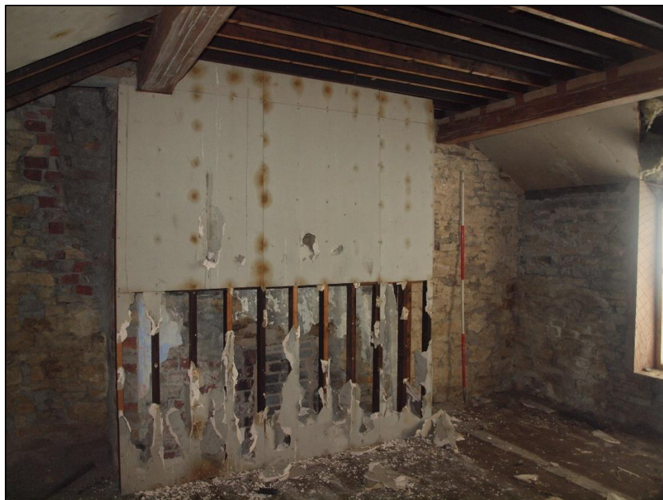
Plate 69: Stone fireplace, blocked with brick and plastered over
