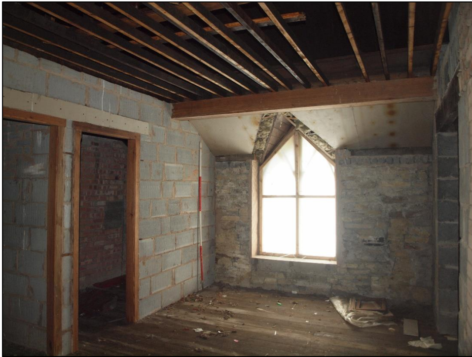
Plate 67: Stone wall to south elevation
