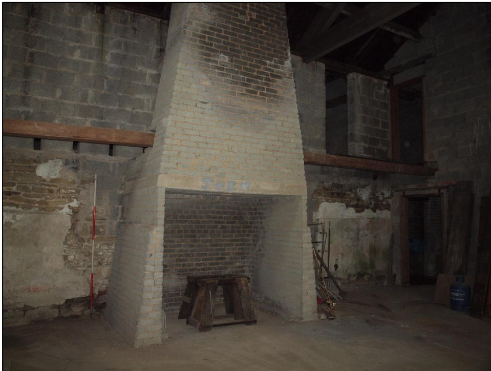
Plate 42: Inserted fireplace
