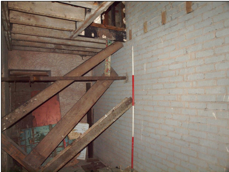
Plate 54: Room at east end fo corridor
