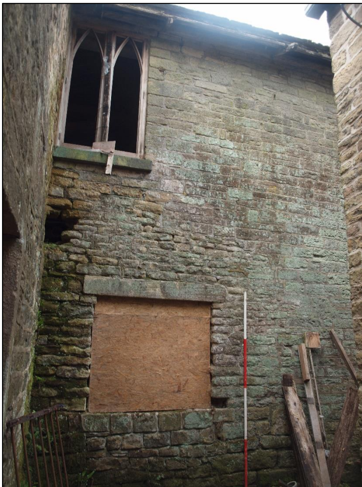
Plate 18: Northern end of east elevation
