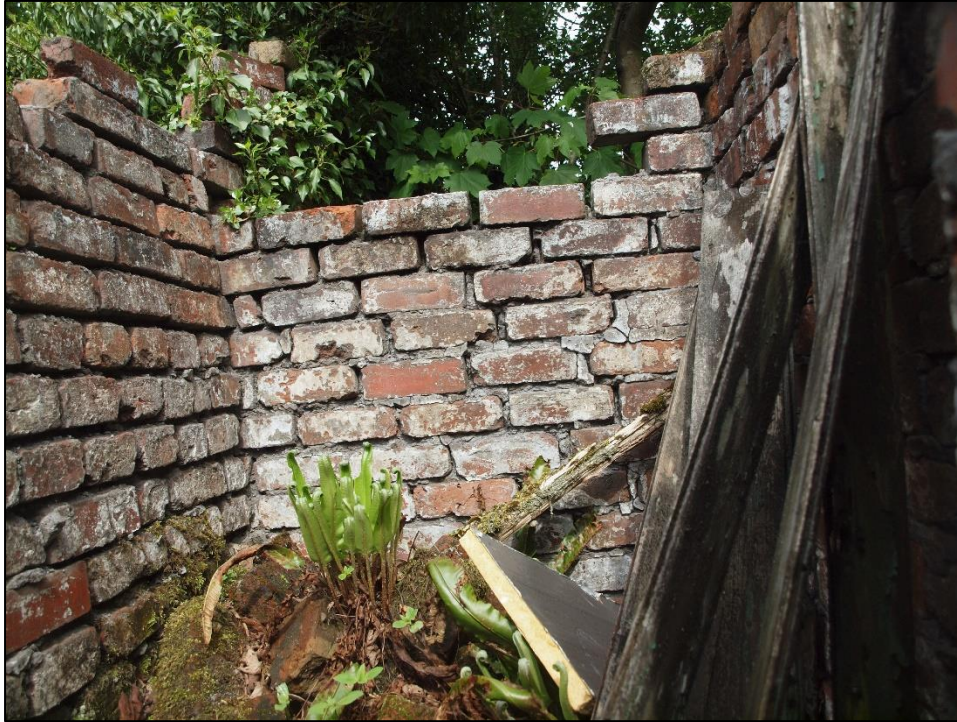
Plate 89: Interior of privy
