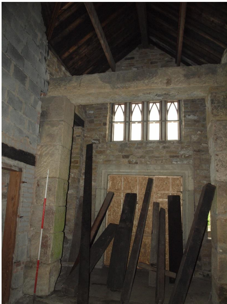
Plate 34: Porch detail showing reused stone
