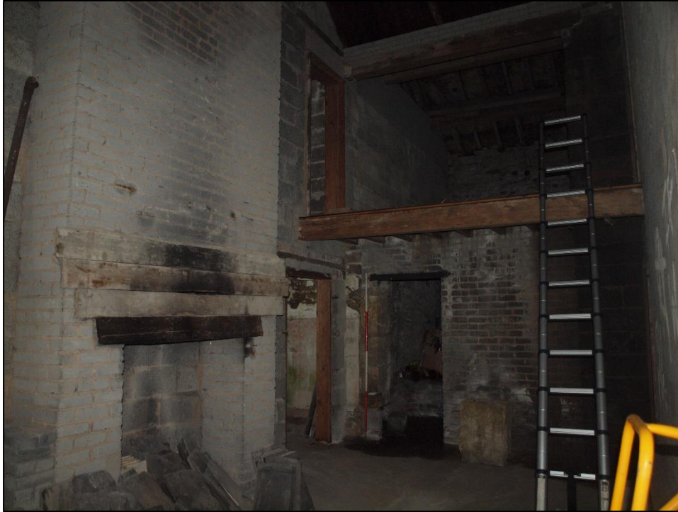
Plate 35: Corridor looking north
