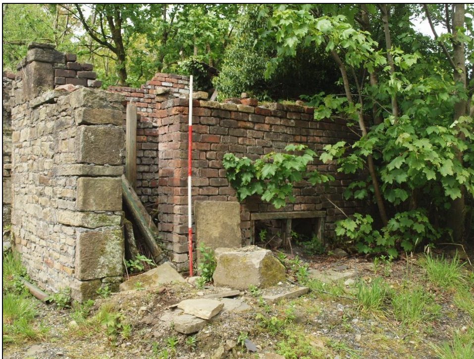
Plate 88: East elevation detail
