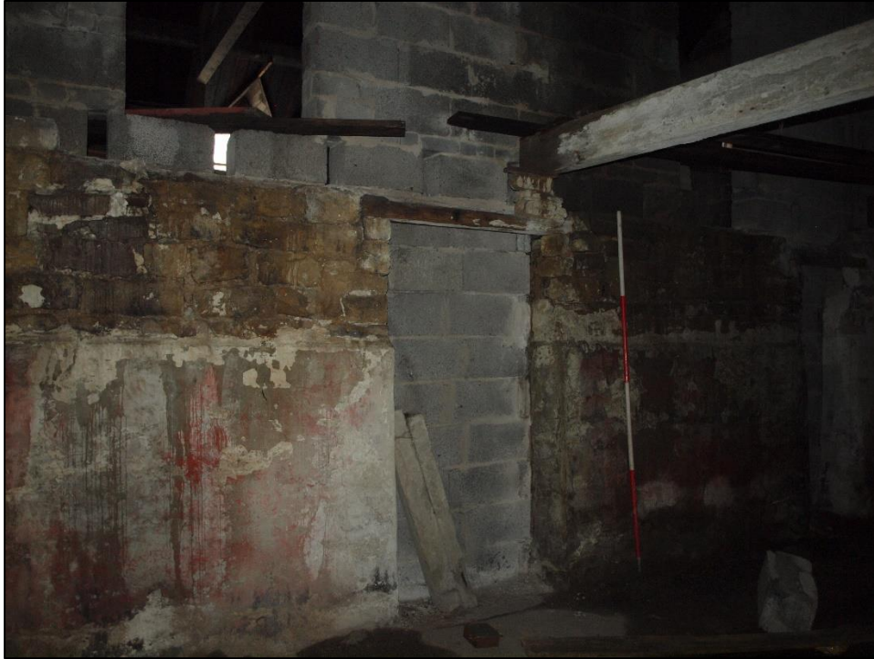
Plate 49: Blocked doorway at eastern end
