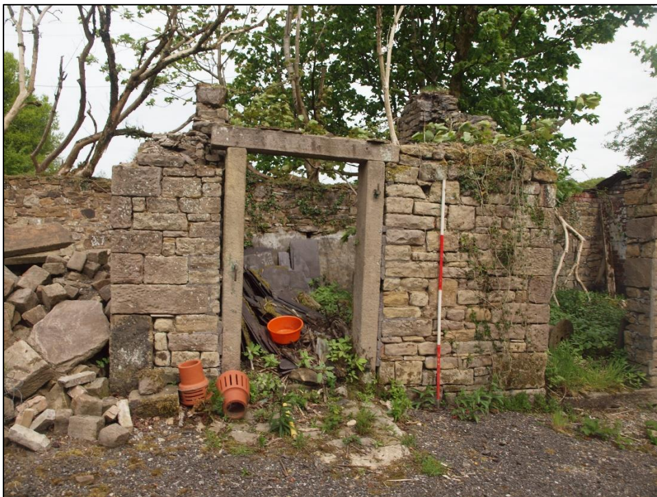
Plate 80: Doorway detail to second unit
