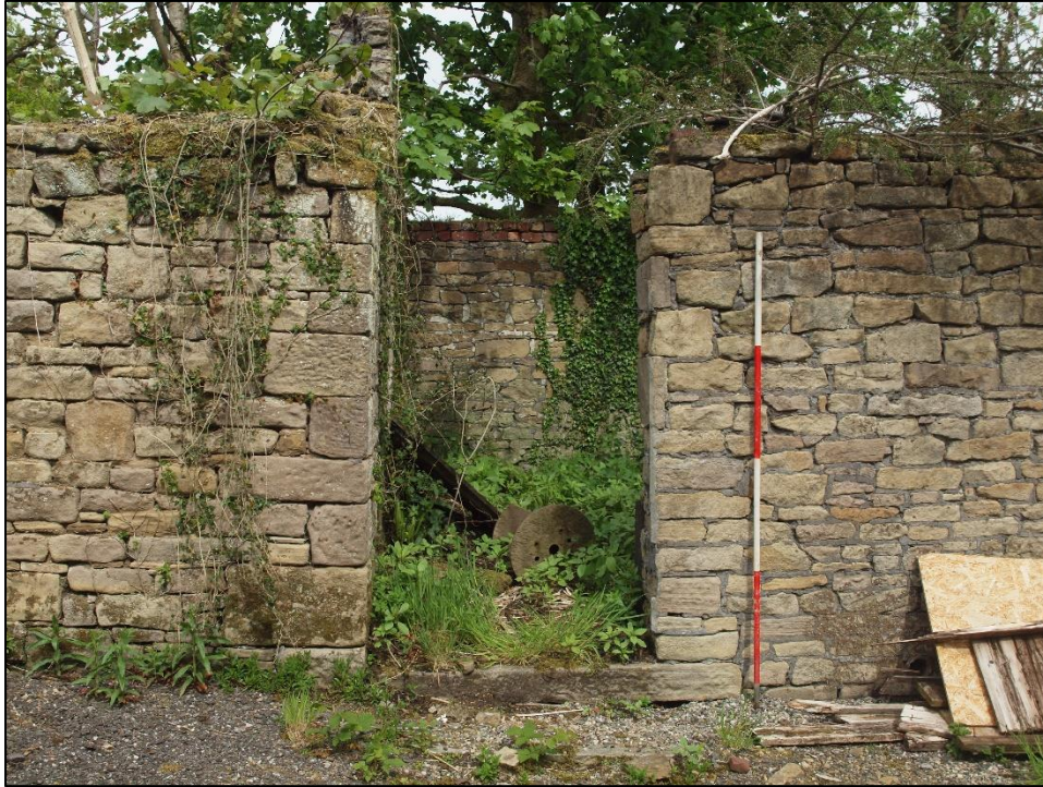
Plate 83: Doorway to third unit
