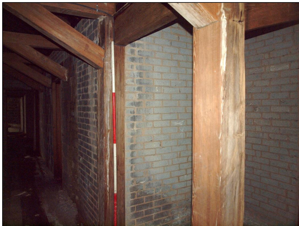
Plate 71: First floor landing showing modern timberwork
