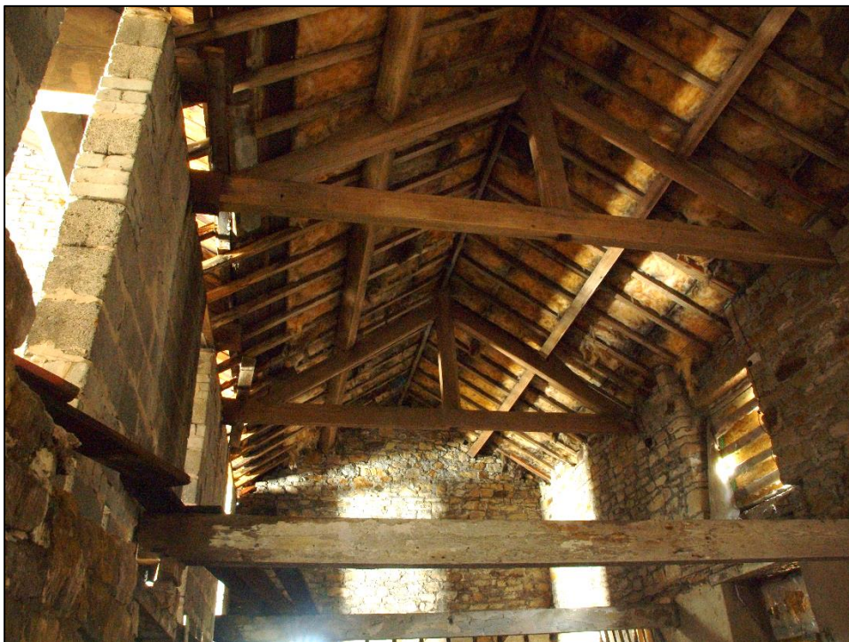
Plate 50: Machine cut timber king post trusses
