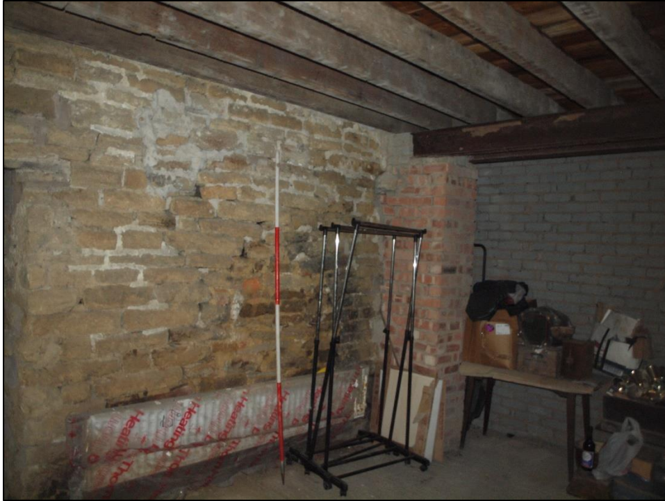
Plate 59: Room to bay 5 showing stone walls
