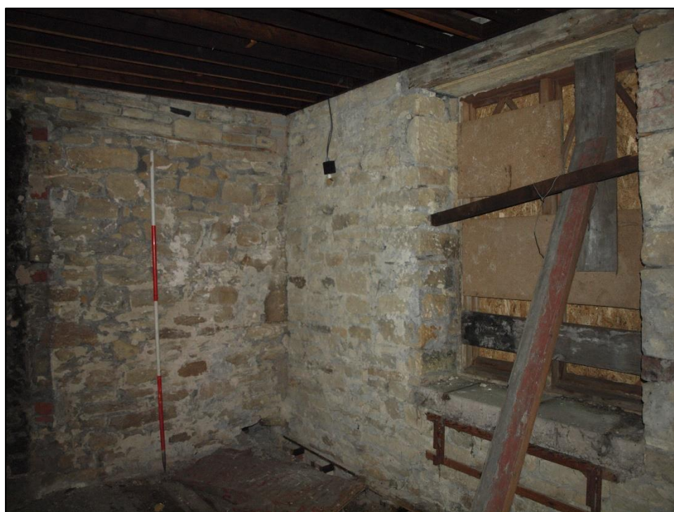
Plate 70: Room to northeast corner
