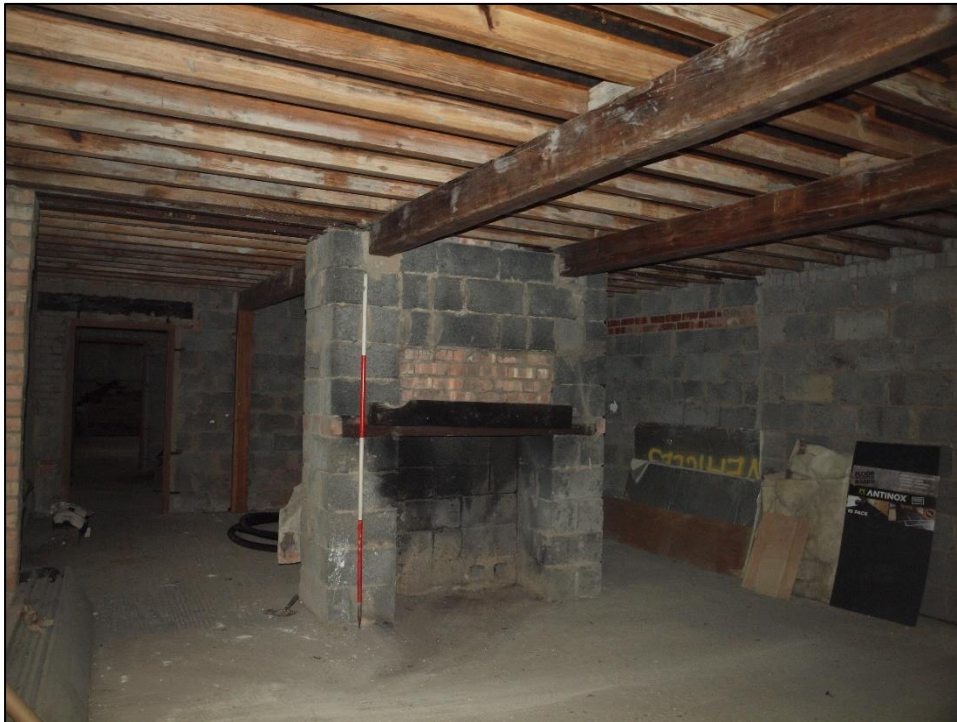
Plate 55: Large open room to southeast
