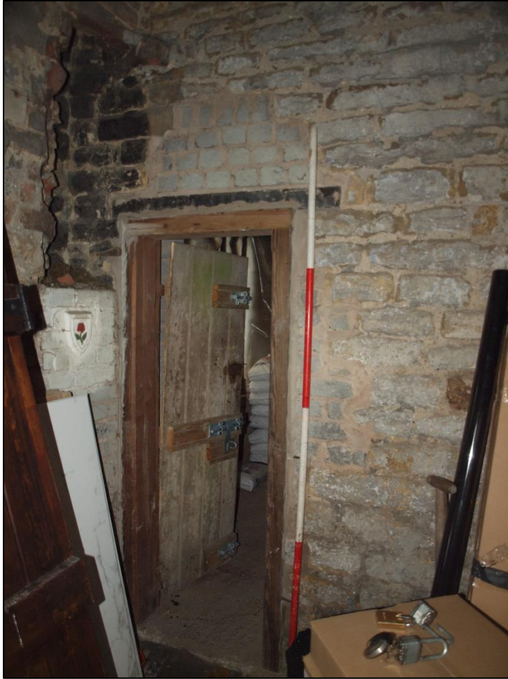
Plate 63: Inserted doorway to house
