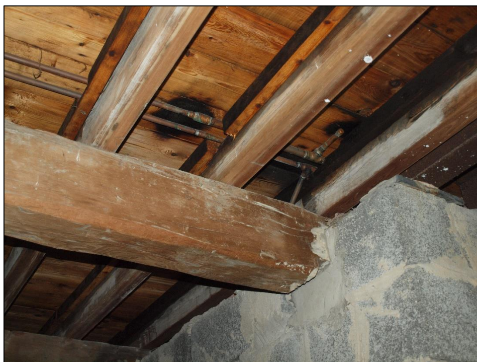
Plate 58: Modern ceiling detail
