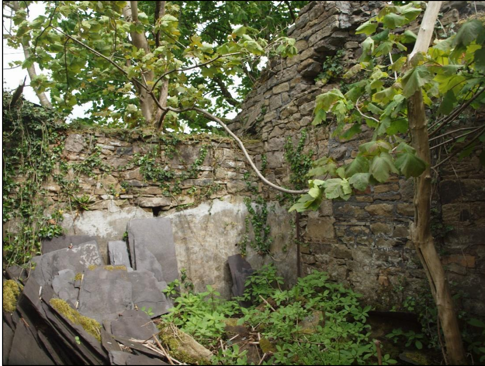
Plate 81: Interior of second unit
