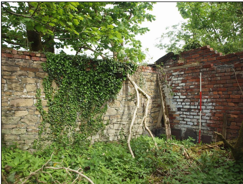
Plate 84: Interior of third unit showing inserted brick wall to the east
