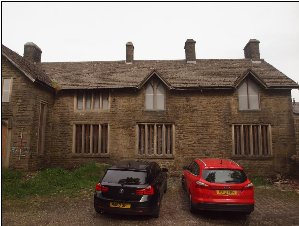
Plate 8: East end of elevation
