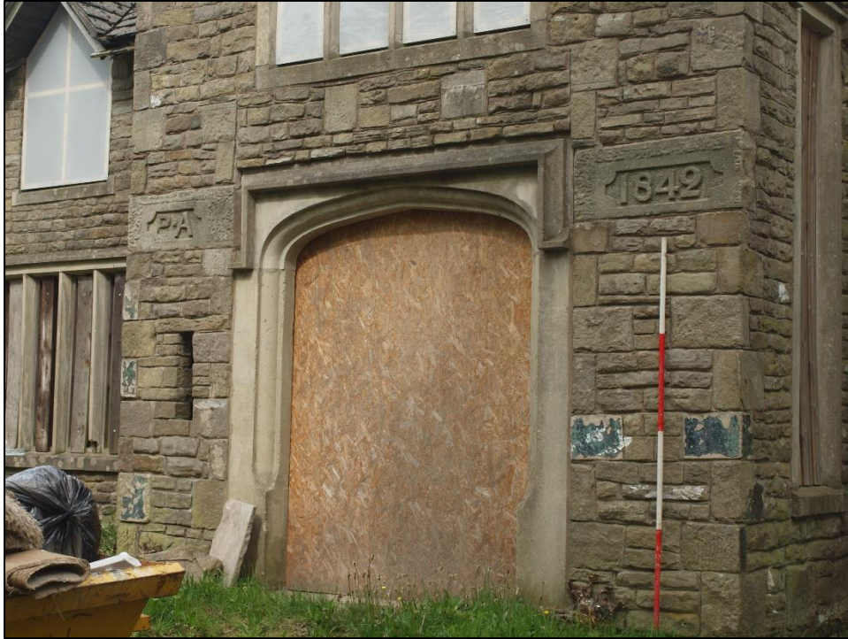
Plate 7: Detail of doorway and flanking datestones
