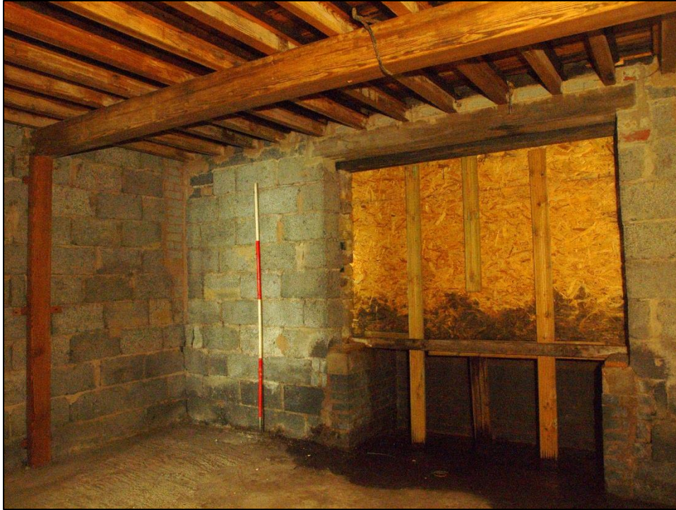
Plate 51: Inserted room northwest of east - west corridor
