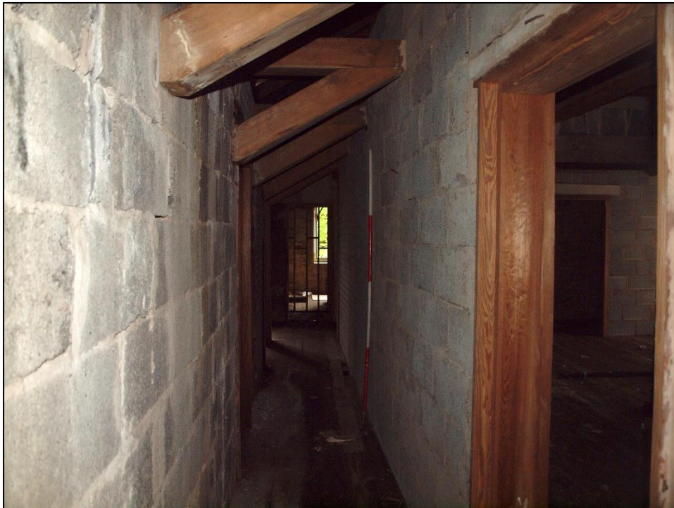
Plate 64: First floor corridor
