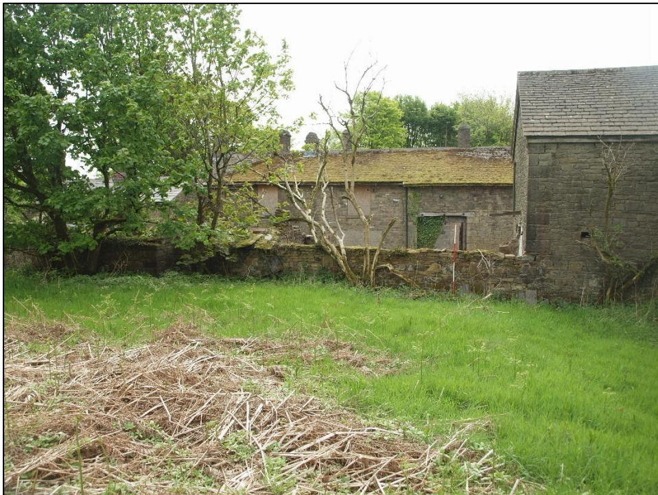
Plate 92: North elevation, west end
