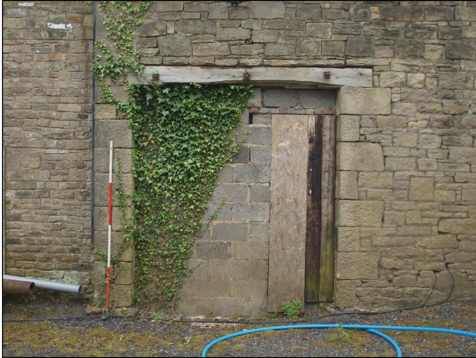
Plate 25: Detail of doorway
