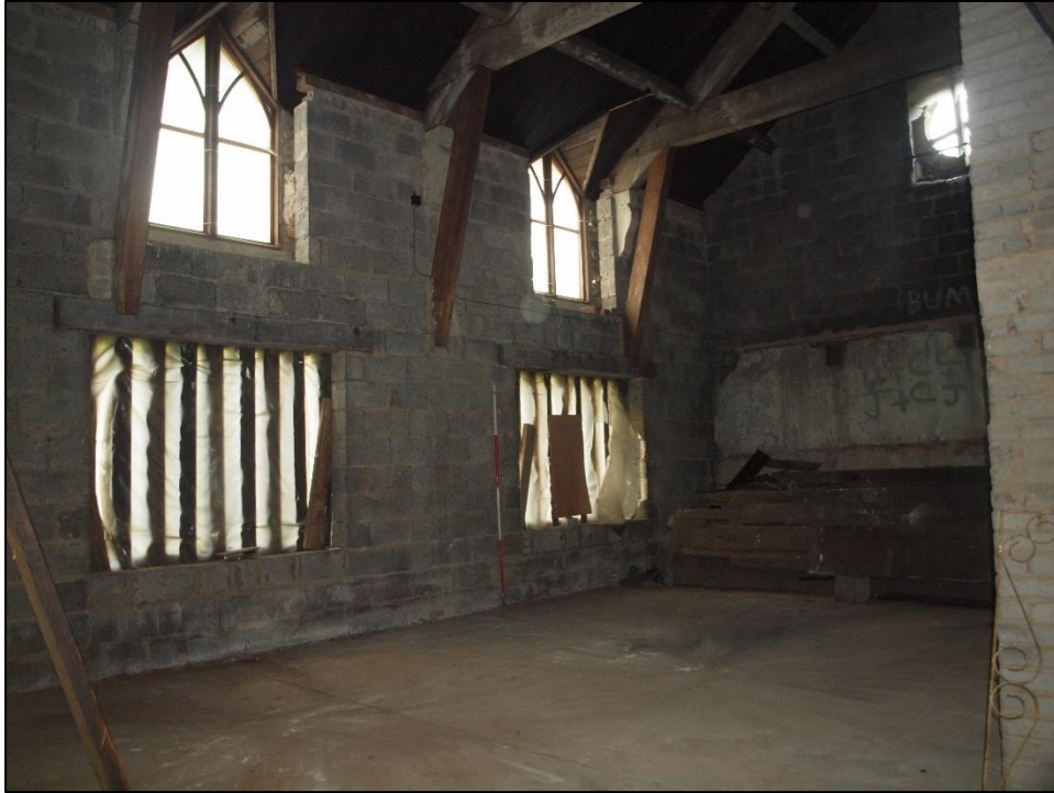
Plate 41: Large room to southwest corner
