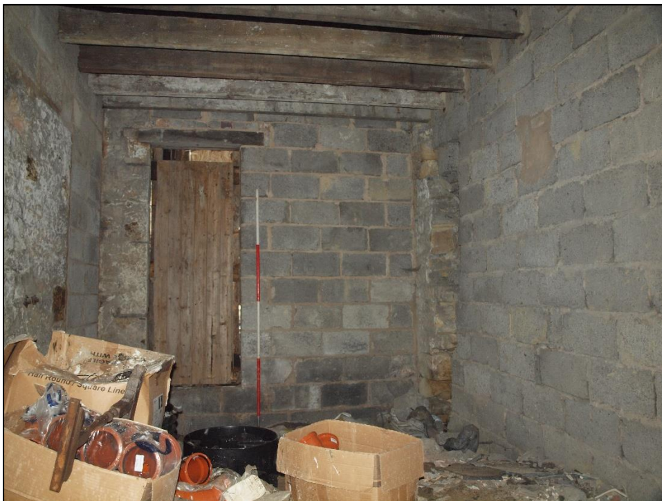
Plate 38: Room to north of corridor with raised floor
