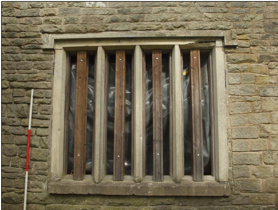
Plate 10: Detail of window
