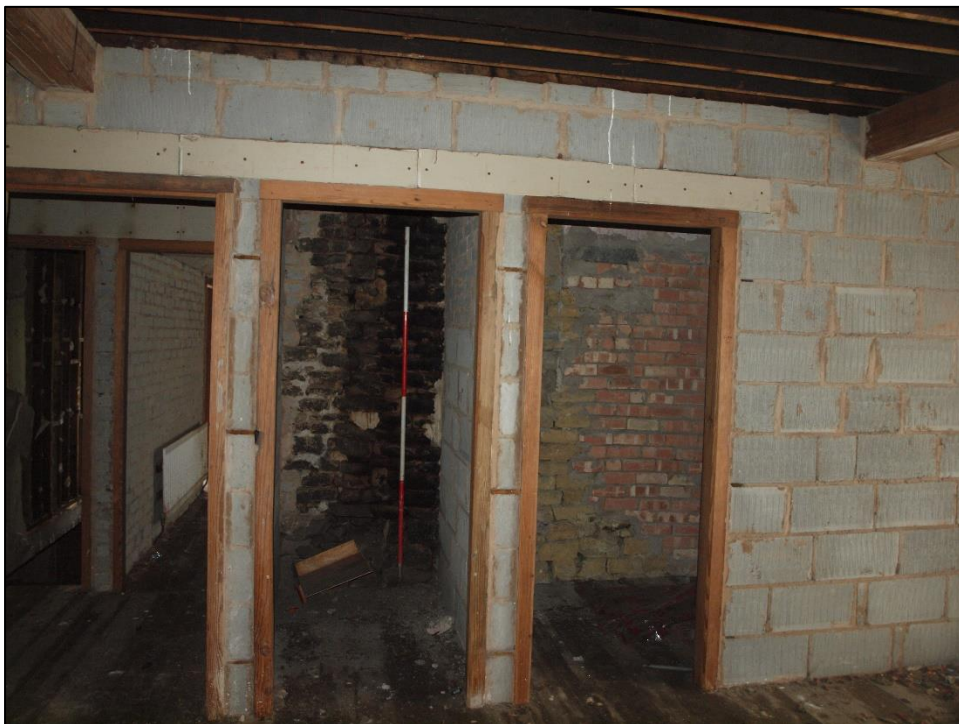
Plate 66: Inserted wall to east side showing stone and brick walls beyond
