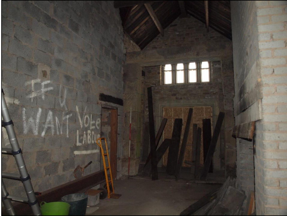
Plate 33: Central corridor showing entrance porch
