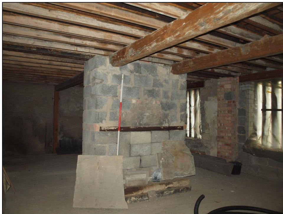
Plate 57: Inserted fireplace
