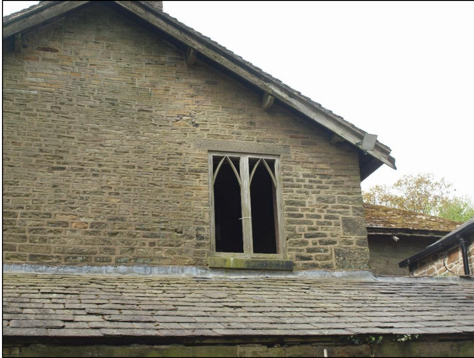
Plate 17: First floor southern gable
