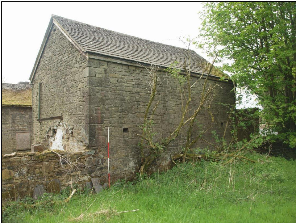
Plate 94: North elevation of barn
