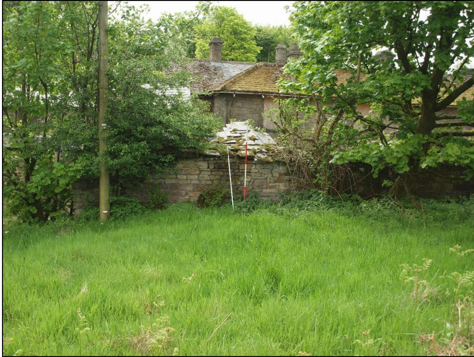
Plate 91: North elevation, east end
