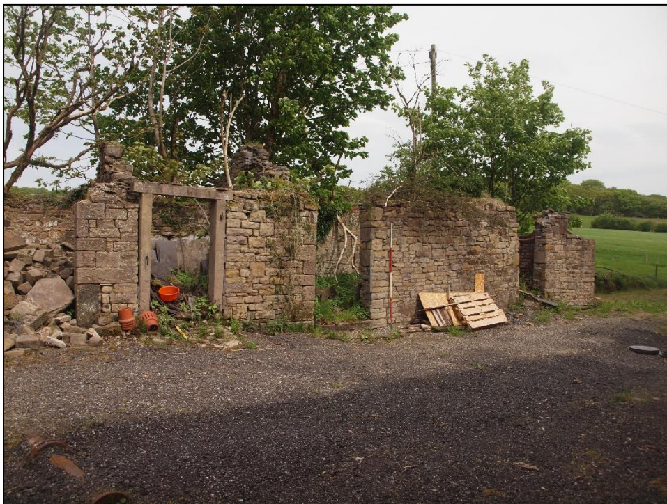
Plate 82: General shot of east end of south elevation
