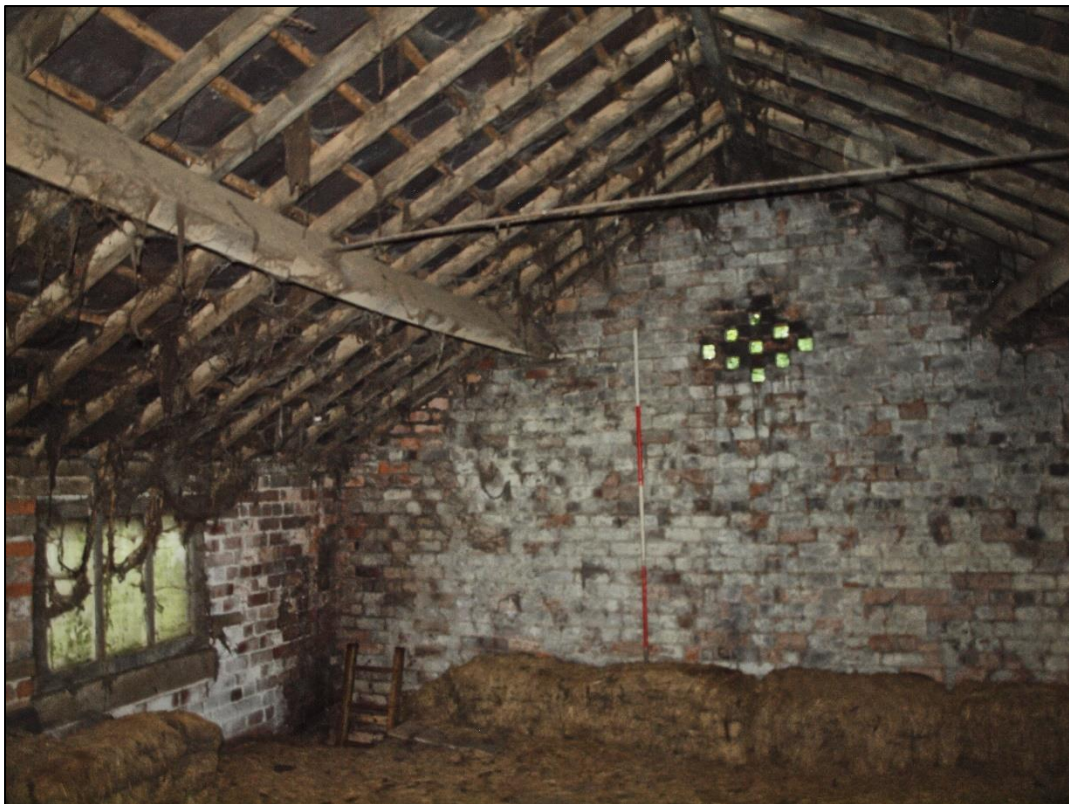
Plate 74: Eastern unit looking east, showing hatch to corner
