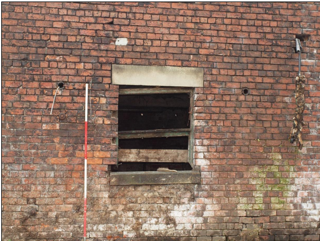
Plate 62: Window to western unit
