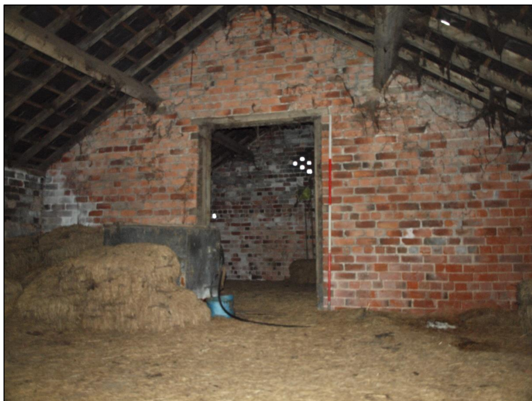
Plate 72: First floor showing doorway in cross wall
