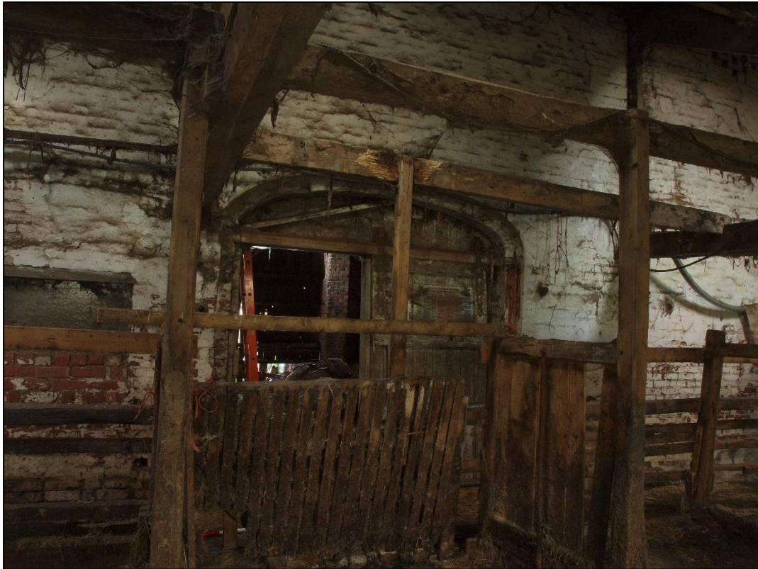
Plate 43: Timber stall with barn door behind
