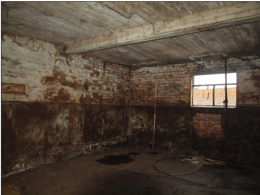
Plate 70: Eastern unit looking southeast
