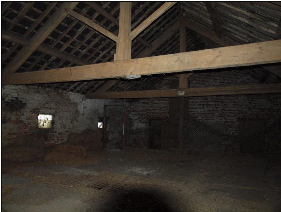
Plate 52: First floor looking west
