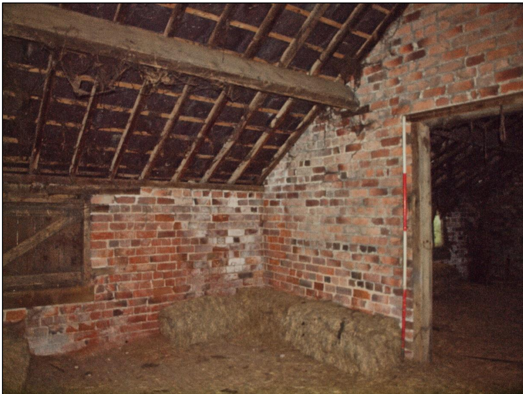
Plate 76: Western unit showing pitching eye
