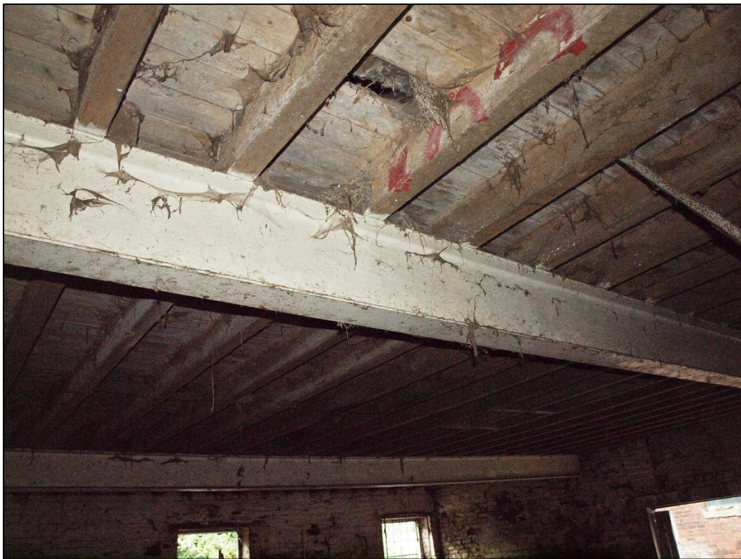
Plate 32: Detail of steel beam and modern timber boards and joists
