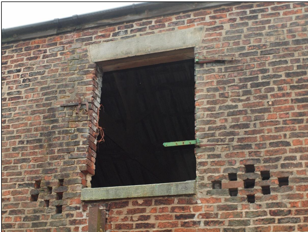
Plate 10: Inserted doorway to first floor bay 5
