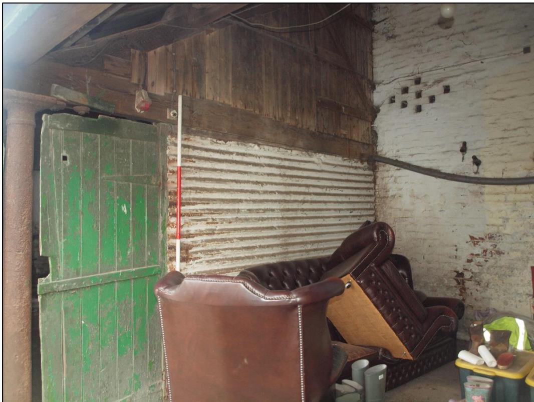
Plate 48: Inserted timber wall to northern side as seen above
