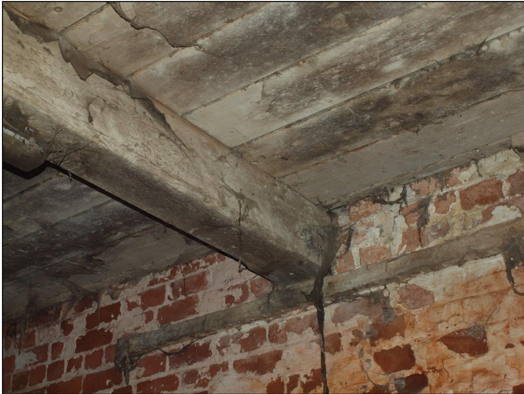
Plate 69: Detail of chamfered and stopped timber beam
