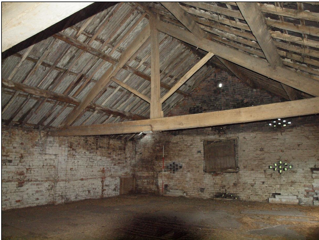
Plate 50: First floor of barn, looking northeast showing kingpost truss
