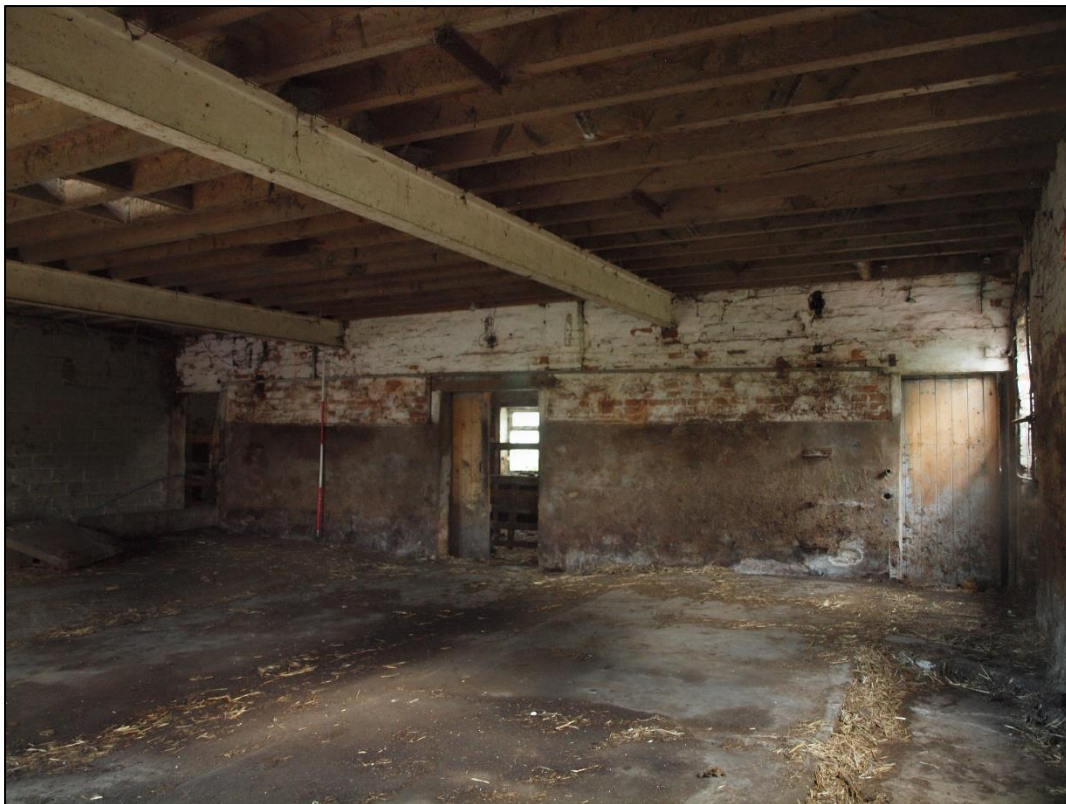
Plate 30: Inserted doorways in north wall into lean-to
