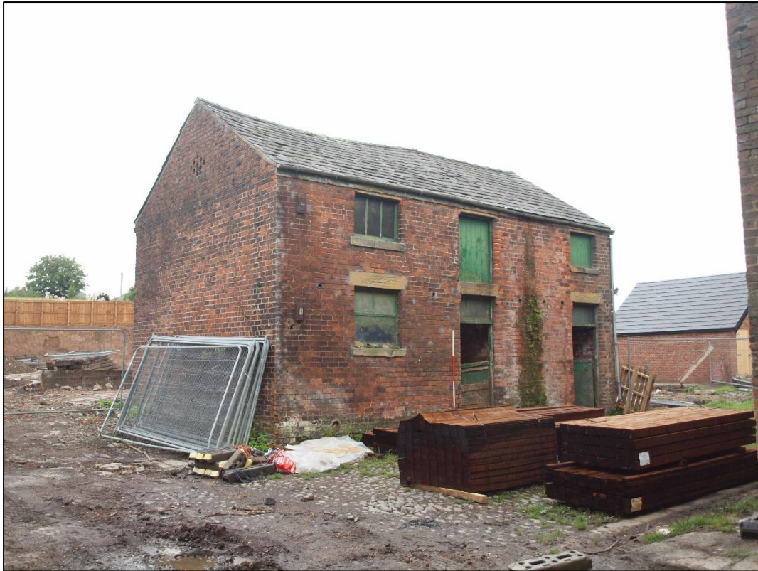
Plate 55: North elevation of barn 2
