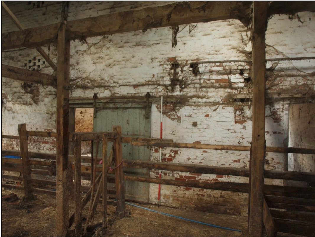
Plate 45: Whitewashed walls and inserted doorways to barn
