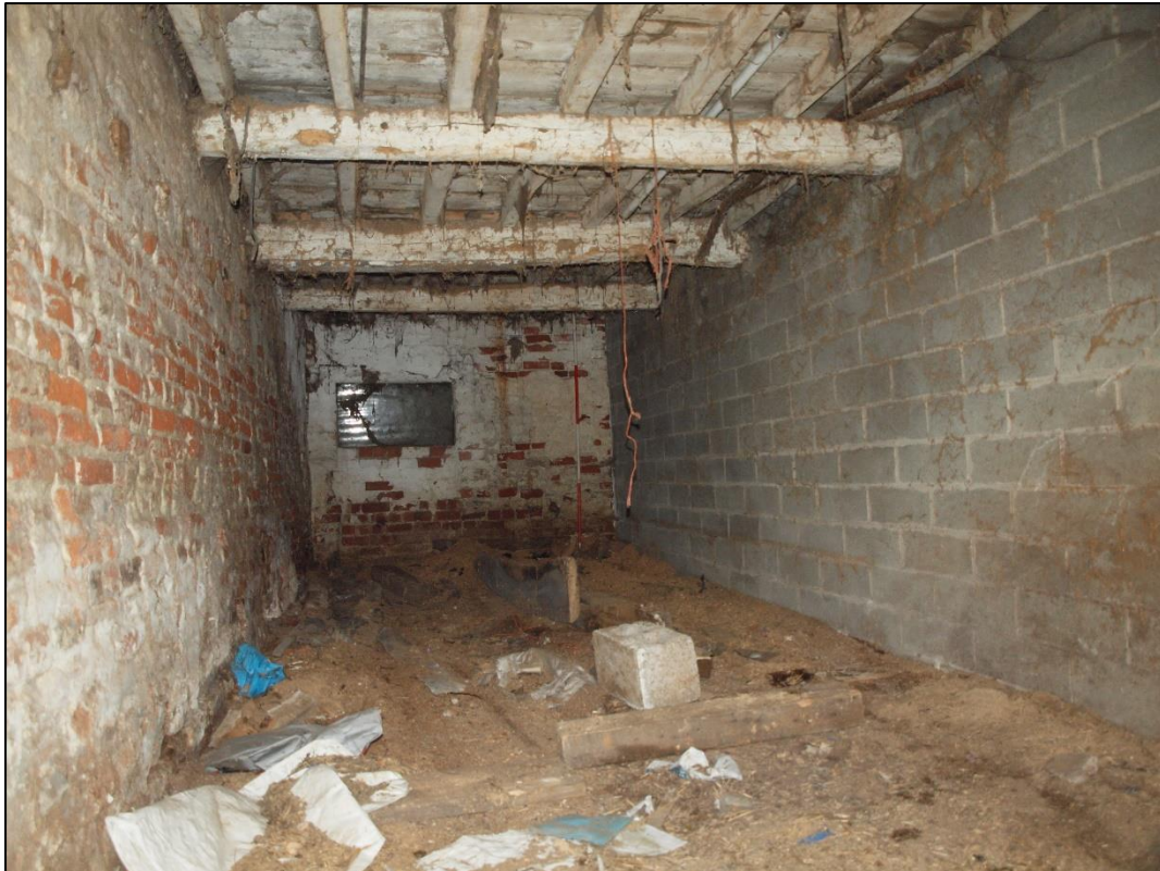
Plate 33: Inserted storage area to bay 3 showing reused beams
