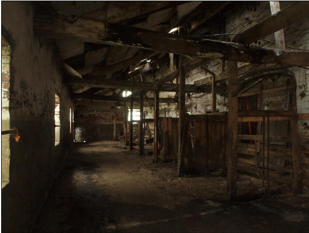
Plate 41: Lean-to looking east showing timber stalls
