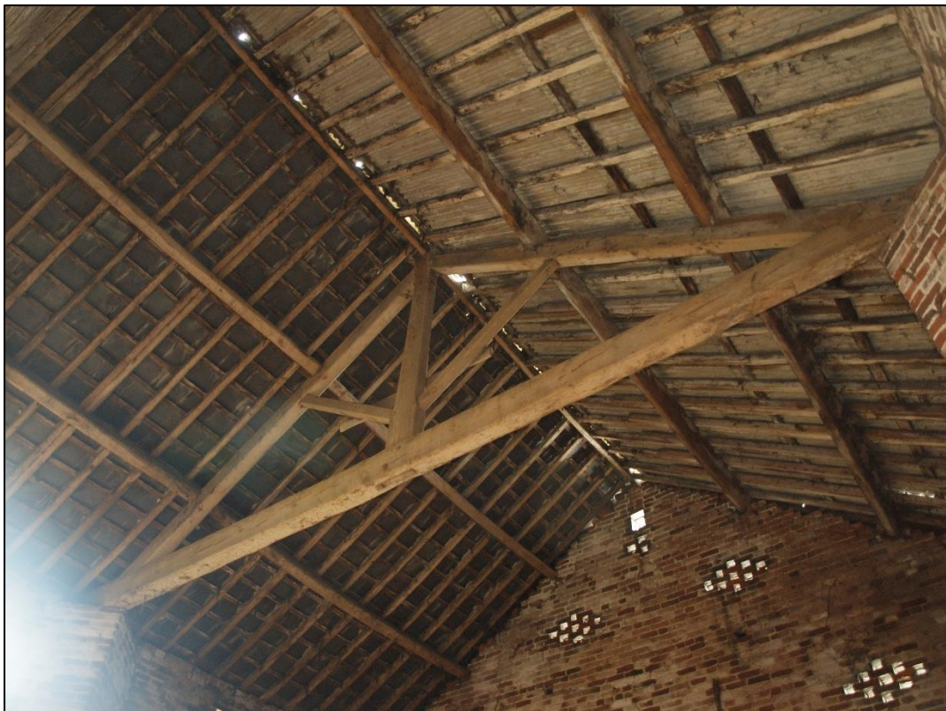
Plate 40: King post truss and roof structure
