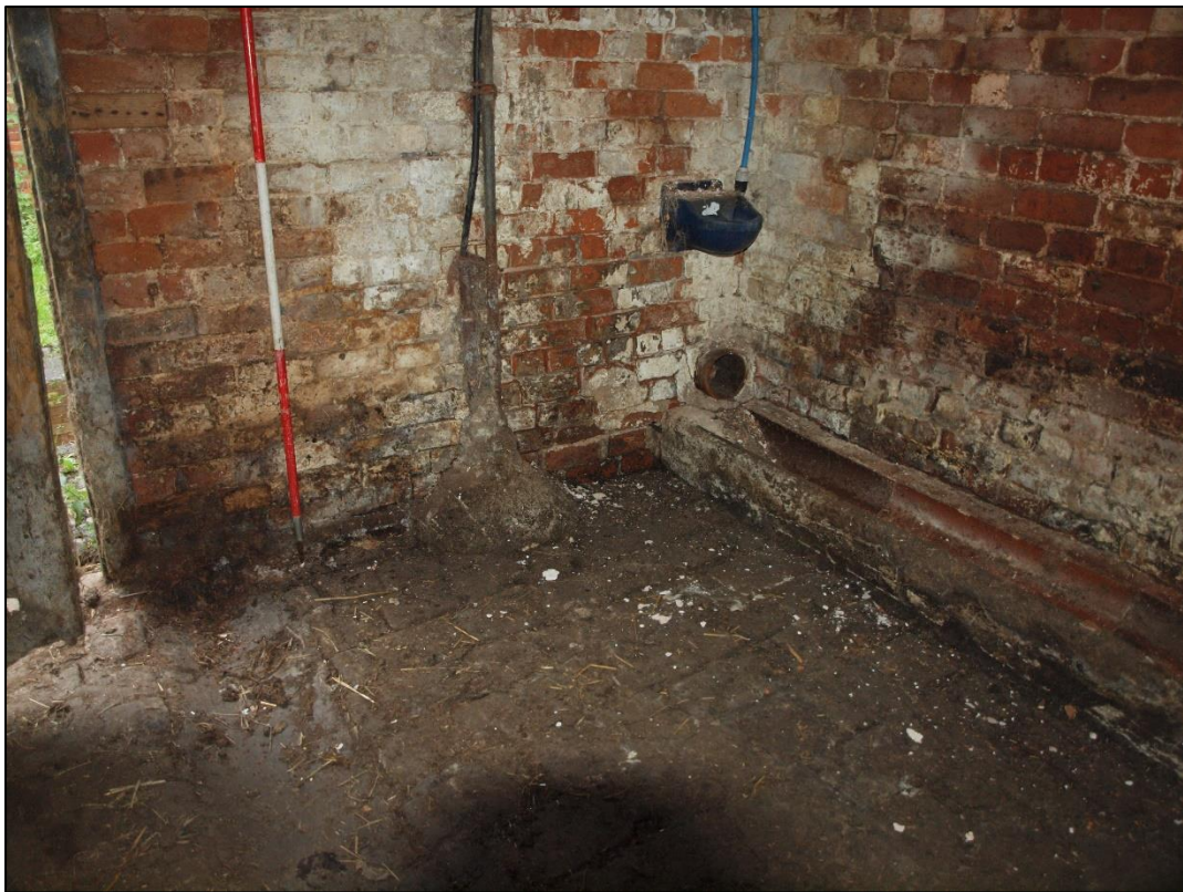
Plate 68: Inserted drain and cobbled floor
