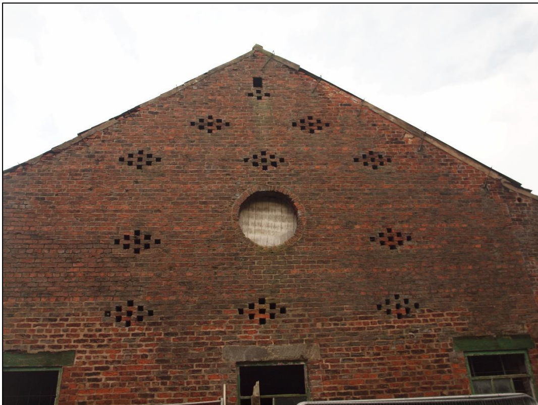
Plate 12: Detail of first floor ventilation slots
