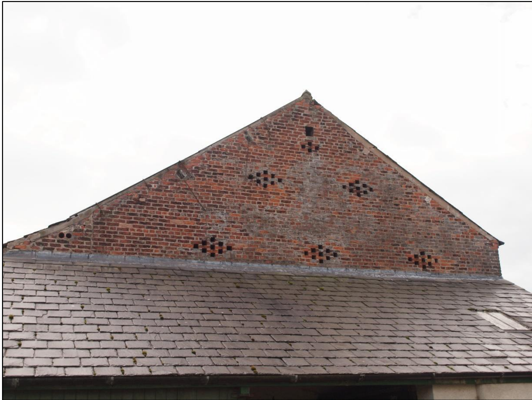
Plate 27: Detail of gable at first floor level
