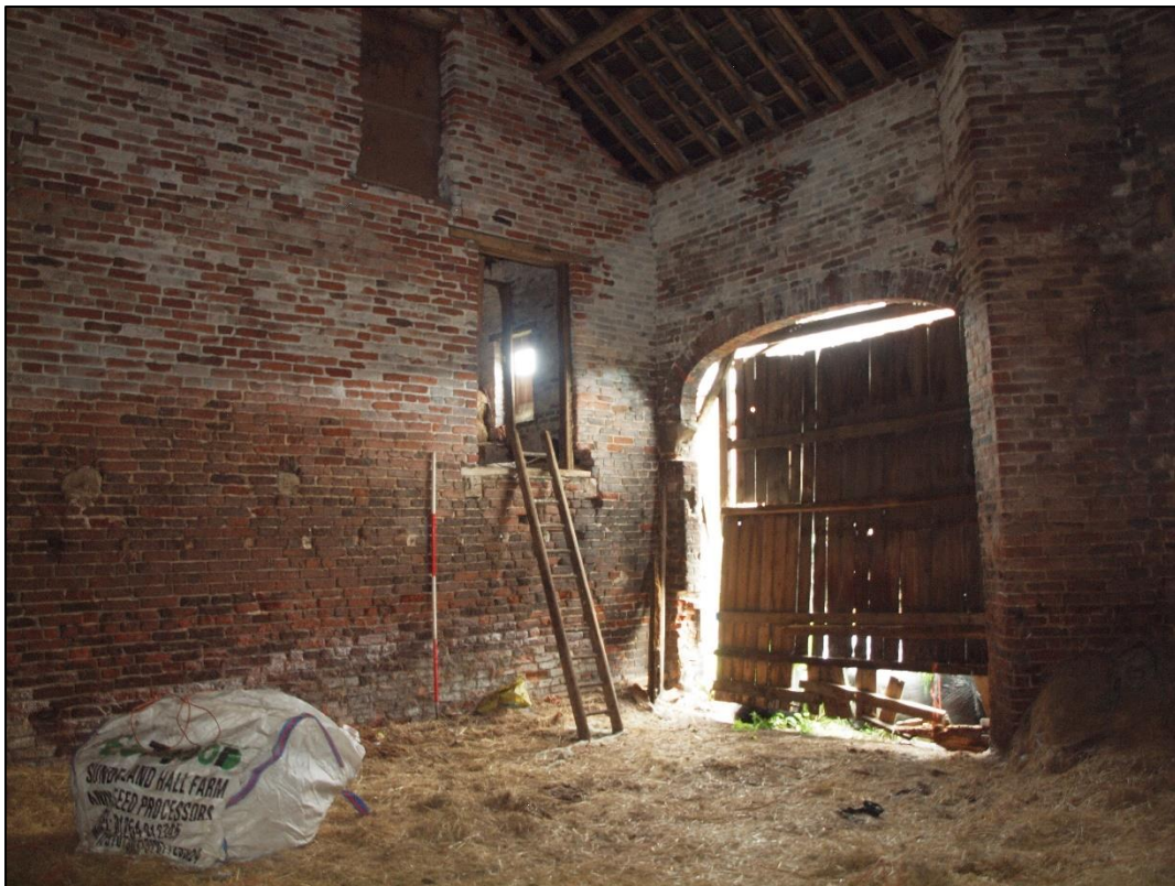
Plate 38: Barn door to south elevation
