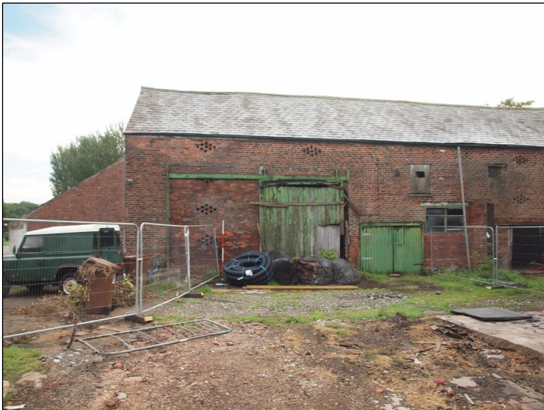
Plate 2: Barn 1 south elevation, western end
