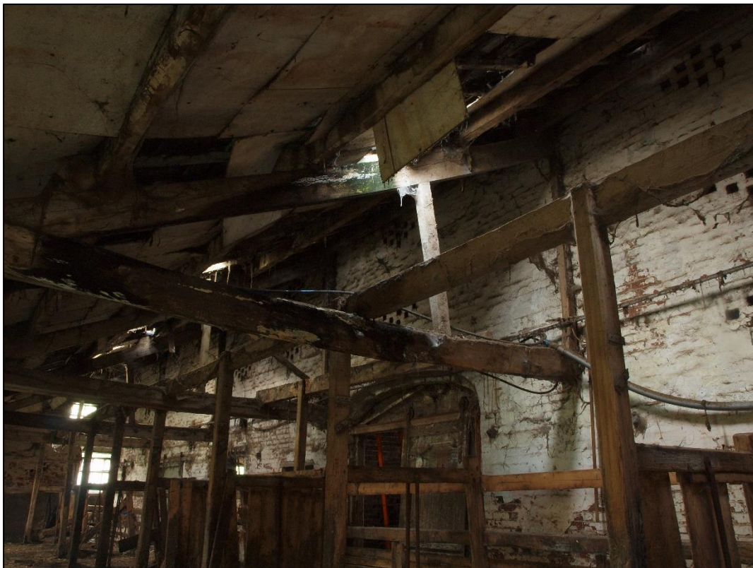
Plate 42: Brace truss roof structure
