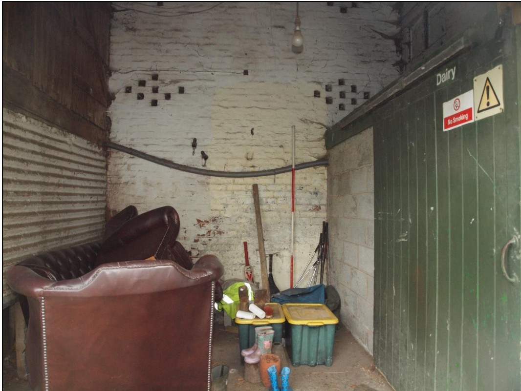
Plate 47: Central area of extension, open fronted, showing whitewashed barn wall
