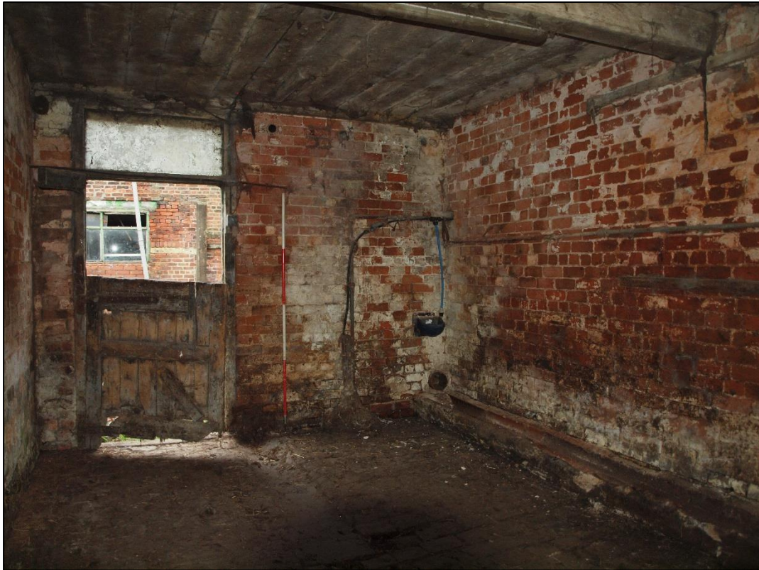
Plate 67: Western unit looking north
