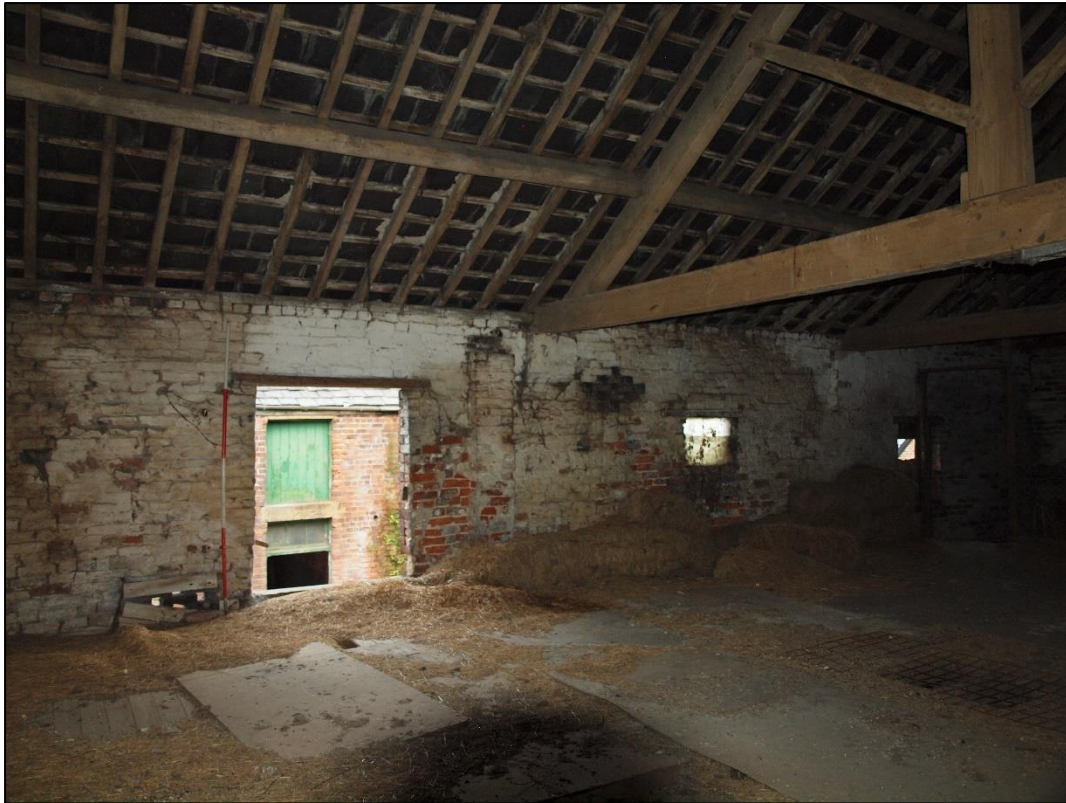
Plate 51: First floor showing inserted doorway to south
