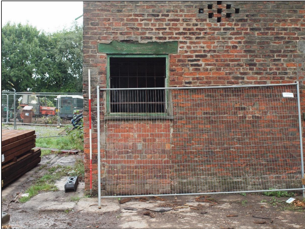
Plate 13: Blocked doorway at southern end
