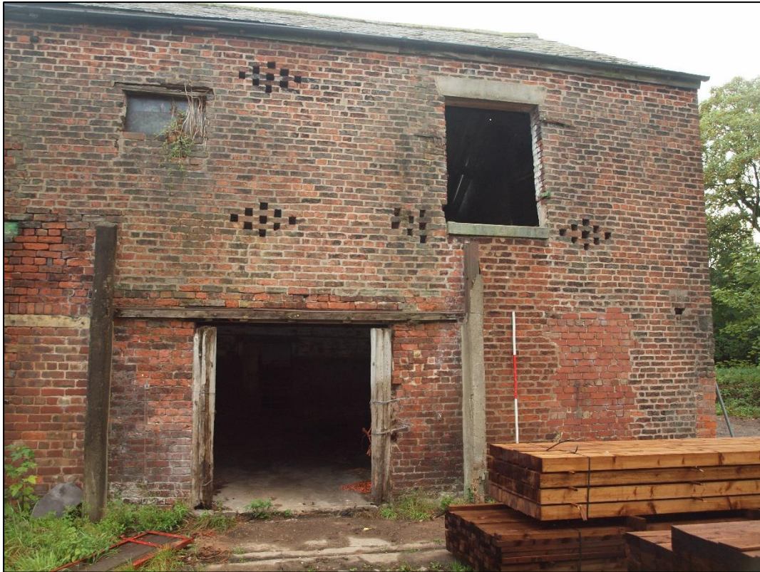
Plate 7: Doorway to bay 4
