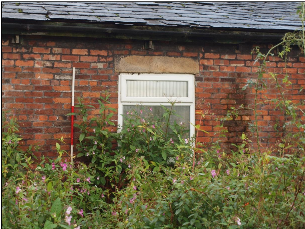
Plate 22: Detail of window
