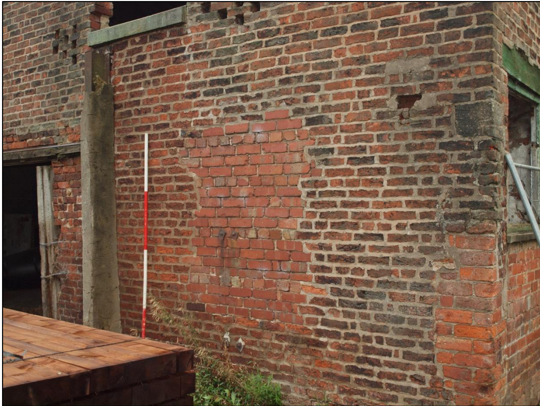
Plate 9: Blocked window to bay 5
