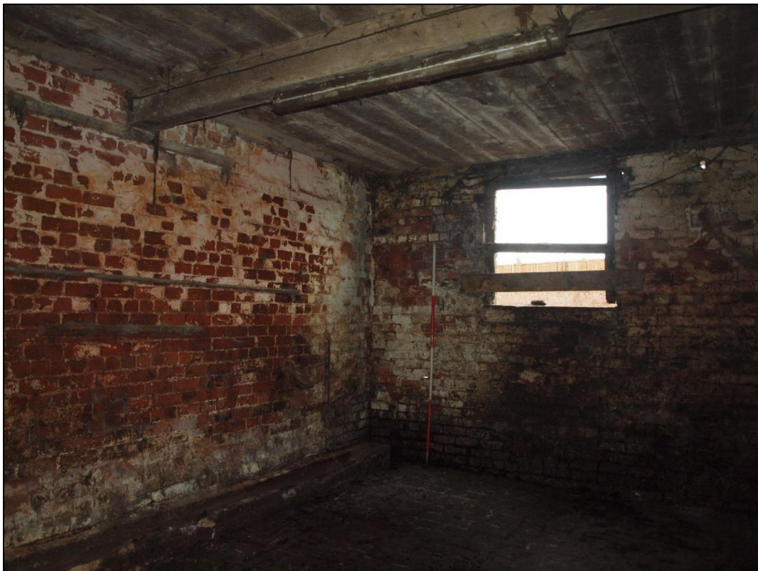
Plate 66: Western unit looking south
