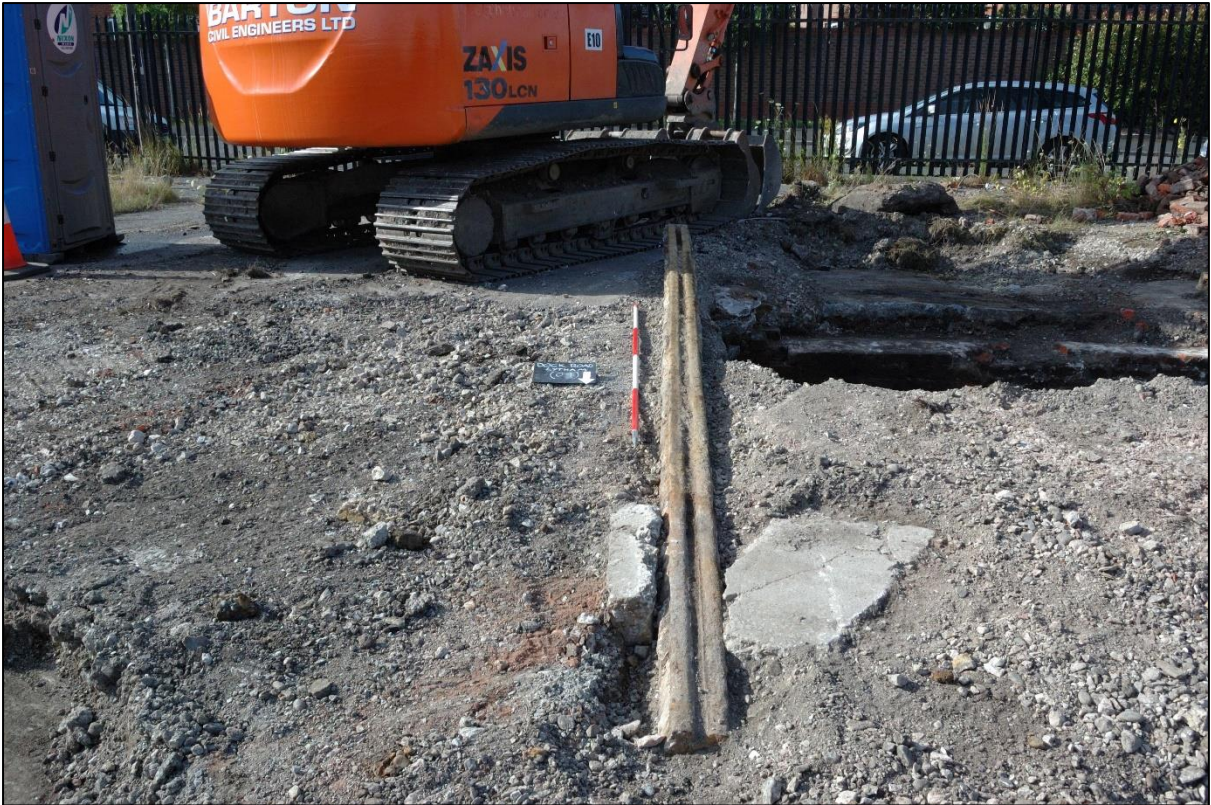
Plate 15: Grooved cast iron rail [09]
