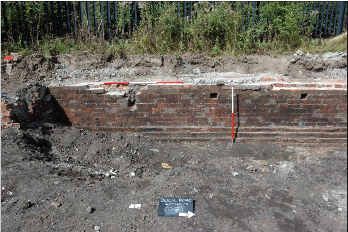
Plate 6: Stepped foundation of wall [07]
