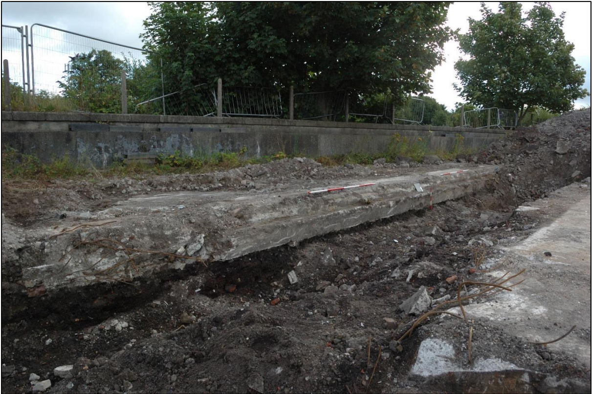
Plate 1: Stepped concrete sill [05]
