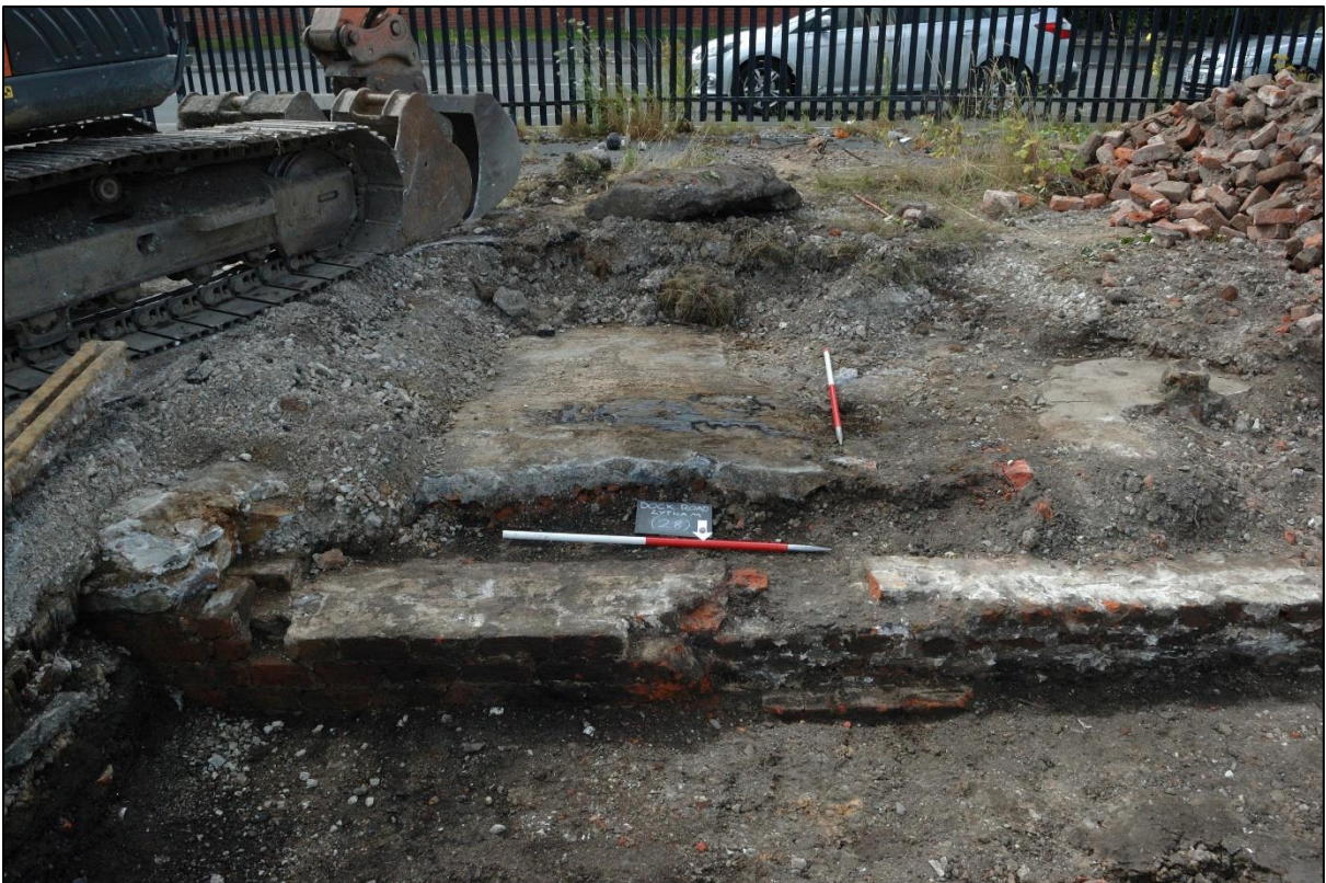
Plate 26: Concrete with bitumen [28]
