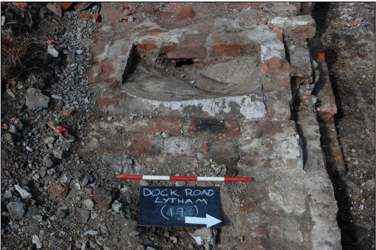
Plate 24: Concrete and brick drain [19]
