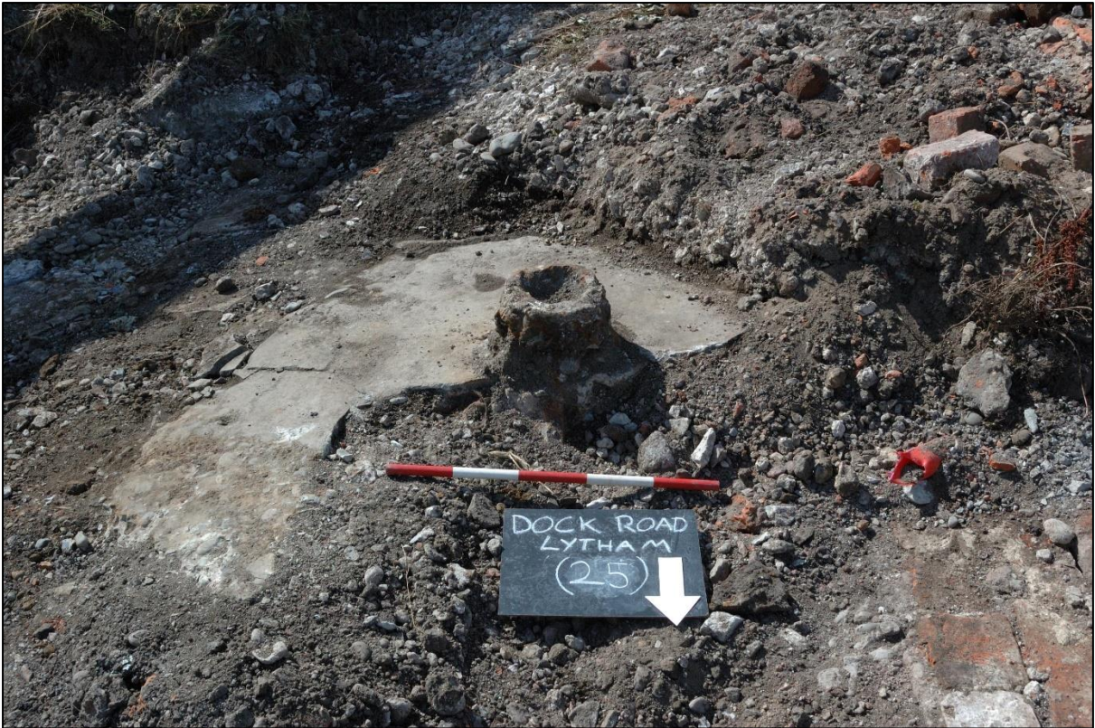
Plate 25: Cast iron stanchion within concrete floor [25]
