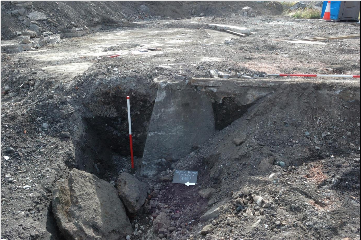
Plate 13: Concrete pillar [11] north of rail [10] above
