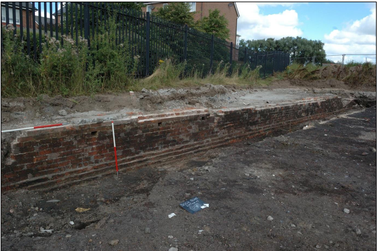
Plate 4: Wall [07] looking north
