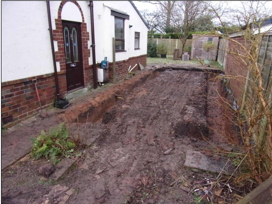
Plate 1: General shot of site looking south
