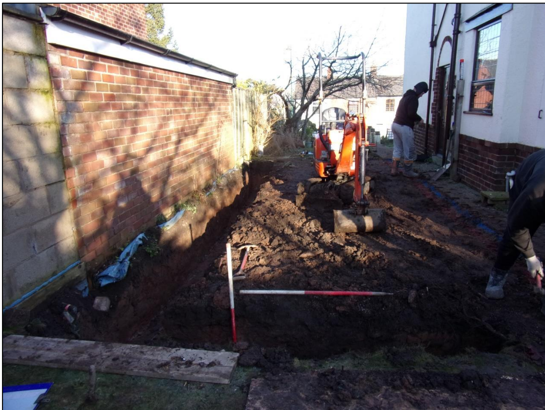
Plate 12: Working shot looking north
