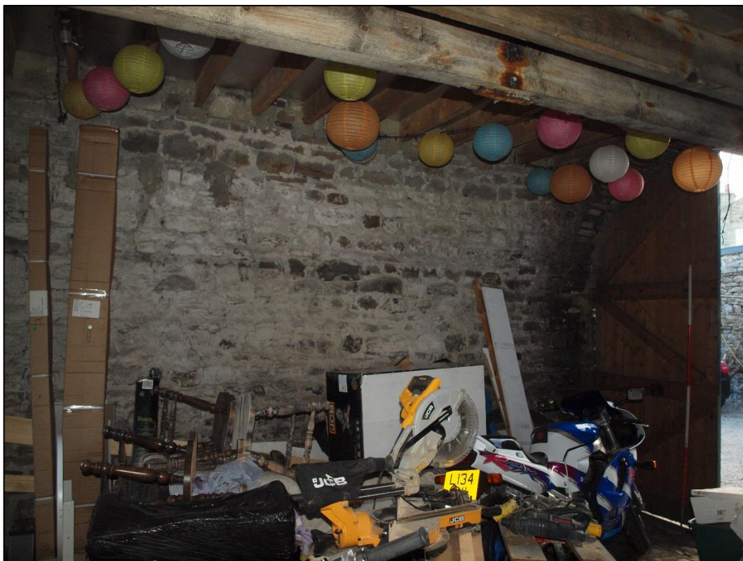
Plate 38: General shot showing whitewashed walls looking southeast
