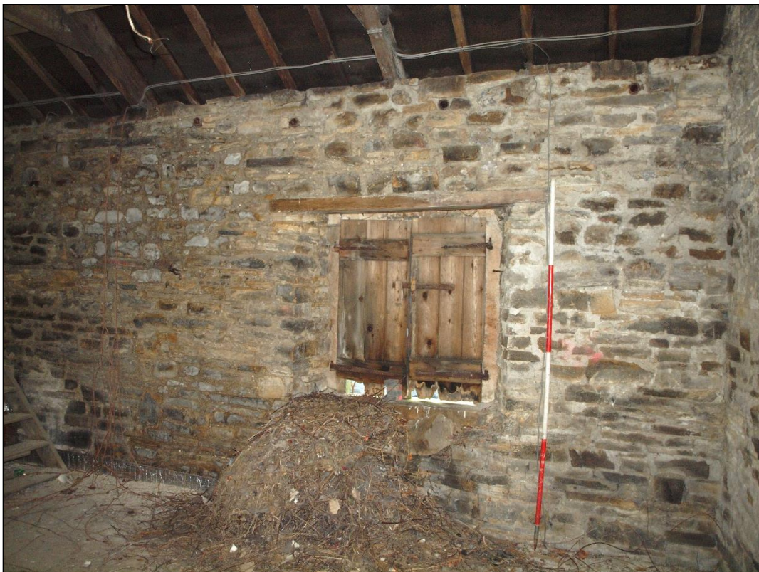
Plate 62: Pitching eye to south elevation looking south
