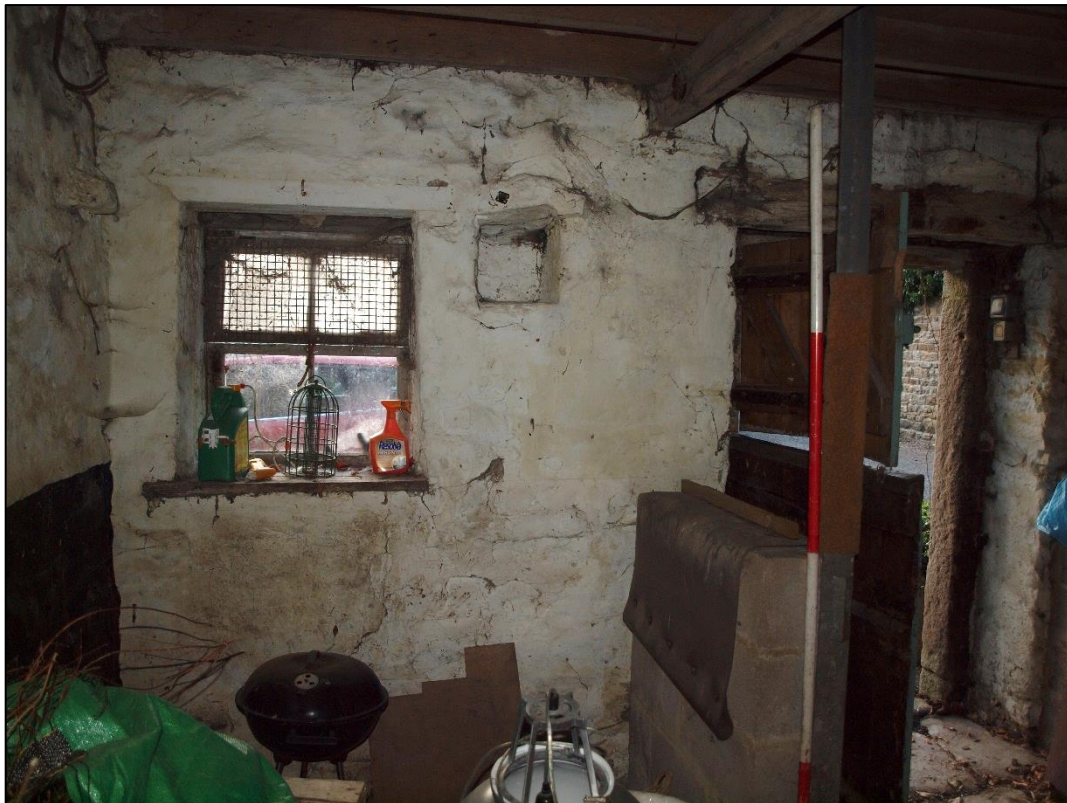
Plate 43: Southern wall showing window and doorway
