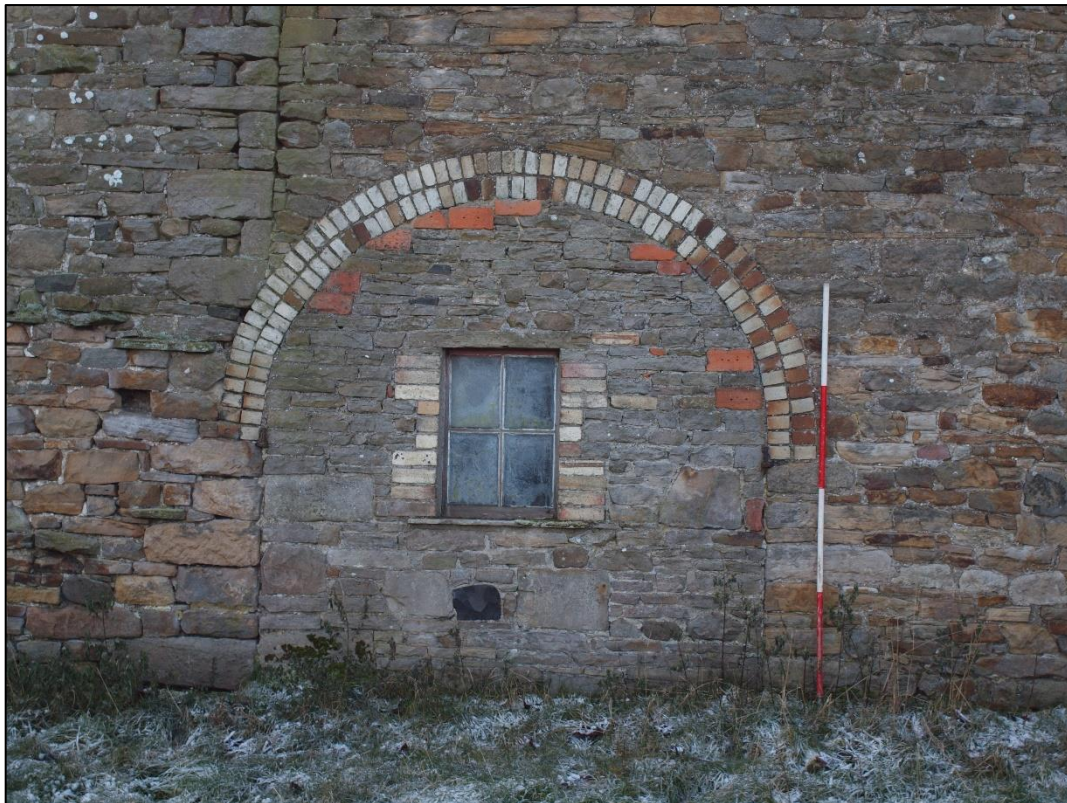
Plate 27: Blocked barn door with window inserted looking south
