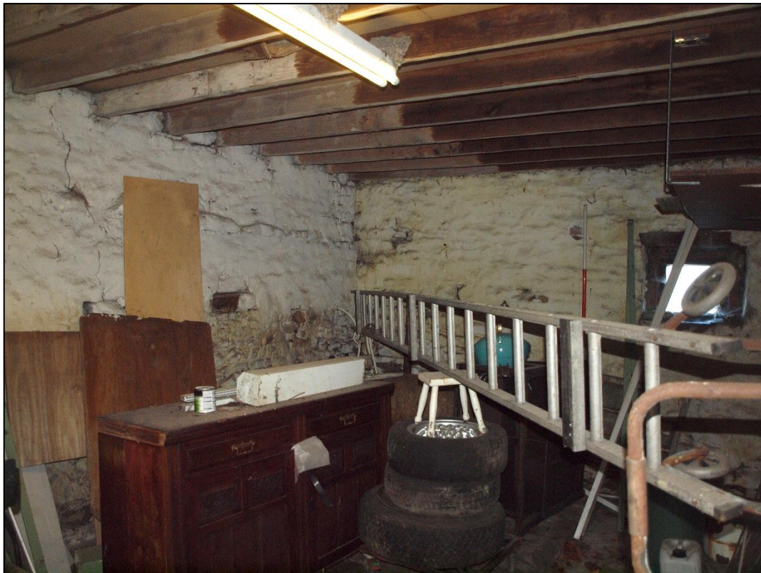
Plate 45: Room in bays 9 & 10 looking northwest
