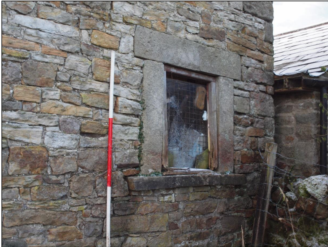
Plate 29: Window to bay 1 looking southwest
