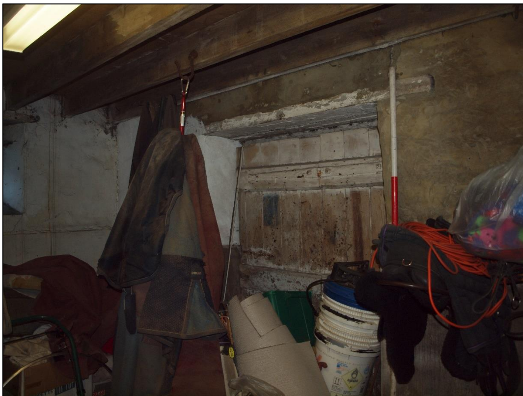
Plate 34: Room to bay 3 showing doorway in east wall looking northeast
