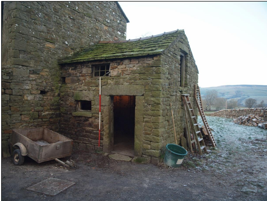
Plate 17: Bay 11 extension looking northwest
