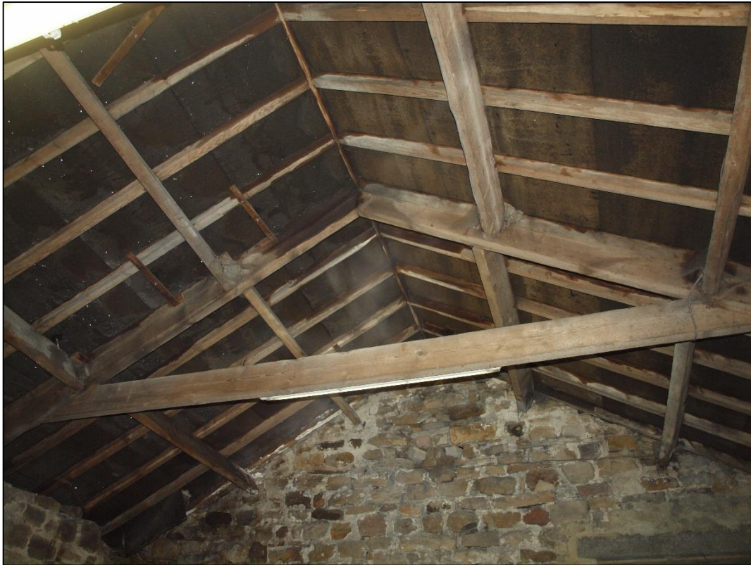
Plate 61: Detail of roof structure looking east
