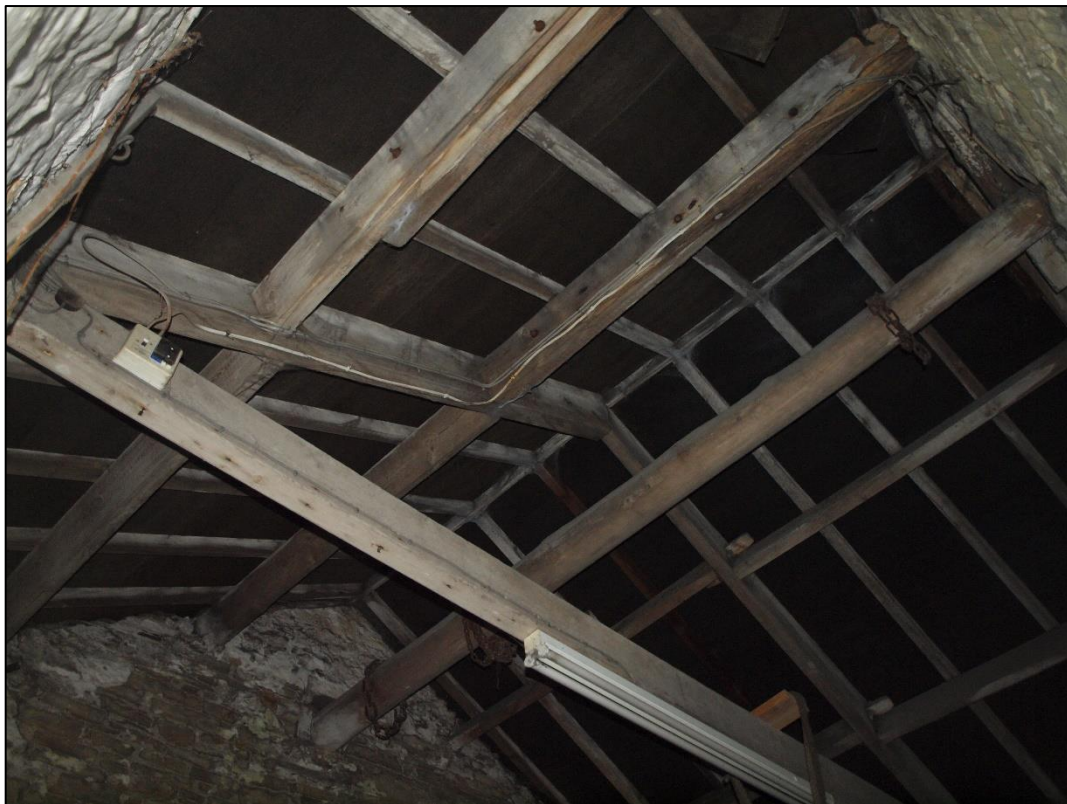
Plate 32: Details of roof structure looking northwest
