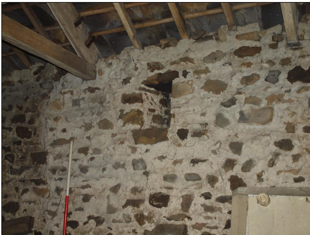
Plate 56: Ventilation slot in north wall looking northwest
