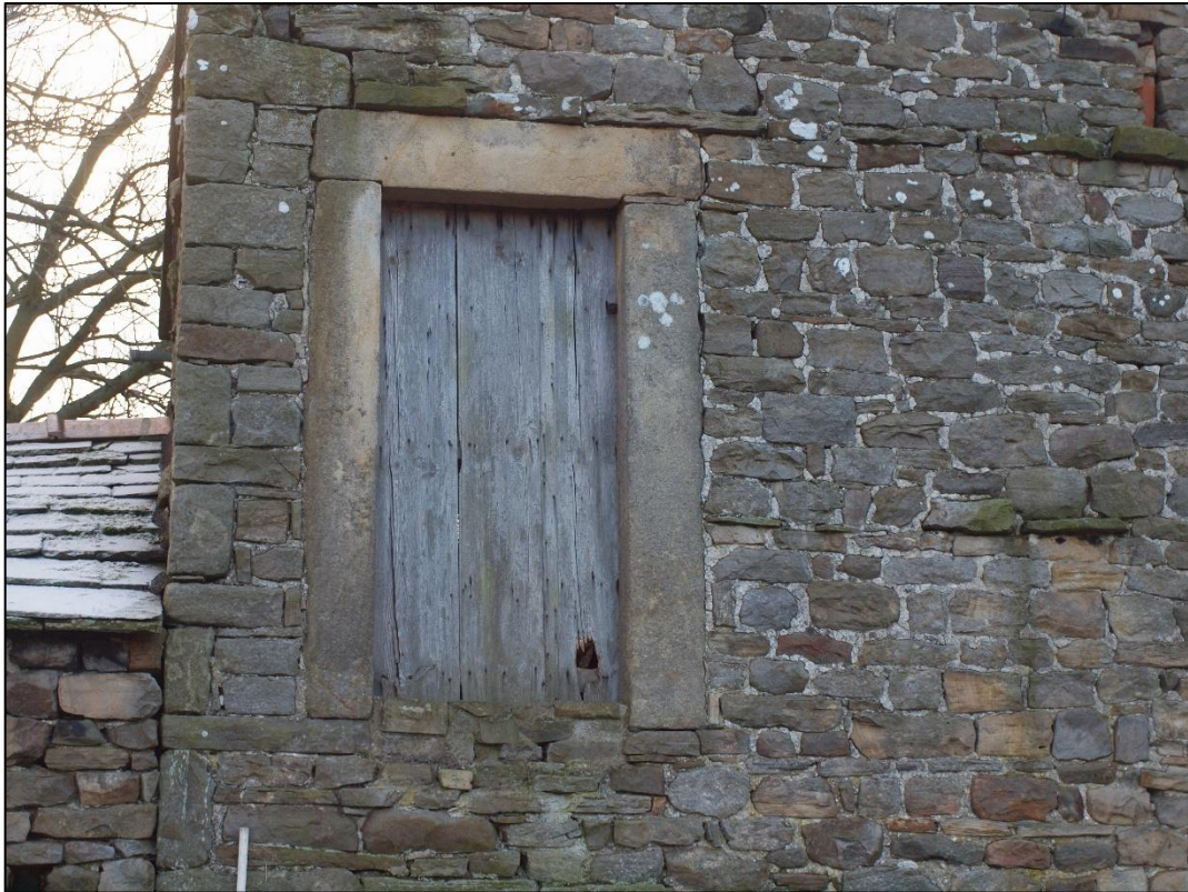
Plate 25: First floor doorway to bay 10 looking south
