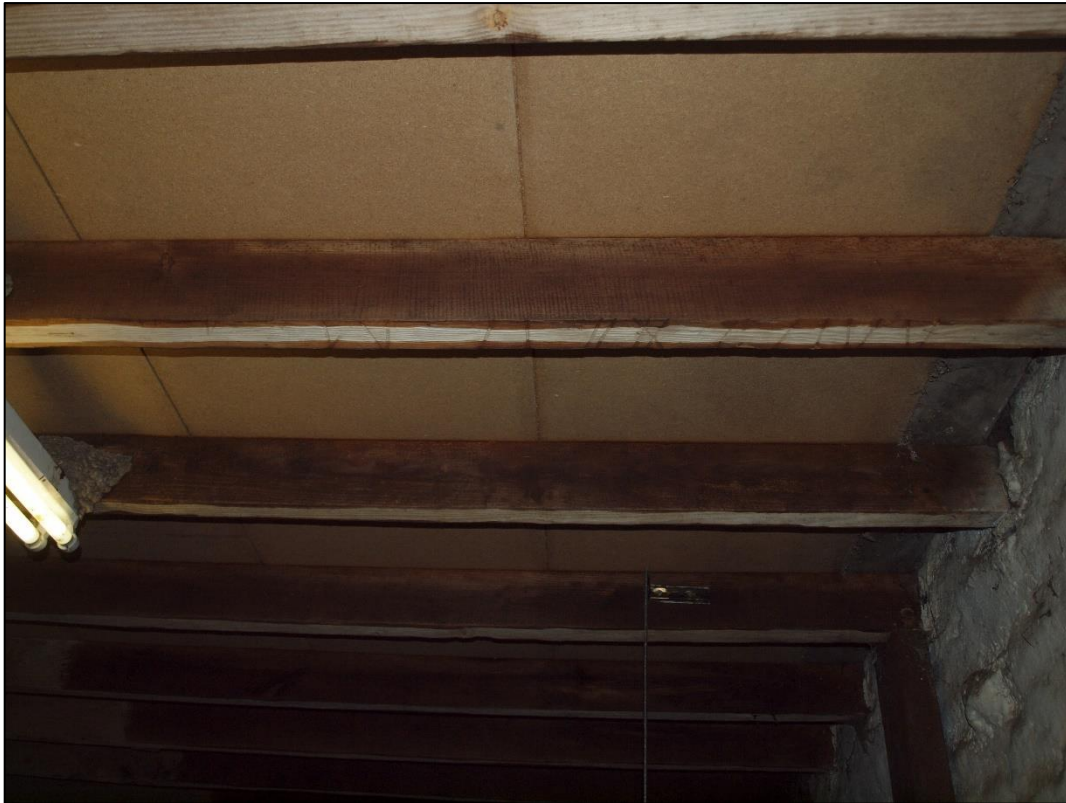
Plate 47: Modern ceiling looking south
