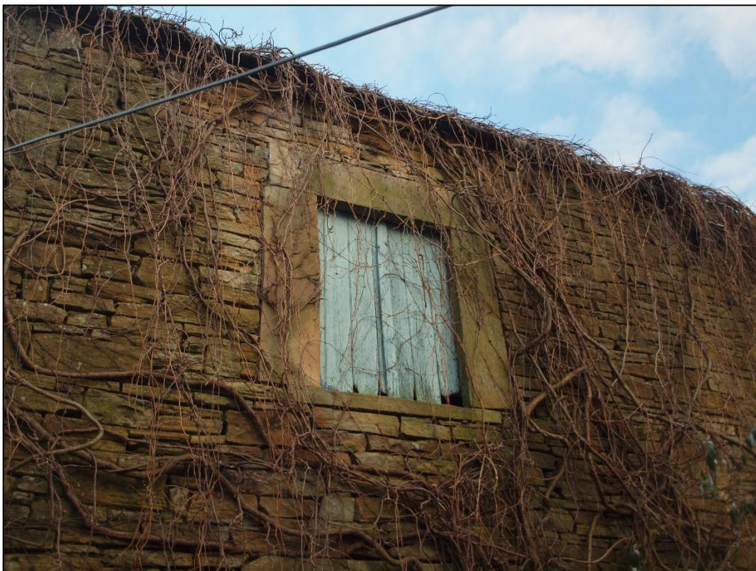
Plate 6: Pitching eye at first floor level, bay 3 looking northeast
