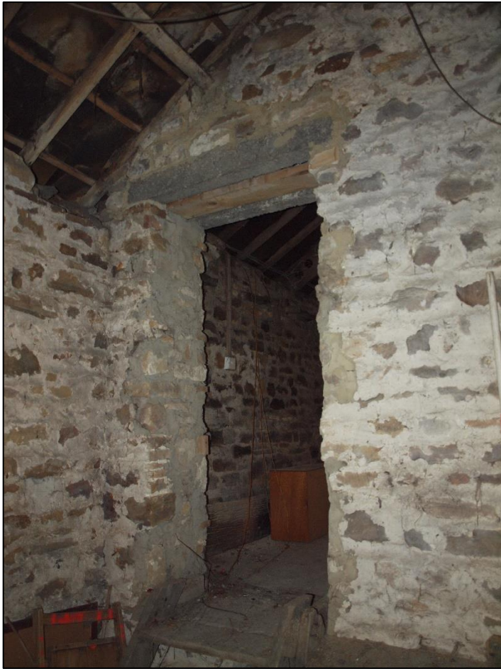
Plate 53: Detail of inserted doorway looking southwest
