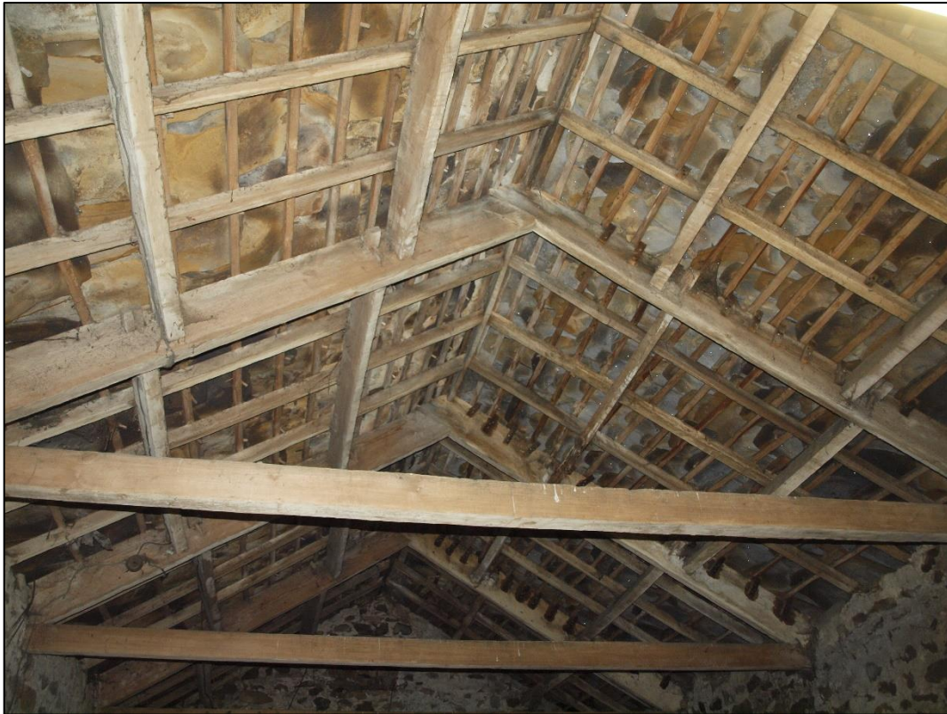
Plate 51: Truss detail looking west
