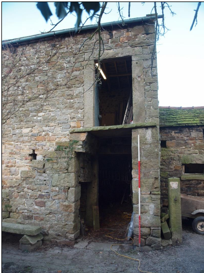
Plate 14: Bays 9 and 10 looking north
