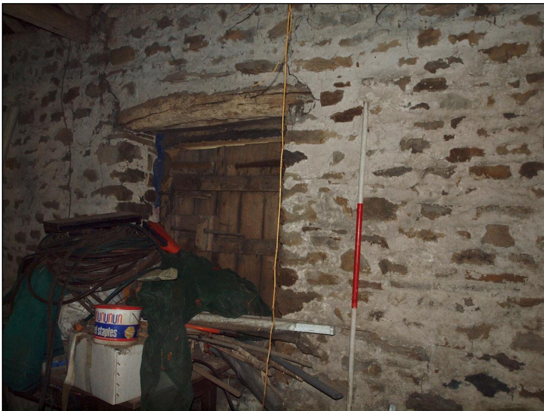
Plate 54: Pitching eye to south elevation looking south
