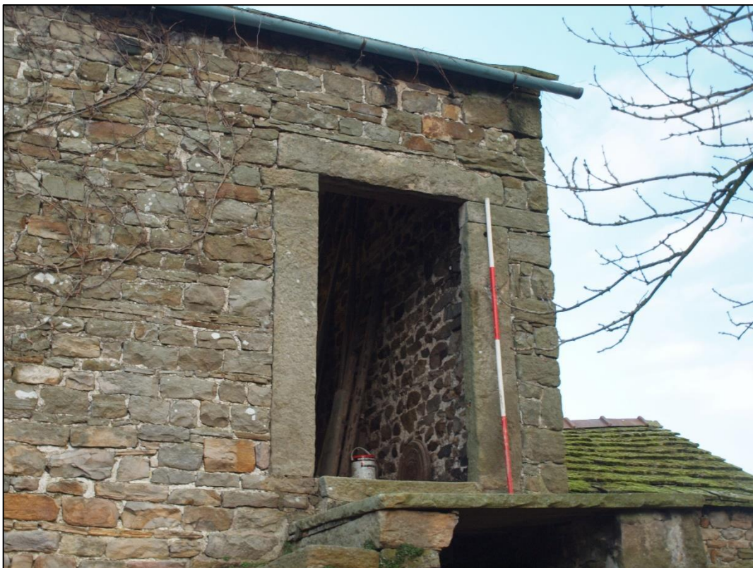
Plate 16: First floor doorway to bay 10 looking north
