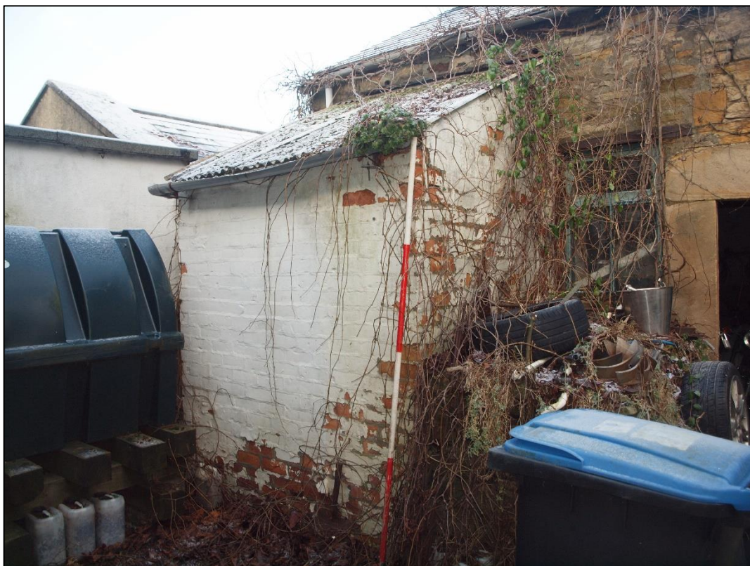
Plate 2: Brick lean-to to bay 1 looking northwest
