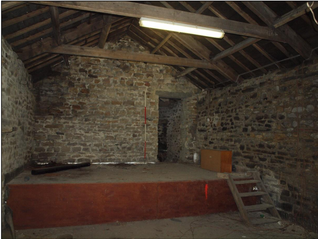
Plate 63: Former external west gable of barn with door inserted looking east
