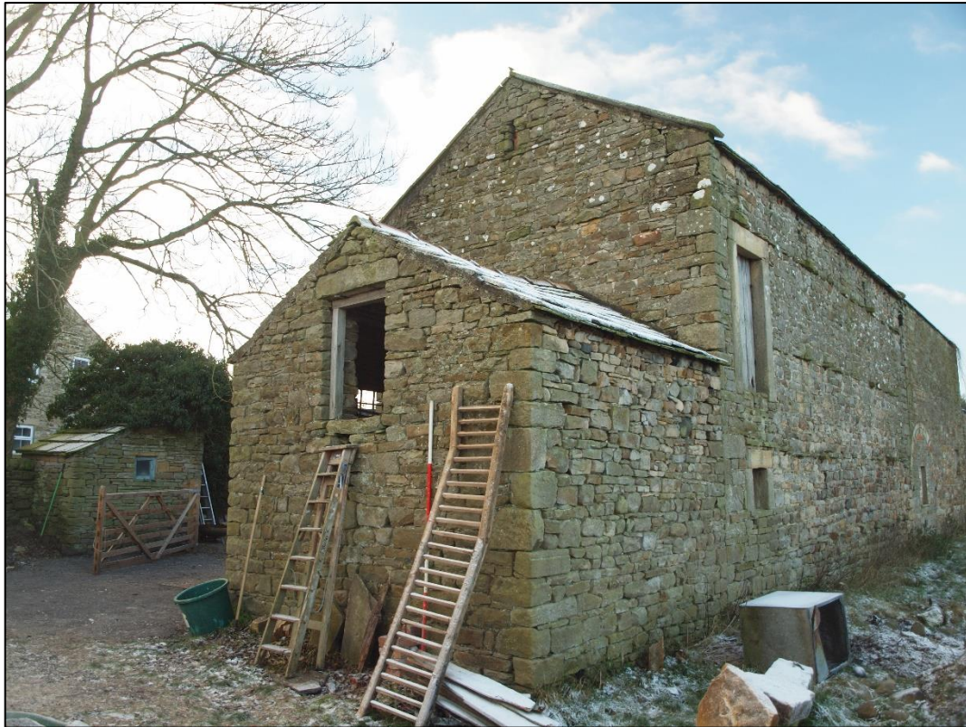
Plate 21: East gable looking west
