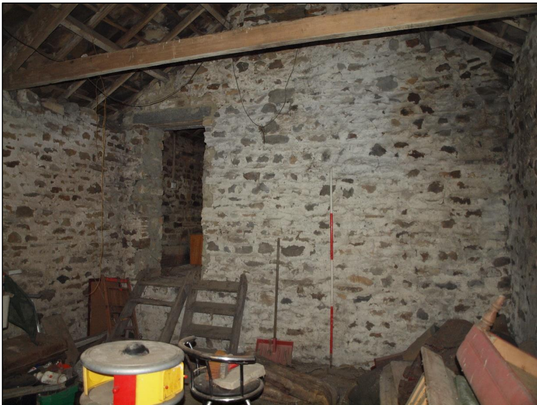
Plate 52: Internal cross wall of barn showing inserted doorway looking southwest
