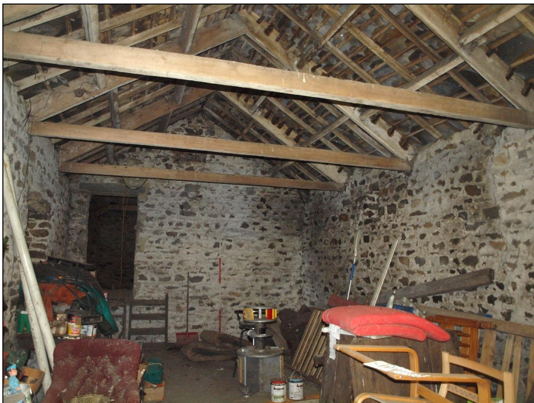
Plate 50: East end of first floor looking west
