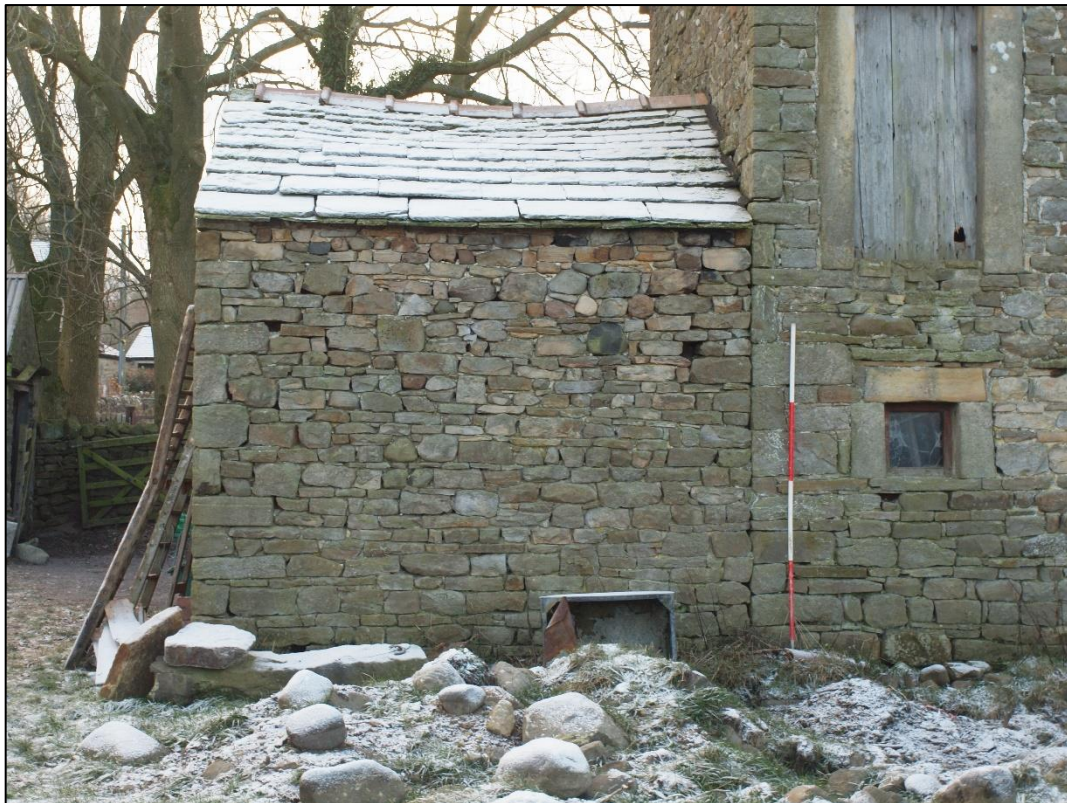
Plate 23: North elevation of eastern extension looking south
