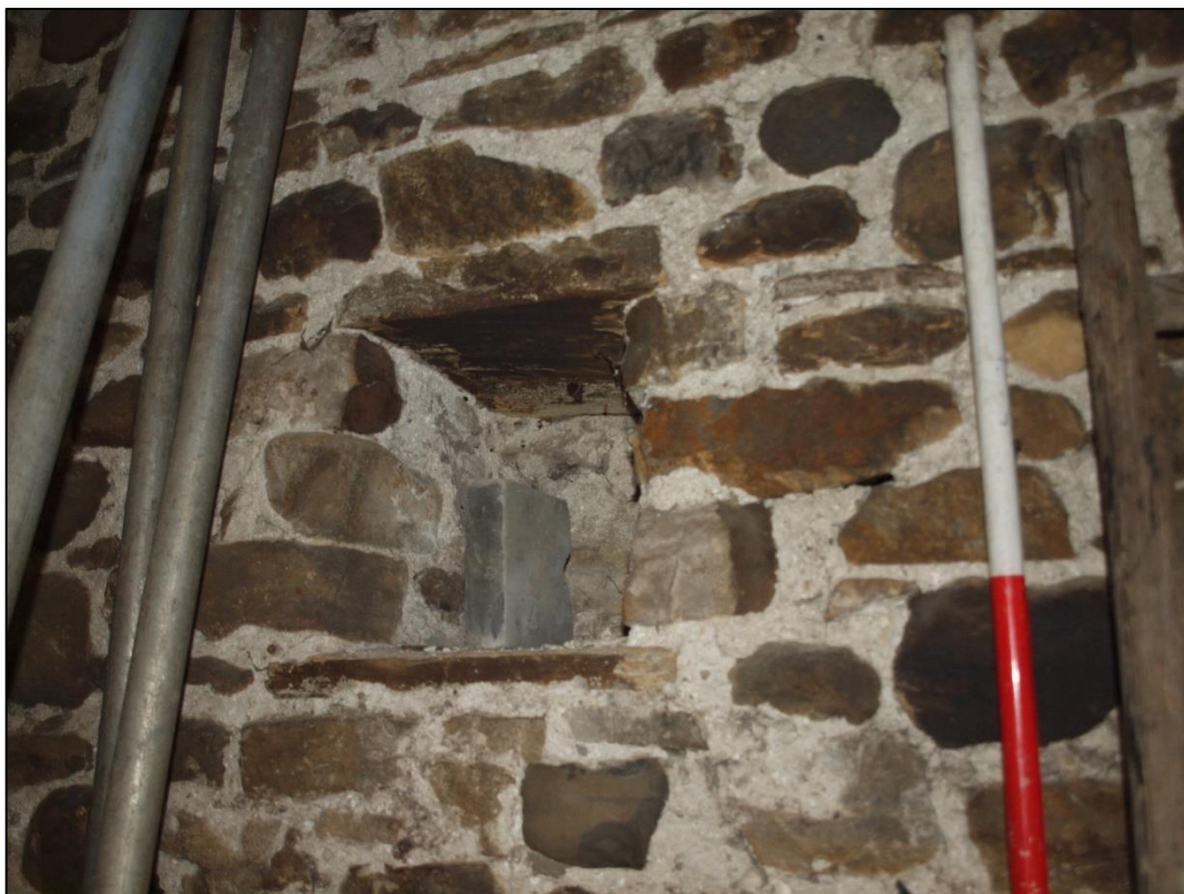
Plate 58: Niche in east wall looking east
