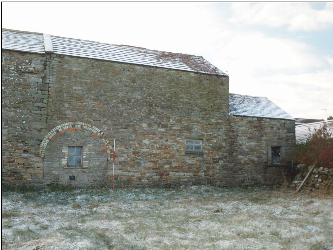
Plate 26: West end of elevation, bays 1 - 5 looking southwest
