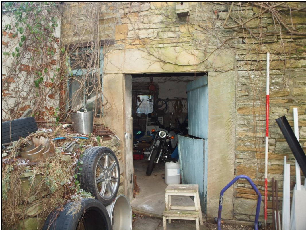
Plate 3: Doorway and window to bay 2 looking north
