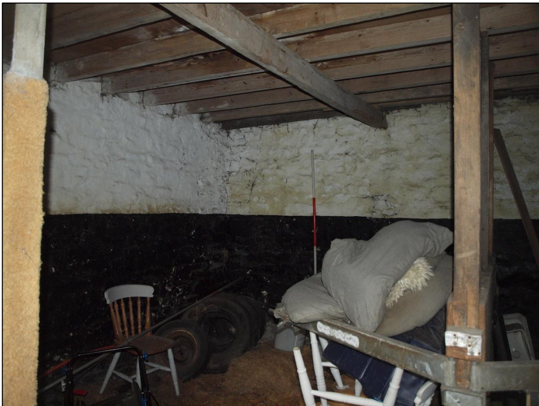
Plate 40: Eastern end of room in bays 6 – 8 looking northwest
