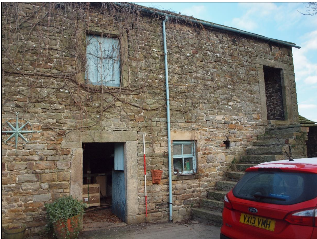
Plate 10: General shot of east end of barn showing bays 6 – 10 looking northeast
