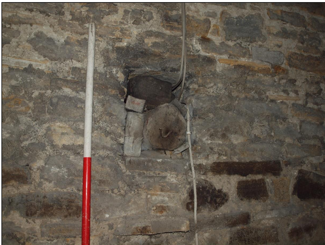
Plate 60: Ventilation slot in west gable
