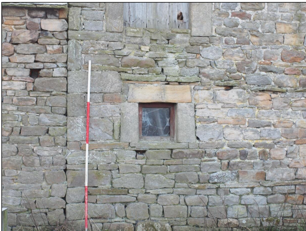
Plate 24: Ground floor window to bay 10 looking south
