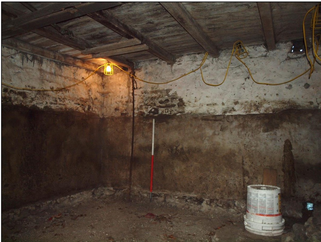
Plate 48: Interior of eastern gable extension looking northwest
