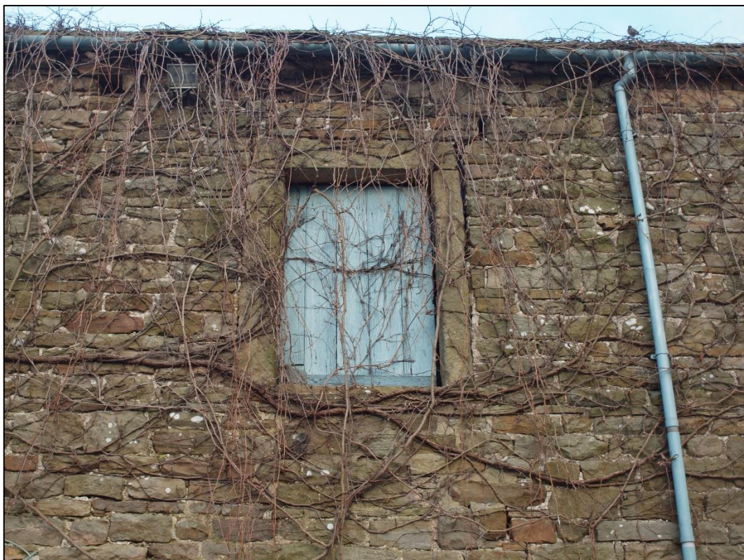
Plate 12: Pitching eye to first floor level in bay 7 looking north
