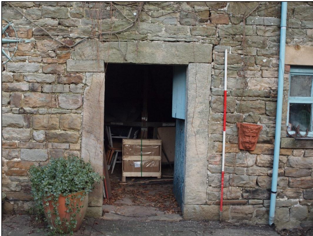
Plate 11: Doorway to bay 7 looking north
