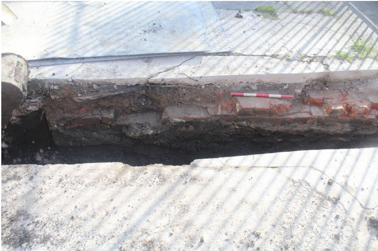
Fig. 7 View looking west of brick tank structure [25]; scale 0.5m
