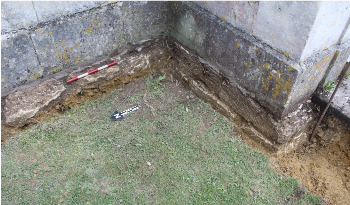
Fig. 3 View of nave [2] and porch foundations [3] looking southwest showing superstructure sitting directly on natural clay; scale 0.5m
