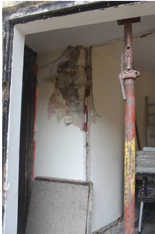
Fig. 18 Masonry corner of Community House (or predecessor) encapsulated within ground floor of Monument House; looking southeast, scale 0.5m
