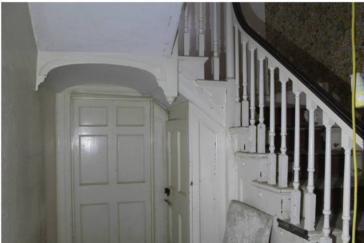
Fig. 21 Original panelling, doors, stair and banisters on ground floor stairwell of Monument House; looking east.
