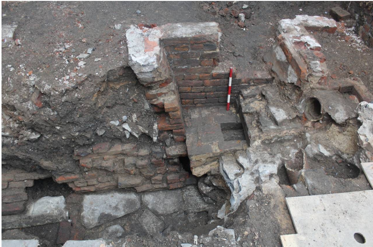
Fig. 5 Brick chamber [14], built against masonry foundation [29] and over brick vaulted culvert roof [31], looking southwest; scale 0.5m
