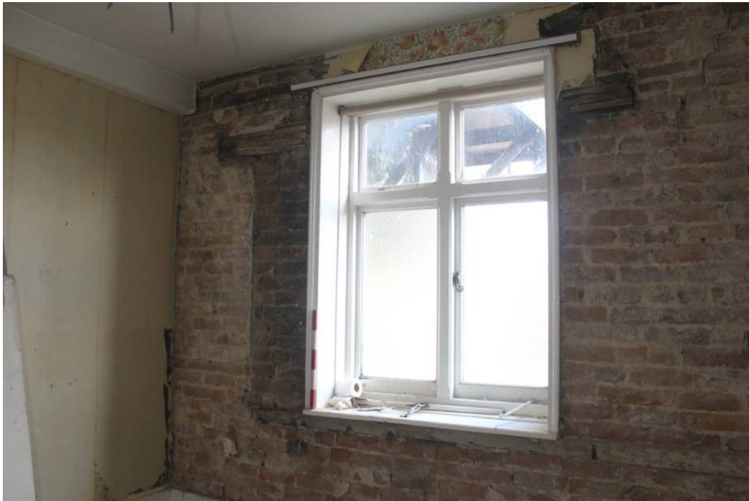
Fig. 28 Window alteration in north wall of Monument House, second floor, showing partial blocking of original window with insertion of enlarged window; looking north, scale 0.5m
