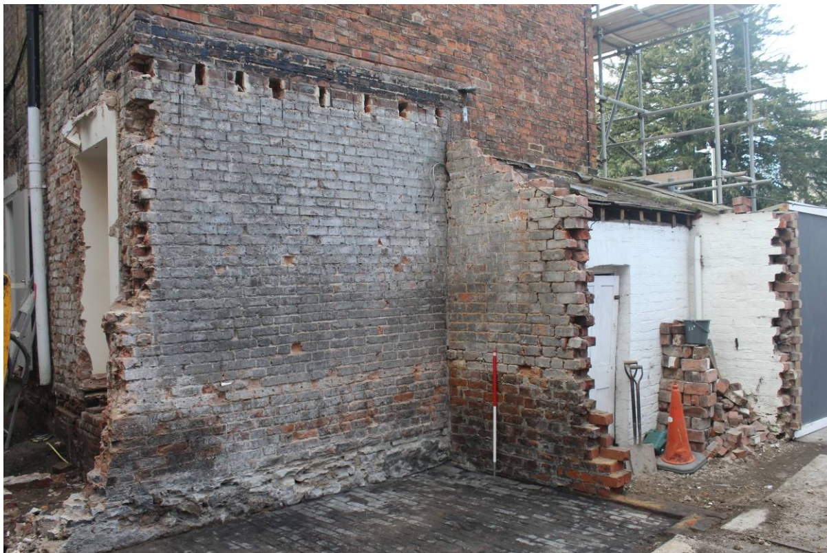
Fig. 15 Outbuilding to north of Monument House, with cavity brick wall [16], and brick floor [28], note stone foundation to Monument House superstructure [11], and superstructure extending east of building, looking southwest; scale 1m
