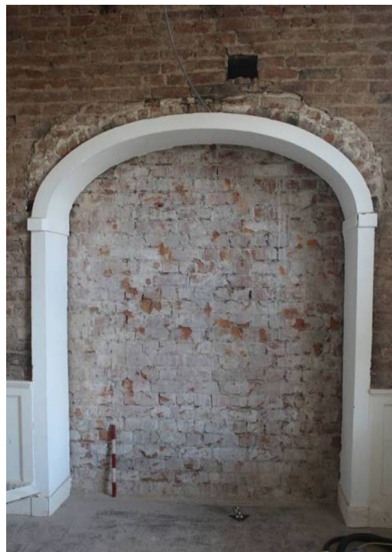
Fig. 25 South wall of Monument House, ground floor, showing inserted arched niche; looking south, scale 0.5m
