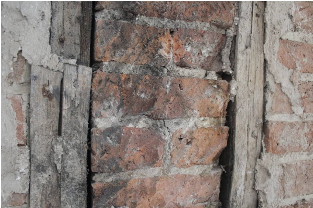
Fig.20 Axe marks on encapsulated brick wall within Monument House, ground floor.
