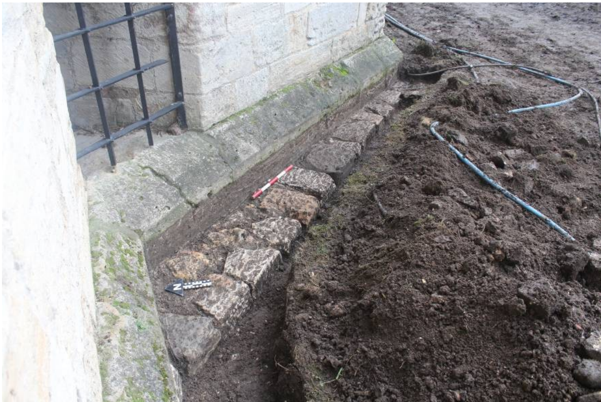
Fig. 4 View looking east showing the southeast Ambulatory chapel foundation [7]; 0.5m scale
