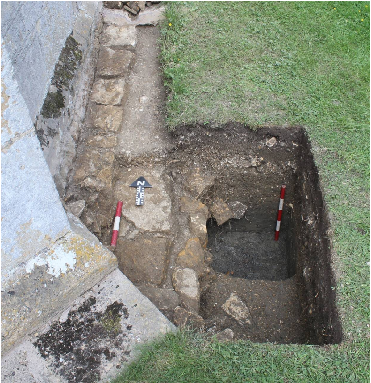
Fig. 5 Test Pit 1 showing foundation [6] sealed by layer (4) looking north; scales 0.3 and 0.5m
