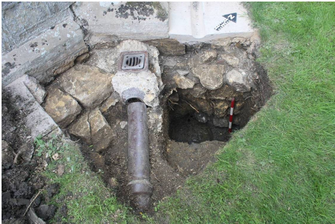
Fig. 9 Test Pit 1 showing foundation [18] looking northwest; scale 0.5m
