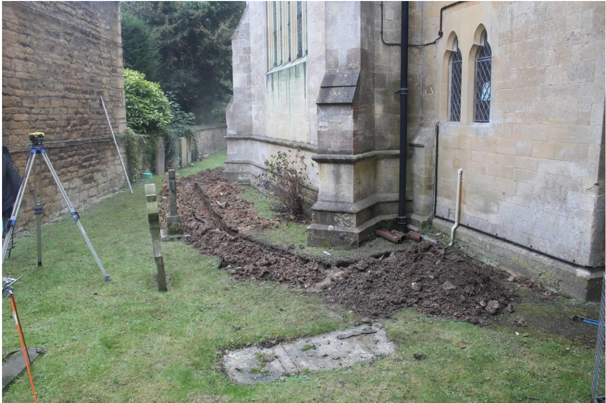
Fig. 3 The trench, looking south; scale 1m
