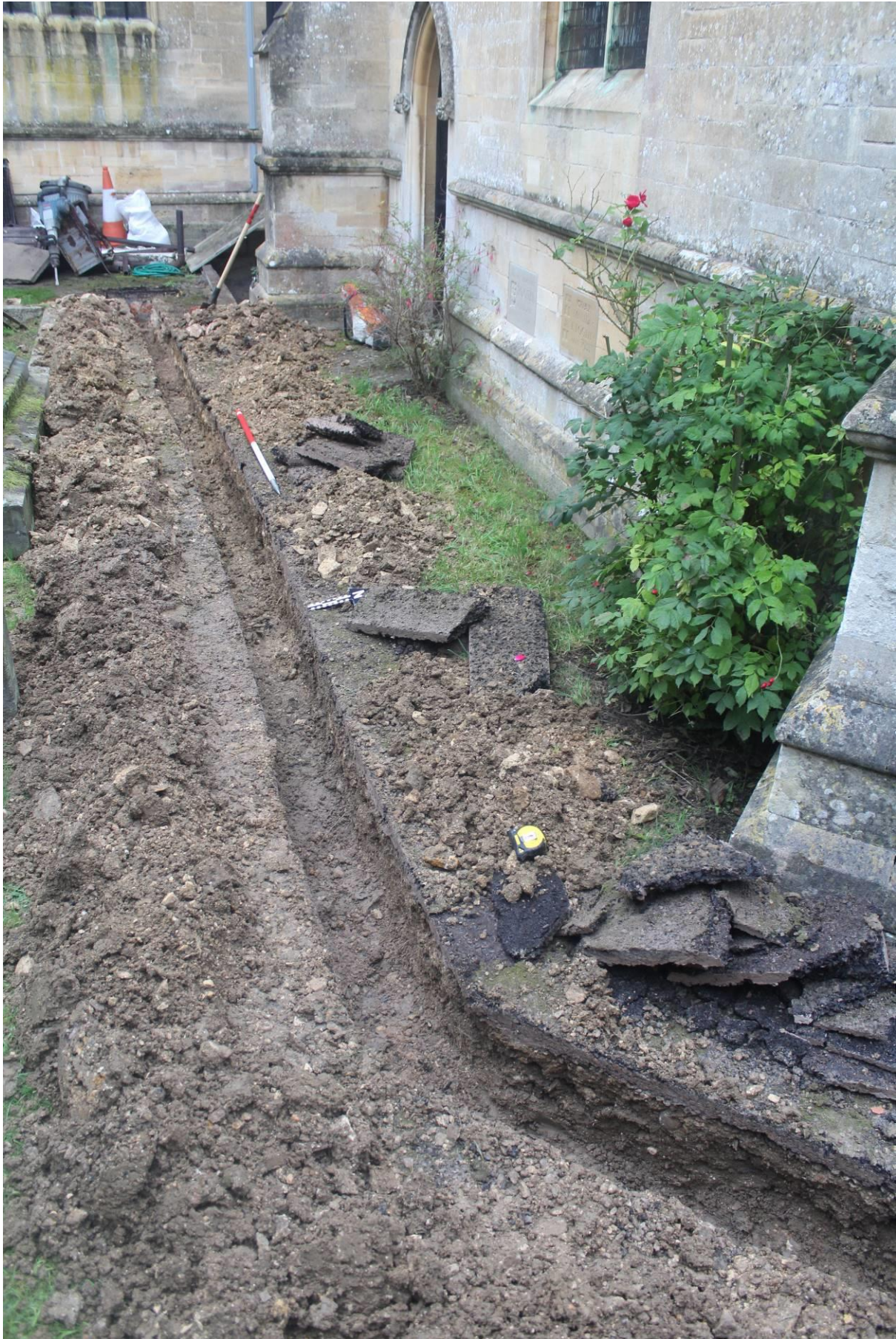
Fig. 5 The southern trench, looking west; scale 1m
