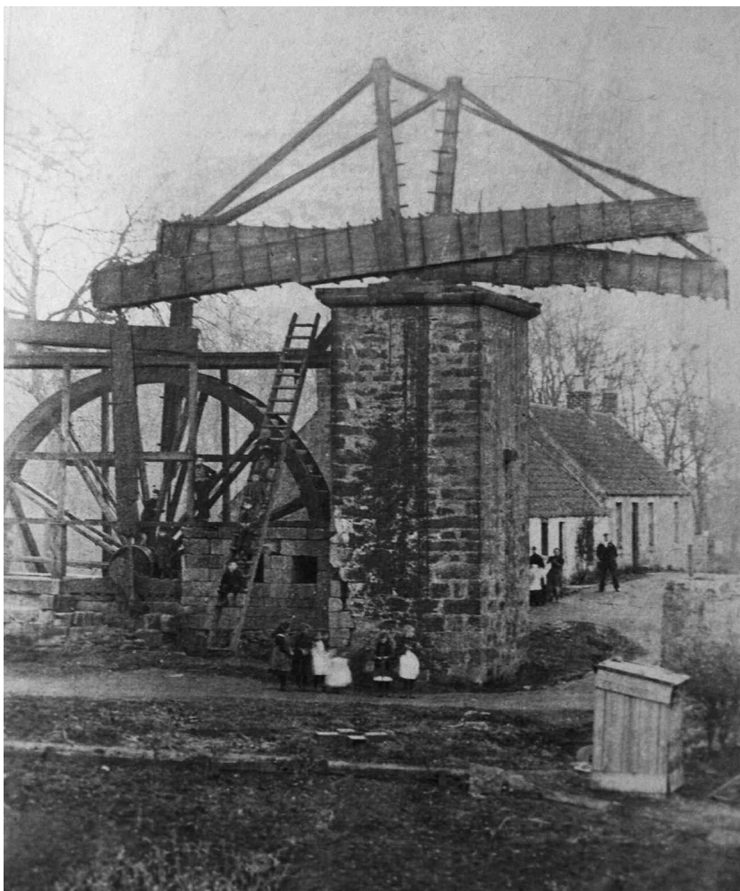
Figure 7. Water Powered Pumping Engine at the Old Watermill Pit (Photograph belonging to the late James and Isabella Snaddon, by kind permission of their granddaughter, Mrs Sadie Archibald.)
