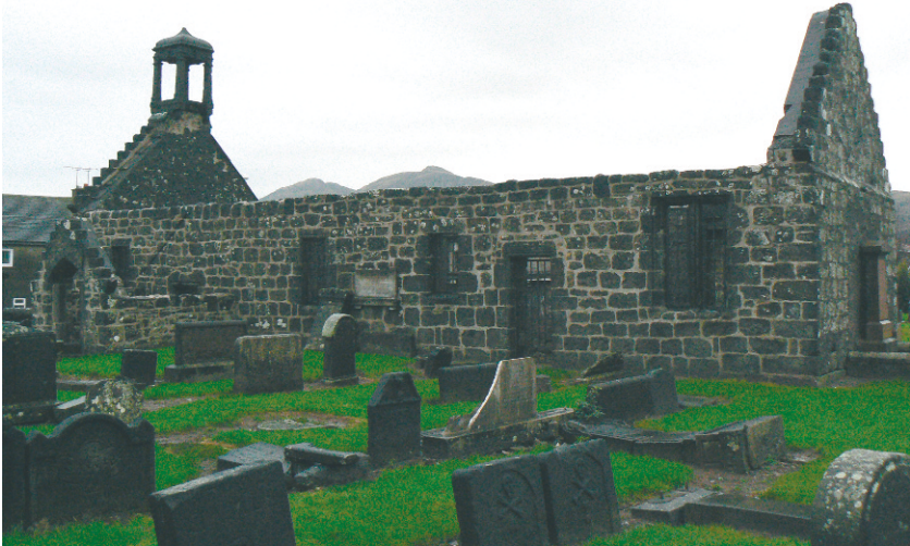
Plate 12. Tullibody Kirk – the parish was appropriated to the abbey in the thirteenth century and its income diverted to the uses of the canons, but this did not mean that they neglected the spiritual needs of the parishioners, Abbot Myln paying to have the church rebuilt in the 1530s to provide a suitable setting for parochial services.
