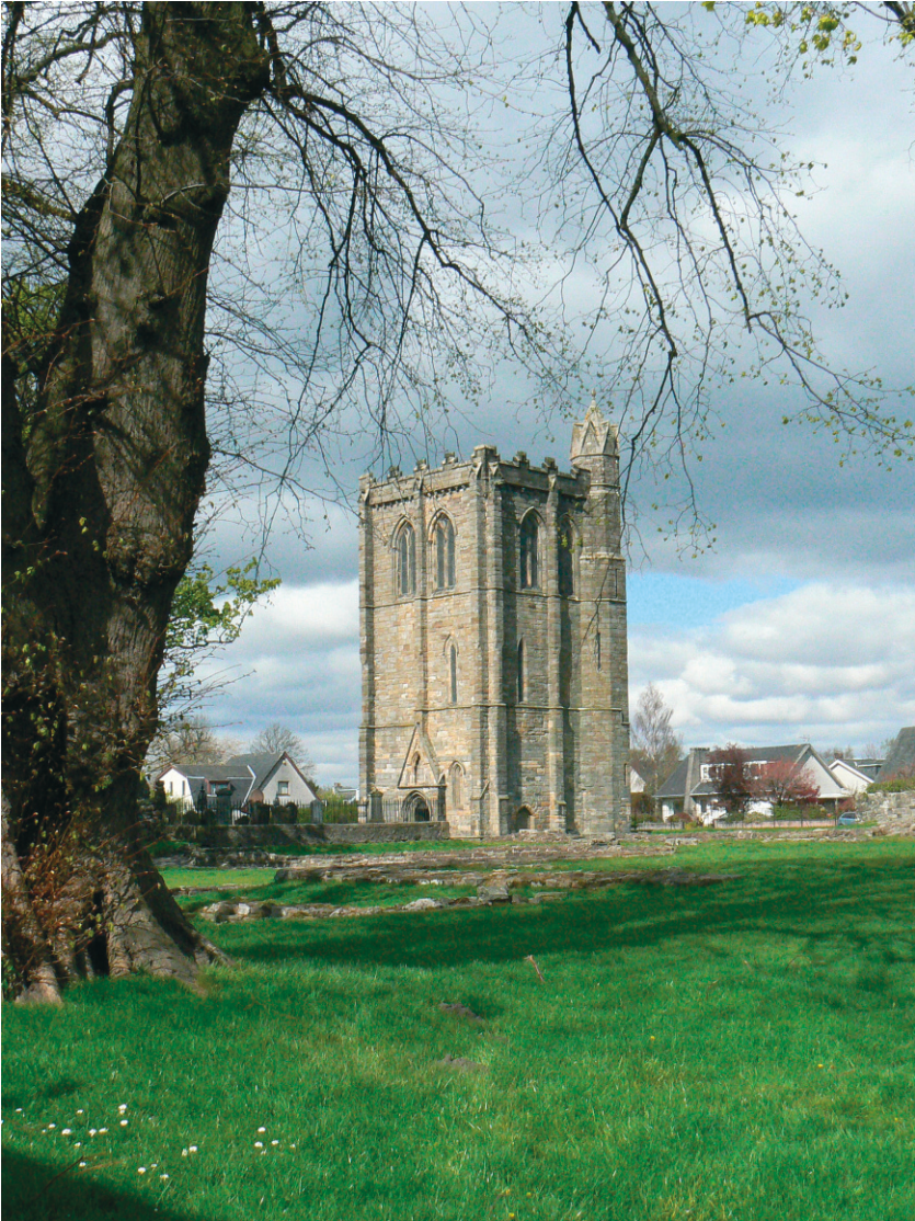
Plate 9. Cambuskenneth Abbey – little of the monastic complex remains above foundation level, but the detached thirteenth-century campanile survives to give an impression of the scale and quality of the buildings that were funded on the income from the monastic estate.
