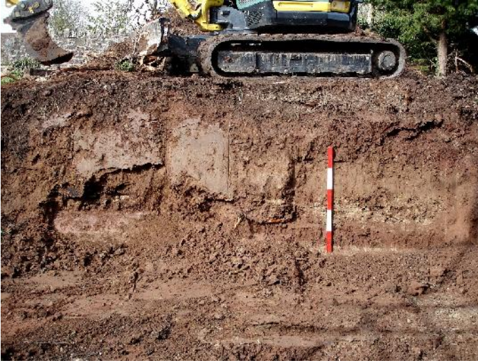
Plate 13 – Deep section through natural and overlying deposits, immediately to east of former pub garden revetment wall. The geology here consists of the Triassic Mercia Mudstone.
