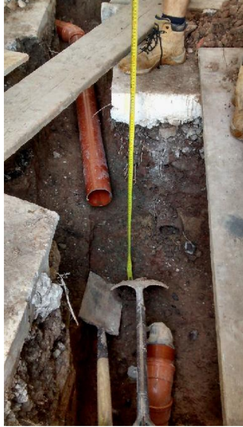
Plate 14 – One of the narrow service trenches that was monitored during the course of the watching brief, containing backfill, and heavily truncated and disturbed deposits.
