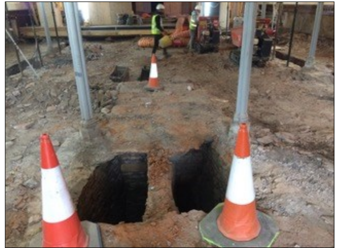
Plate 4: Two burial vaults directly underneath gallery supports, view east in the nave (photo courtesy of M. Nichols).
