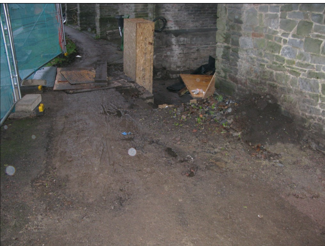
Plate 5: South side of Church where two ledger slabs removed prior to work to open south entrance.
