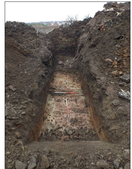
Plate 6: Looking north-east at Trench 3. 2 x 1m scales.
