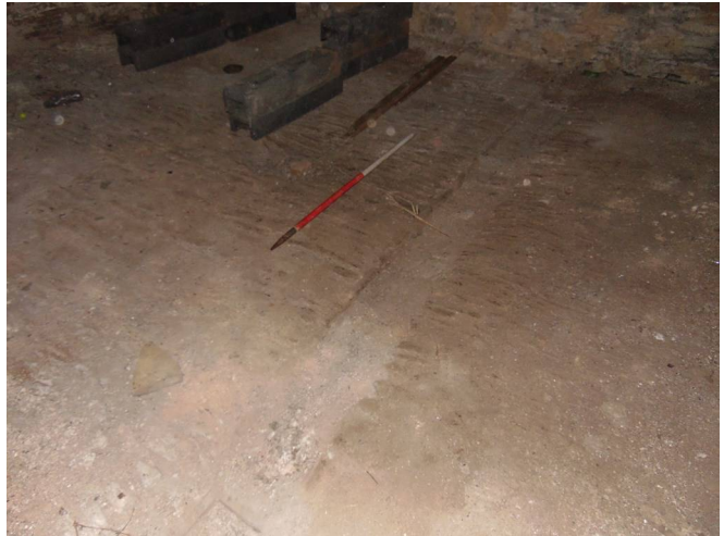
Plate 64: Looking north-east at cobble floor and drain in Barn A.
