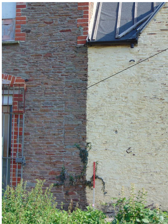
Plate 59: Detail of 17th century stub wall adjoining 19th century extension on south-west facing elevation.
