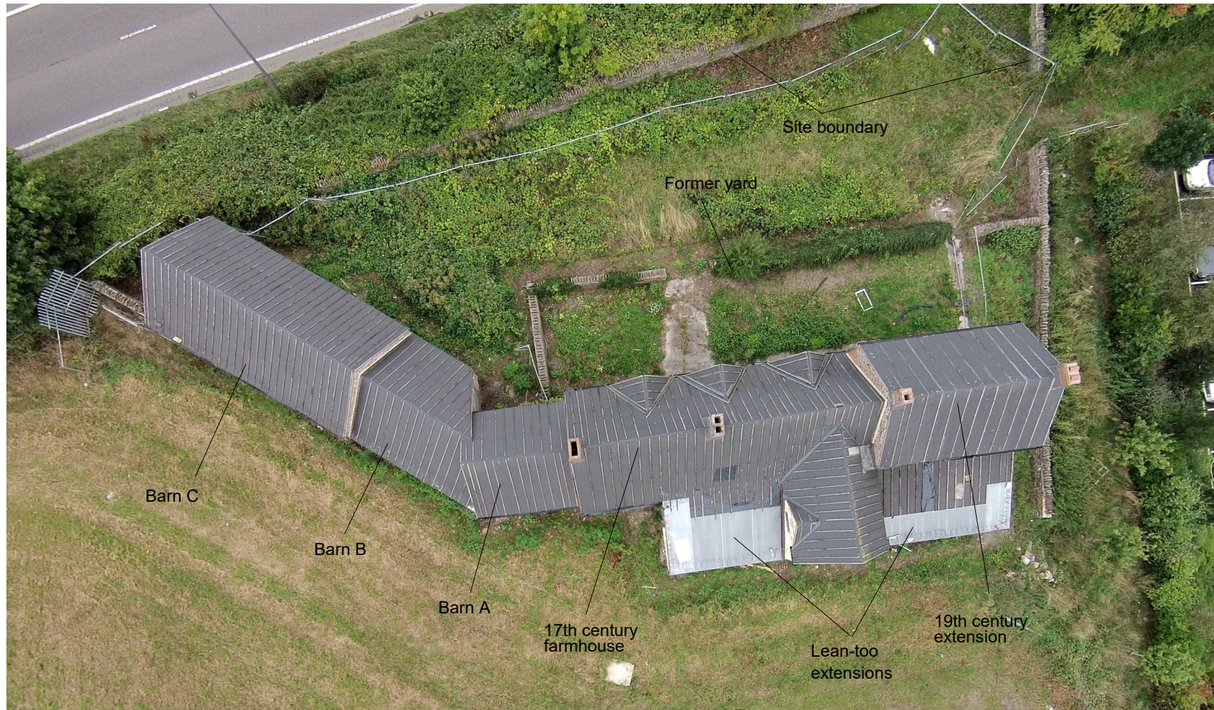
Plate 58: Drone image showing various structural elements of Newlands Farmhouse
