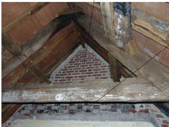
Modern brickwork
