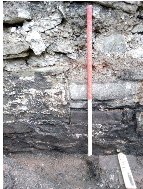
Plate 10. Detail of relationship between walls [121] and [122], looking north. 1m scale
