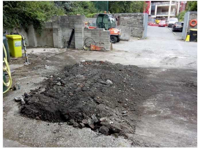
Plate 14. Post-excavation shot of Trench 1, looking north-east
