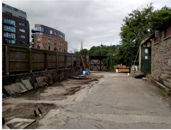
Plate 2. Pre-excavation shot of Trench 2, looking west
