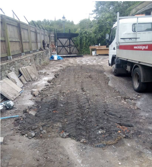
Plate 15. Post-excavation shot of Trench 2, looking west
