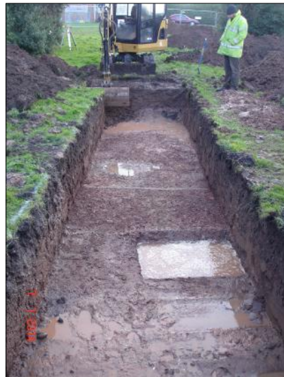
Plate 10. Looking south at Trench 5 during machine excavation.
