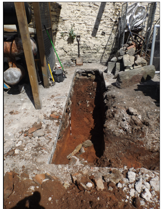
Plate 4. General view of trench once excavated to the required depth.
