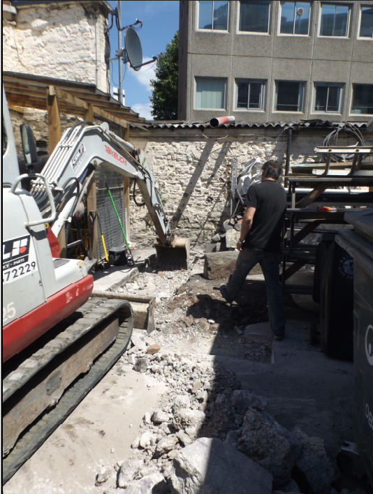
Plate 1. View of trench looking north east before excavation.
