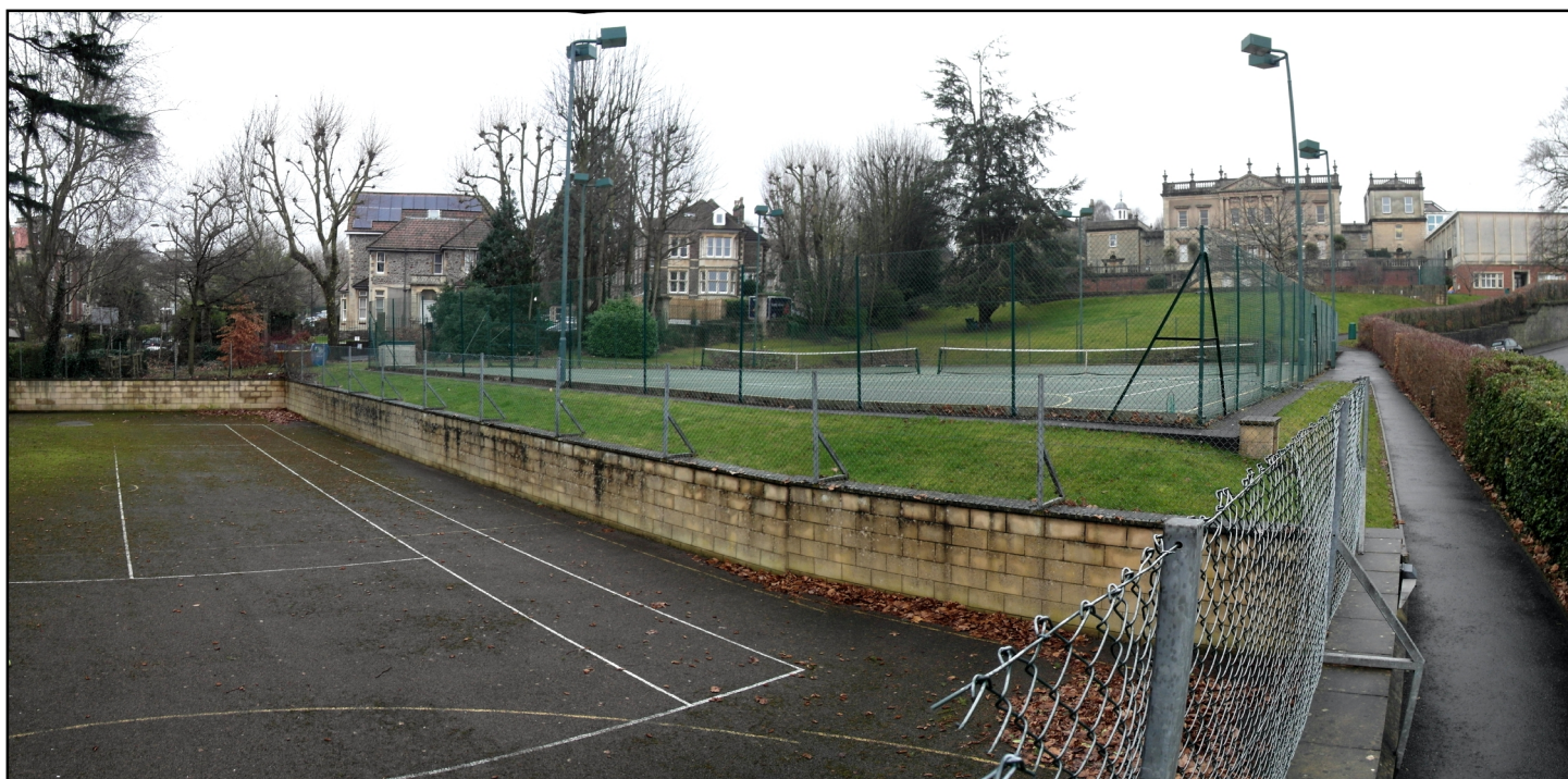
5. Composite panoramic view of the site from the eastern side of the lower tennis court, looking west and north-westwards. The construction of both of this court and the one immediately beyond it to the north, clearly entailed a degree of terracing, and therefore disturbance of the original slope profile. It is intended to remove the courts, and to construct on their site six new houses, in two blocks of three on the former area of each court. This image was taken from very roughly the position of the walled, ornamental circular raised planting bed that is shown intermittently on historic maps from 1811 onwards, as lying just inside the southern gated entrance to the original park.
