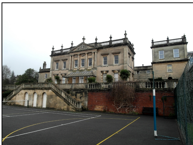
3. Southern elevation of the Palladian house, from the upper tennis court. On the right, the original, 18th century parapet of the eastern pavilion wing was truncated in the late 19th century so that an additional storey could be added for teacher accommodation. This gives a good impression of the degree of terracing that has taken place to accommodate the house, and there is a suggestion that at least a part of it may have been undertaken for the 16th century house on the site. It is intended that the area of the tennis court itself will be incorporated in the new communal gardens. View to north-west.
