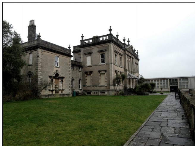
2. The main, south-facing elevation of John Cossins's Palladian house. The western pavilion wing, closest to the camera, its access corridor, and its counterpart on the eastern side of the house, were later additions of the 1740s. It is intended that the modern sports hall in the background should be removed and its site turned over to communal gardens. View to north-east.
